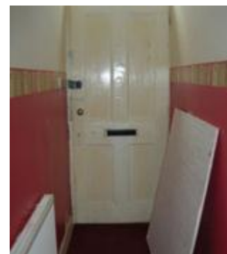
Fig 6: Interior side of front door prior to application of aerogel board
