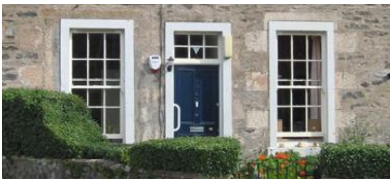
Fig 5: Windows and door upgraded, with secondary glazing and aerogel board applied to door panels
