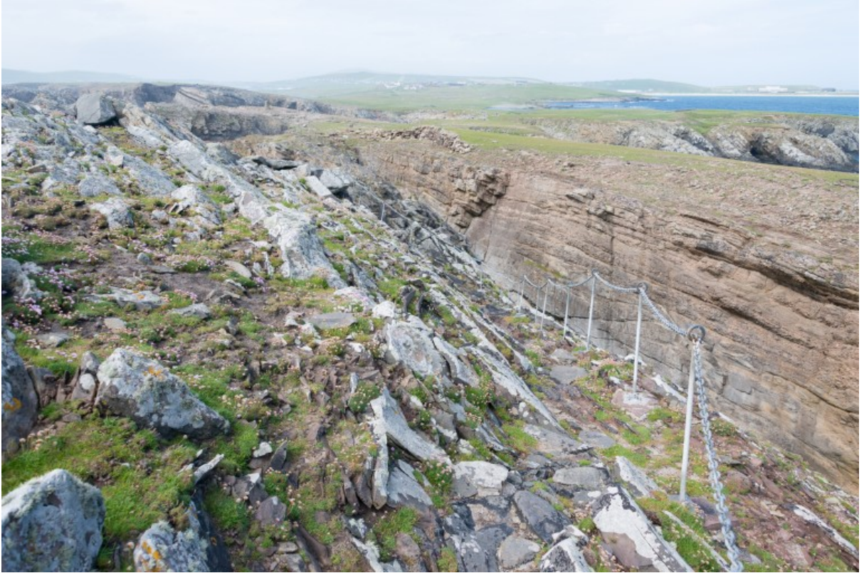
View of approach to site showing rock ridge and safety rail fixing:
