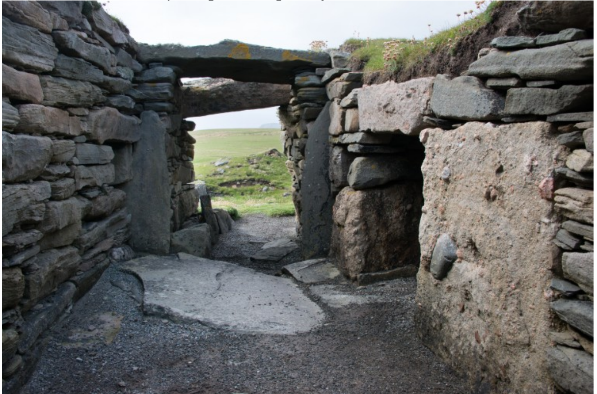
Interior view of entrance passage showing door jambs:
