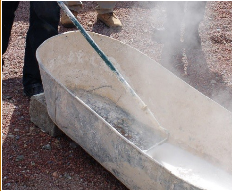
Fig. 1 Slaking quicklime to produce lime putty.
