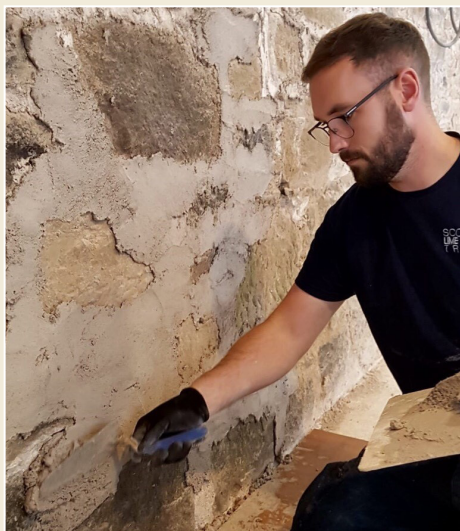
Fig. 8 A wall being 'dubbed out.' (Photo credit: Scottish Lime Centre Trust)
