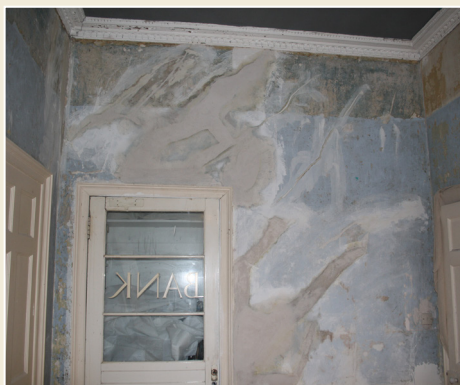
Fig. 15 Finishing coat applied to patch repairs. (photo credit: Darren McLean)
