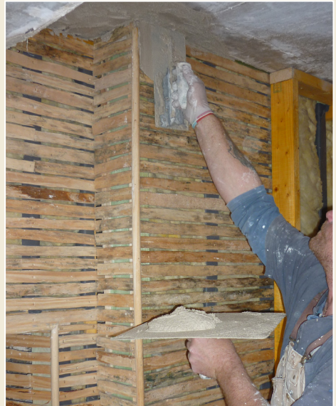
Fig. 7 Timber laths ready for application of first coat.
