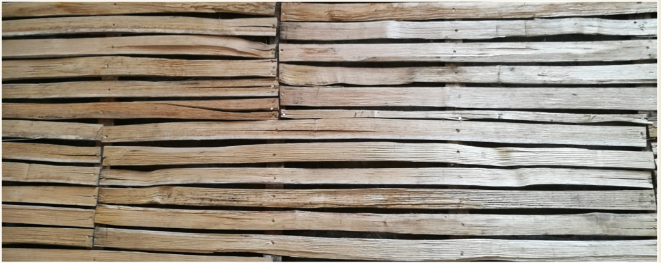
Fig. 6 New riven lath butt jointed and staggered.
