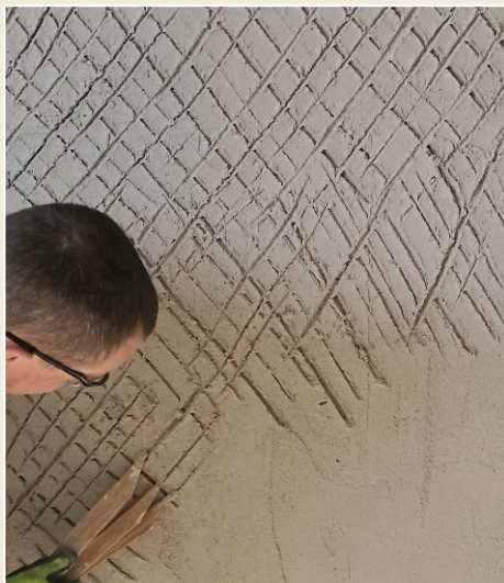
Fig. 10 Scratching first coat plaster with a lath scratch.
