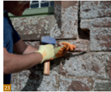
Fig. 23 Raking out old decayed mortar.
