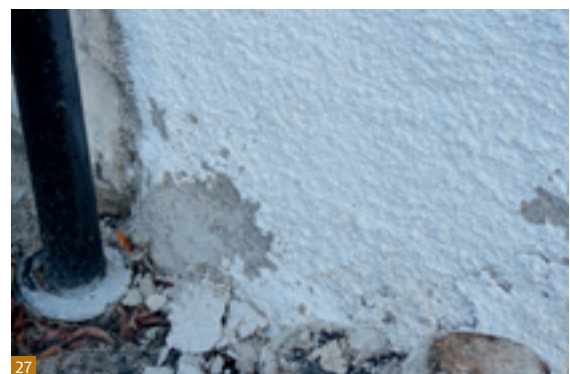
Fig. 27 Frost damage to lime harling.
