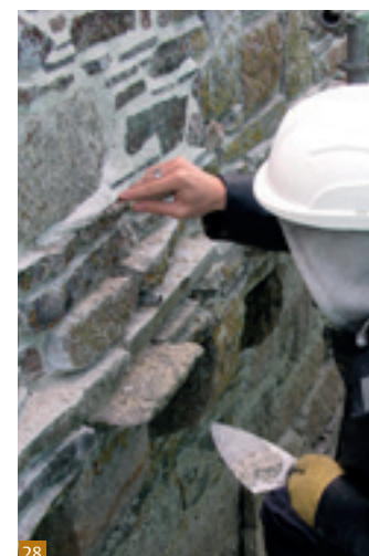
Fig. 28 Repointing rubble masonry.
