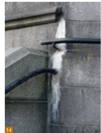
Fig. 14 Example of streaking caused by excess free lime content on the lime mortar.
