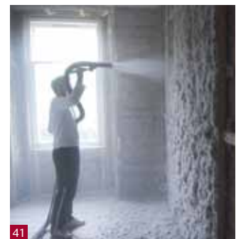
Fig 39 Hemp fibre insulation with clay board.
