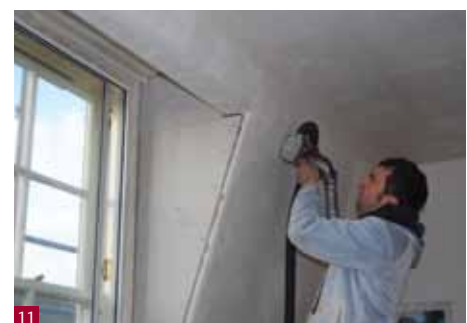
Fig 11 Blowing in bonded bead insulation to a coom.
