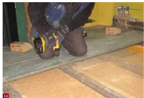
Fig 14 Floor boards being re-fixed following insulation.
