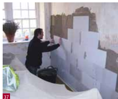
Fig 37 Application of the insulating boards.
