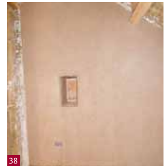
Fig 38 Insulated lime plaster prior to limewashing. Image by Eden Lime.
