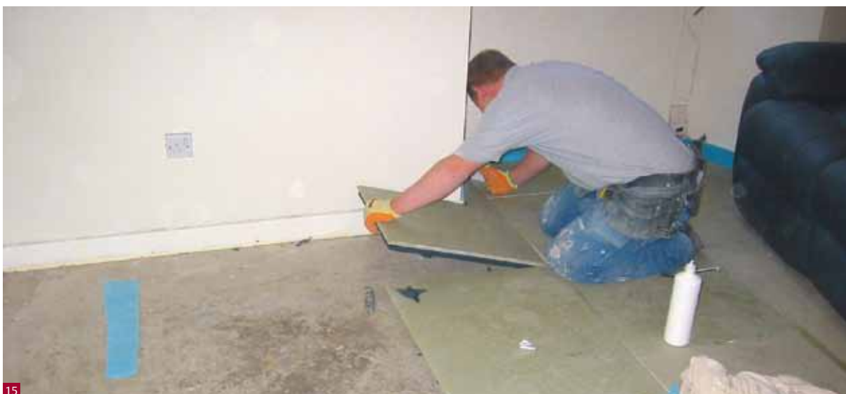
Fig 15 Aerogel board being laid onto a concrete floor. Image by Changeworks.
