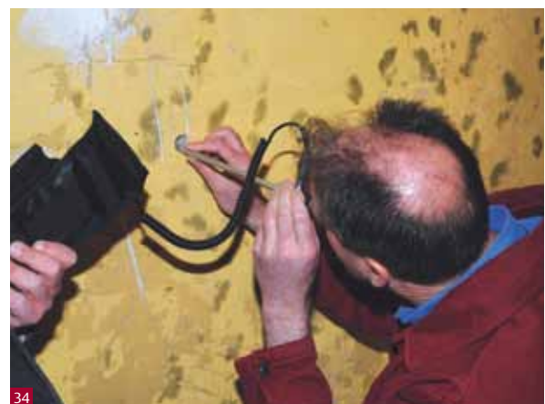
Fig 34 Inspecting the void with a borescope during the insulation process.
