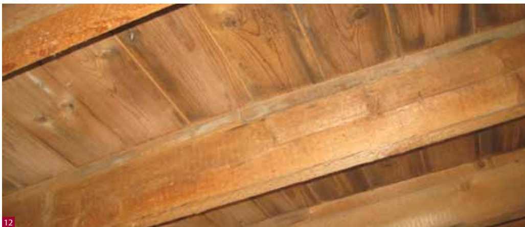
Fig 12 A typical underside of a flat roof.
