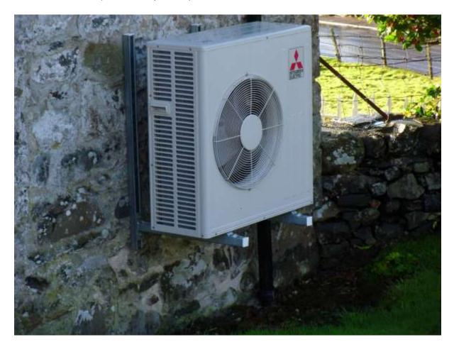
Fig. 8: The external fan unit of the ASHP on the NW corner of the church
