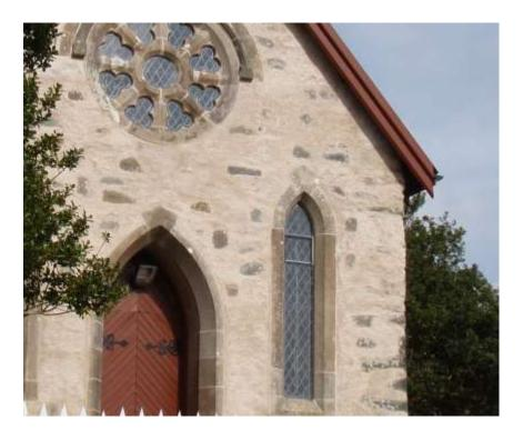
Fig. 2: Detail of the lime pointing on the west gable; this resulted in much drier masonry
