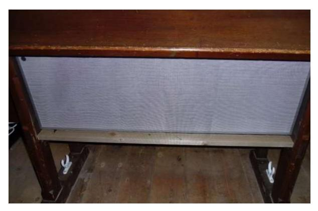
Fig. 5: The new pew backed radiant panels
