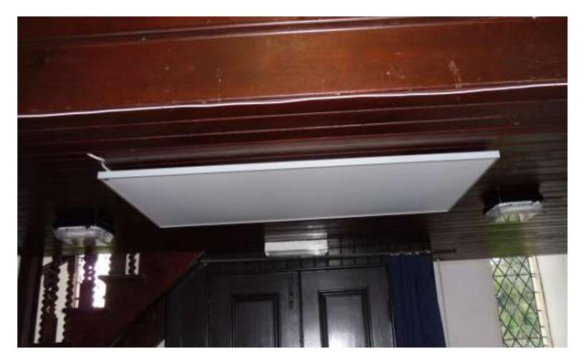
Fig. 6: The radiant panels underneath the mezzanine layer
