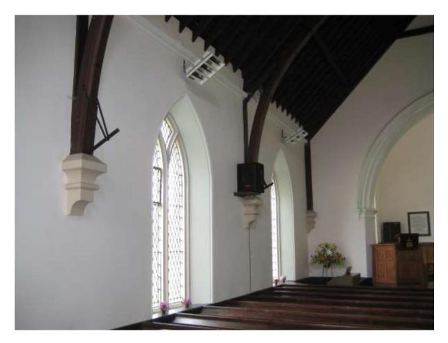
Fig. 3: Hobkirk Church in the Scottish Borders is heated by radiant panels at cornice level
