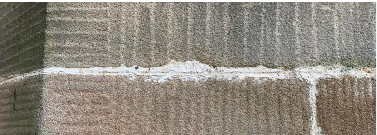
Figure 117.4. Ashlar masonry, with fine pointing, lined out.
