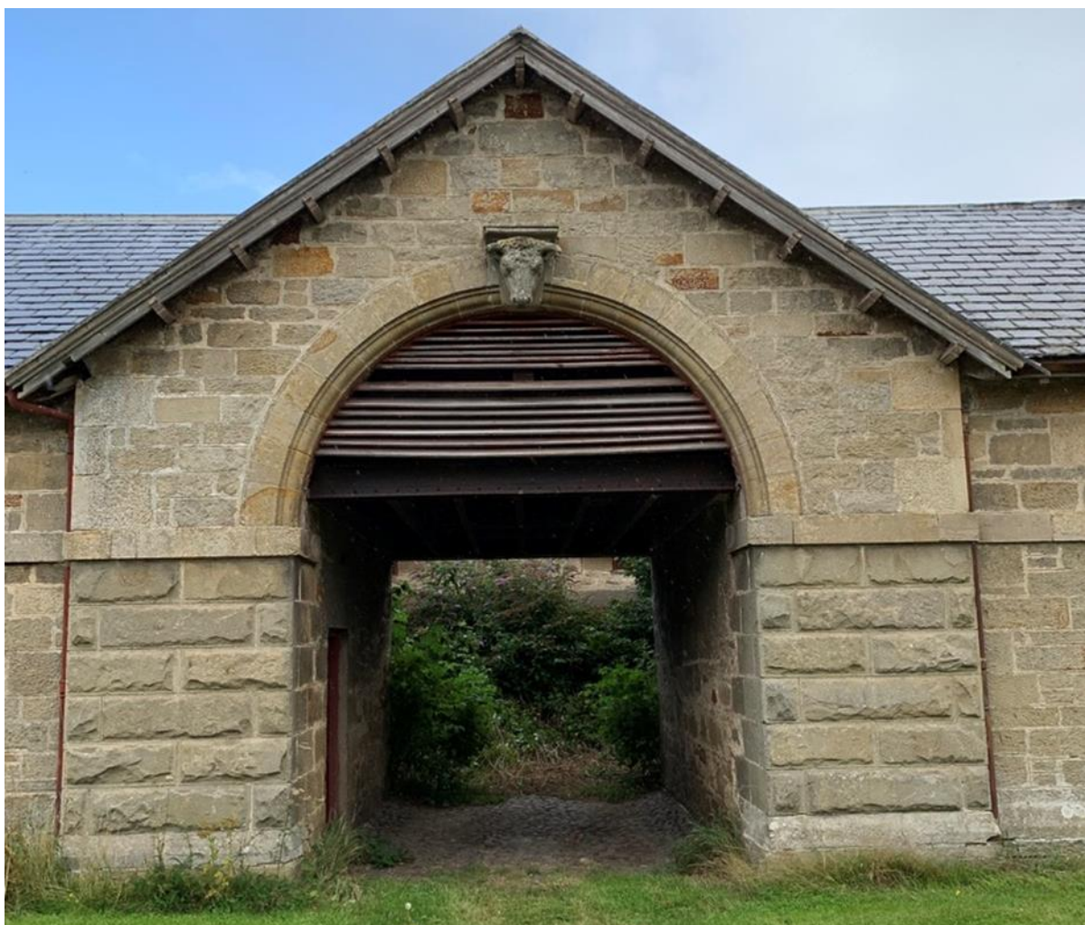
Figure 100.1. The main steading complex facing Kinloss House. Rusticated ashlar blocks containing semi-coursed, sawn-squared blocks of sandstone.
