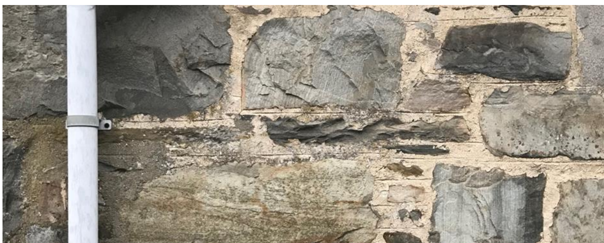
Figure 066.2. The crude flush and informal lining out finish.
