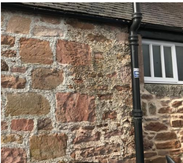
Figure 051.2. Three samples of pointing: 1 (left) recent lime mortar sneck harl; 2 (middle) original sample; 3 (right) earlier re-pointing.
