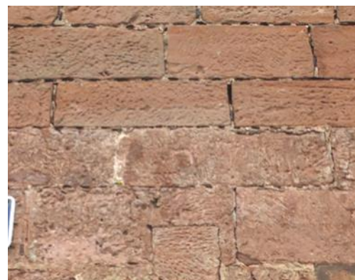
Figure 019.3. Some of the joints are filled with sandstone chips.
