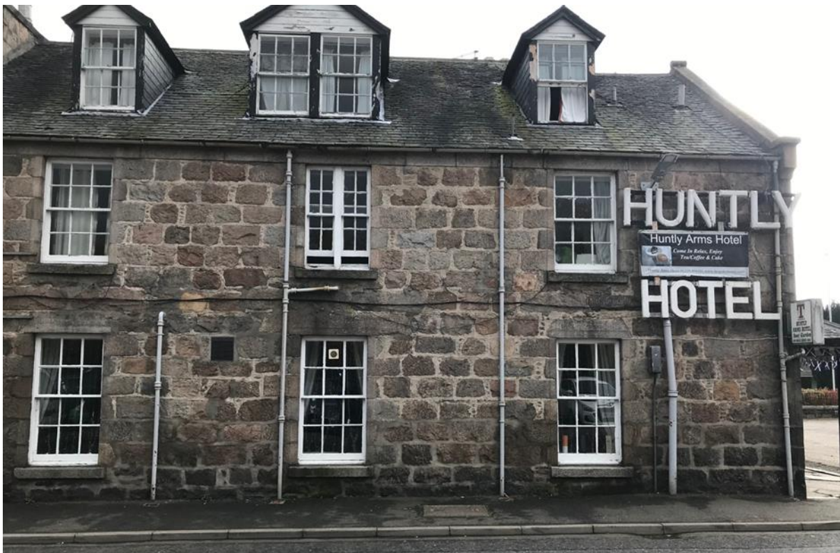
Figure 009.1. The North elevation of the Huntly Arms Hotel, Aboyne.
