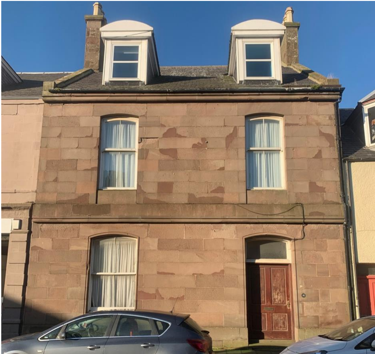
Figure 114.1. King Street, southeast elevation.
