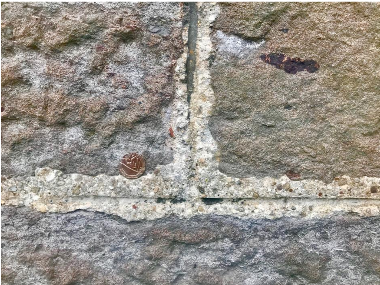
Figure 069.3. Angular and variable aggregates.
