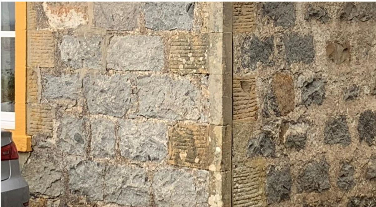
Figure 116.2. Flush pointing on the front principal elevation and sneck harl on the side.
