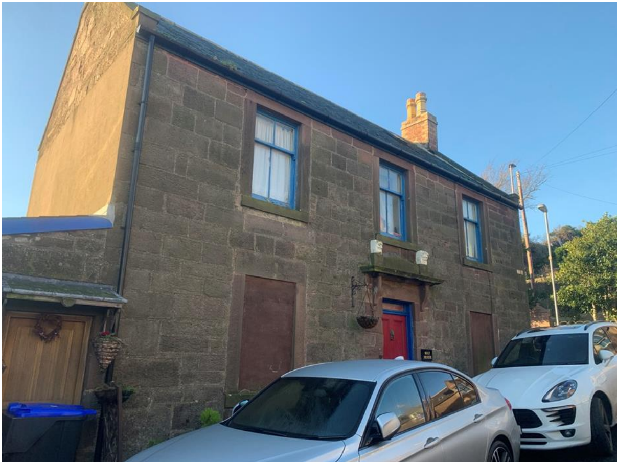
Figure 063.1. House on Mid Street, northeast elevation.
