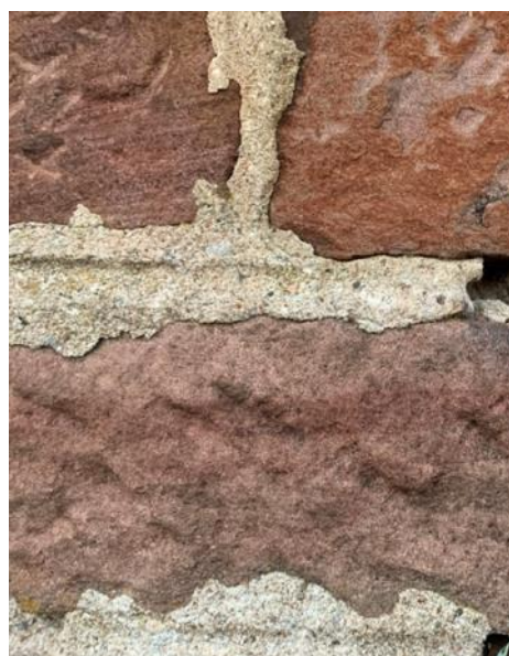
Figure 048.3. Marine sand with shell and lime inclusions.
