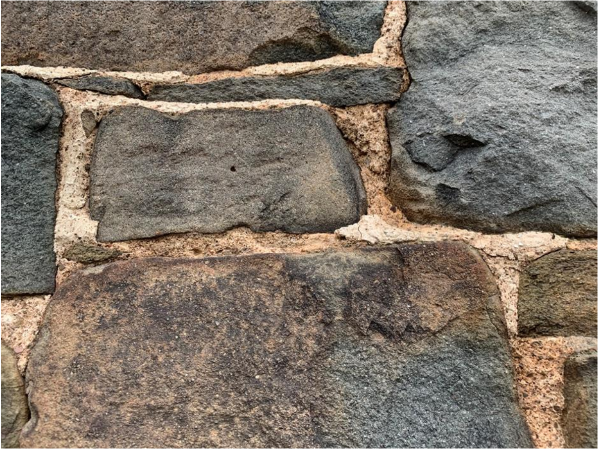
Figure 083.2. Raised and rounded finish, following the contours of the masonry.
