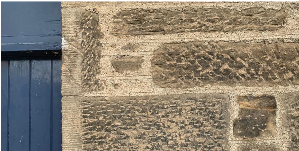
Figure 109.2. The flush finish and horizontal lining out.
