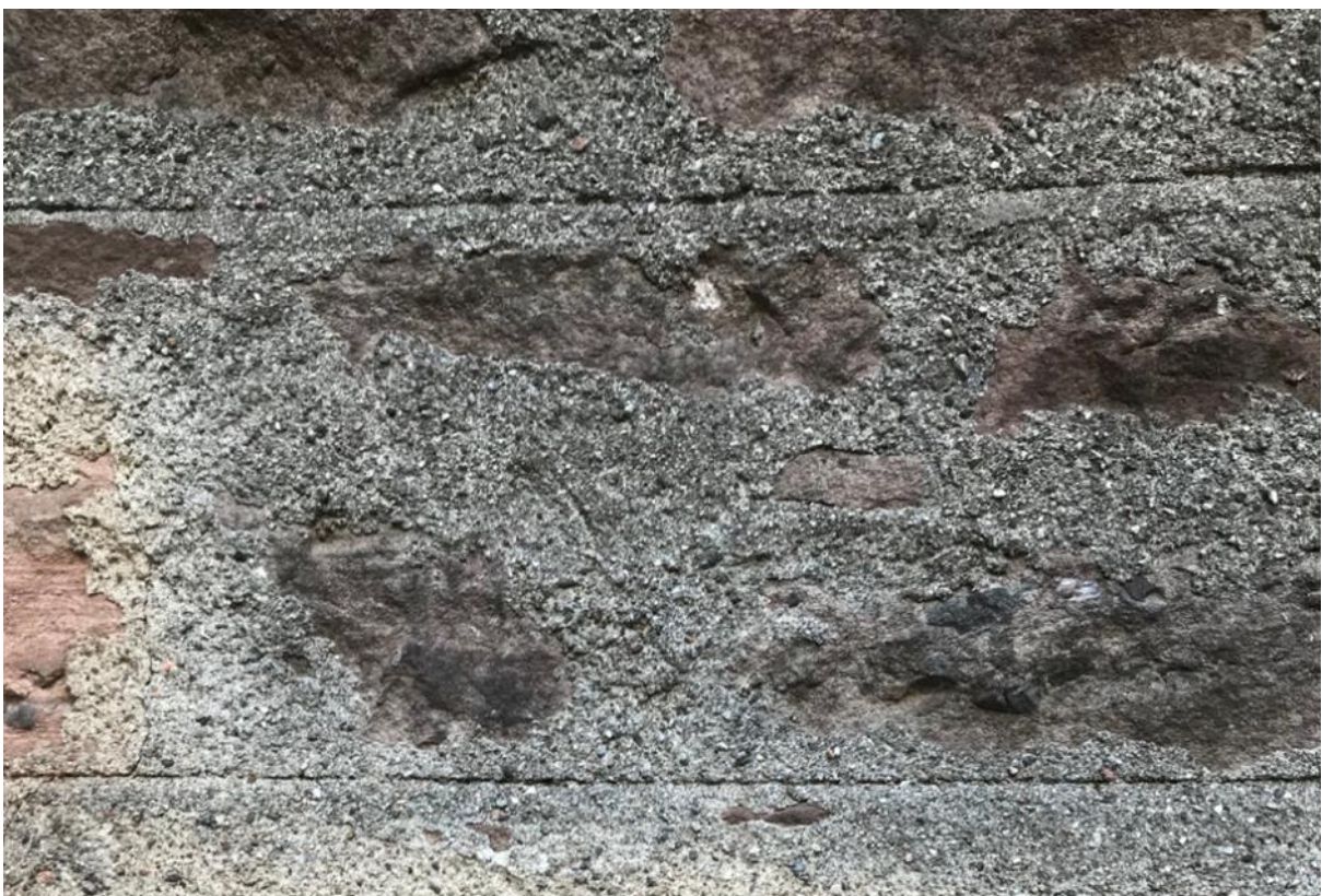
Figure 052.3. Sneck harl with ruling out.
