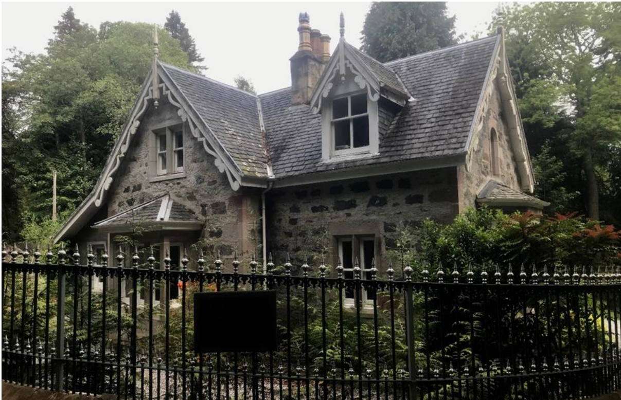
Figure 097.1. View of the lodge from the south east.
