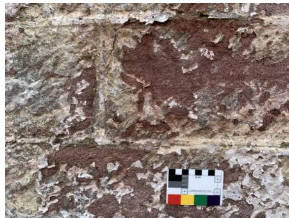
Figure 032.3. The raised ribbon pointing with limewash finish.
