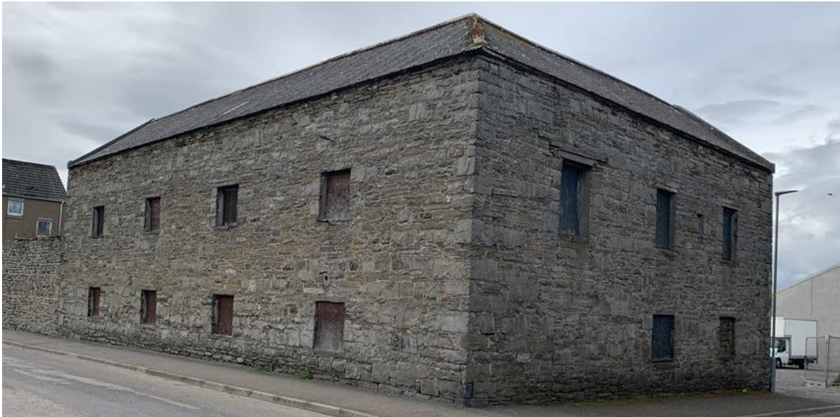
Figure 015.1. Main aspect of the warehouse.
