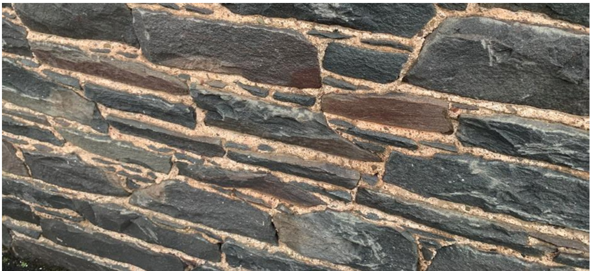
Figure 035.3. Random whinstone masonry.
