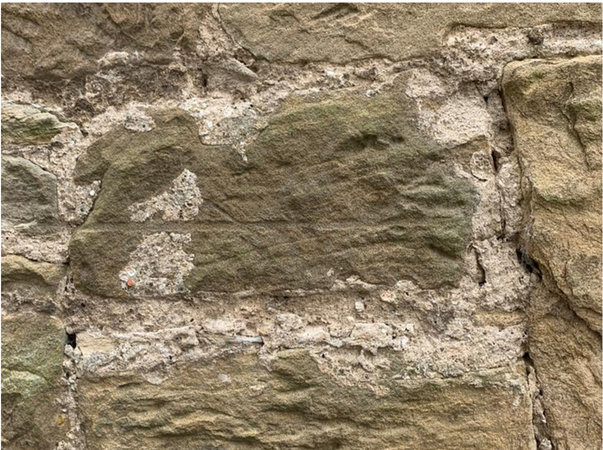
Figure 079.3. Fragmentary remains of an extensive flush finish and covering.
