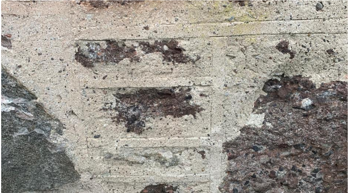
Figure 042.3. Horizontal and perpendicular ribbon pointing.
