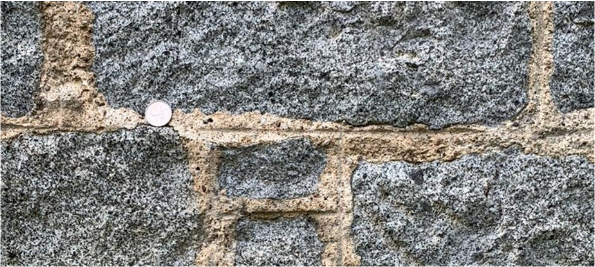
Figure 117.5. The annex built with squared granite blocks, flushed, with both horizontal and perpendicular ruling out.
