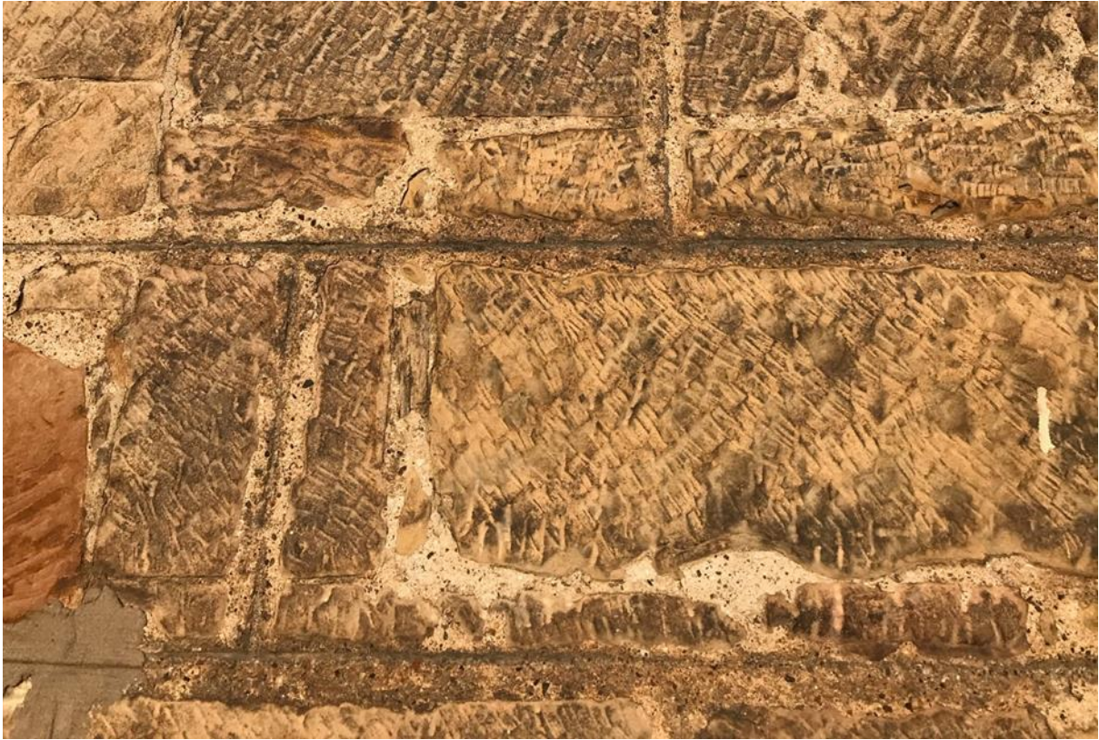
Figure 075.2. Horizontal and perpendicular ruling out with traces former lime harl.
