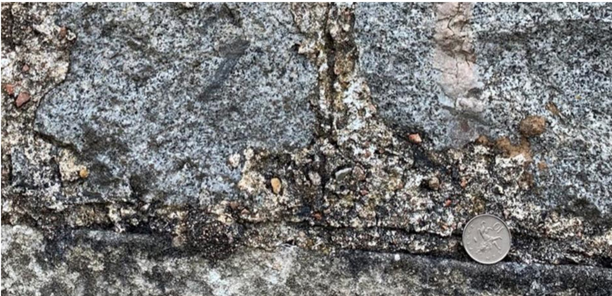
Figure 117.3. Flush pointed monochrome granite blocks with horizontal and perpendicular ruling out.
