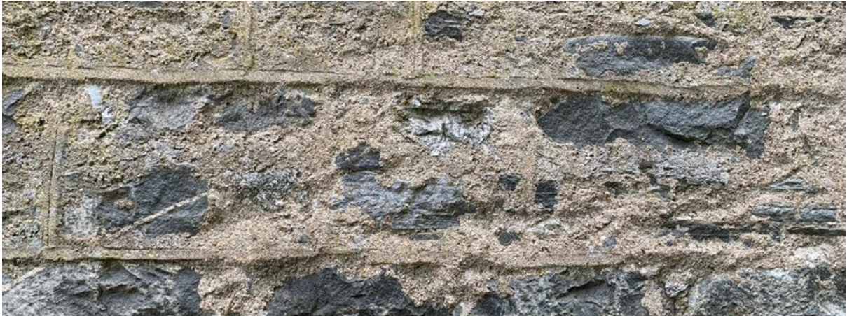
Figure 024.4. Sneck and raised band or pointing.
