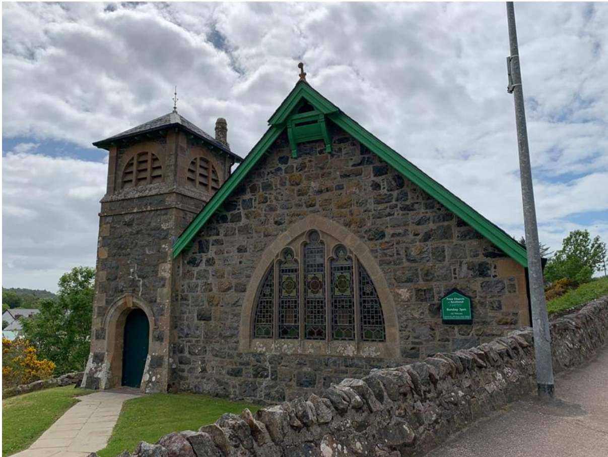
Figure 104.1. The principal elevation of the church.
