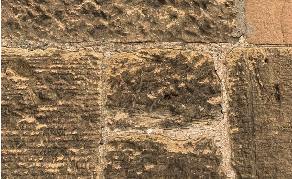
Figure 080.2. Relatively wide flush finish.
