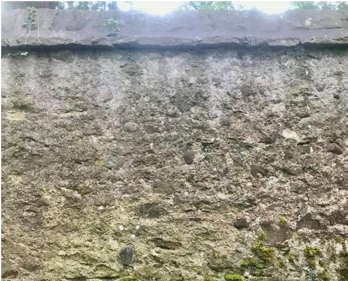
Figure 073.1. The wall viewed from the South West.
