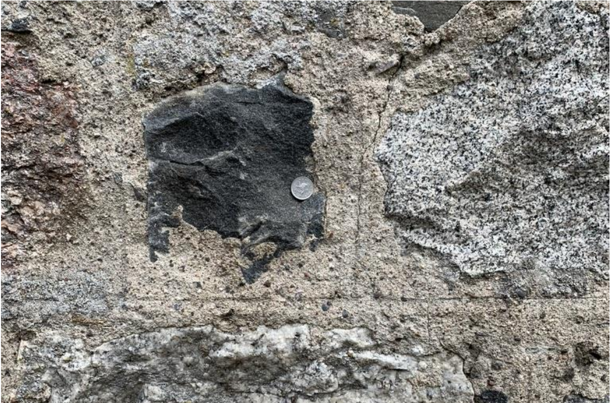
Figure 024.2. Sneck, ruled weather-shot point.
