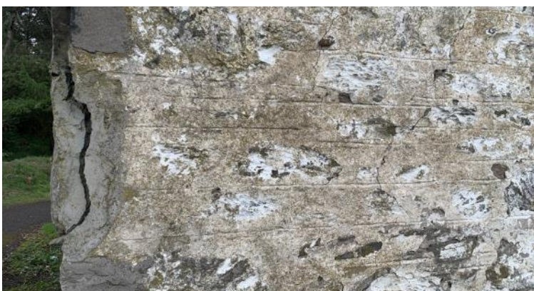
Figure 026.2. Flush pointing and informal ruling out with limewash.
