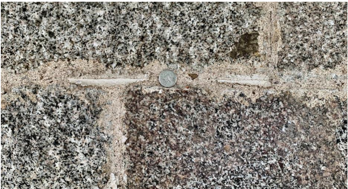
Figure 023.2. Flush ruled pointing with overlaying whitewash.
