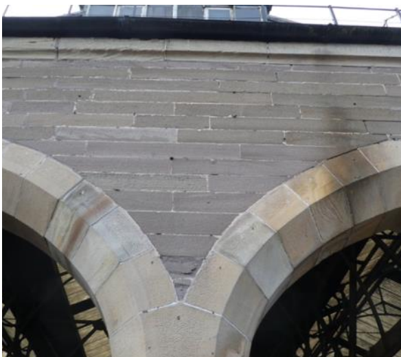
Figure 068.2. Stugged ashlar for the walls with lighter detailing on the arches.
