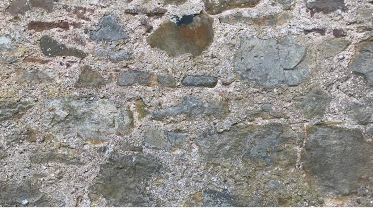
Figure 091.2. The sneck pointing on the south extension of the mill.
