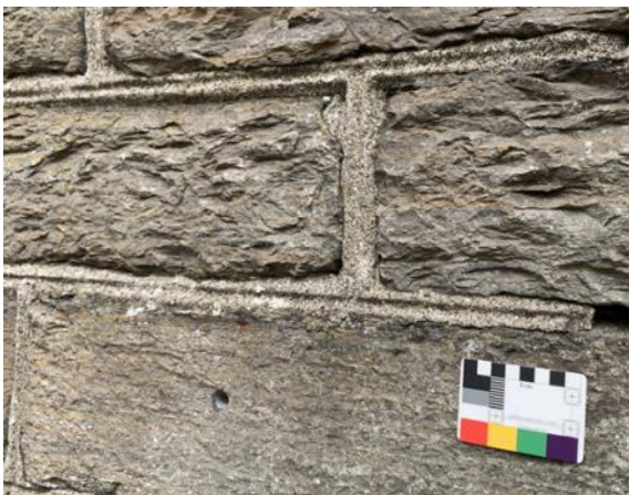
Figure 012.2. Flushed and ruled out mortar on the front façade.
