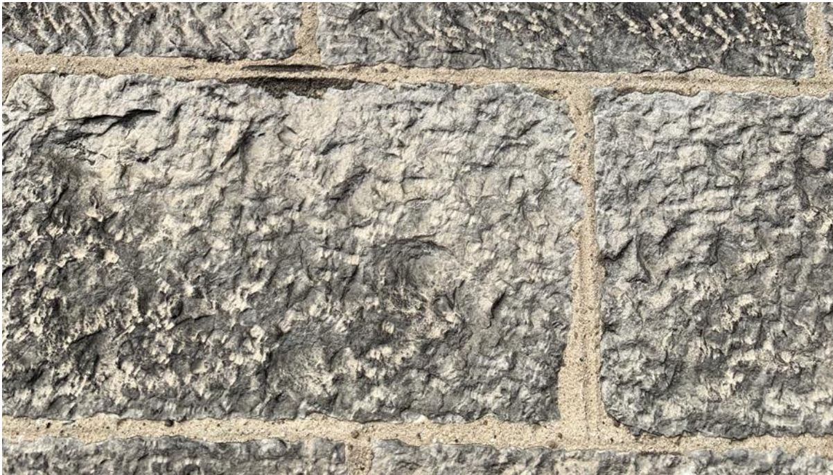
Figure 098.2. Flush ruled lime pointing, also showing aggregate and lime inclusions.
