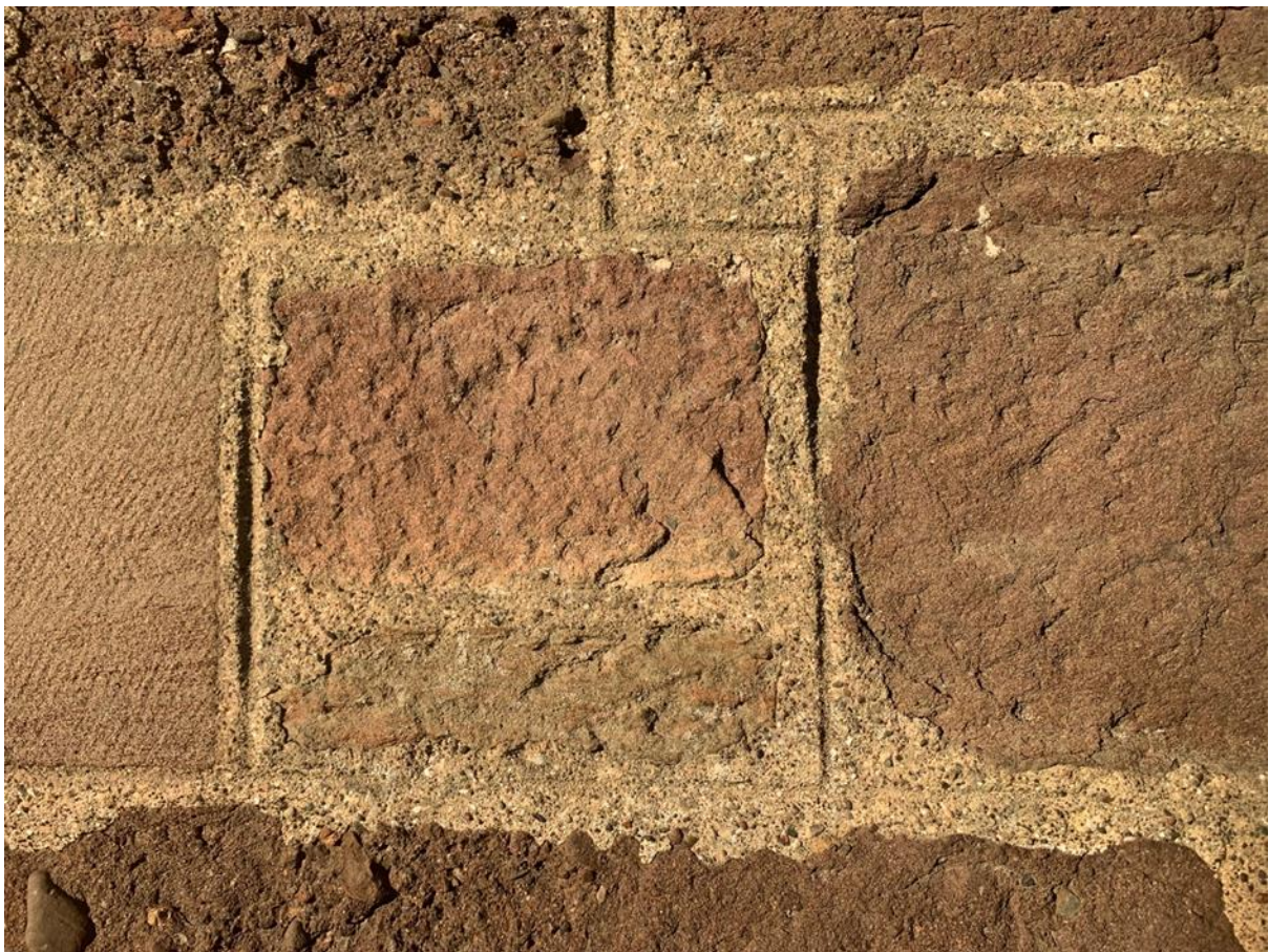
Figure 020.3. Horizontal and perpendicular ruling out.
