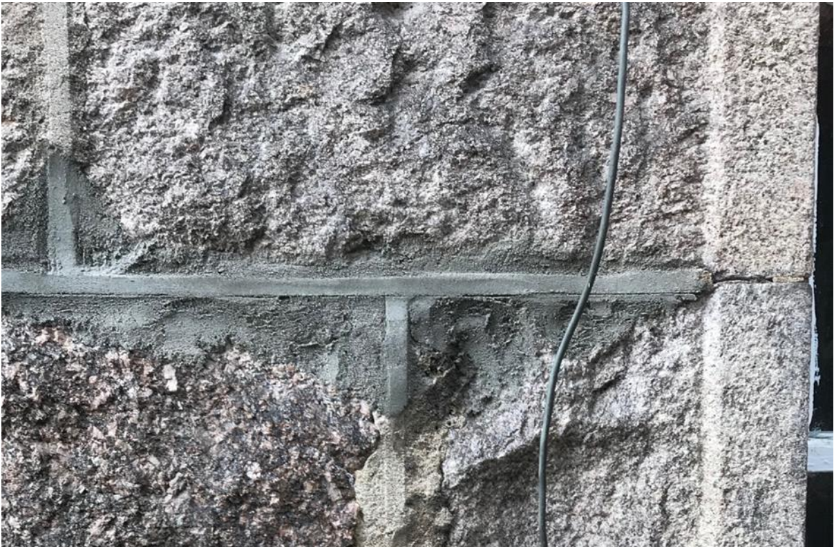
Figure 009.3. Raised band repairs in cement mortar.
