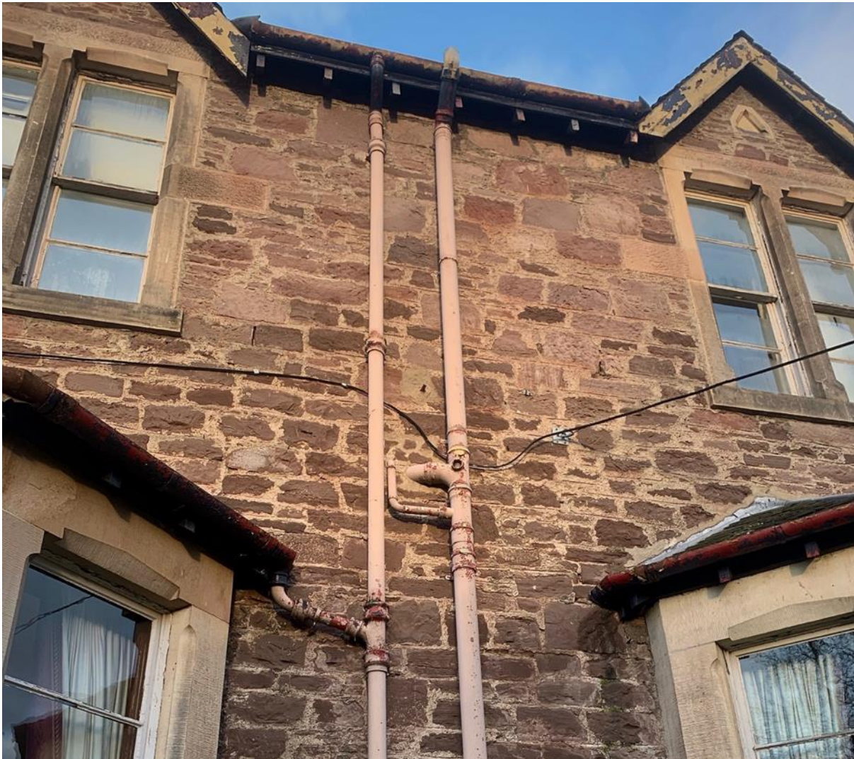
Figure 072.1. The Woodside Hotel, South East front.
