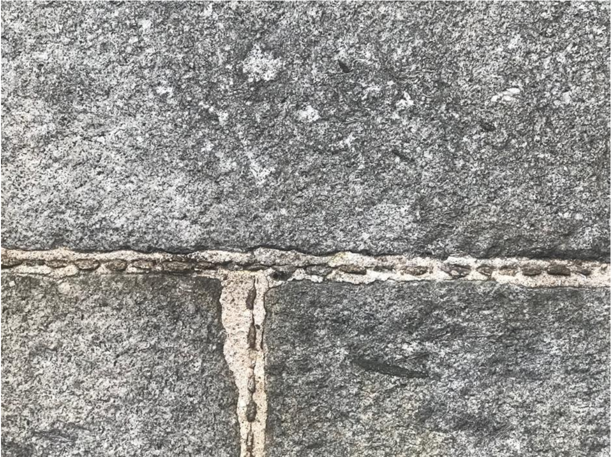
Figure 006.2. Granite built and cherry-stoned with what appear to small granite chips.
