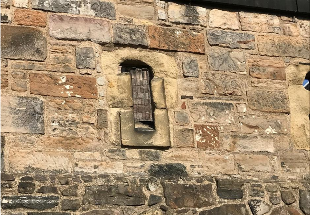
Figure 003.2. The Foogs Gate forework masonry probably dating from the mid-18th century. Several masonry units either side of the lancet show limewash surviving in the tooling marks suggesting that this area was flush pointed and limewashed.
