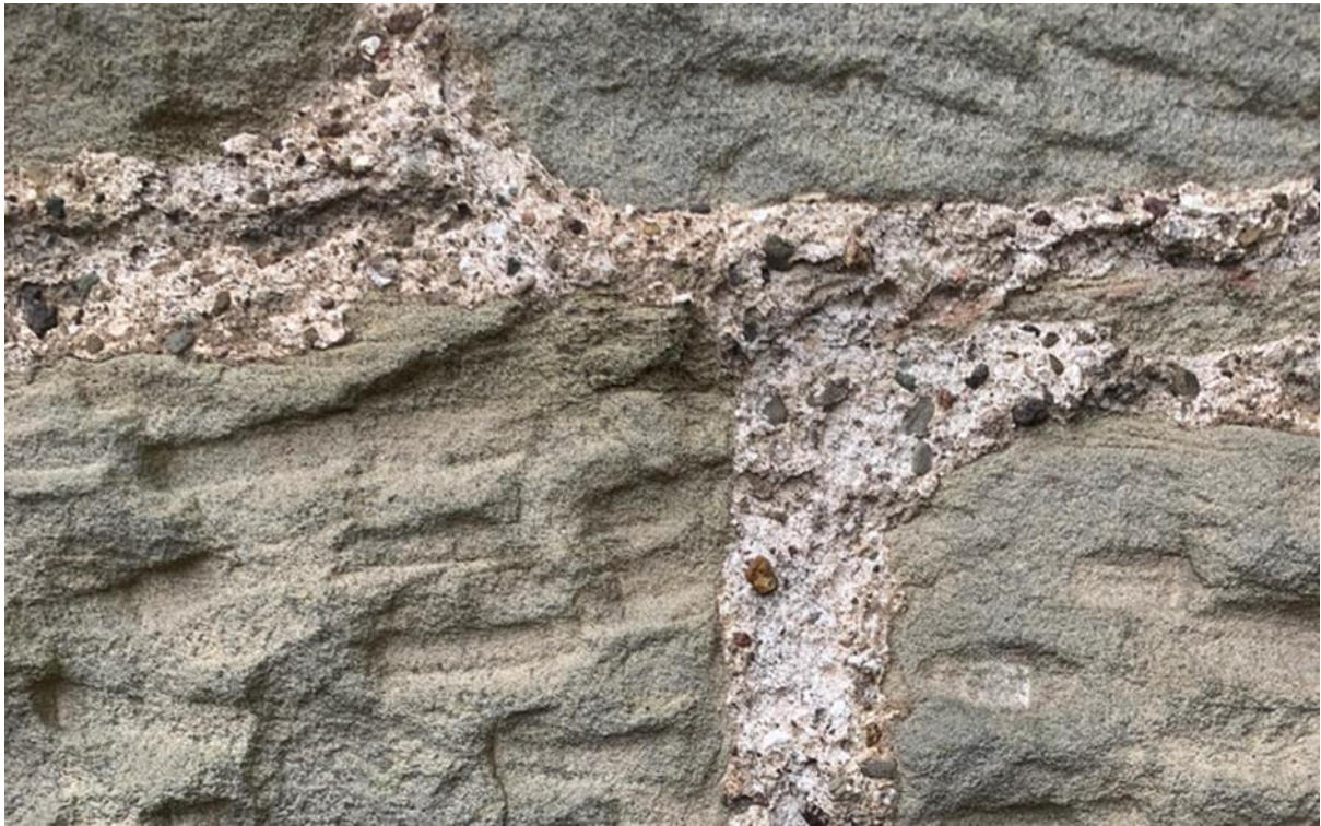
Figure 086.3. Coarse angular and rounded aggregates.
