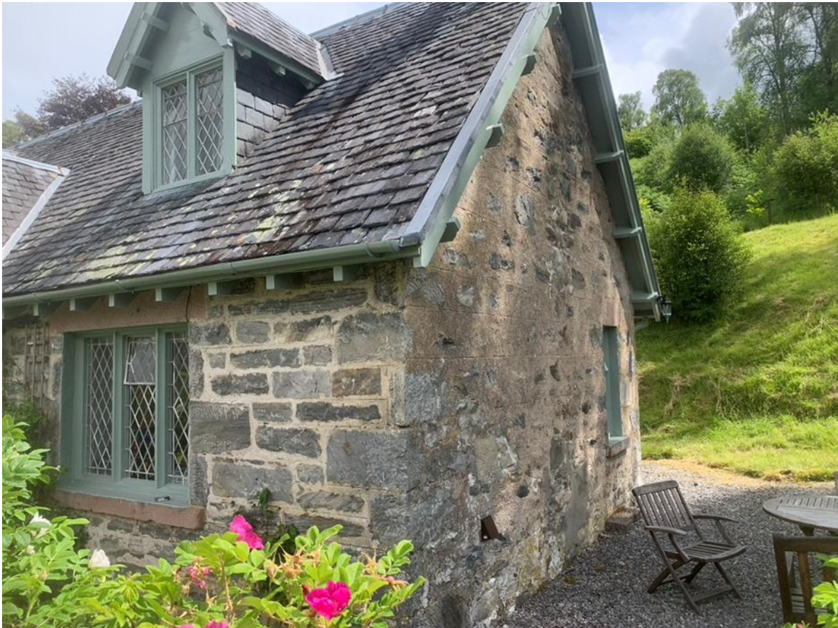
Figure 102.4. Tomich estate farm cottage with ruled flush finish on the front elevation and ruled sneck harl on the gables and rear.
