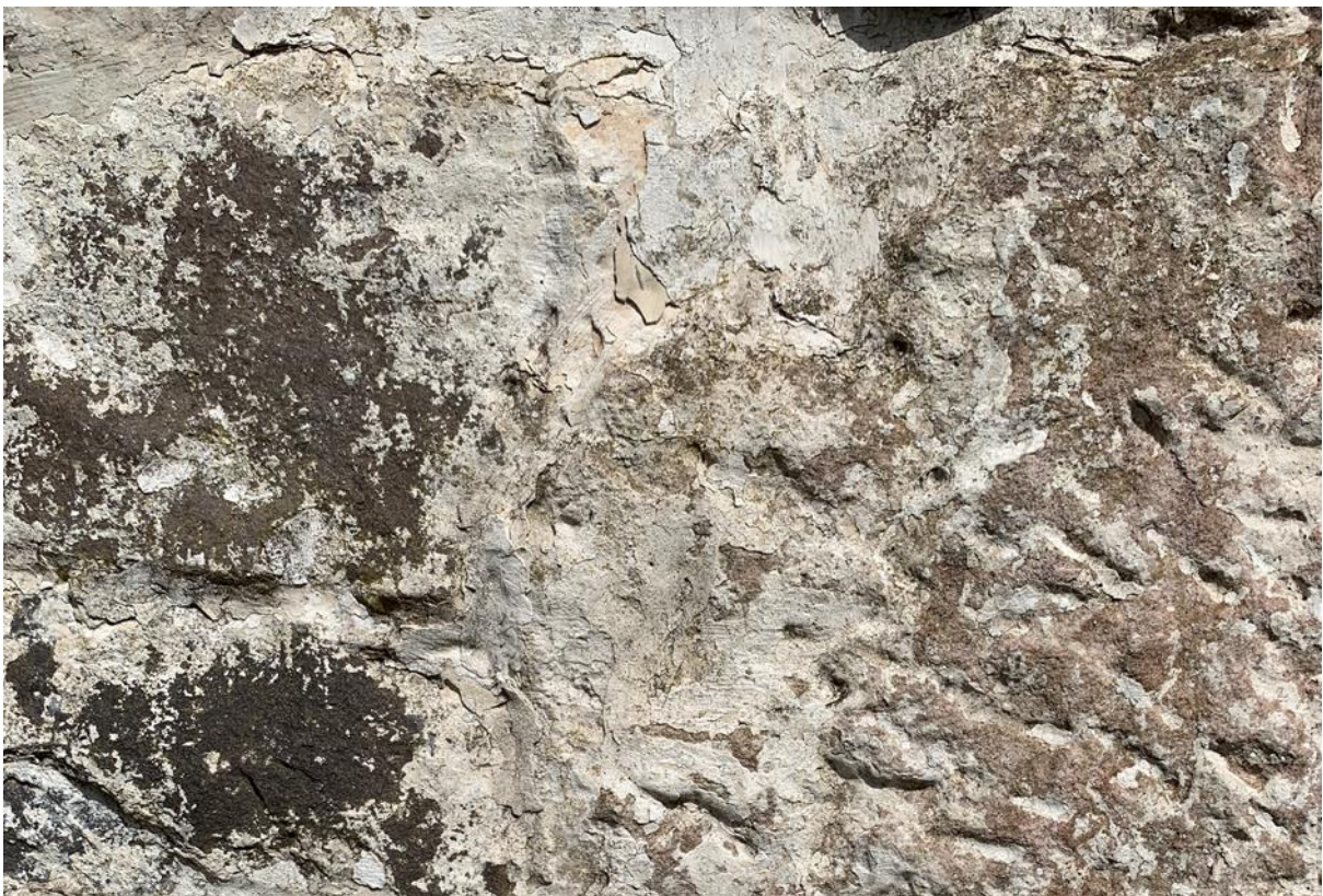
Figure 037.3. The many layers of limewash surviving in some areas.
