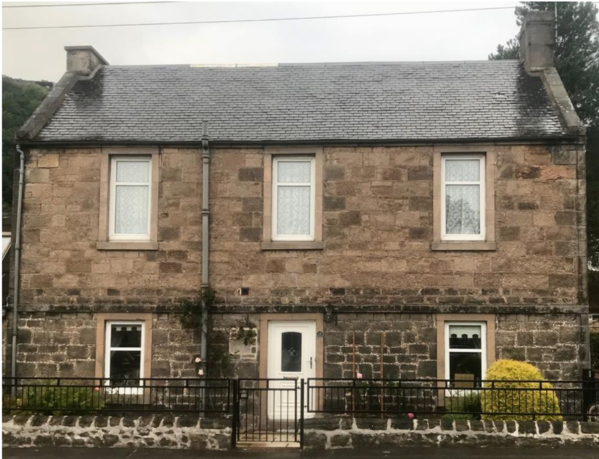
Figure 041.1. Southern view of a house on Main Street West, Menstrie.
