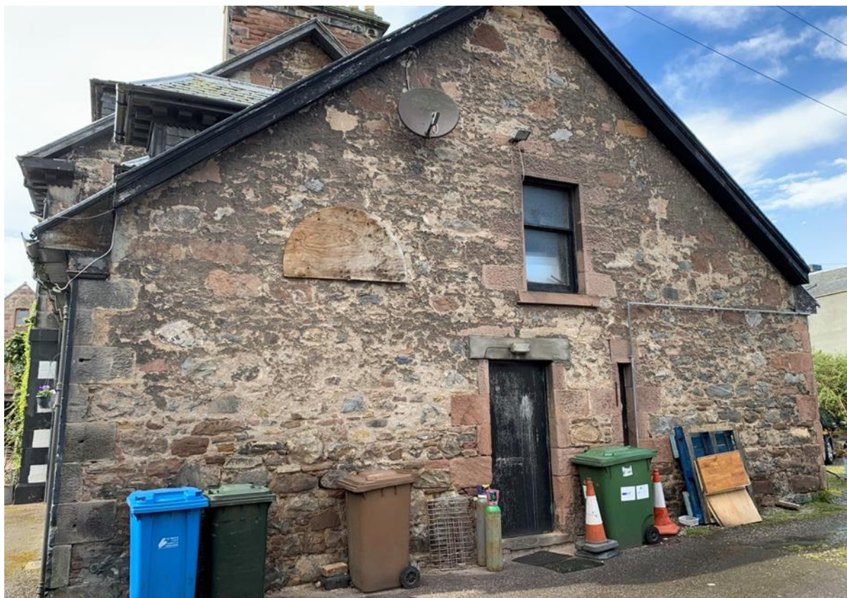
Figure 045.1. The Anderson Hotel, rear elevation.
