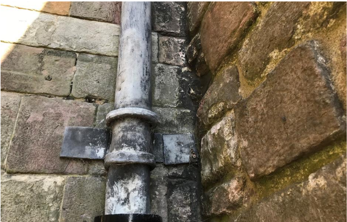
Figure 003.3. Ashlar work of the Portcullis Gate dating from the 16th century. Limewash fragments visible to the left and right of the downpipe.
