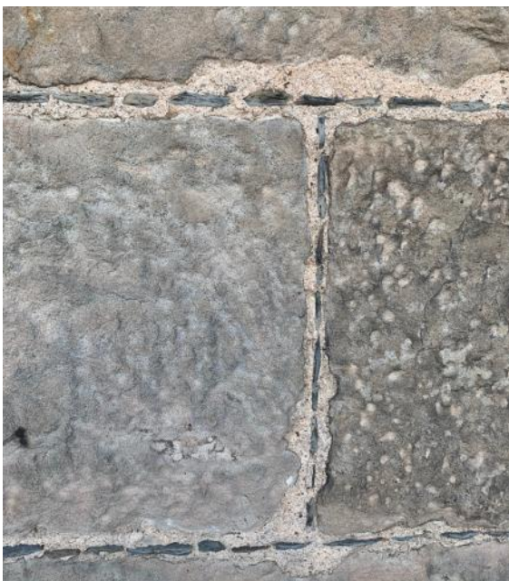
Figure 005.2. Detail of the cherry-stoned finish.
