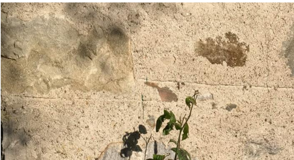
Figure 054.2. Example of horizontally ruled out sneck harling.
