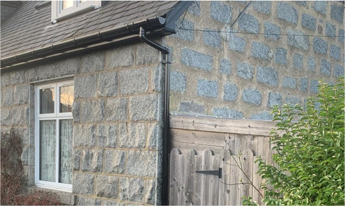
Figure 112.2. Hierarchy of finishes between front and sides.
