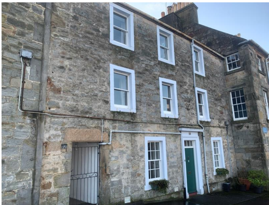
Figure 010.1. East Terrace, north elevation.
