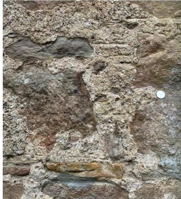
Figure 044.3. Later marine sneck harl (left) overlaying earlier mortar without marine inclusions.
