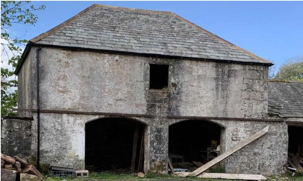
Figure 032.1. The south west corner of the steading complex at Muiryhill.
