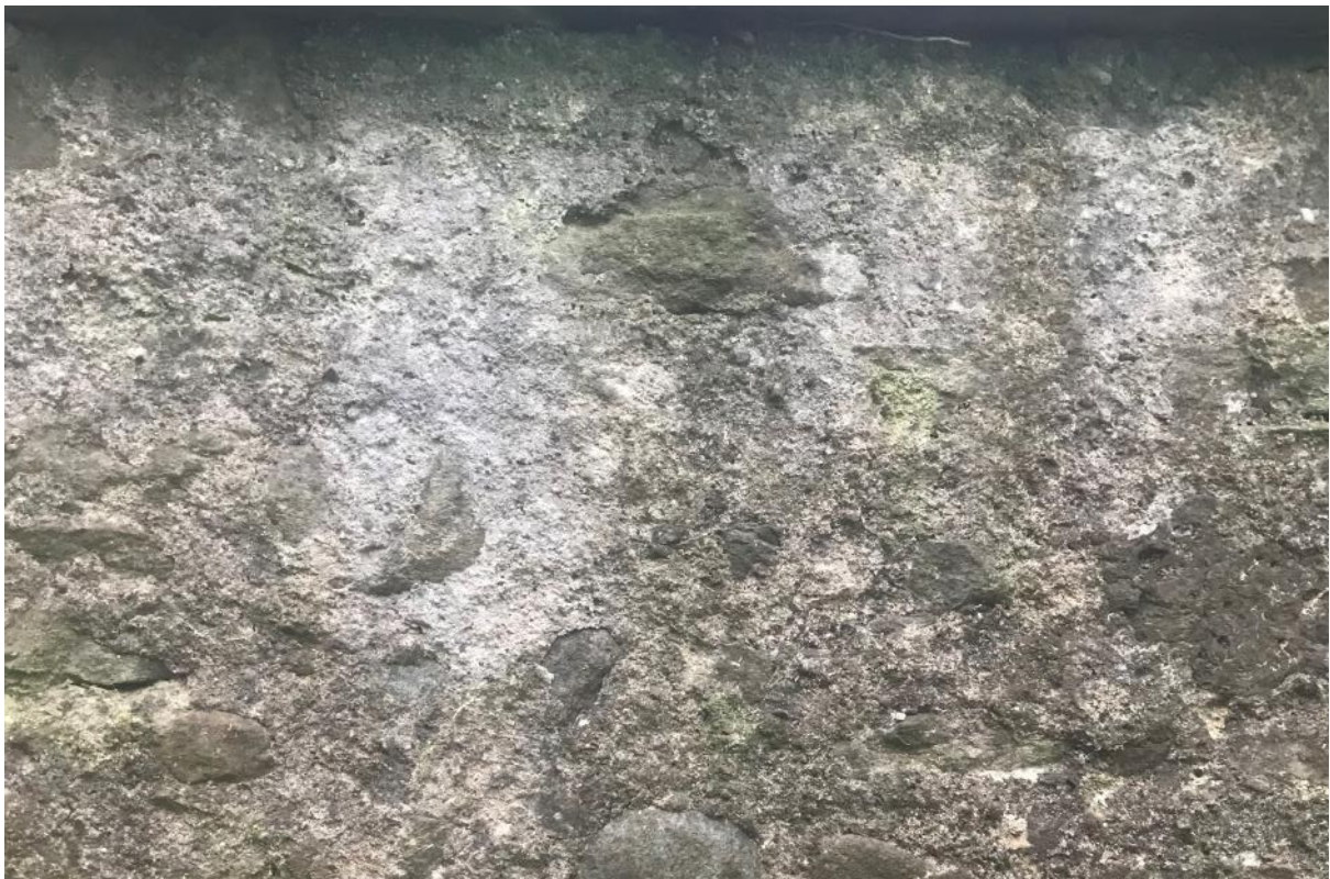
Figure 073.3. Extensive remains of flush finish.
