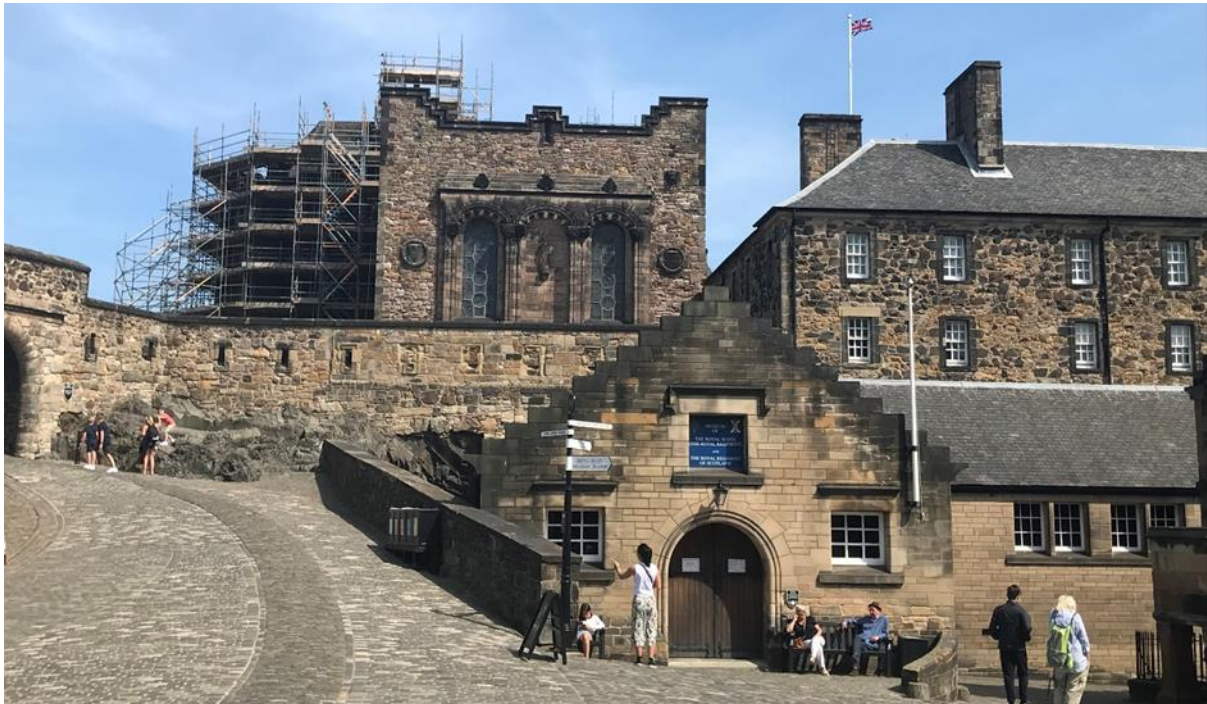
Figure 003.1. The Foogs Gate forework middle left, and magazine bottom right, at Edinburgh Castle.
