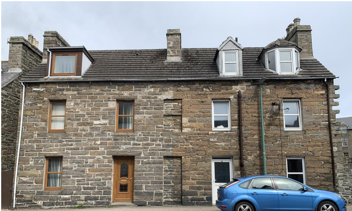
Figure 014.1. The terrace at Dempster Street in the Pultneytown district of Wick.
