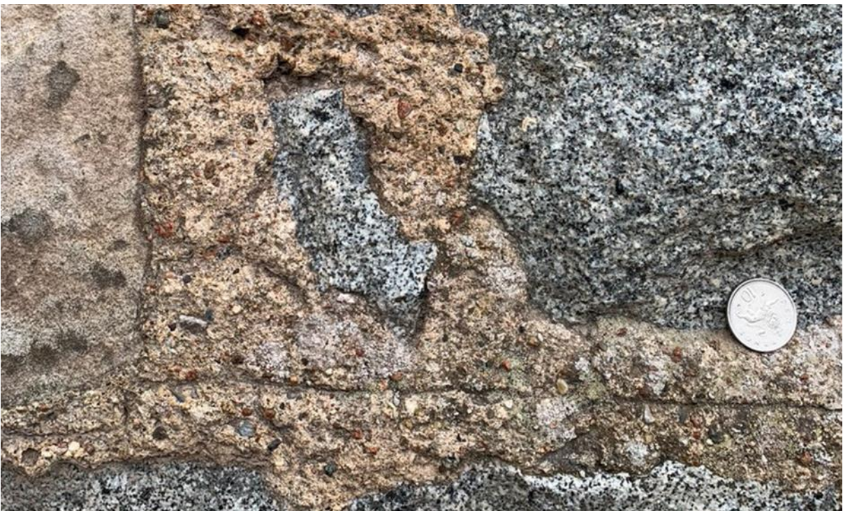
Figure 117.6. The former stable block pointing with informal ruling out.
