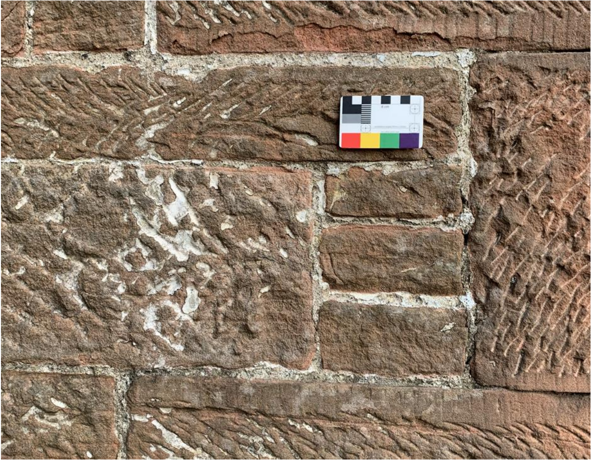
Figure 126.2. Detail of mortar with remains of limewash.
