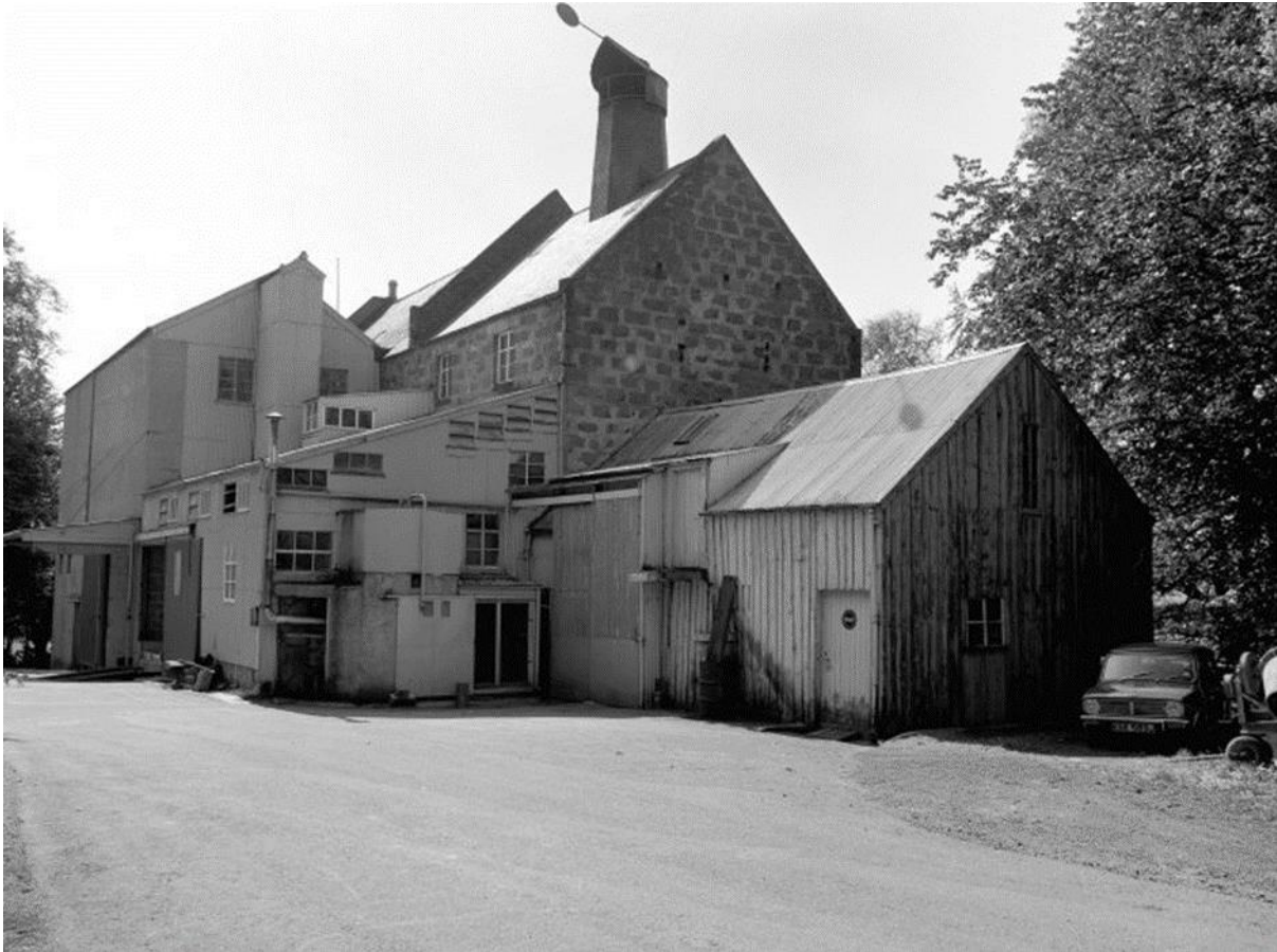
Figure 022.1. Montgarrie Mill from the northeast (20th Century). © HES. Reproduced curtesy of J R Hume.
