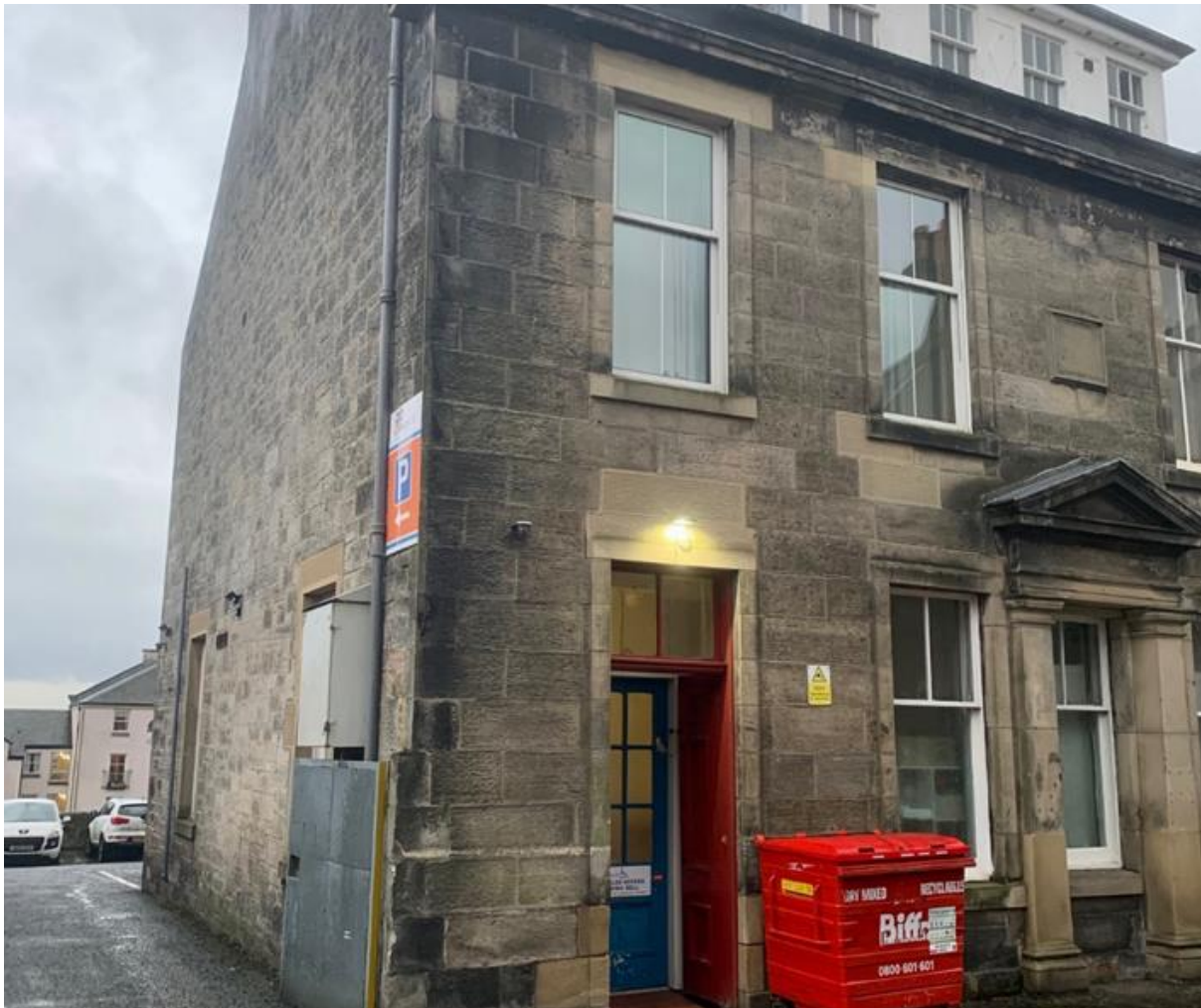
Figure 029.1. St Margaret Street, west façade.
