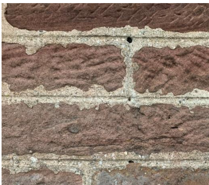
Figure 048.2. Horizontal and perpendicular ruling out.
