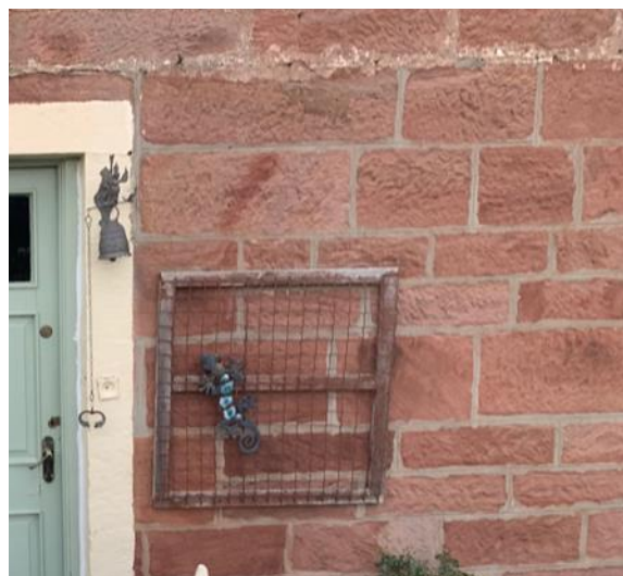
Figure 039.3. Ruled out cement mortar repairs made to the ground floor.
