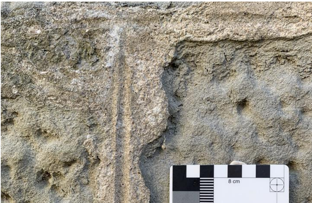
Figure 034.3. Flush lime pointing, ruled out with fine sand mortar containing lime inclusions.
