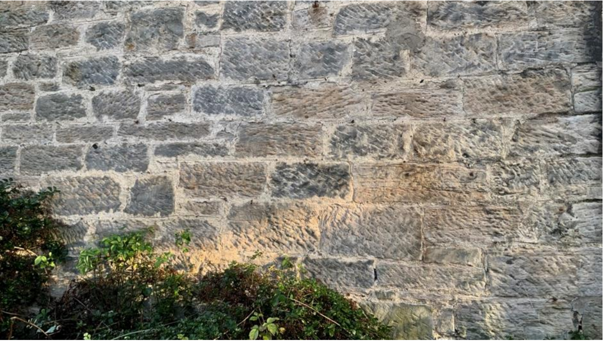
Figure 122.2. Ruled flush finish.
