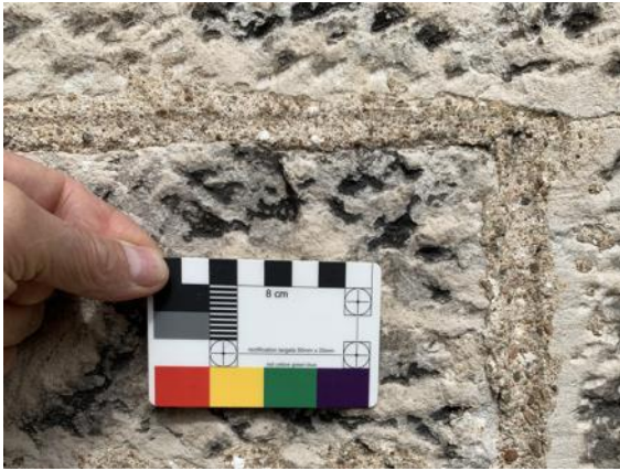
Figure 101.2. Formal mortar on the front elevation, ruled out horizontally and vertically. Also showing coarse aggregate and lime inclusions.
