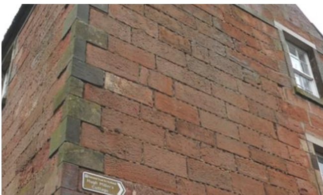
Figure 019.2. The decorative, yet functional cherry-stoning is visible from street level.
