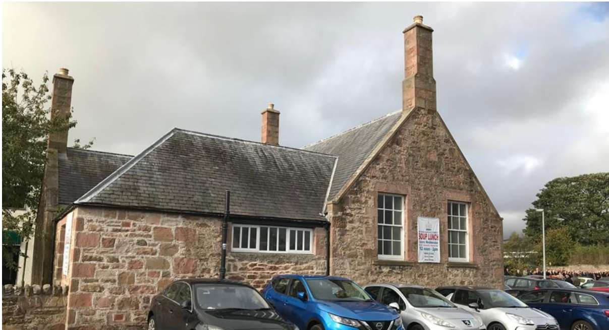
Figure 051.1. St Clement's Church Hall, eastern elevation.
