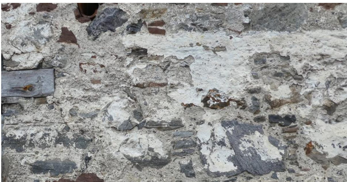
Figure 056.2. Remains of ruled sneck harl and limewash coats.
