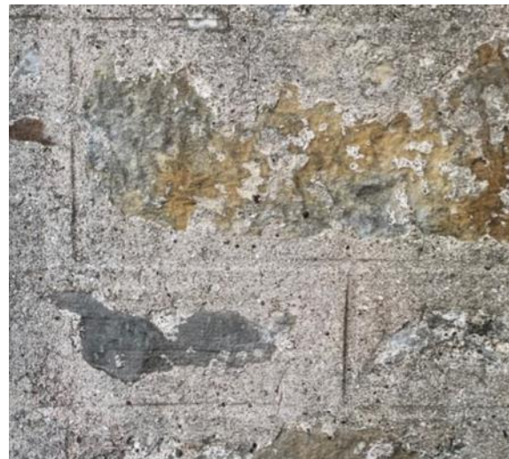
Figure 010.4. Horizontally and perpendicularly ruling out on the sneck finish.
