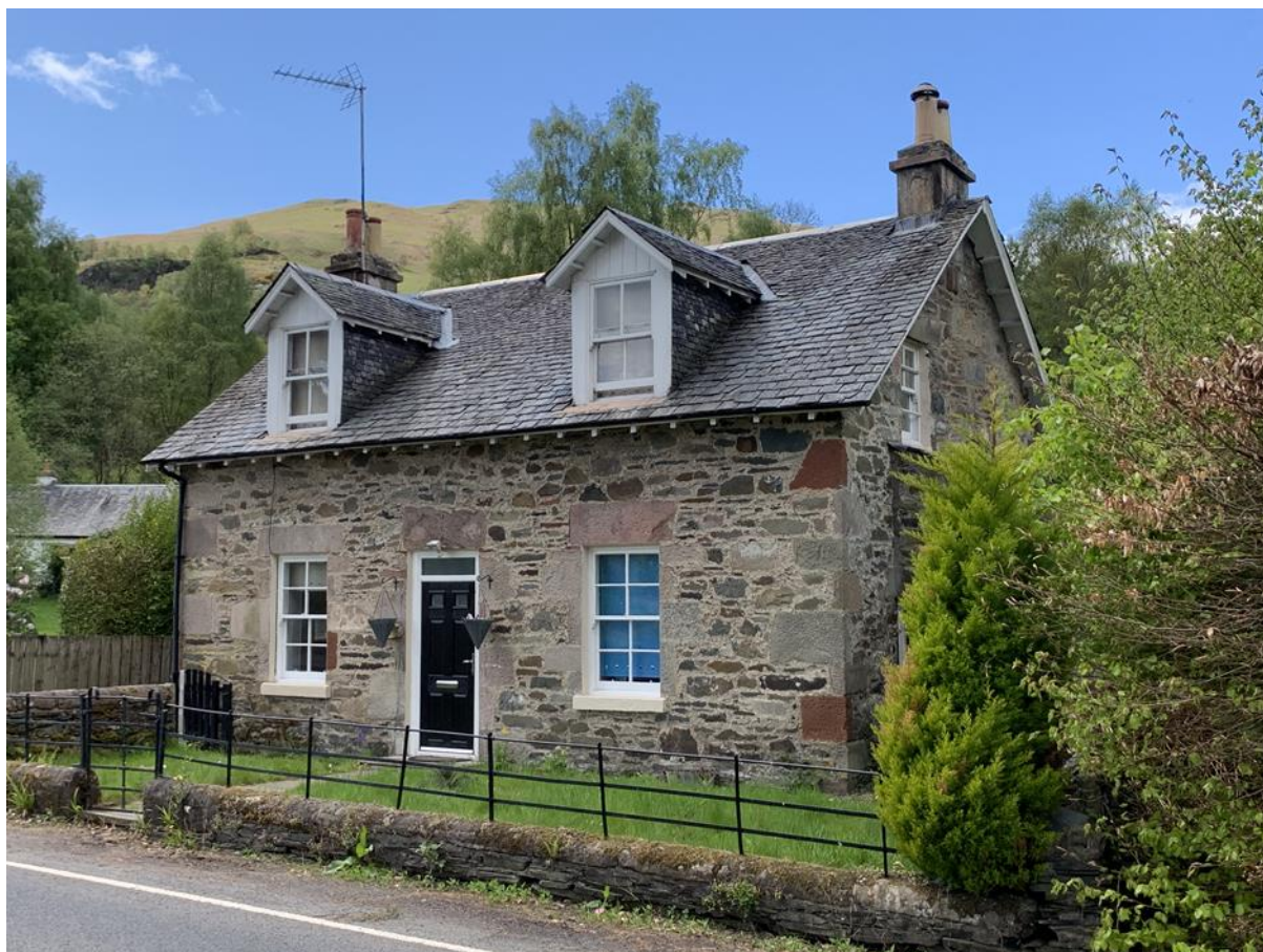
Figure 076.1. Front elevation of fully lime sneck pointed cottage, Luss.
