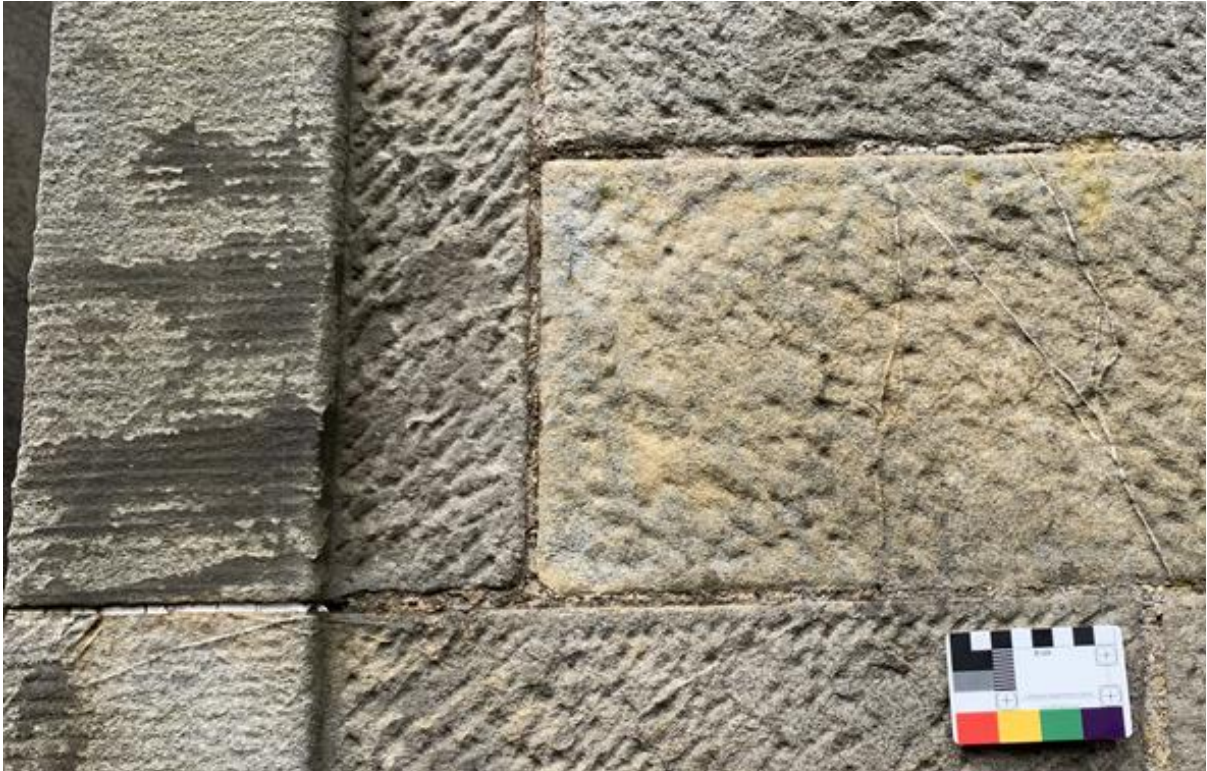
Figure 125.2. Squared ashlar blocks with coarse mortar pointing.
