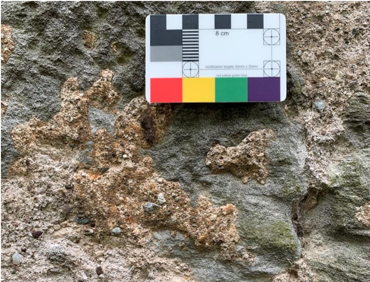
Figure 002.2. Surviving orange coloured harl in the centre, overlain with a later white pointing bottom left. This harl could be part of the original finish matched to the Great Hall close by.
