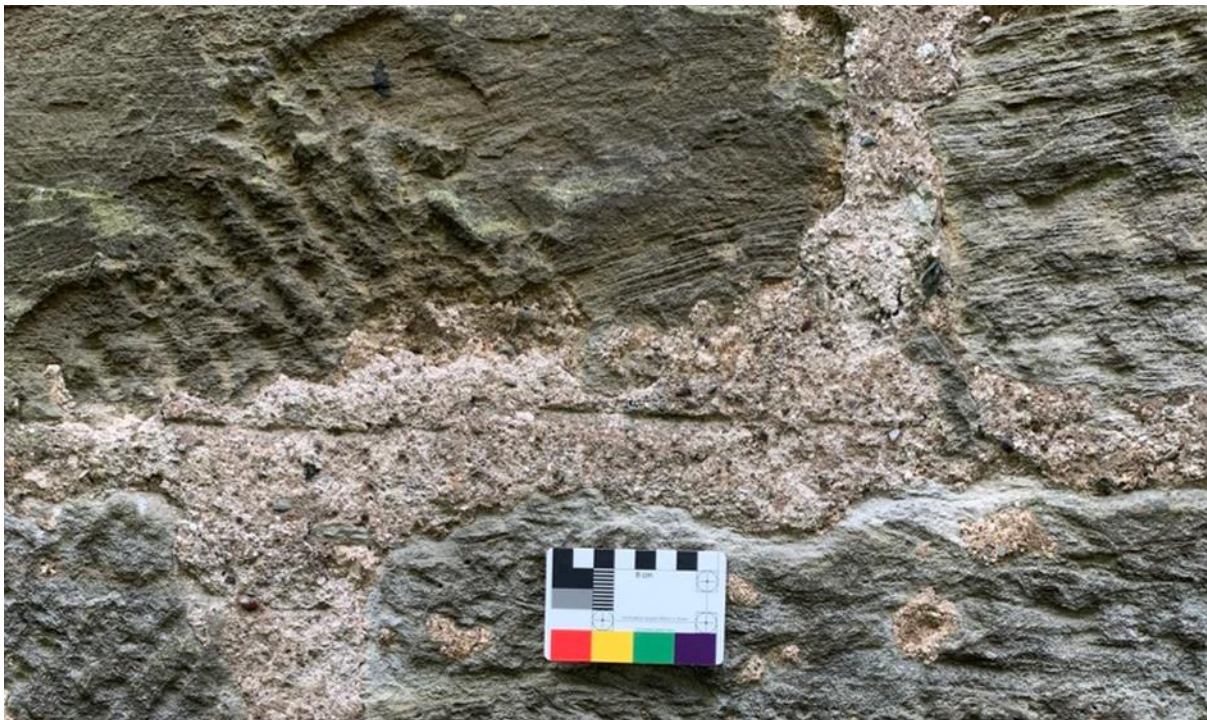
Figure 002.3. Overlying white pointing with horizontal ruling out, probably dating from the 19th century.
