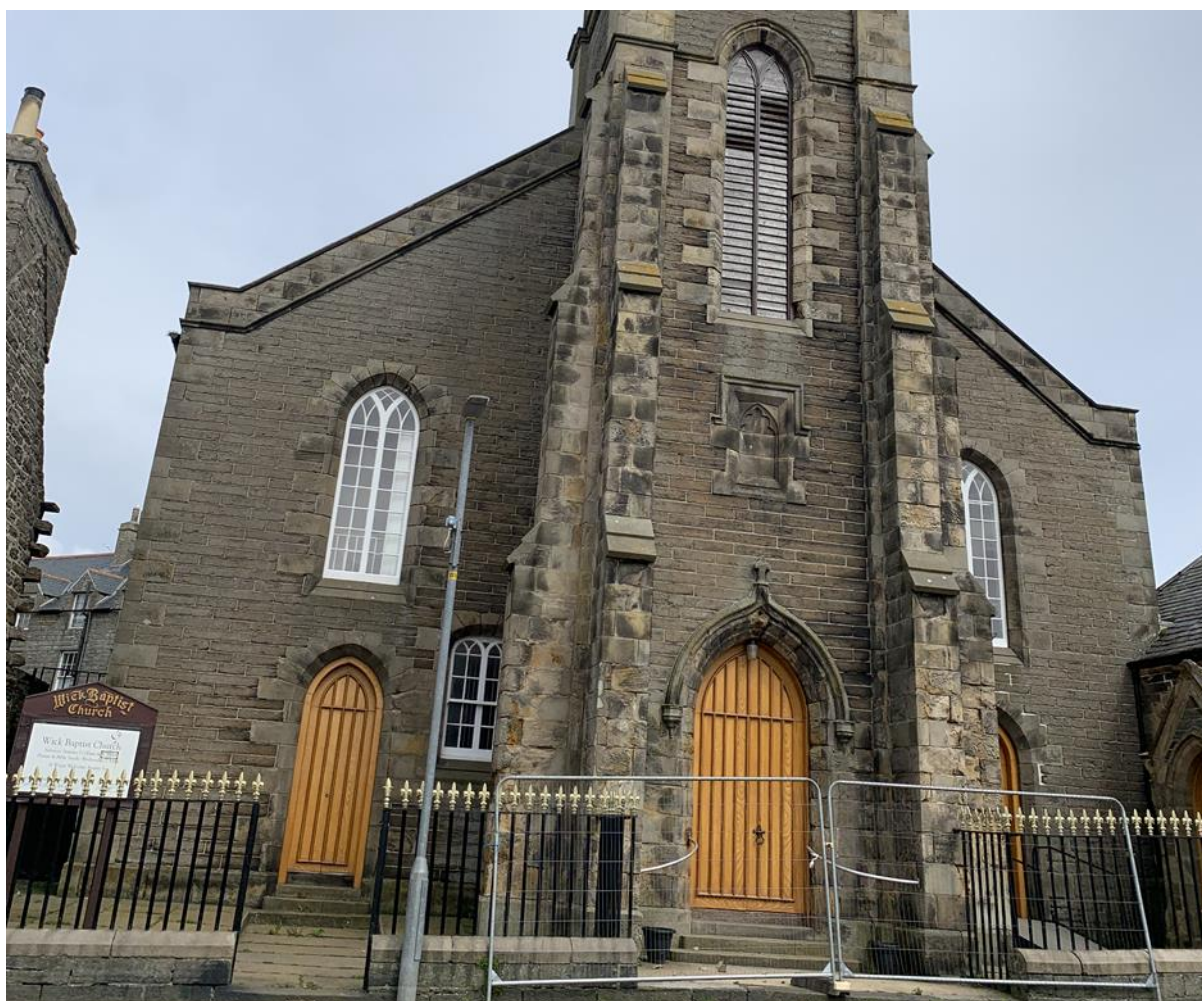
Figure 099.1. Baptist Church, Wick. The main façade on Dempster Street.
