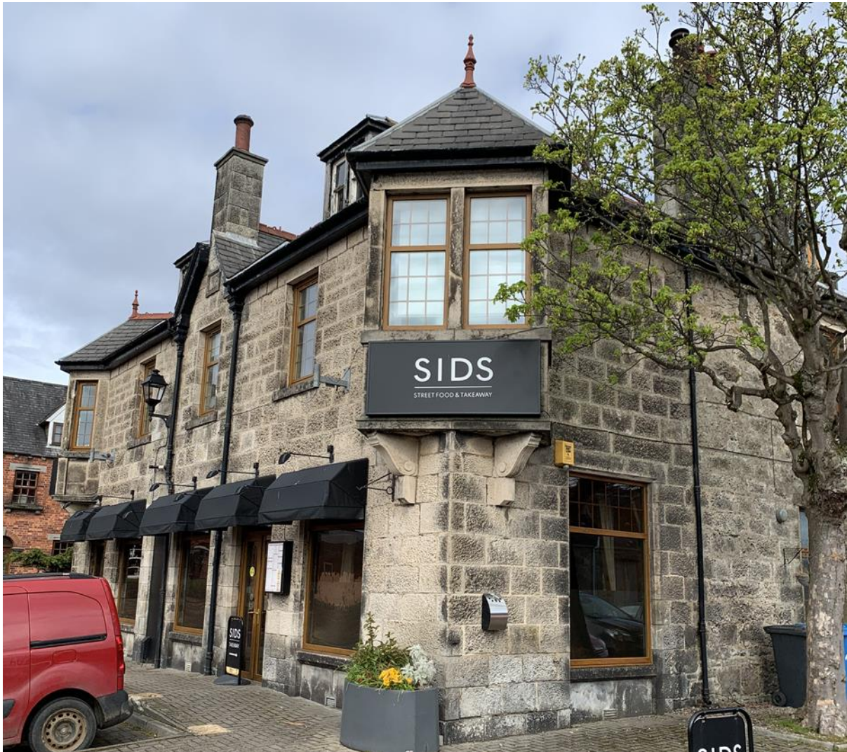
Figure 098.1. The south and east elevations of the building.
