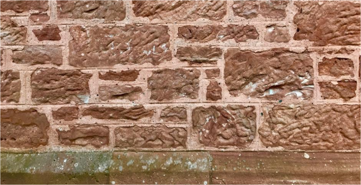
Figure 106.2. Pink flush finish with horizontal and perpendicular ruling out.
