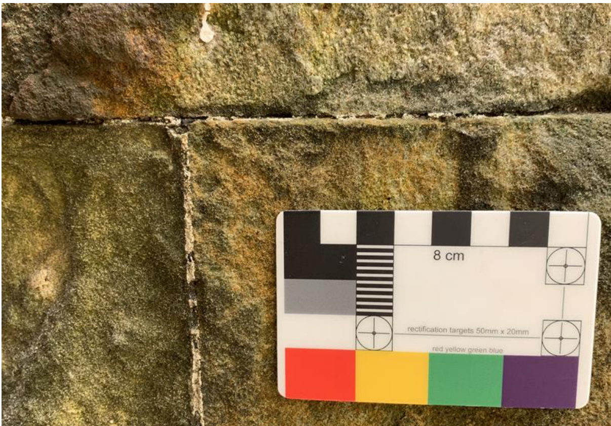
Figure 099.3. Fine ashlar pointing made with a lime putty.
