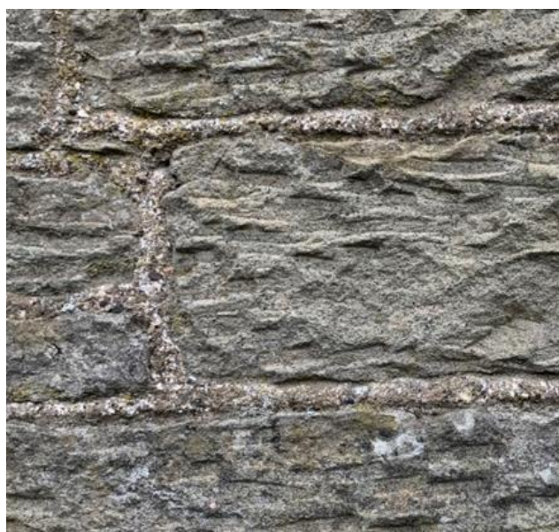
Figure 088.2. Raised convex ribbon.
