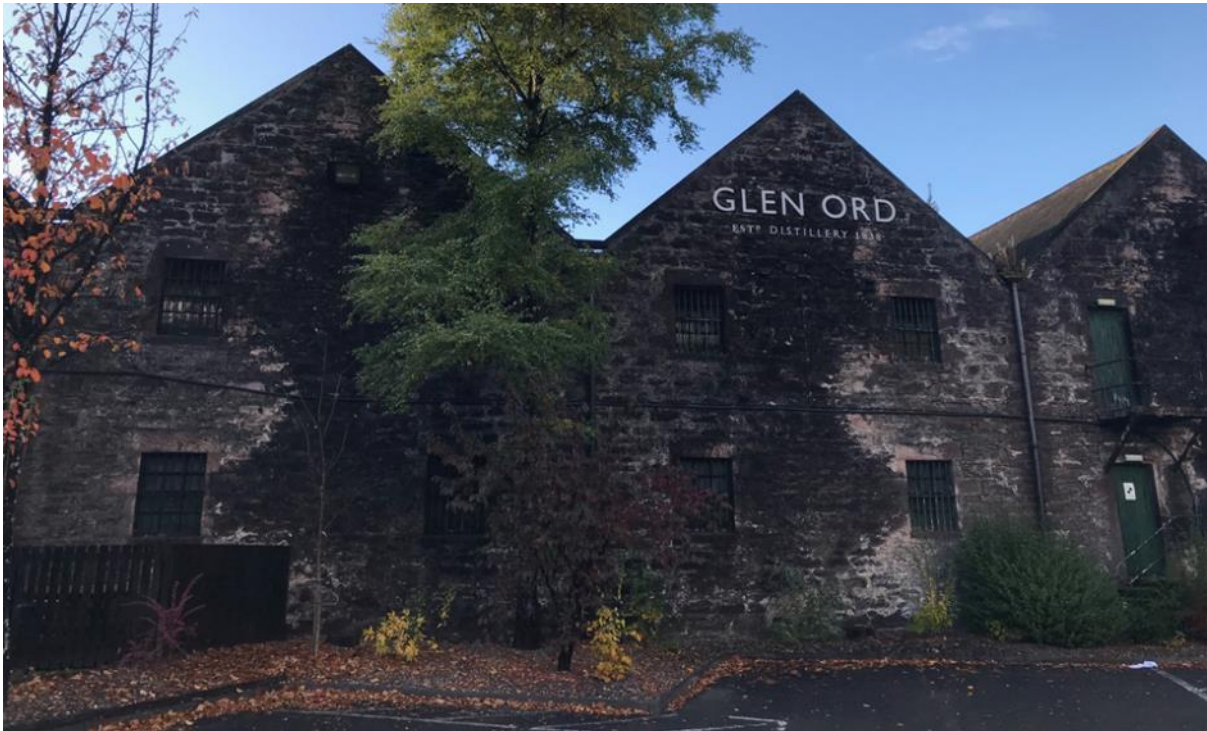
Figure 052.1. Glen Ord Distillery covered in lime finish but obscured by sac fungus.
