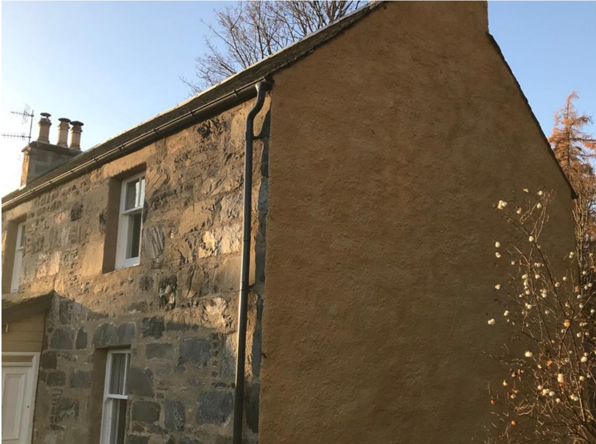
Figure 043.2. Ruled semi-formal front and repaired and limewashed gable and rear elevation.
