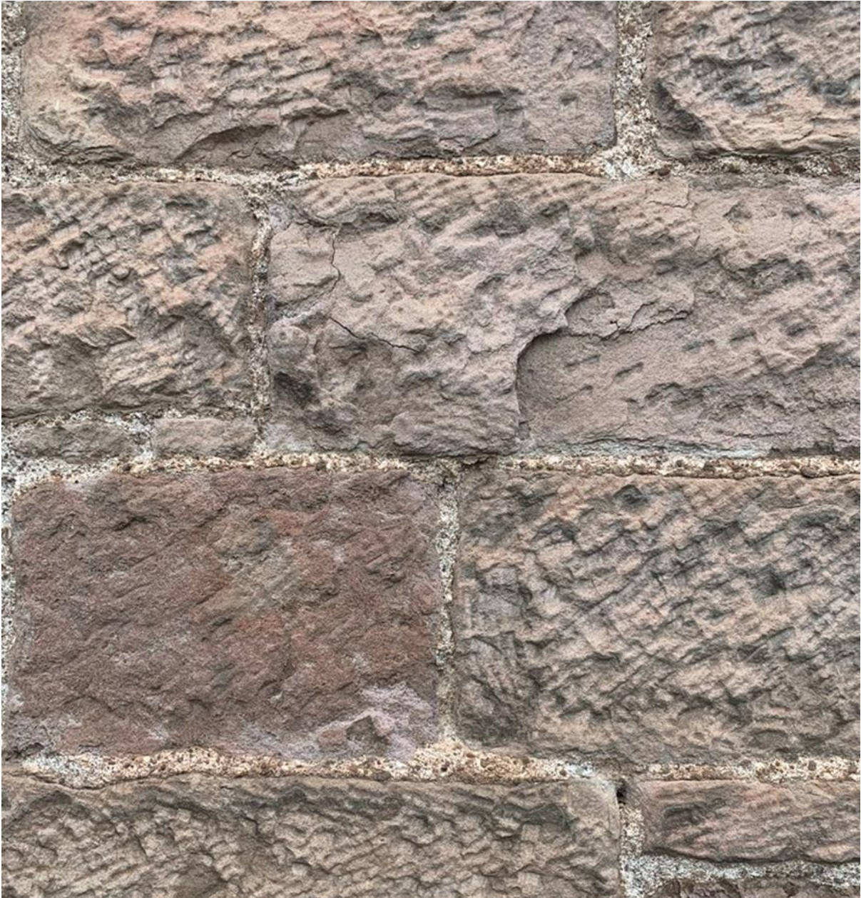
Figure 084.2. Joints with convex and rounded profile.
