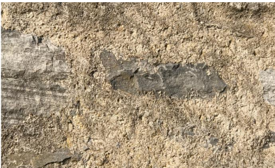
Figure 053.2. Detail of the flush finish on the west gable.
