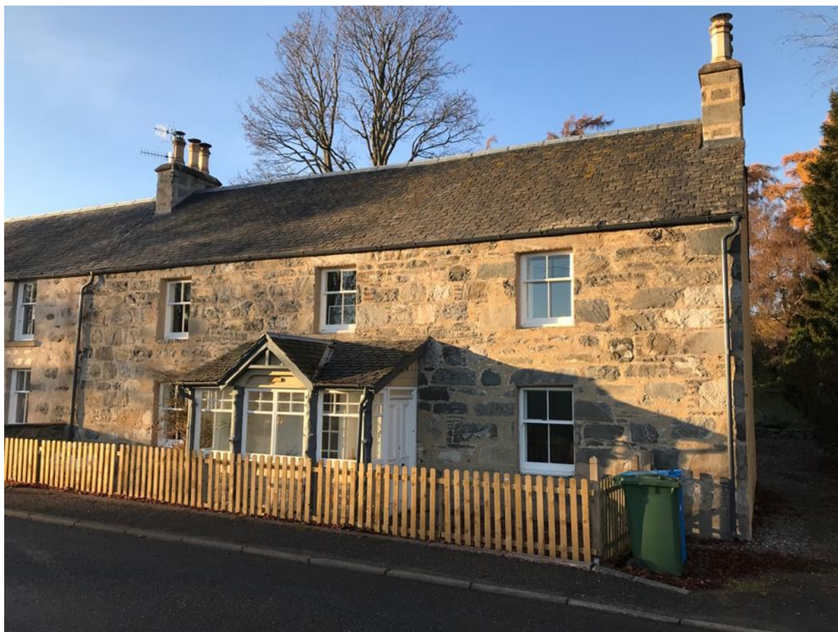
Figure 043.1. The cottage, with recently repaired ruled sneck harl.
