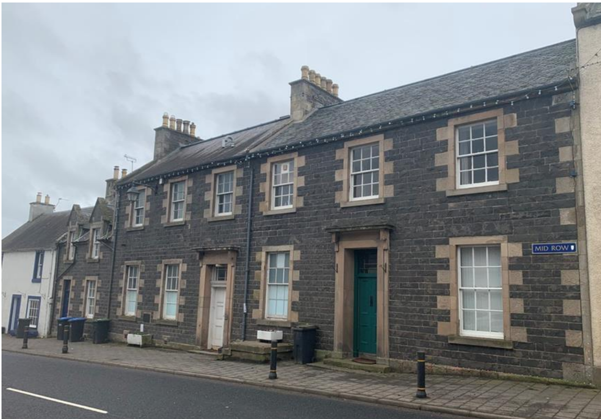
Figure 035.1. A pair of houses on Mid Row, Lauder, viewed from the north-east.
