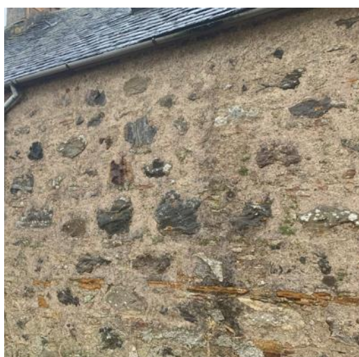
Figure 129.2. Rear elevation showing sneck harl and masonry.
