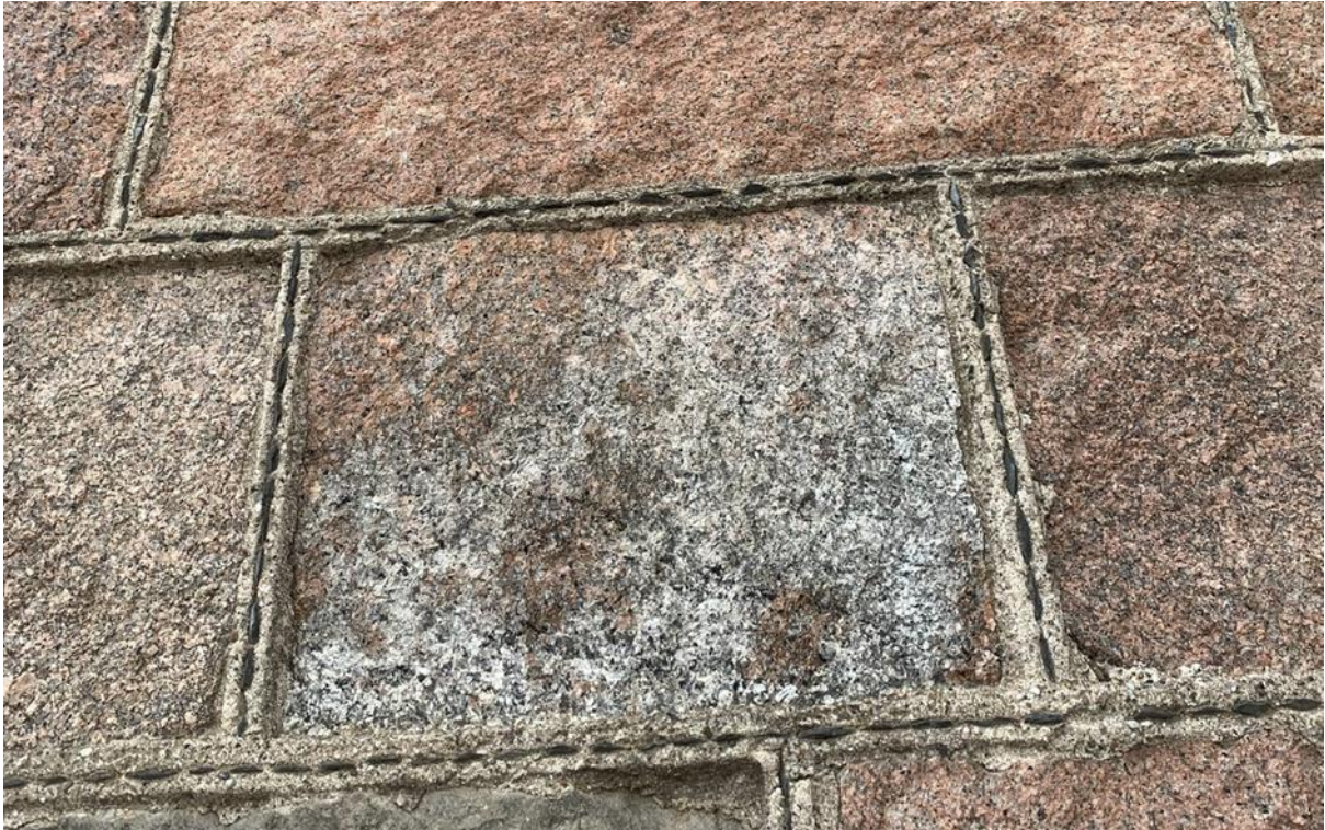
Figure 021.2. Raised ribbon lime finish with slate cherry-cocking.
