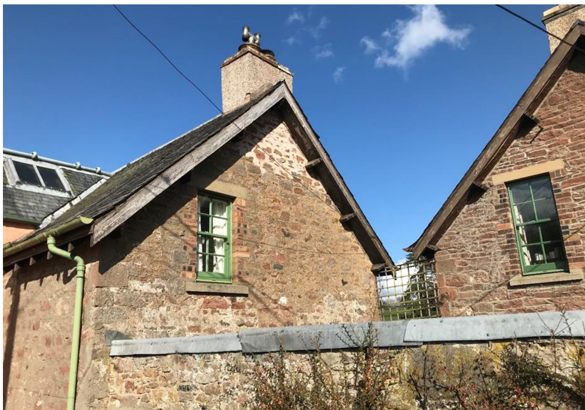
Figure 007.1. The Gable end of one of the stable cottages.
