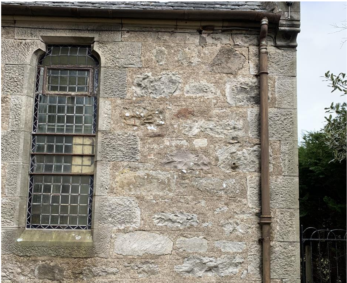
Figure 101.4. Associated building, wider sneck-pointed rubble, ruled out horizontally aligned with the sandstone dressings.
