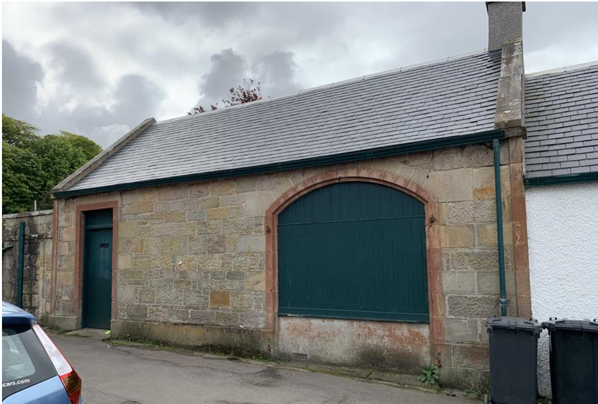
Figure 124.1. Small single storey carriage house, Largs.
