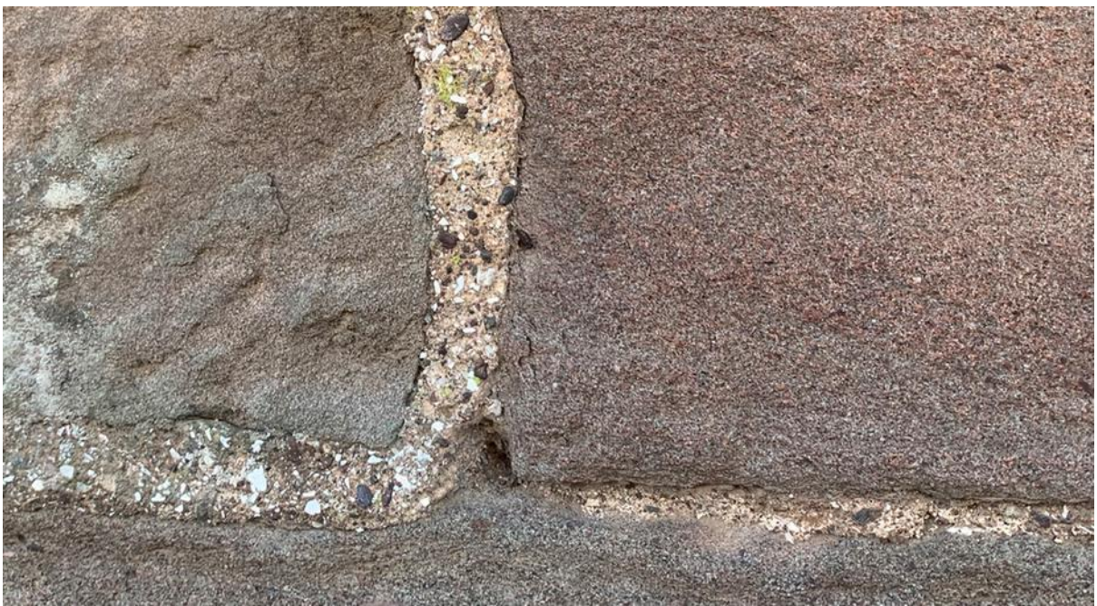
Figure 063.3. Shrinkage cracks.
