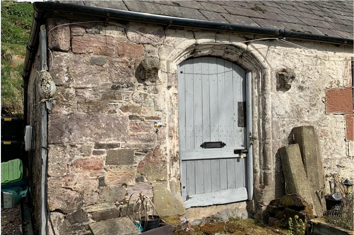
Figure 037.2. The re-used door surround; flush pointing and limewash surviving on the right-hand side.
