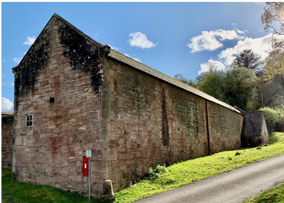
Figure 095.1. Drumlanrig Mains, the former sawmill range, north west corner.
