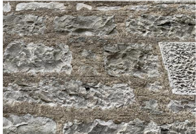
Figure 101.3. Flush and partly rule horizontal pointing on the side elevations.
