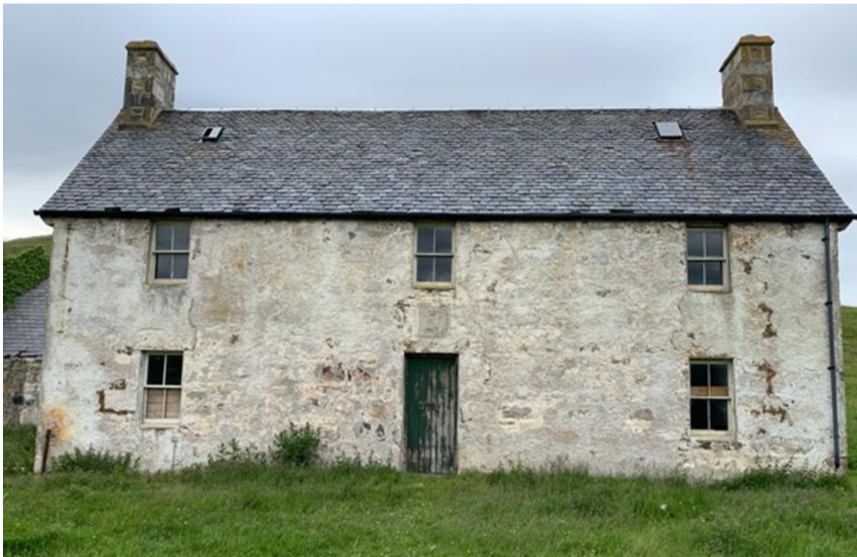
Figure 018.1. The main elevation of the Managers House, dating from the 1830's. The surface finishes survive virtually intact on all elevations.
