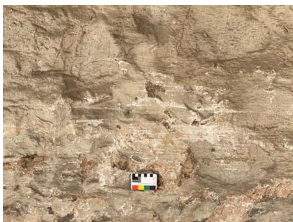
Figure 081.2. A view of the close wall, showing the overall finish.
