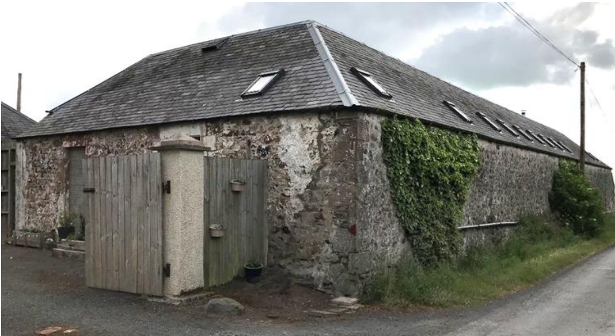
Figure 085.1. The north range of the former steading at Ladyrigg.
