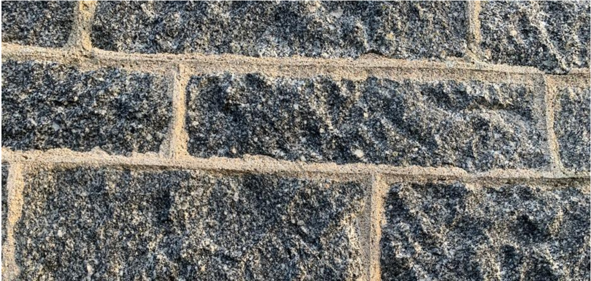
Figure O61.2. Flush point with raised ribbon.
