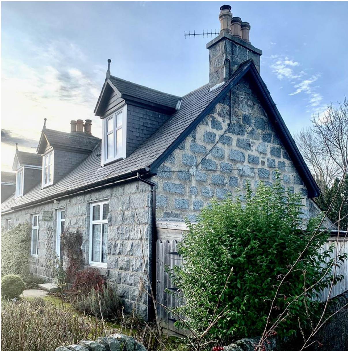
Figure 112.1. Northeastern corner of the cottage.
