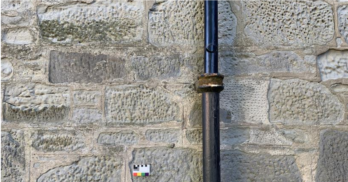
Figure 034.2. Side elevation with some remaining lime pointing.
