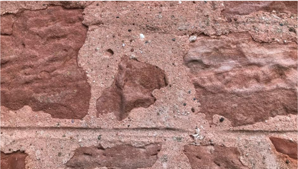
Figure 106.3. Fine and coarse sand with shell inclusions.
