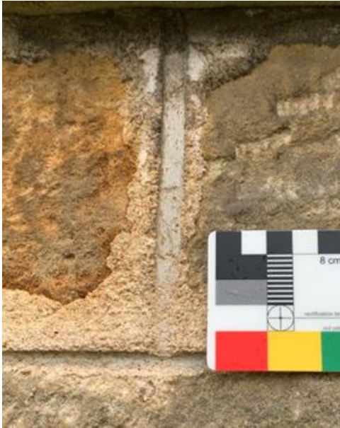
Figure 100.2. Flush pointing ruled out and white lined on the principal elevation.
