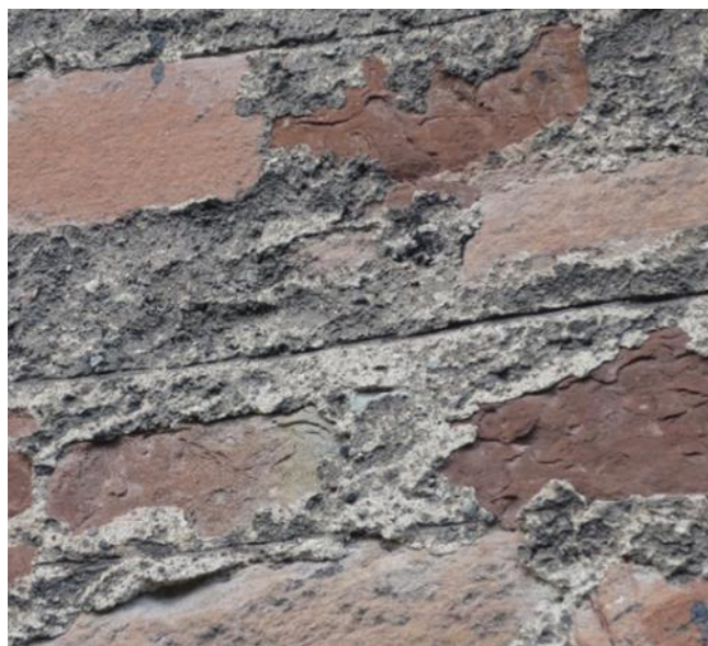
Figure 055.3. West gable, harling and ruled finish.
