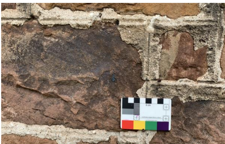
Figure 108.5. Flush-pointed and ruled out mortar, showing the aggregate and lime inclusions.
