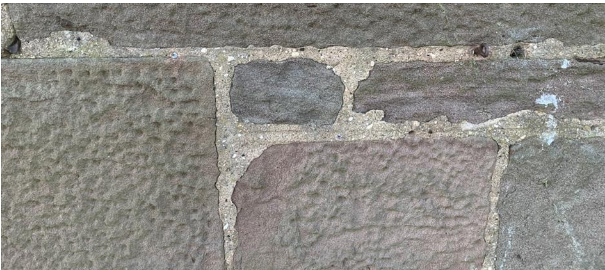
Figure 115.2. Ruling out and lime inclusions.
