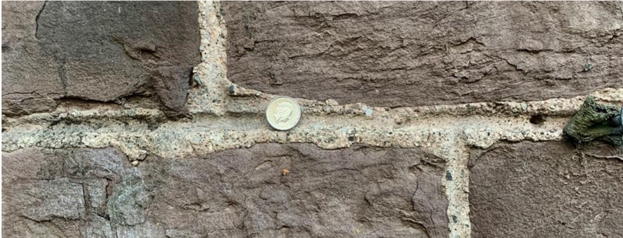
Figure 072.2 Waxy mortar on front elevation with ruling out.
