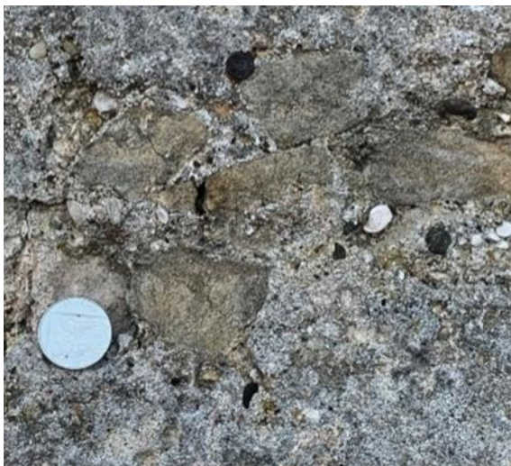
Figure 010.3. Coal inclusions in the aggregate.
