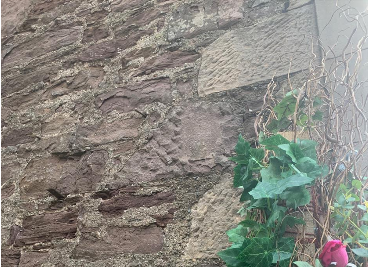
Figure 030.2. Finish on the north gable; this may be the remains of a flush point.
