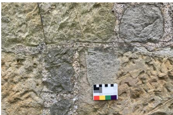
Figure 124.2. Flush pointing and horizontal ruling out.
