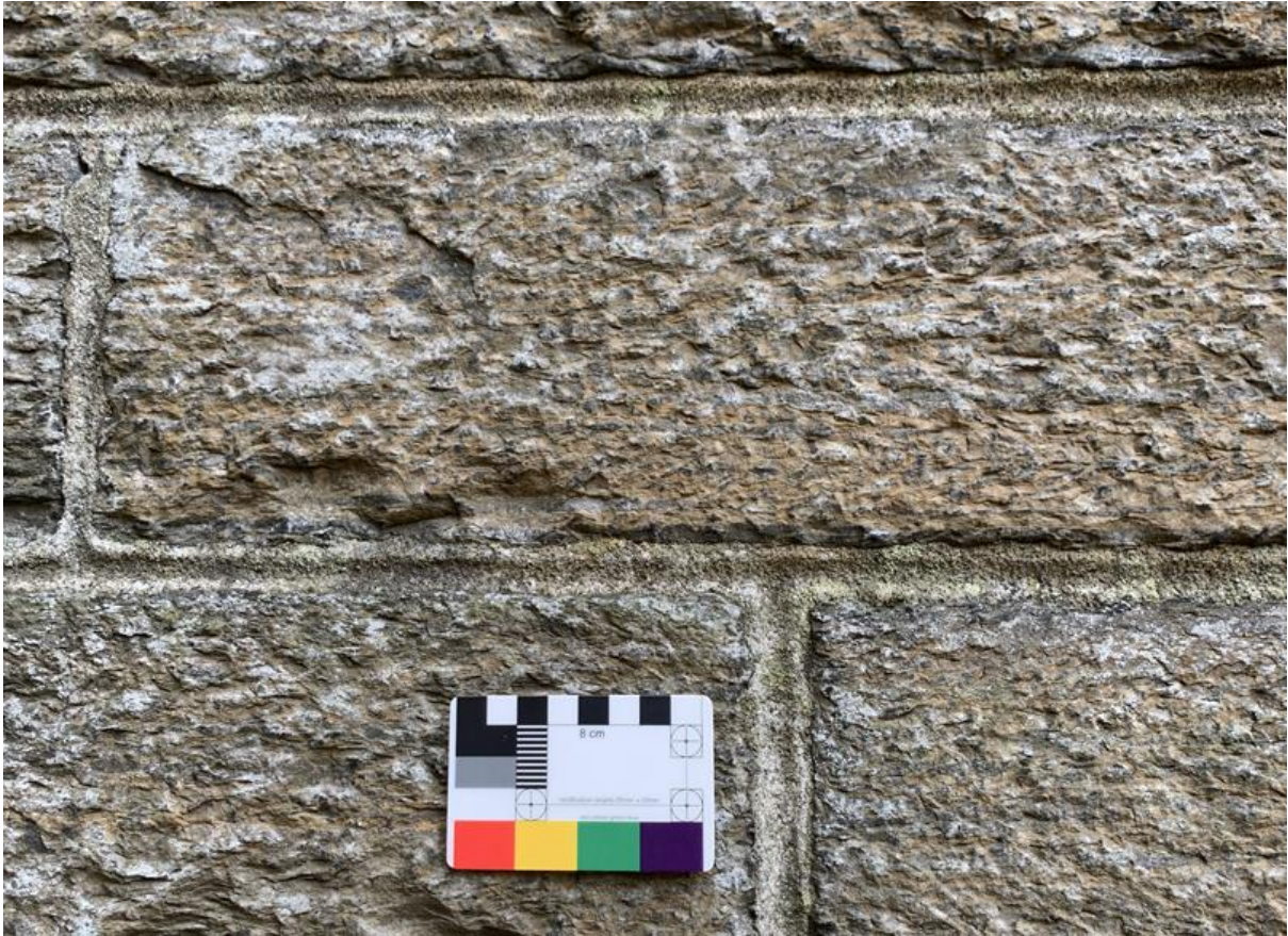
Figure 099.2. Mortar with horizontal and vertical ruling out and crisp joints.
