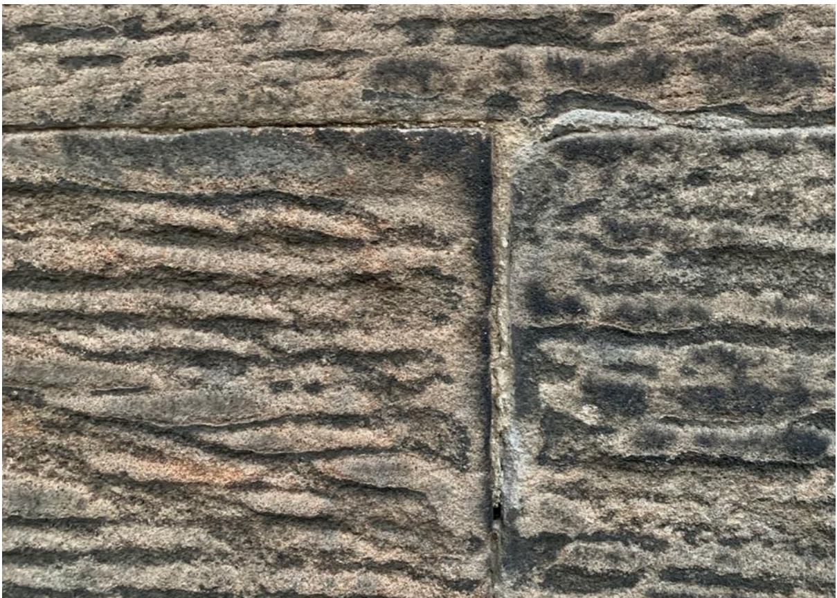
Figure 029.3. The finer ashlar joints on the front elevation.
