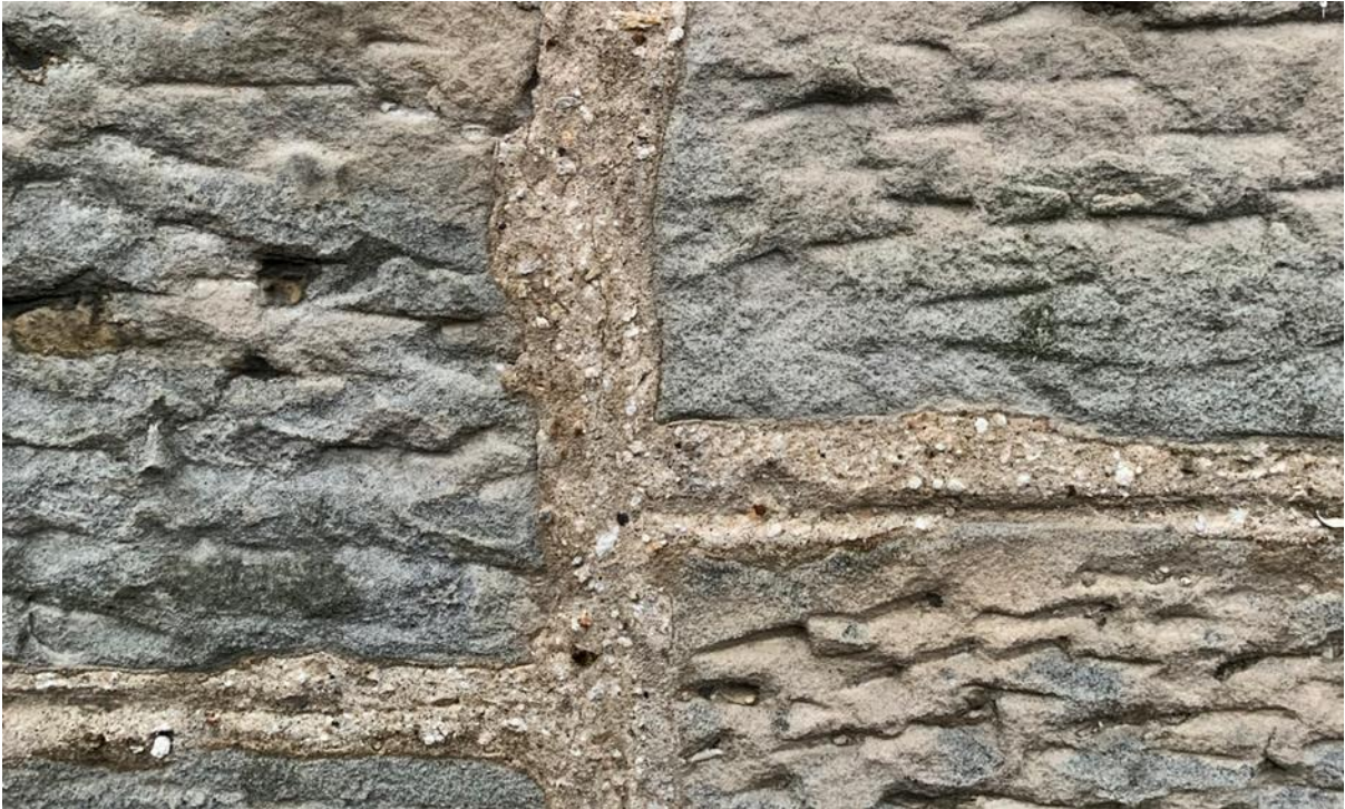
Figure 029.2. Ruling out of the joints on the gable.
