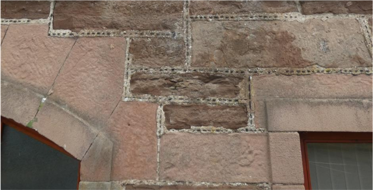
Figure 004.2. Finely detailed masonry and precise cherry-stoning.
