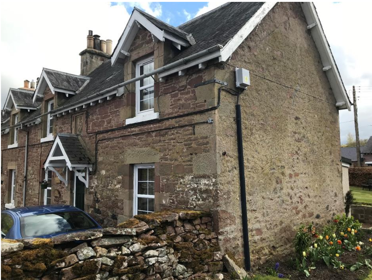
Figure 036.1. Carter Road, Bonchester, a 2 story cottage with a later Victorian first floor and post war sneck harl in a cement based mortar to the gable. Note limewash on original ground floor.
