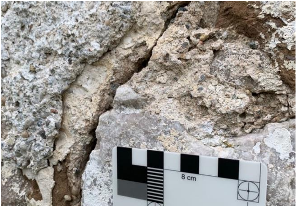
Figure 018.3. The first coat of integrated harl, with cream limewash overlay and final coat of harl.
