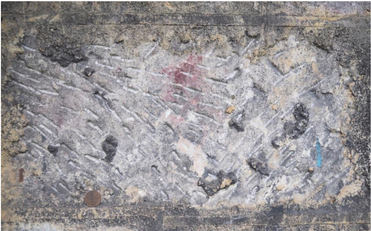
Figure 078.3. Evidence of full lime covering on face of stone, with later ribbon pointing. Image © Sweyn Ross
