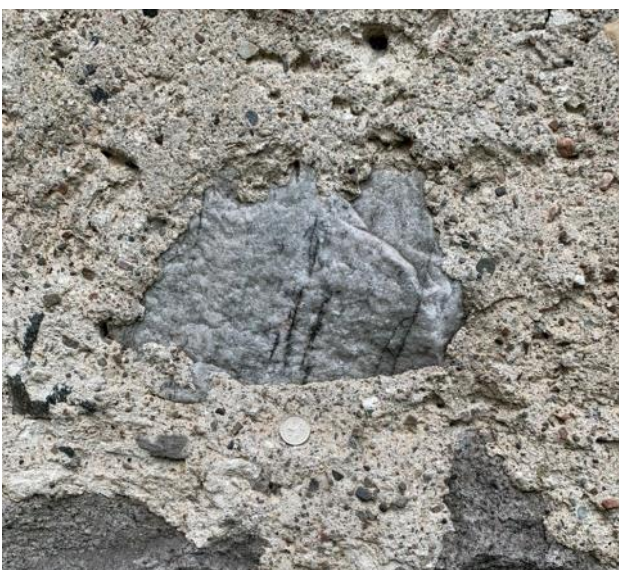
Figure 049.2. Very coarse angular sneck harl.
