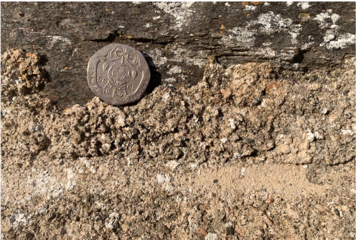
Figure O25.3. Remains of a limewash in the ruling out.
