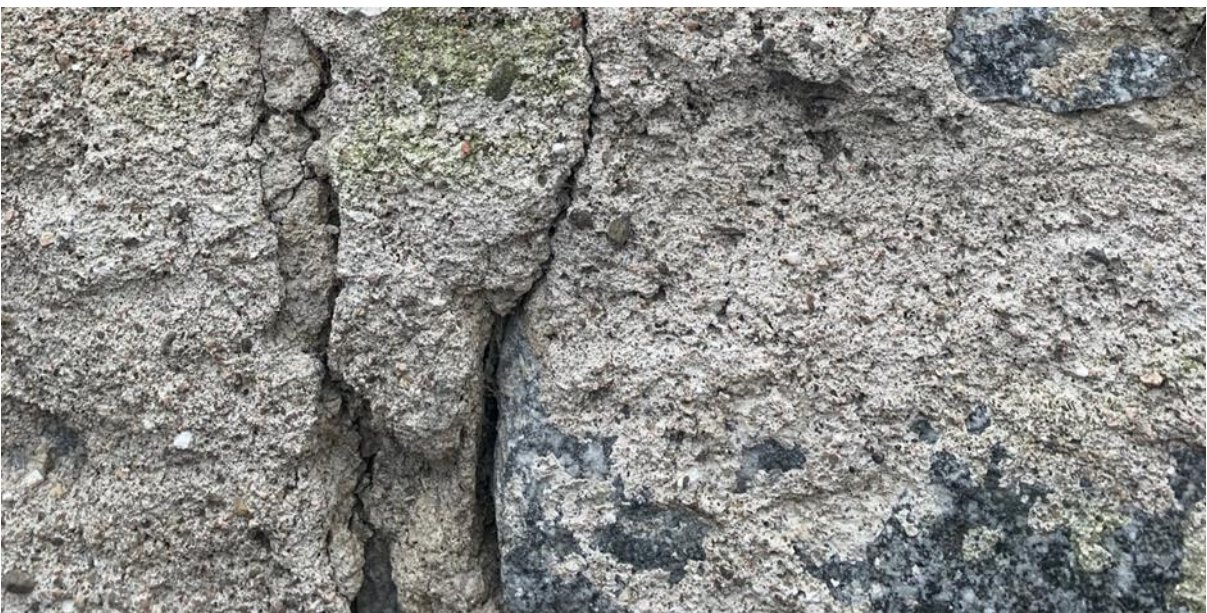
Figure 022.3. Sharp, well graded aggregates with lime inclusions.
