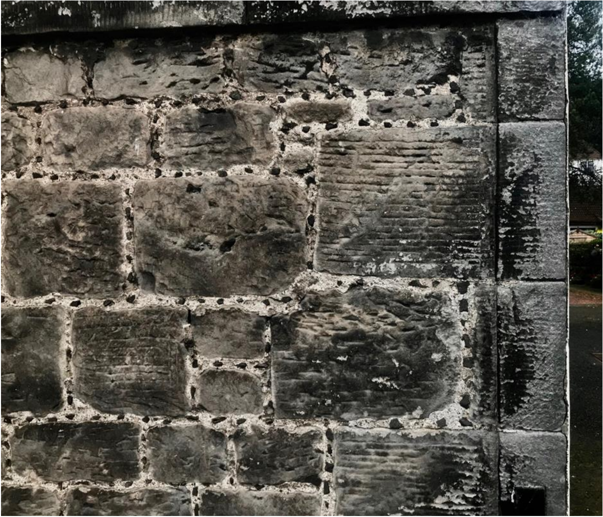
Figure 041..2. Sandstone ground floor, cherry-stoned with basalt.
