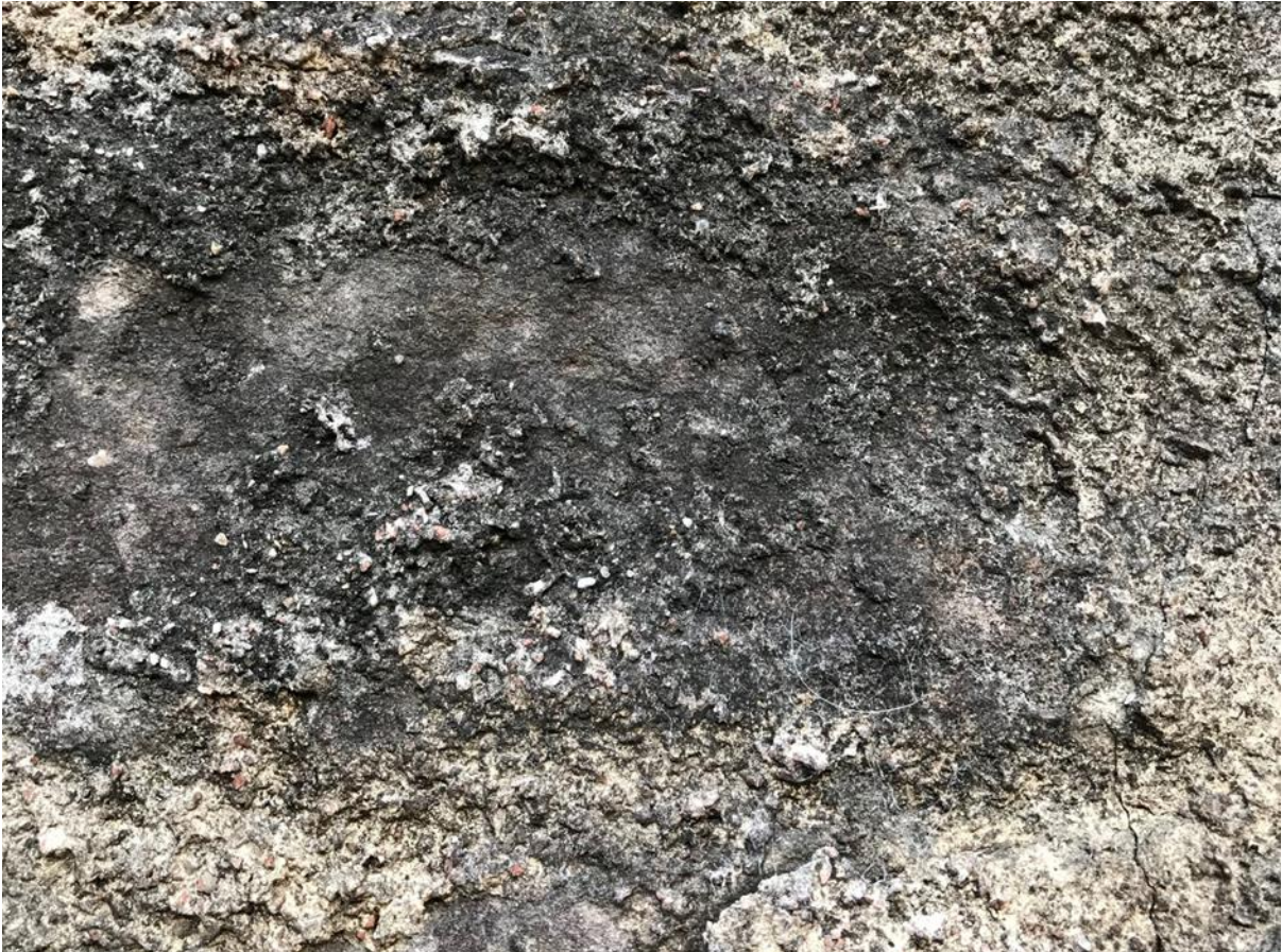
Figure 052.2. Sneck harl or possibly graded away full harl.
