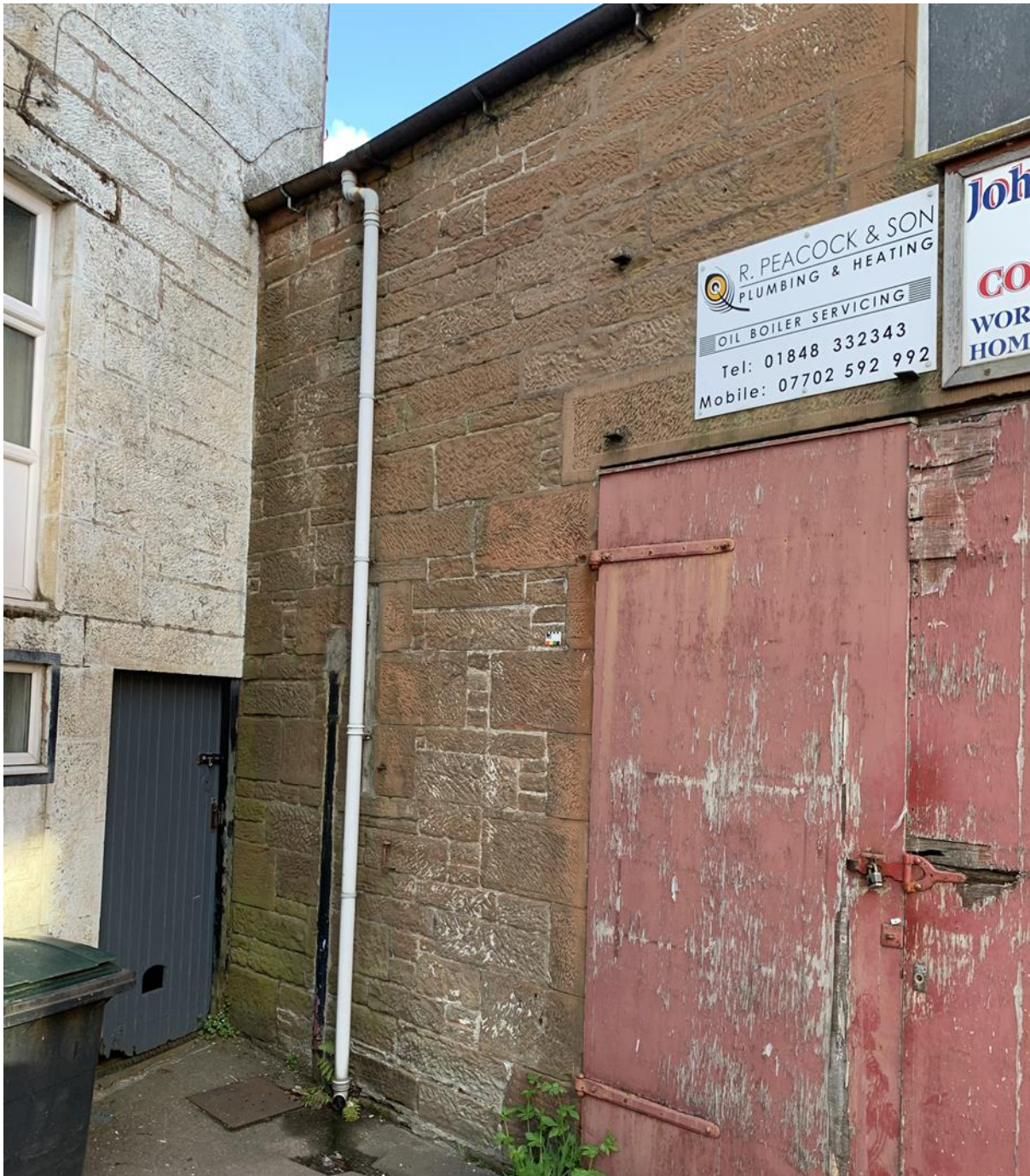
Figure 126.1. The wall of the workshop showing remains of limewash.
