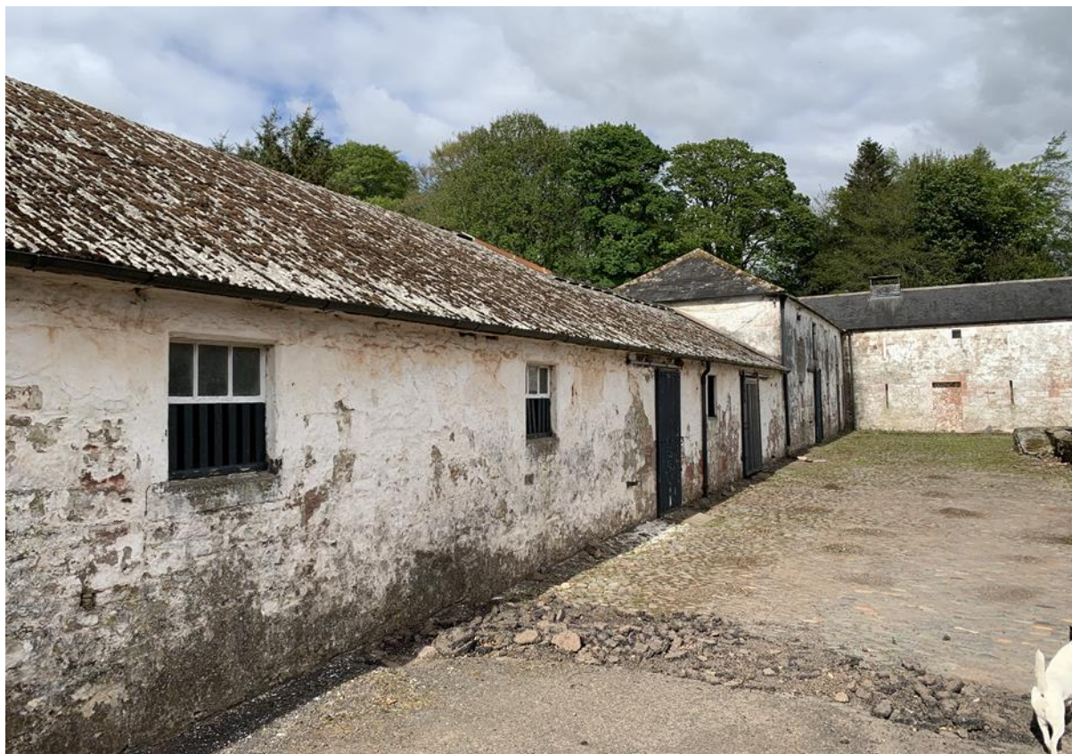
Figure 038.1. View of the North West range of the Coshogle steading where large areas of original finish survive.
