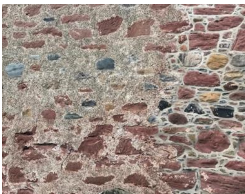
Figure 008.2. Sneck harl with recent lime pointing.
