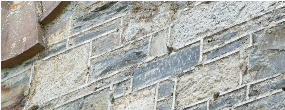
Figure 102.2. Horizontal and perpendicular ribbon work on the front elevation.
