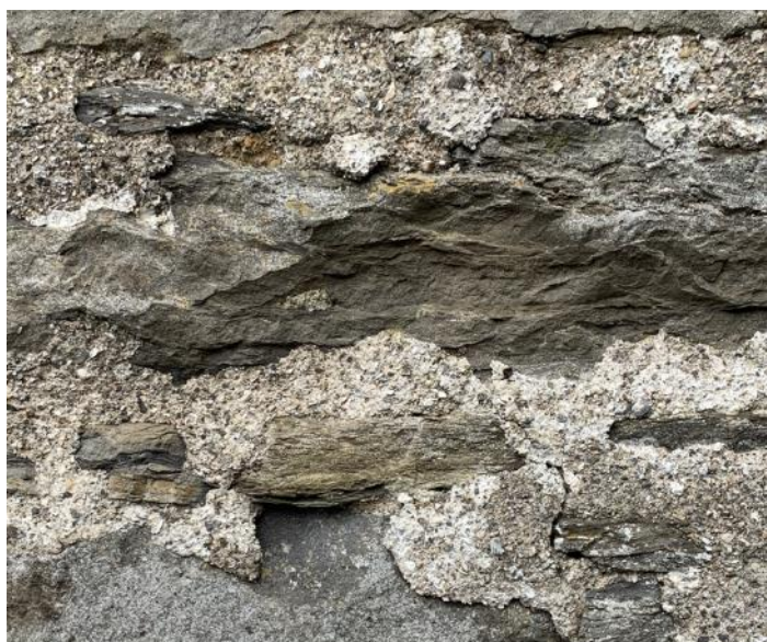
Figure 015.3. Sneck pointing surviving on the more sheltered rear elevation, showing finer aggregate compared to the bedding mortar.
