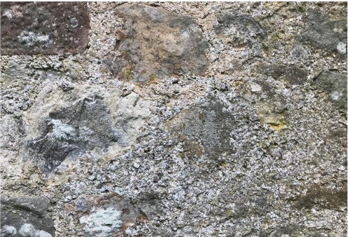
Figure 091.3. A close view of the pointing on the 19th century extension.
