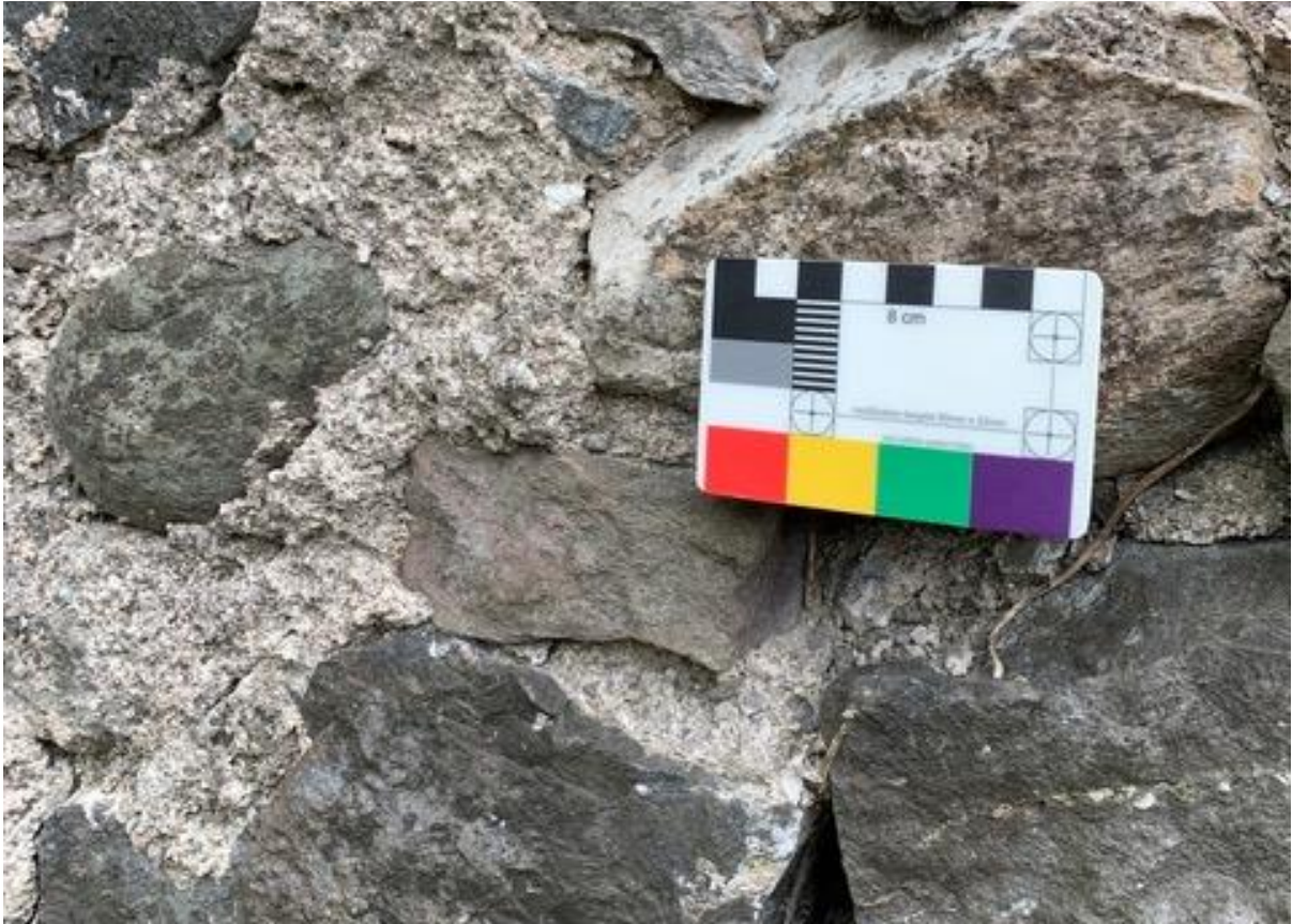
Figure 073.2. Integrated bedding and harling mortar.
