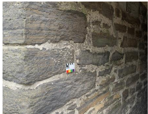
Figure 012.3. The flush pointed masonry finish in the close on the right hand side of the building, showing the hierarchy of finishes.
