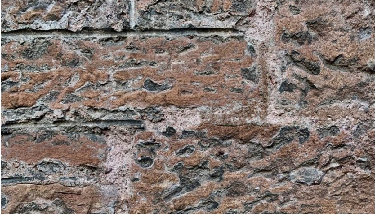
Figure 108.2. Horizontally and perpendicularly ruled flush finish.
