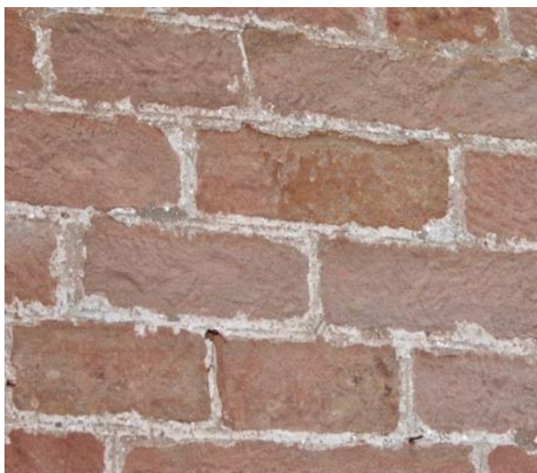
Figure 039.2. Full flush finish with faint horizontal and perpendicular ruling out.
