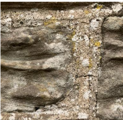
Figure 087.2. Flush finish with the raised ribbon.
