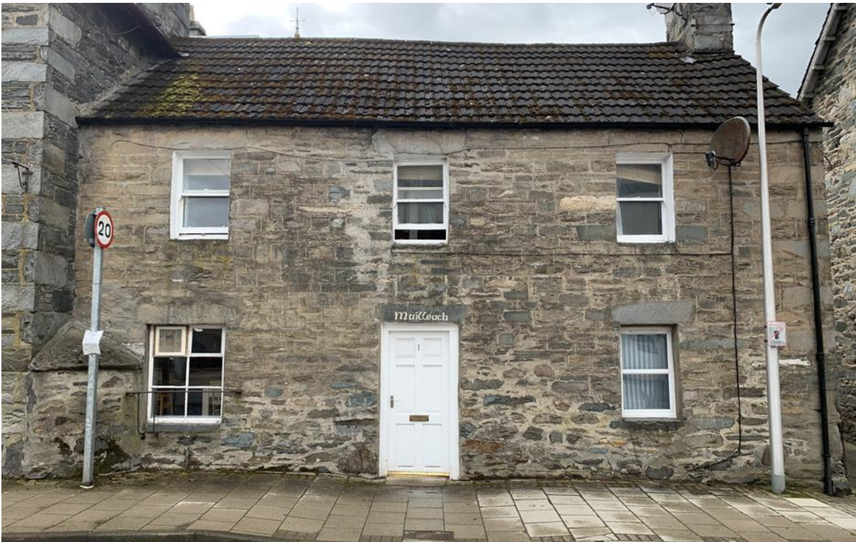
Figure 046.1. The house on Chapel St, Aberfeldy. Flush point with horizontal and vertical ruling out, the pattern of which can still be discerned on the upper levels.
