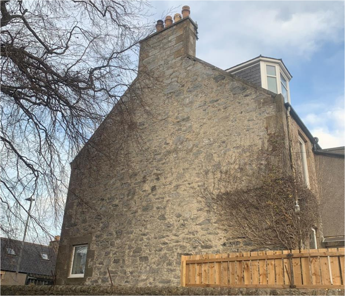
Figure 111.2. Random rubble gable with sneck harl.
