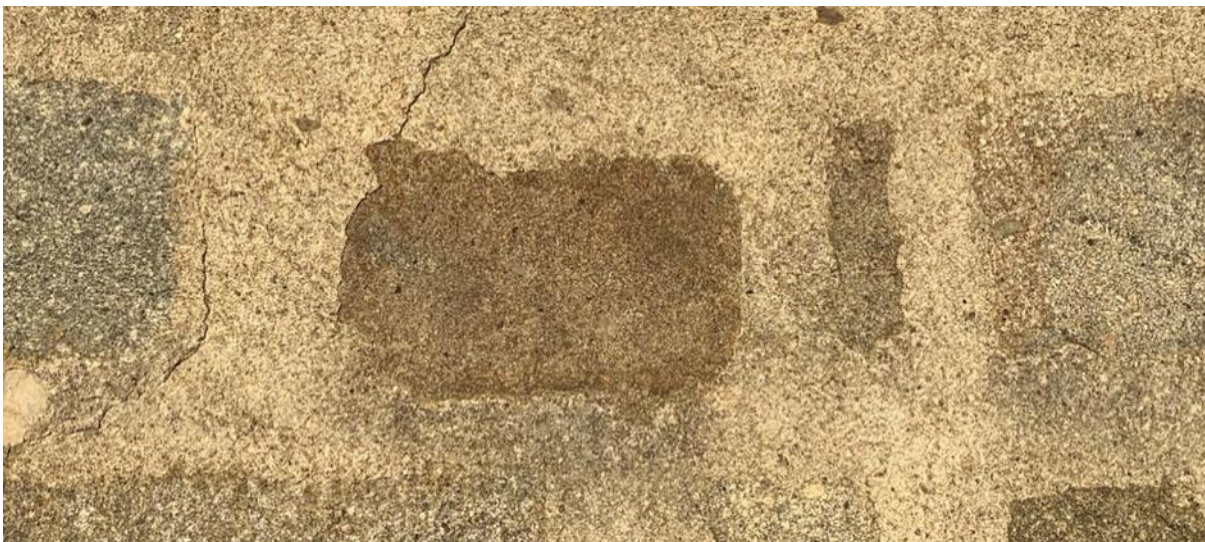
Figure 060.2. Squared sneck harl with sharp, angular aggregates.
