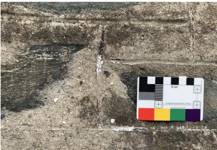
Figure 046.2. Detail of the flush point showing the horizontal and vertical lining out, with traces of white coloring to the incised lines.
