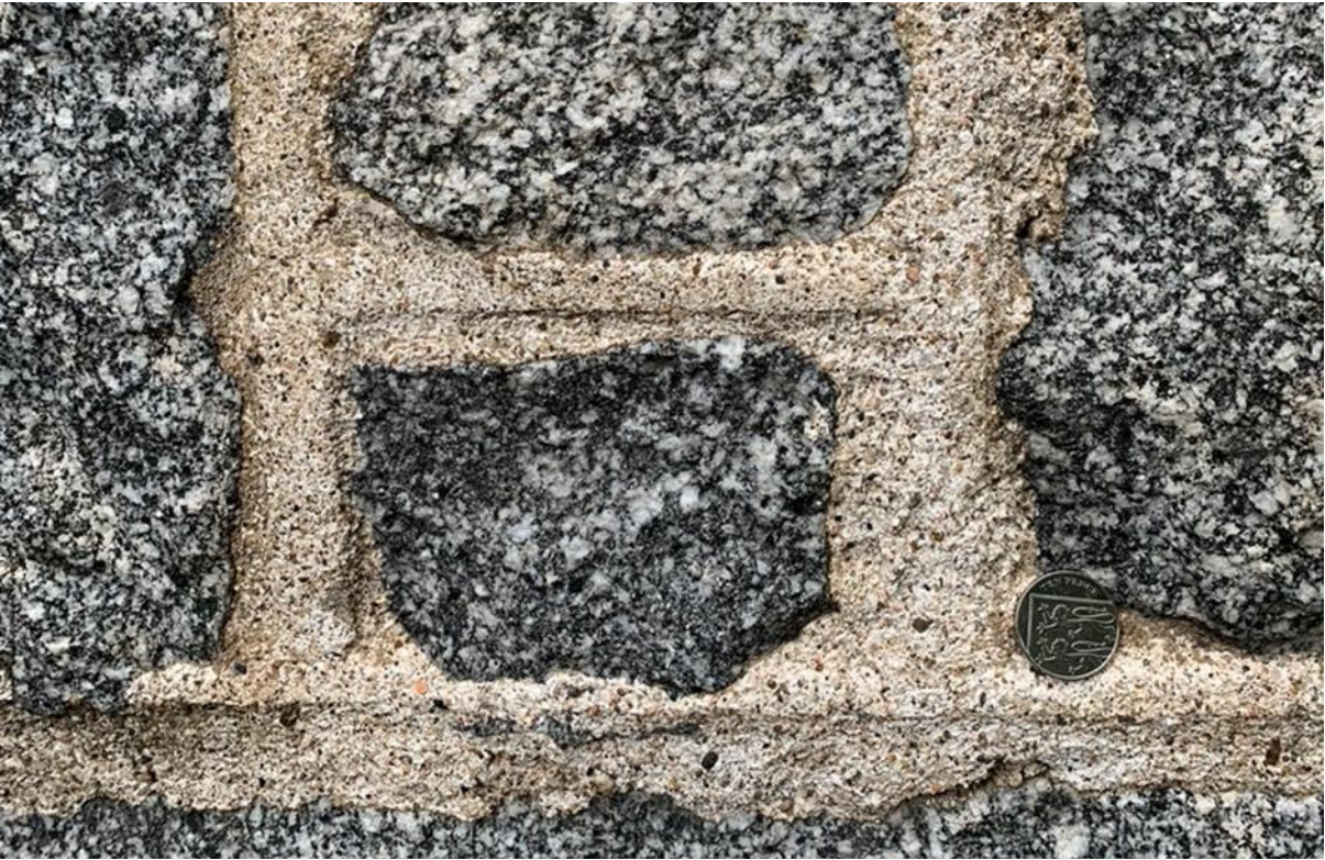
Figure 059.2. Lime mortar ribbon pointing with fine sharp angular aggregates.
