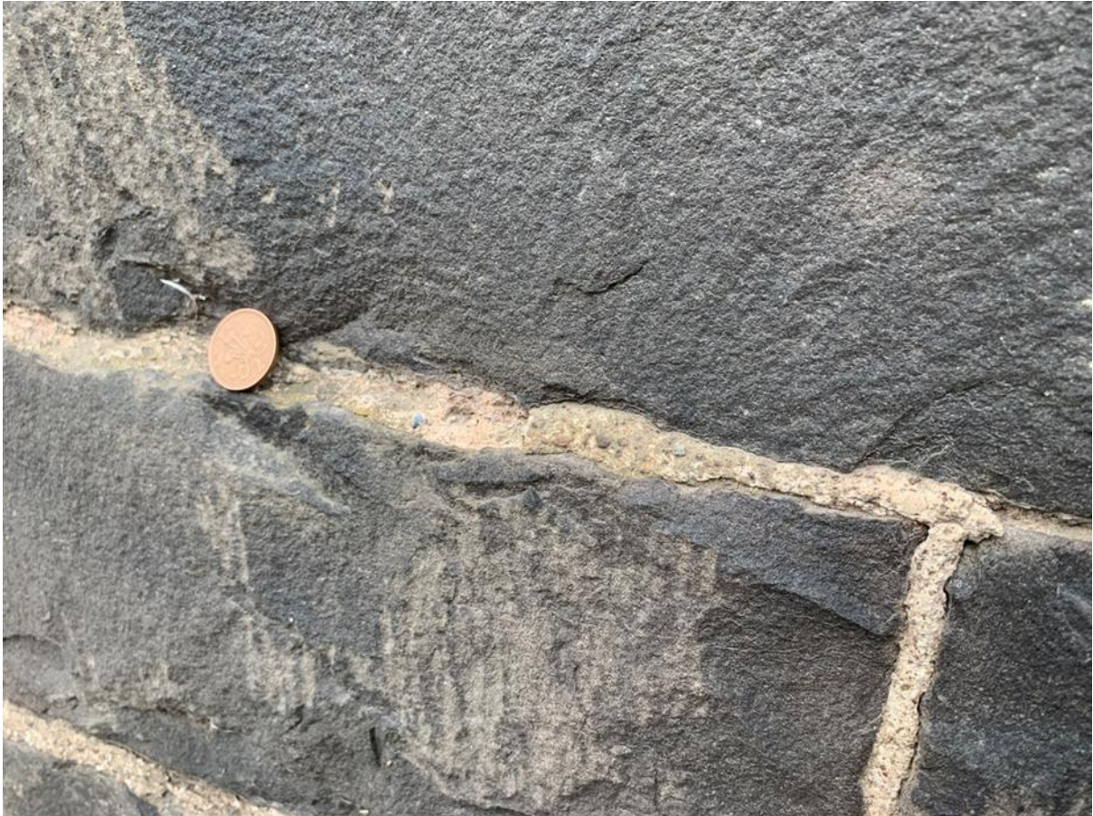
Figure 035.2. Ramped mortar to combat water absorption.
