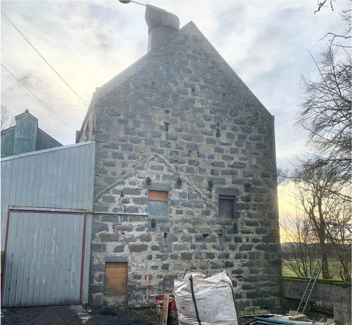
Figure 022.2. Sneck harled granite/gritstone on the northeast gable.
