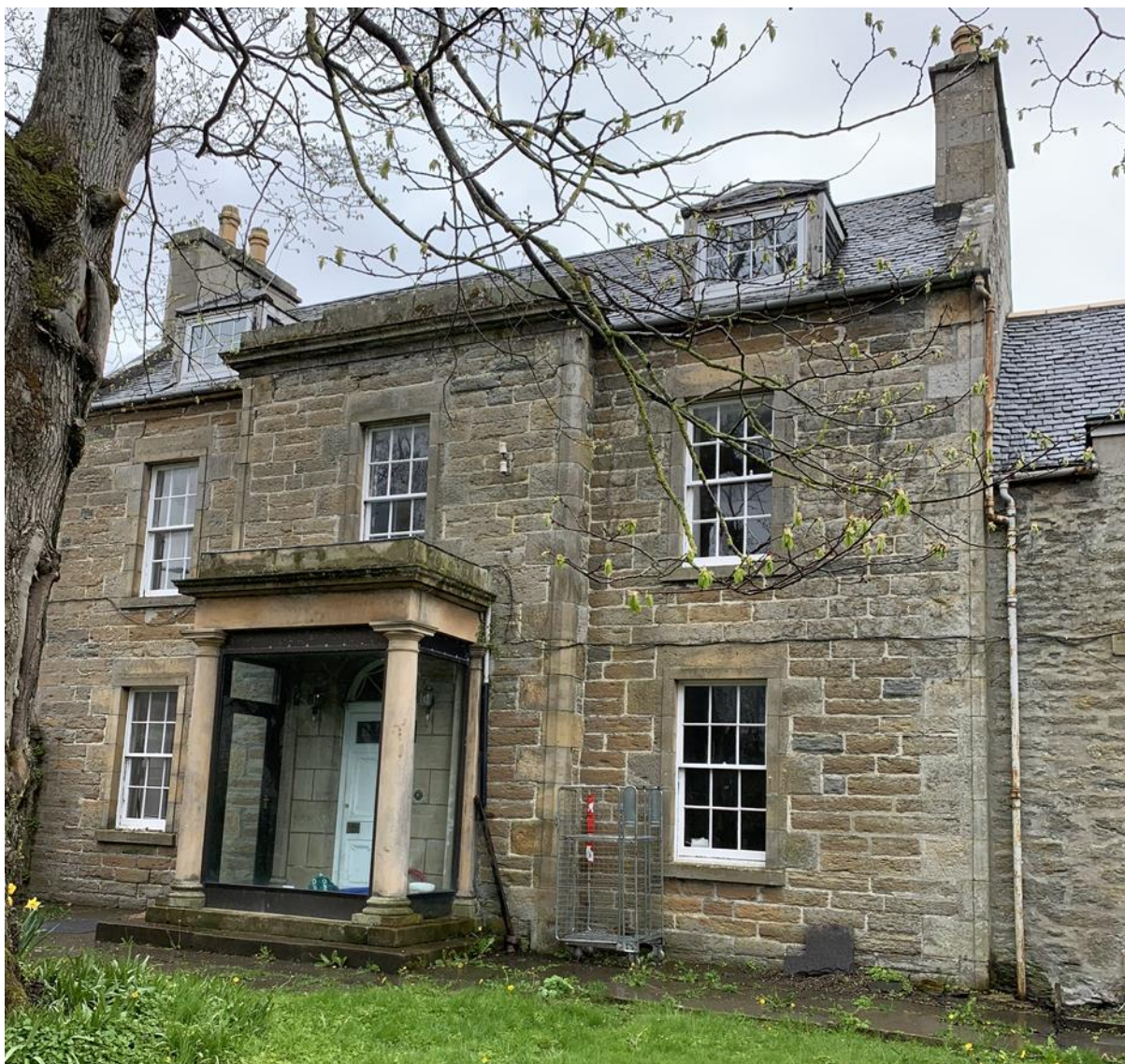
Figure 047.1. Front elevation of building.
