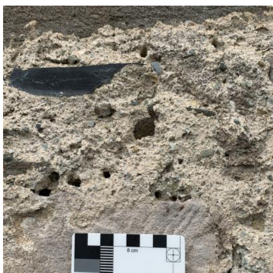
Figure 076.2. Detail of snecked pointing, showing the aggregate.
