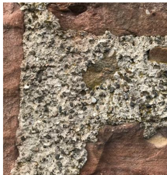
Figure 051.3. Original extant pointing sample.
