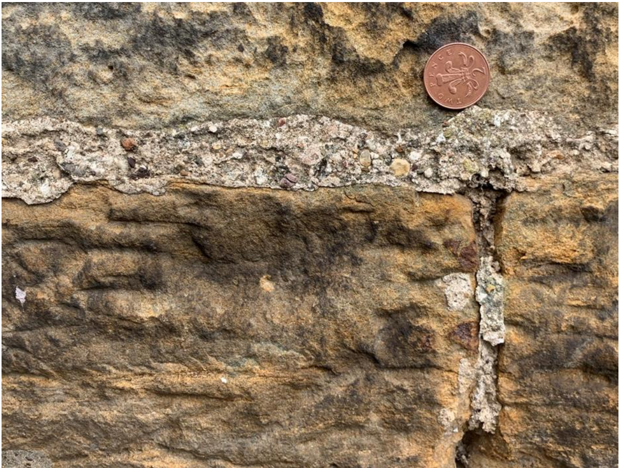
Figure 080.3. Coarse angular and rounded aggregate.
