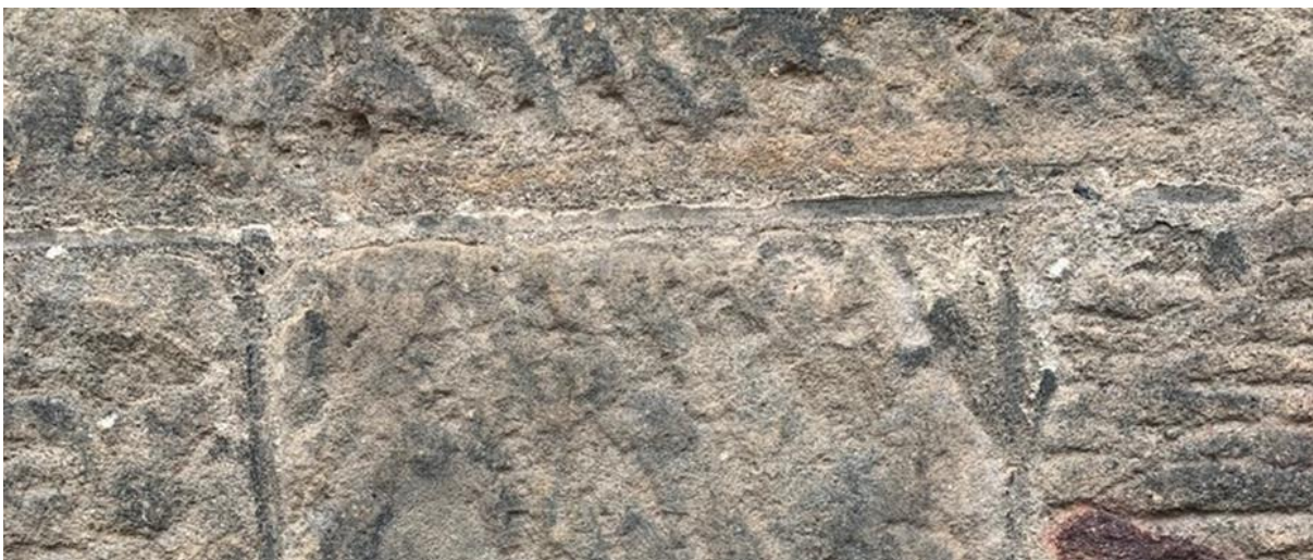
Figure 033.2. Horizontally and perpendicularly ruled flush joints.
