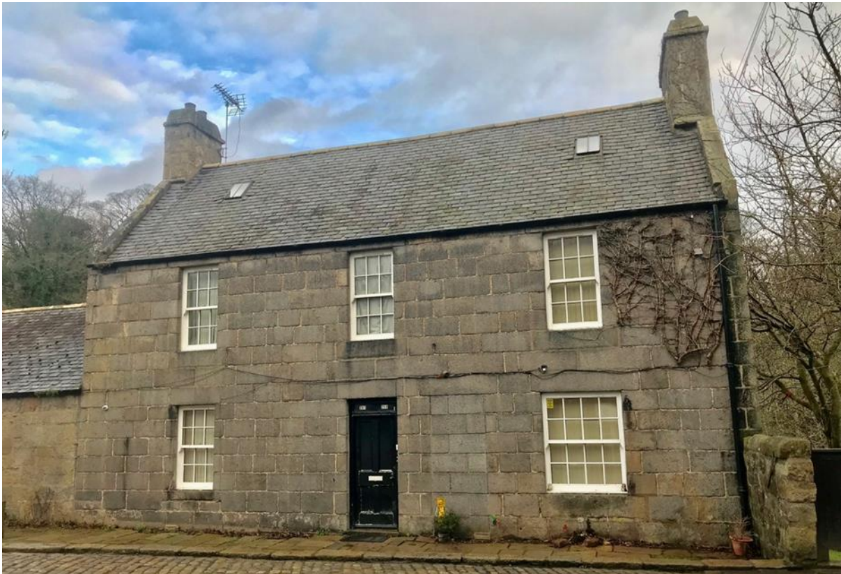
Figure 006.1. Southwest elevation of the house.
