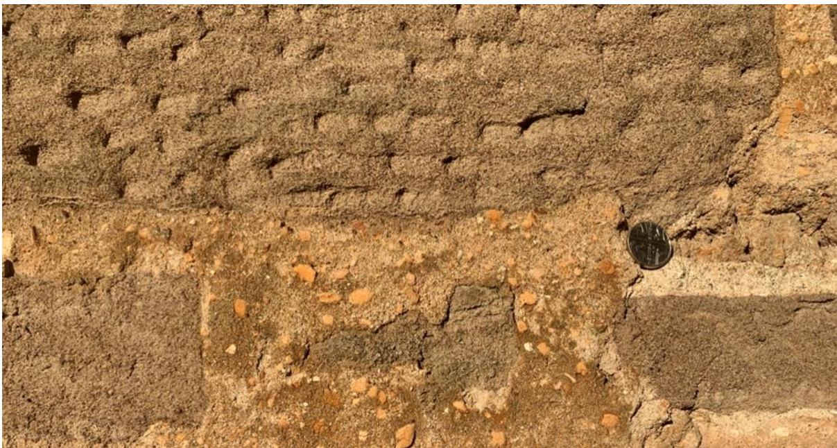
Figure 065.3. Later buff pointing finish overlaying the construction mortar.
