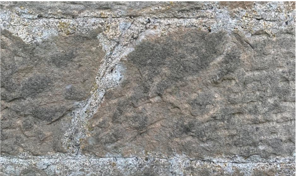
Figure 121.3. Ruling out even on angled junctions.
