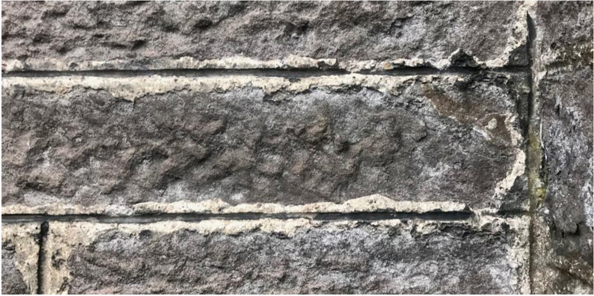
Figure 069.2. Flush lime finish with horizontal and perpendicular ruling out.
