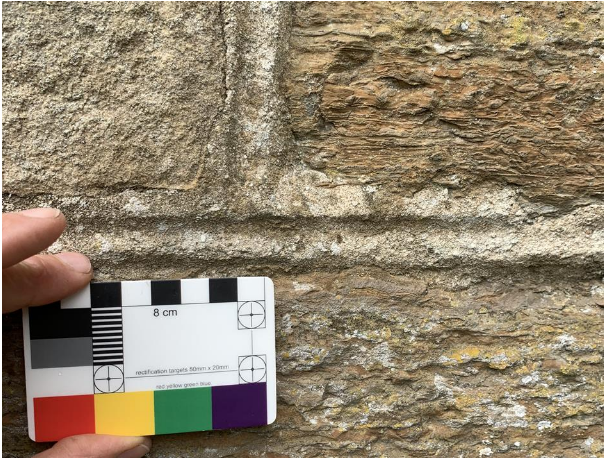
Figure 047.2. Flush pointing lined horizontally and vertically.
