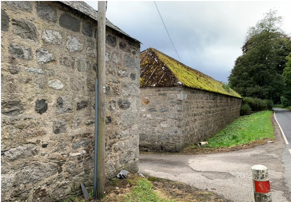
Figure 024.1. Two periods of construction with two different point styles.
