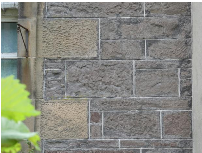
Figure 120.2. Flush pointing and ruling out with whitened lines. Note the relationship between the rubblework and the better quality masonry around the windows and doors.
