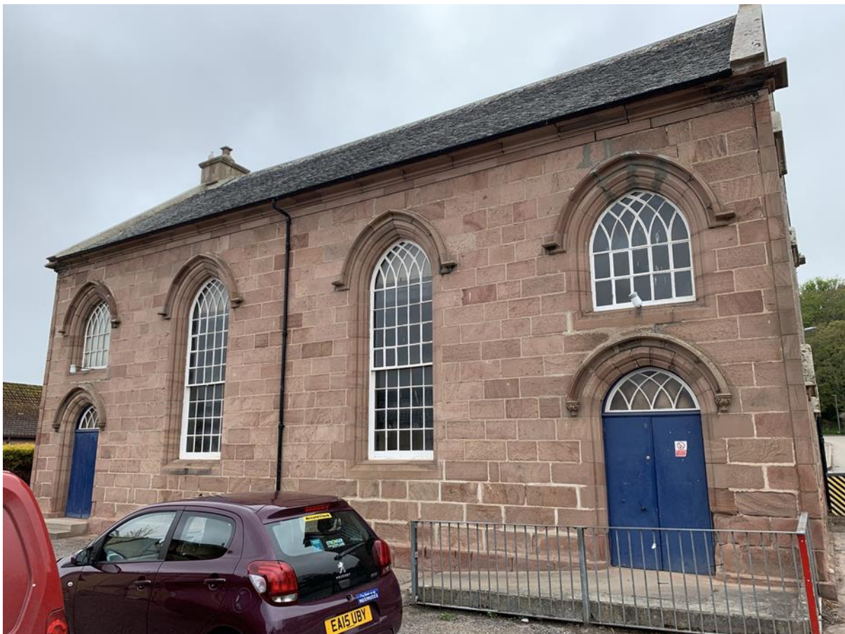
Figure 050.1. The principal elevation of the former Town Hall.
