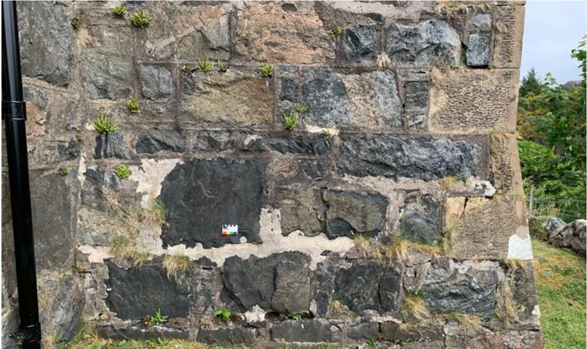
Figure 104.2. Later raised ribbon pointing seen in the upper part of the image, with earlier flush pointing seen lower down, showing much brighter.
