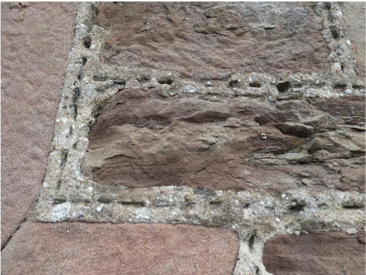
Figure 004.3. Fine sand with shell and lime inclusions.
