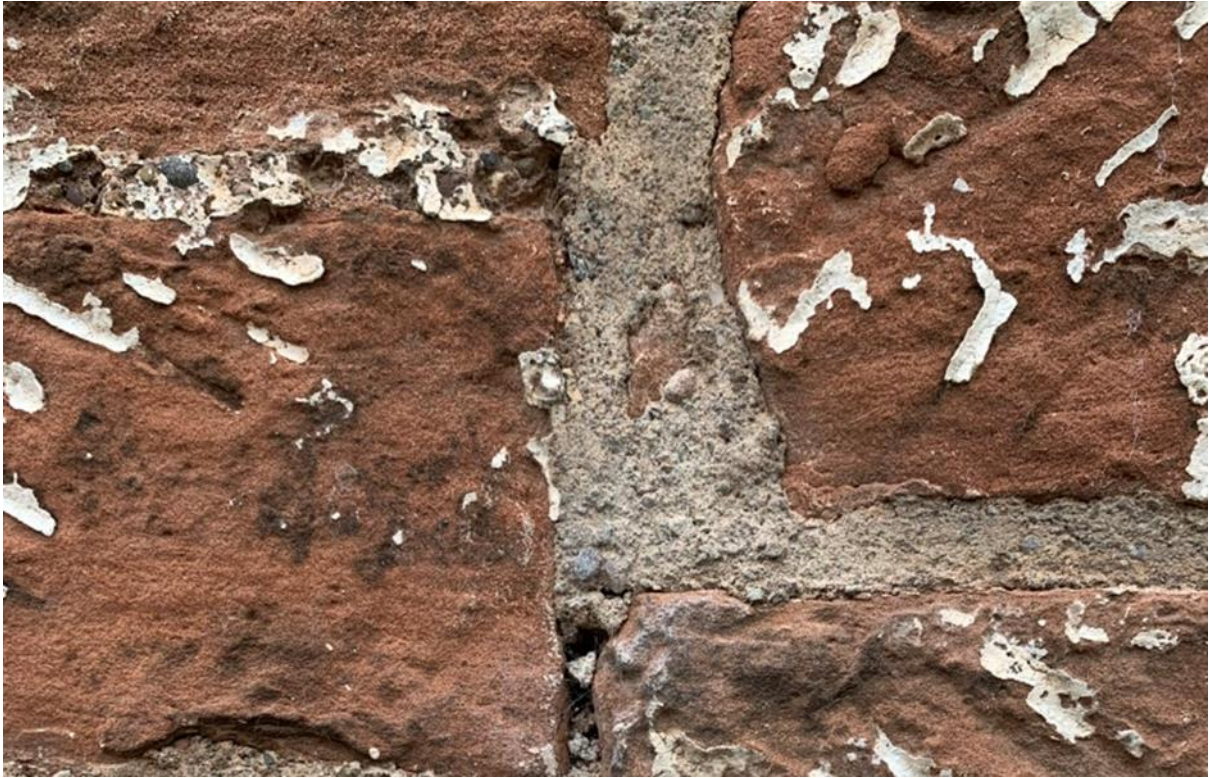
Figure 040.2. Later pointing from 2007 alongside historic evidence for limewash and a flush point.
