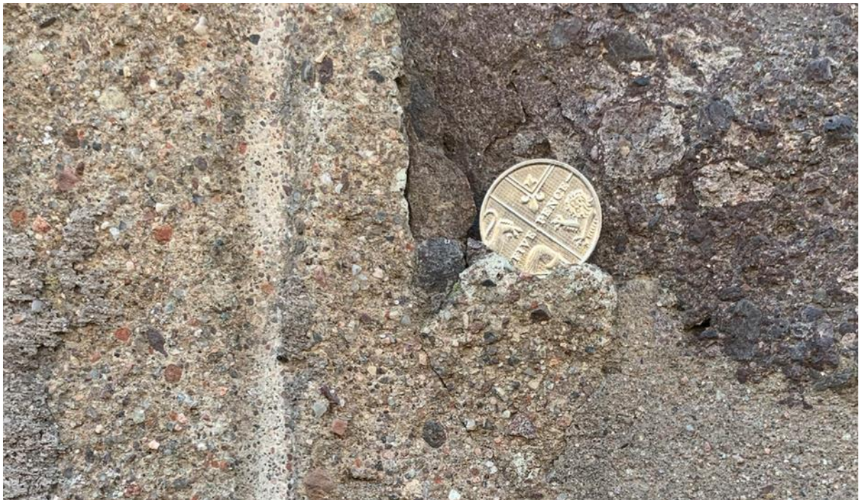
Figure 064.3. Limewash to accentuate the ruling out.
