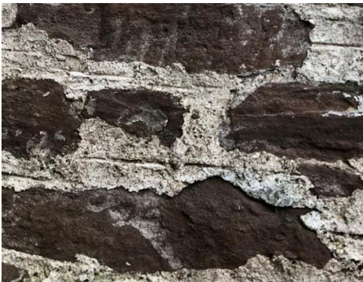
Figure 071.2. Detail of the flush finish with informal ruling out.
