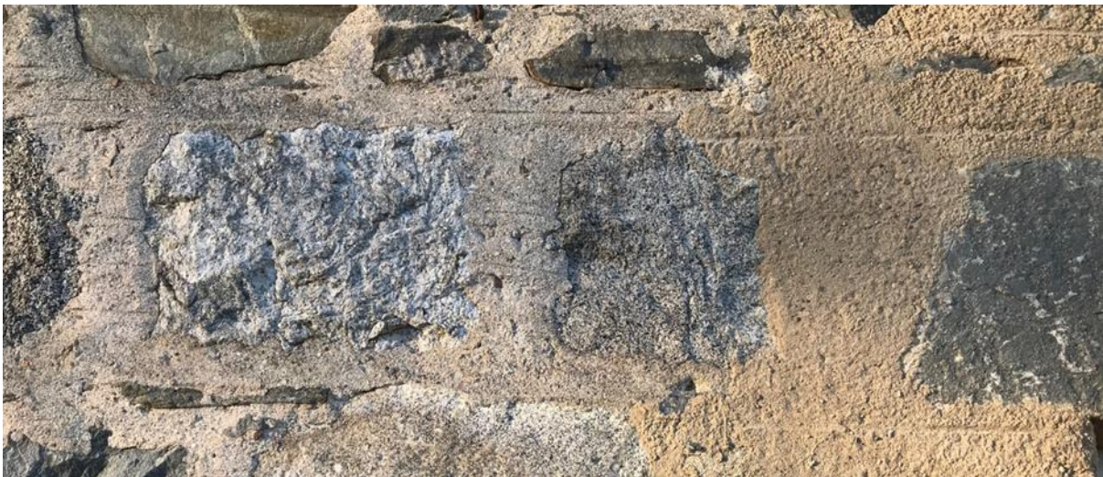
Figure 043.3. Semi-formal ruling out of the original sneck harl to the left and recent lime mortar repair to the right.
