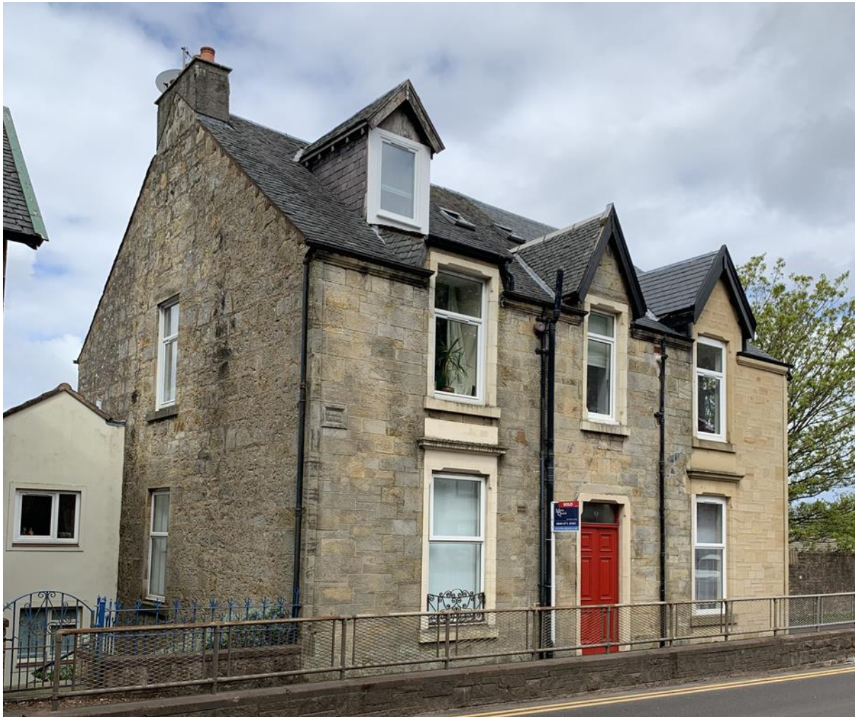
Figure 125.1. Formal front and informal gable of the villa on Main Road.
