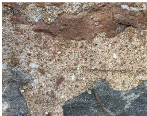
Figure 045.2. Extant ruled sneck pointing made with medium fine shell sand
