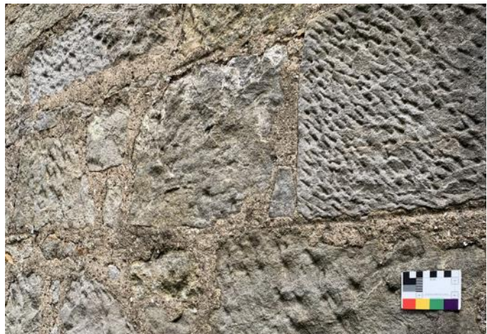
Figure 103.2. Horizontal ruling out on the gable side.
