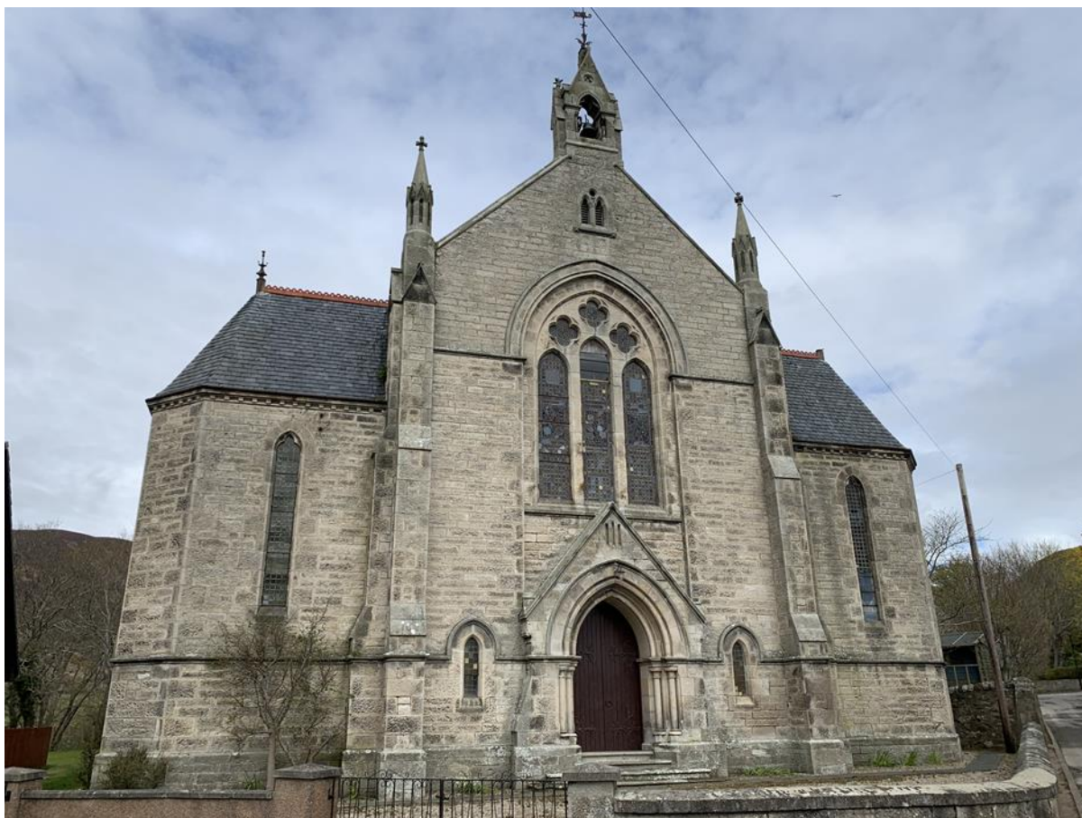
Figure 101.1. The principal elevation of the church.
