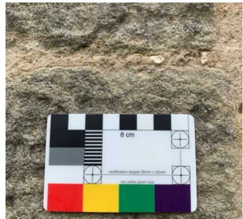
Figure 123.3. Close up of a joint showing the flush finish.
