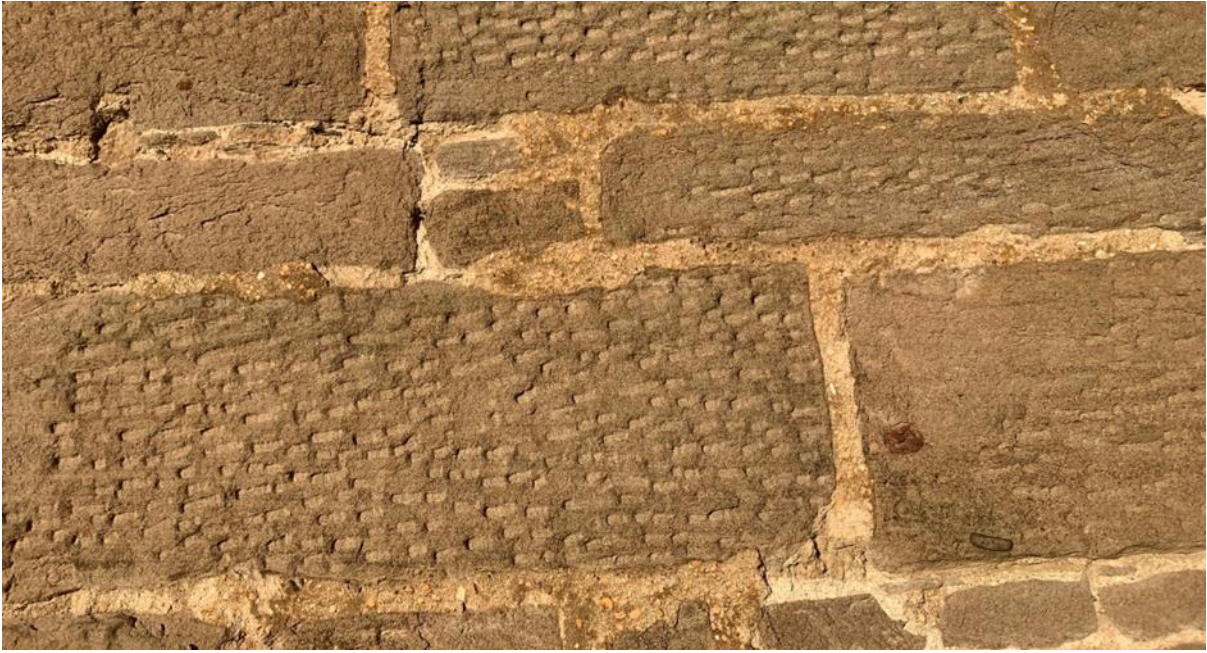
Figure 065.2. Sawn rubble walls with lime mortar.
