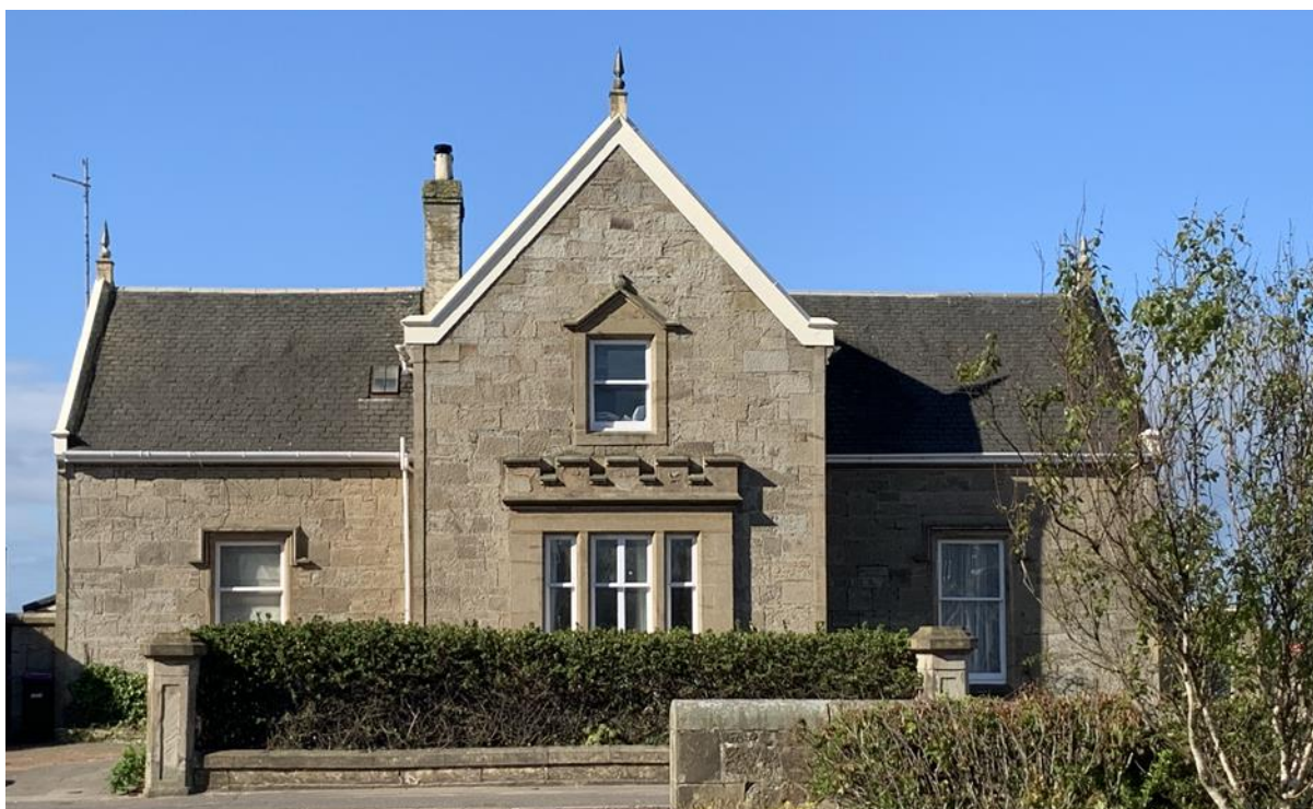
Figure 082.1. The road side elevation of the villa on South Beach.
