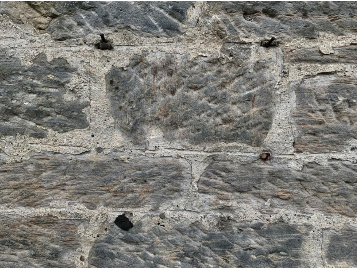
Figure 122.3. Detail of horizontal ruling as well as lime, coal and marine inclusions.
