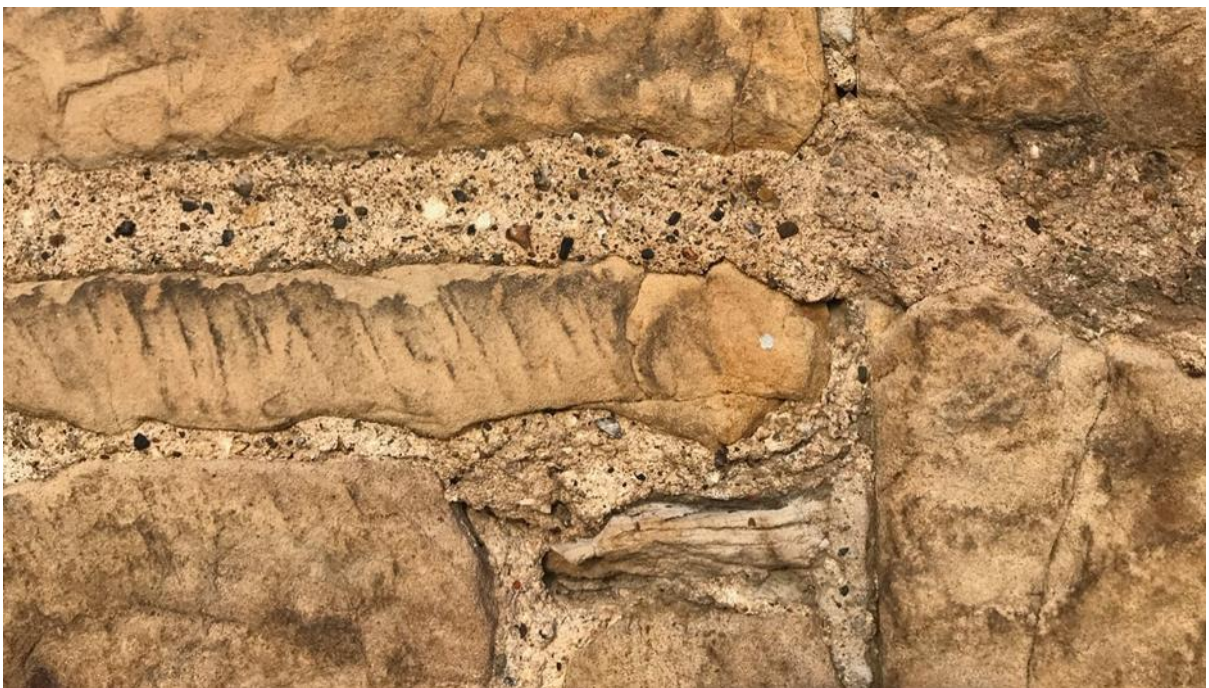
Figure 075.3. Coal, lime and shell inclusions.
