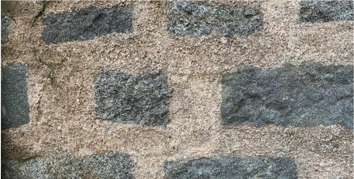
Figure 113.2. The squared sneck harl. Coarse, angular sand with lime inclusions.
