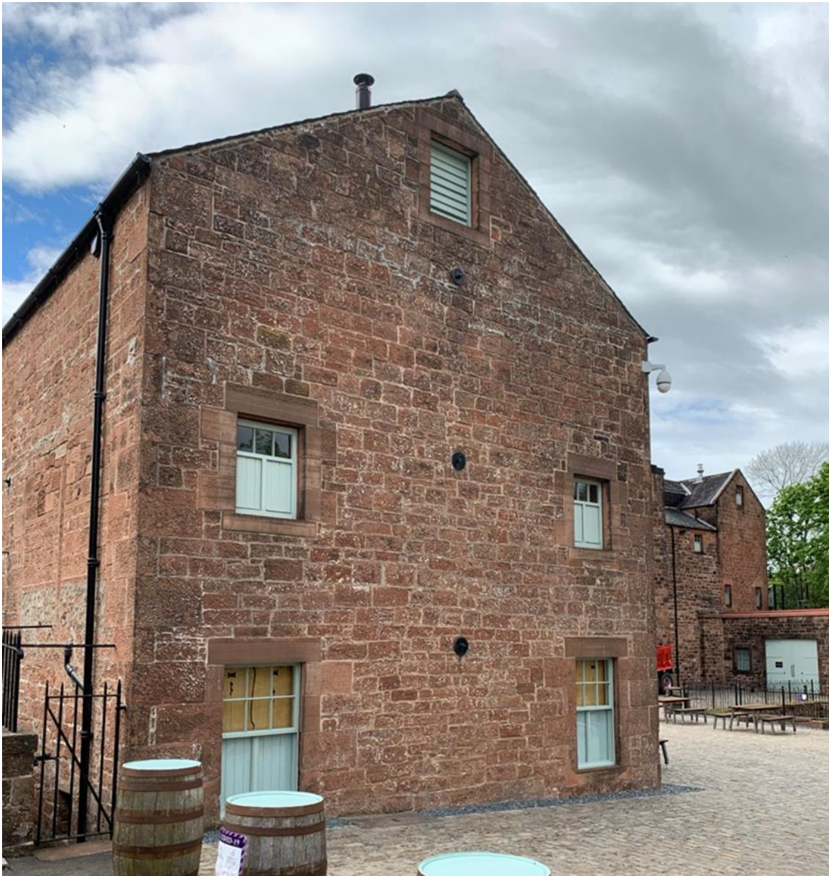
Figure 040.1. The SW gable of the Annan Distillery.
