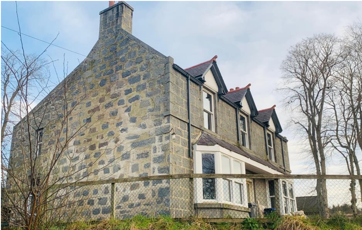
Figure 062.1. View of Miller's House from the southwest.
