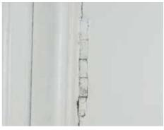
Fig. 9 Butt-hinge connection between the shutter and the shutter case.
