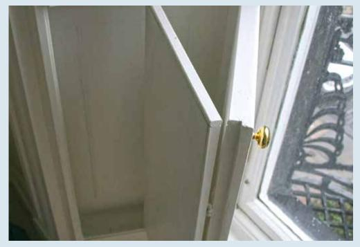
Fig. 5 Shutter divided horizontally into two separate hinged sections, designed to allow light into the room whilst maintaining a level of privacy.
