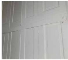
Fig. 7 Iron stay bar in position, spanning the width of the window opening.
