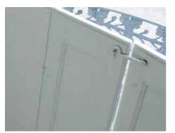
Fig. 8 Small latch used to hold shutters in the closed position at the stiles.
