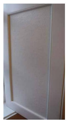
Fig. 12 Newly instated insulated timber shutters.
