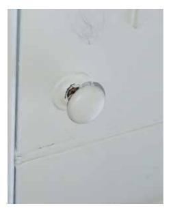
Fig. 10 Painted timber shutter knob fitted to shutter's outer leaf.
