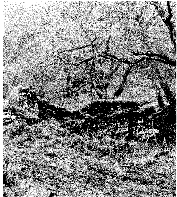
Figure 19. Bracken infested structure in the Western Southern Uplands ESA
