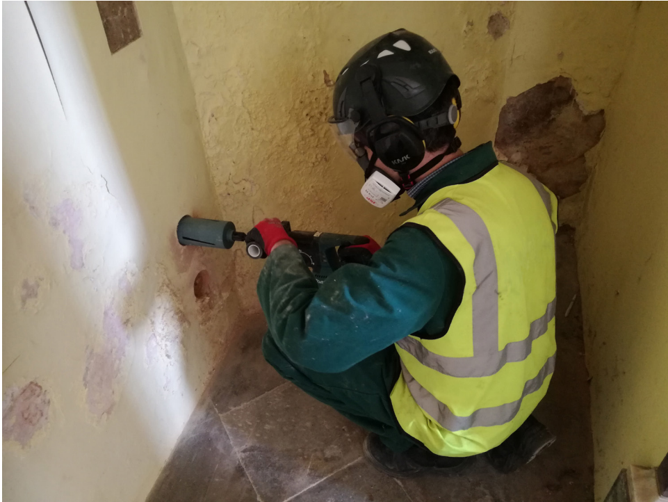
Figure 18 - Drill core being extracted from a rendered masonry wall.
