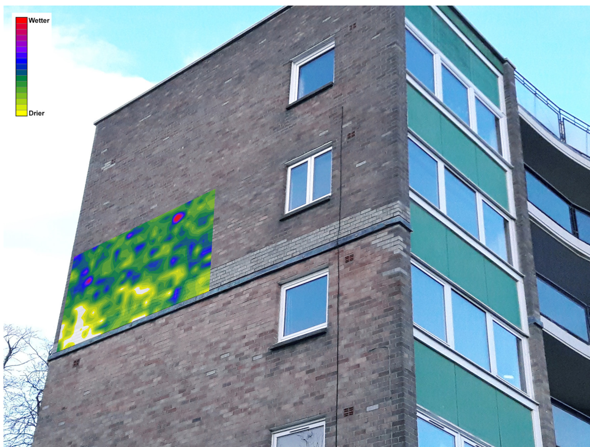
Figure 15 - Visual representation of moisture can be overlaid onto images, so that their context can be better understood.
