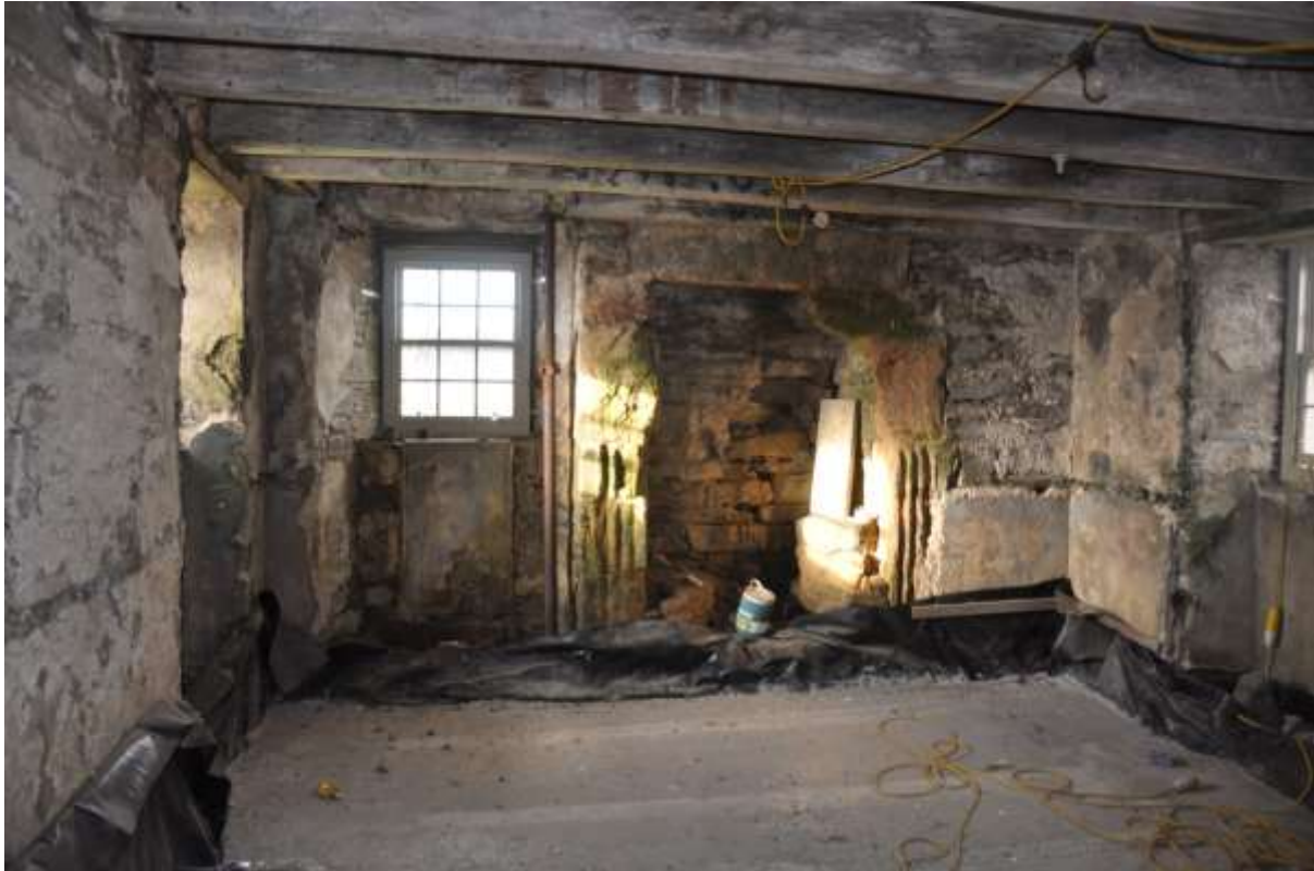
Figure 9: Remains of fireplace in the west wall on the ground floor
