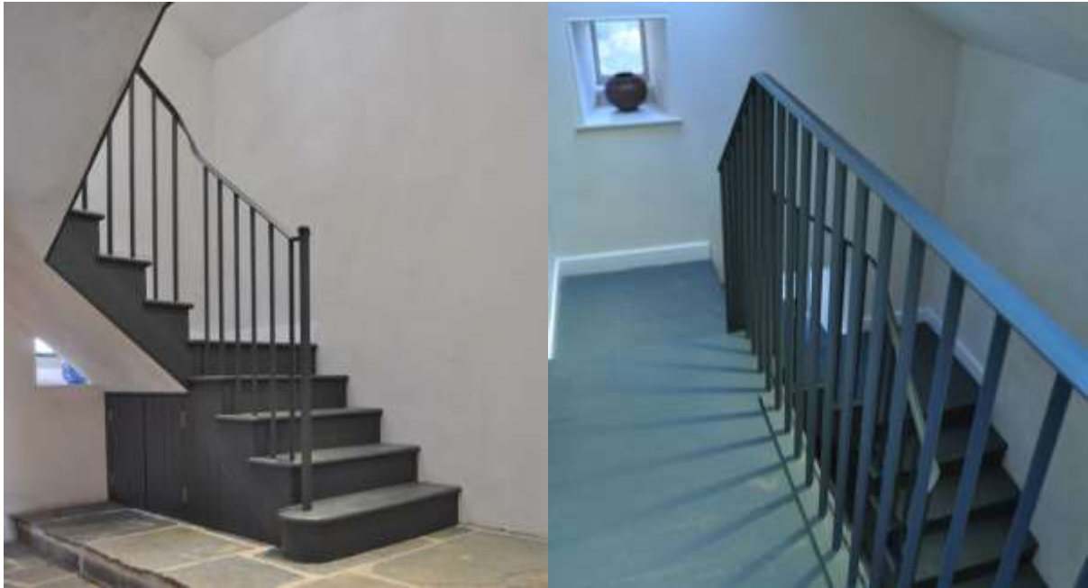
Figure 22: Newly designed timber and steel staircase in entrance wing
