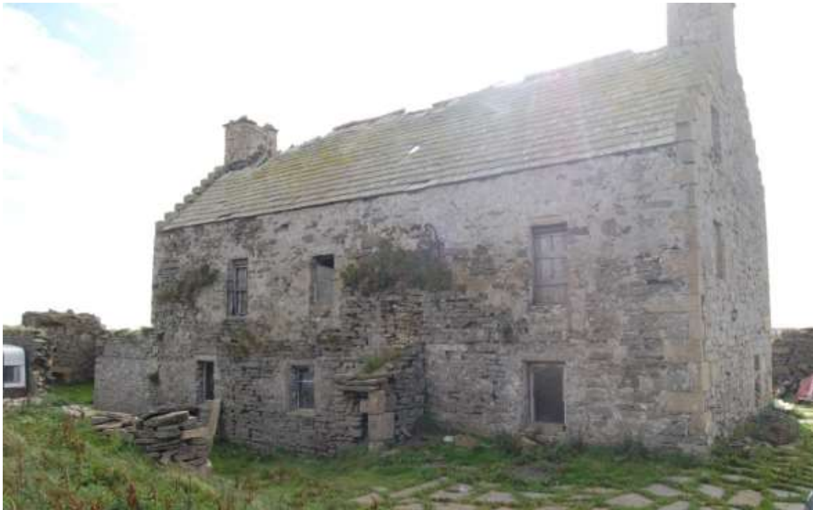
Figure 5: Extensive evidence of lime harl on north elevation
