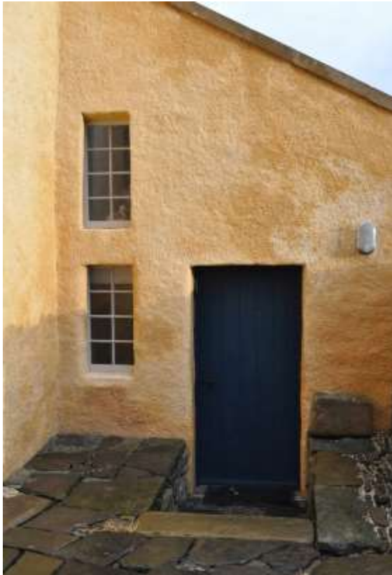
Figure 32: New timber tongue and groove external door
