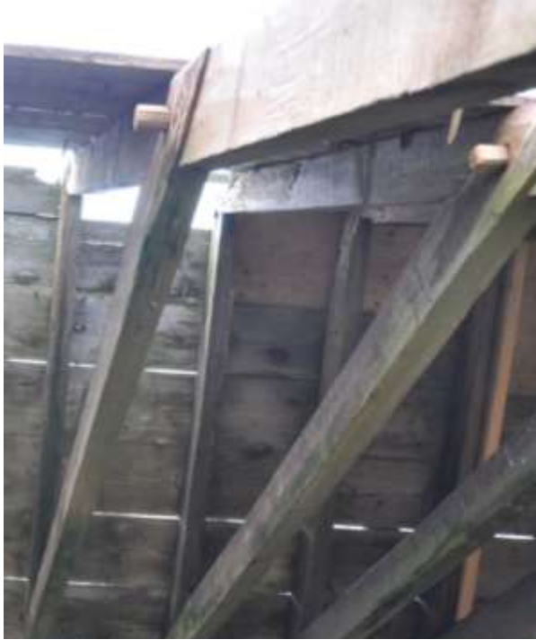
Figure 26: Repaired timber rafters, with splicing on the furthest right rafter
