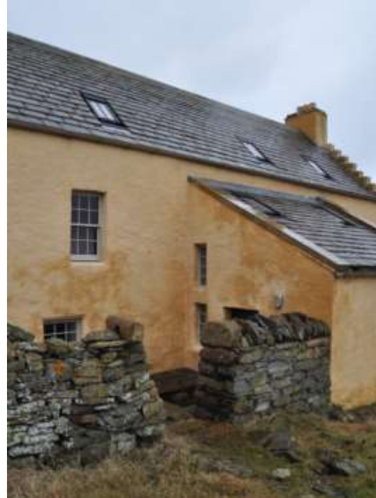
Figure 27: Repaired timber roof with original and reclaimed slates
