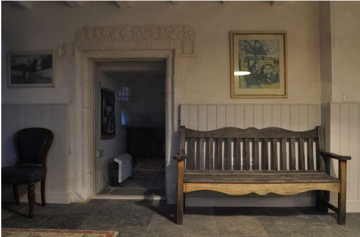
Figure 38: Caithness flagstones laid tightly together on the ground floor
