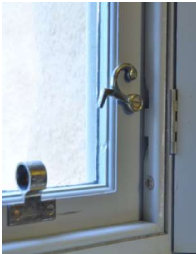
Figure 31: New sash dogs on small sash and case windows
