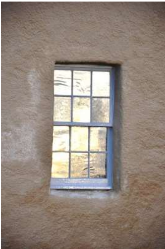
Figure 30: New single glazed sash and case windows with cylinder glass
