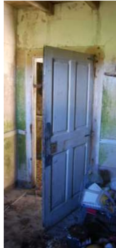
Figure 40: Original door still hanging in the central room
