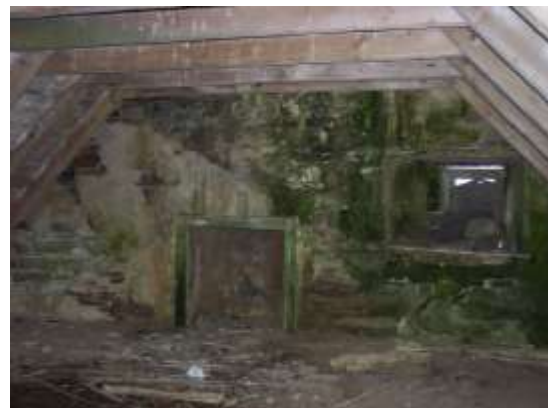
Figure 20: Existing attic condition
