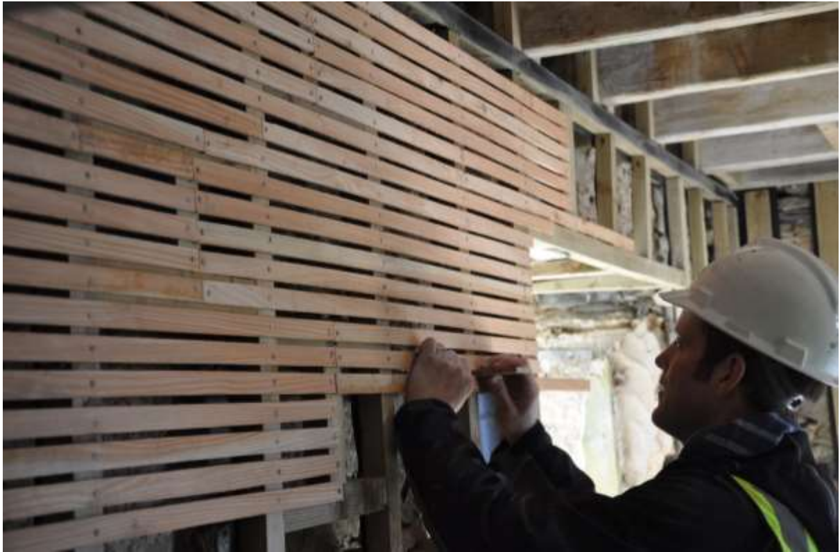
Figure 34: New sawn timber laths being fitted to timber framing
