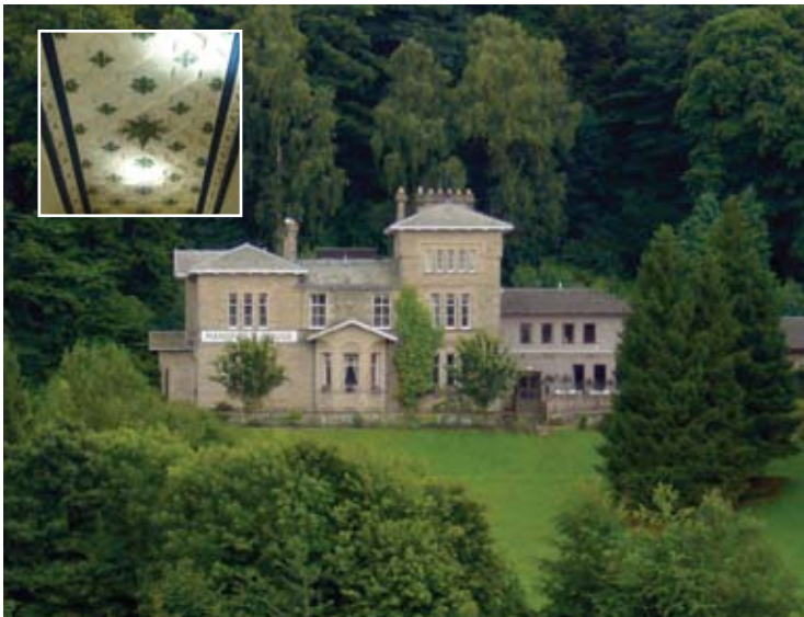
Mansfield House Hotel (inset) ceiling detail in Mansfield House Hotel
