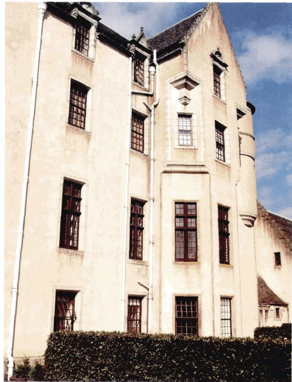
Illustration 37. Detail of part of the west elevation of Keith Hall showing granite lintols, crow's step gable end and new rainwater discharge systems
