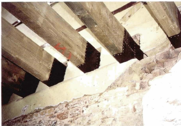
Illustration 33 Use of DPM wrappings to protect beam ends.
