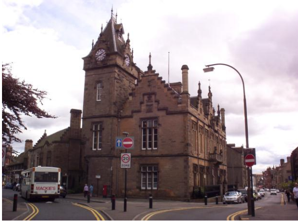
Fig 45. Alloa County Buildings, Brown and Wardrop, 1863, (category B).
