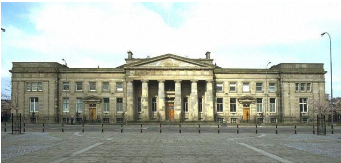
Fig 23. Glasgow High Court, William Stark, 1807–14, (category A). © Architecture on Disc. Licensor www.scran.ac.uk
