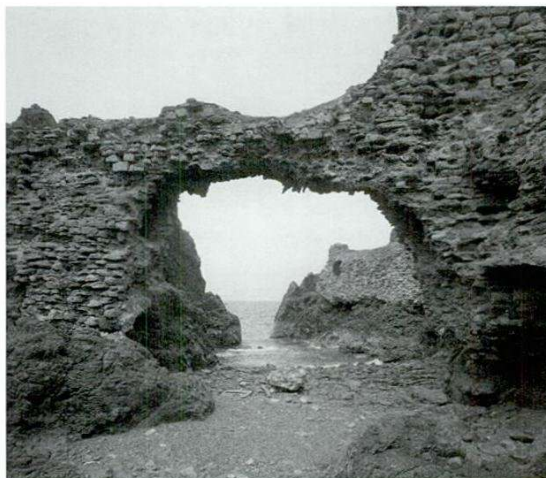
Figure 13.3 View of the covered passage leading from Dunbar Castle to the blockhouse.
