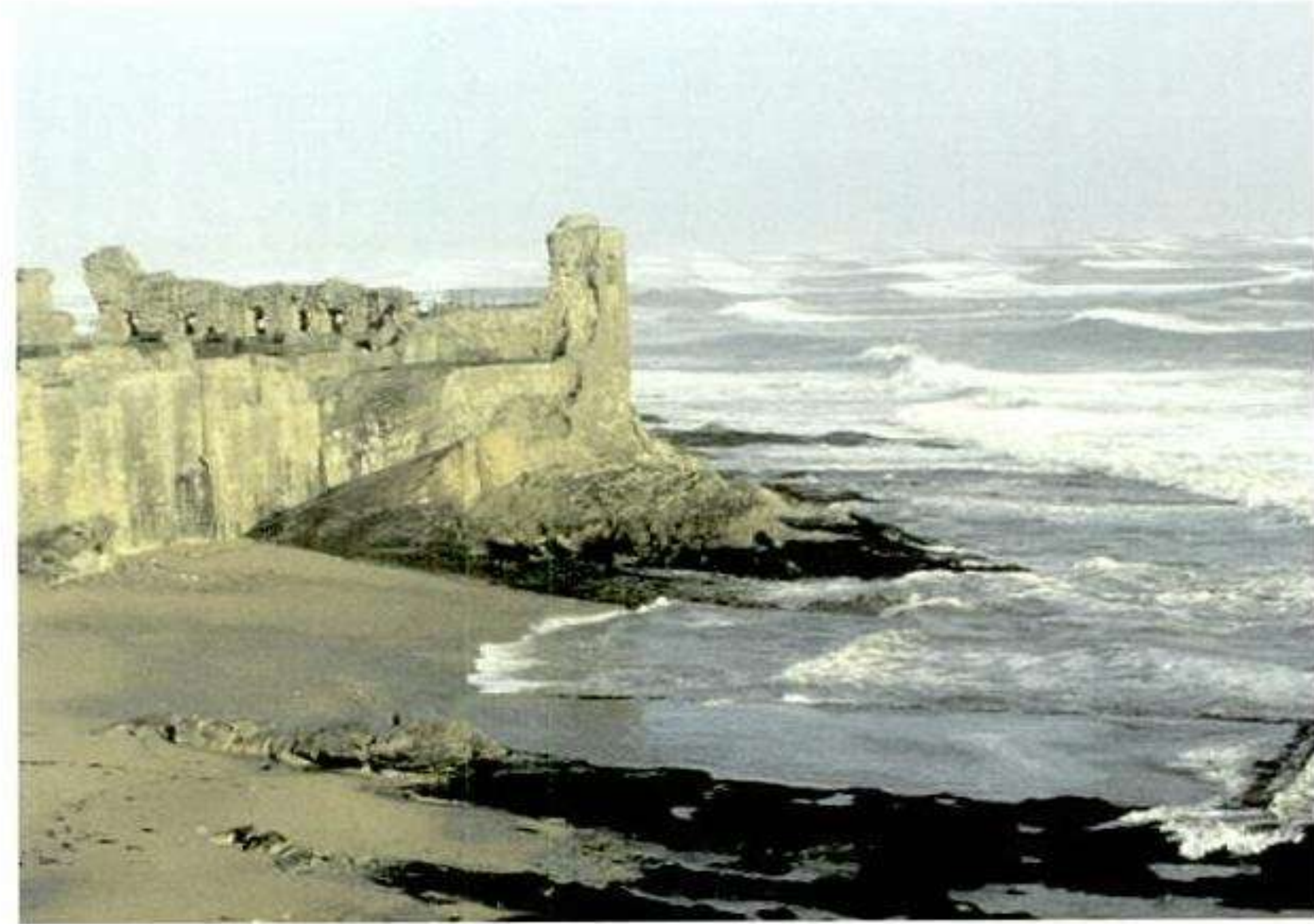
Figure 1.2. St Andrews Castle, Fife, with the strengthened sea cliff visible below the castle.
