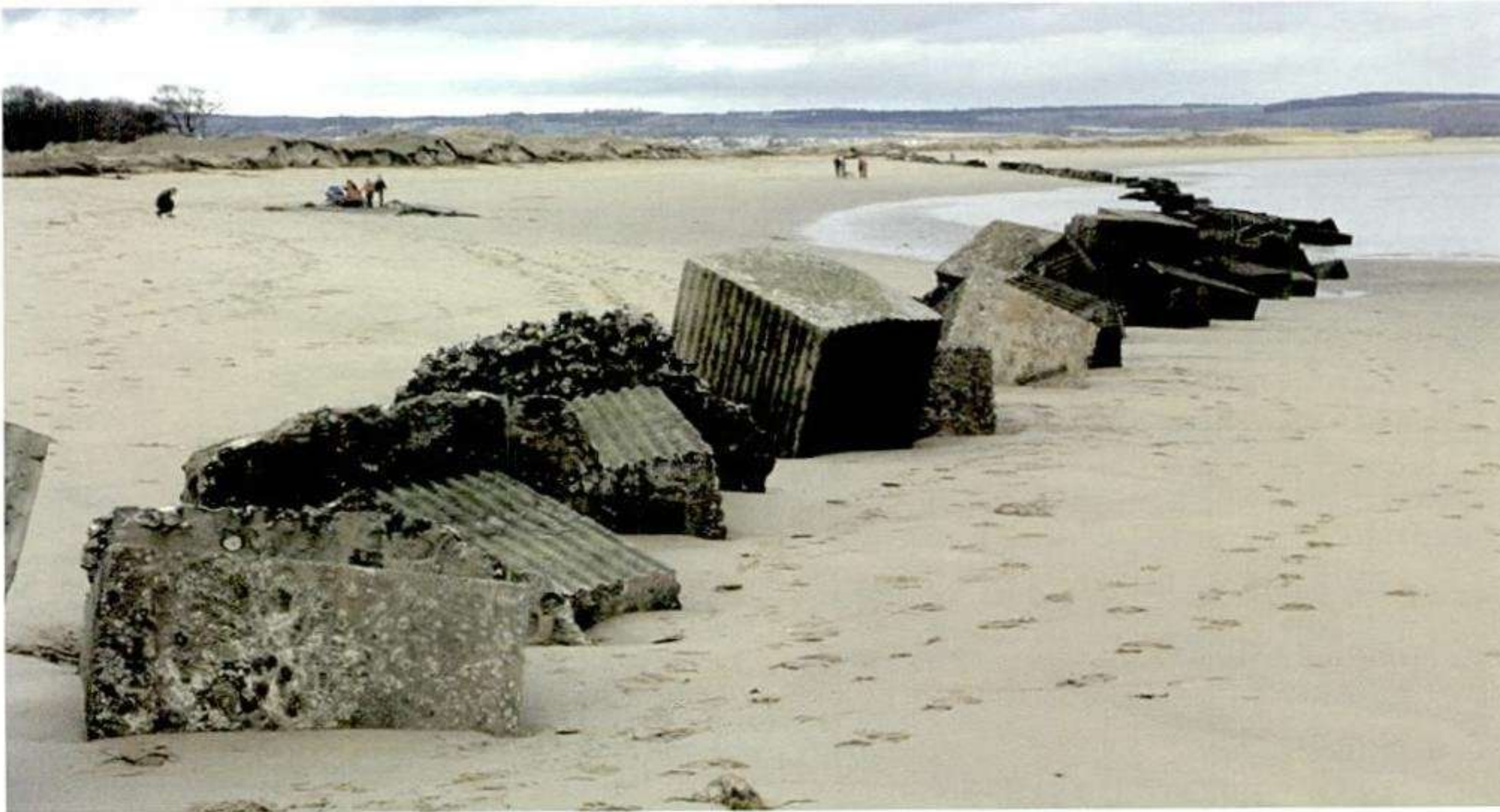
Figure 12.5. Collapsed tank traps at Tentsmuir, originally built on dry land.
