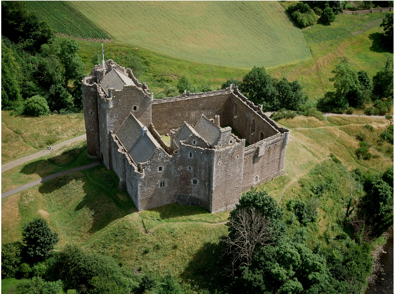
Figure 1: Aerial view of Doune Castle. © Crown Copyright HES.
