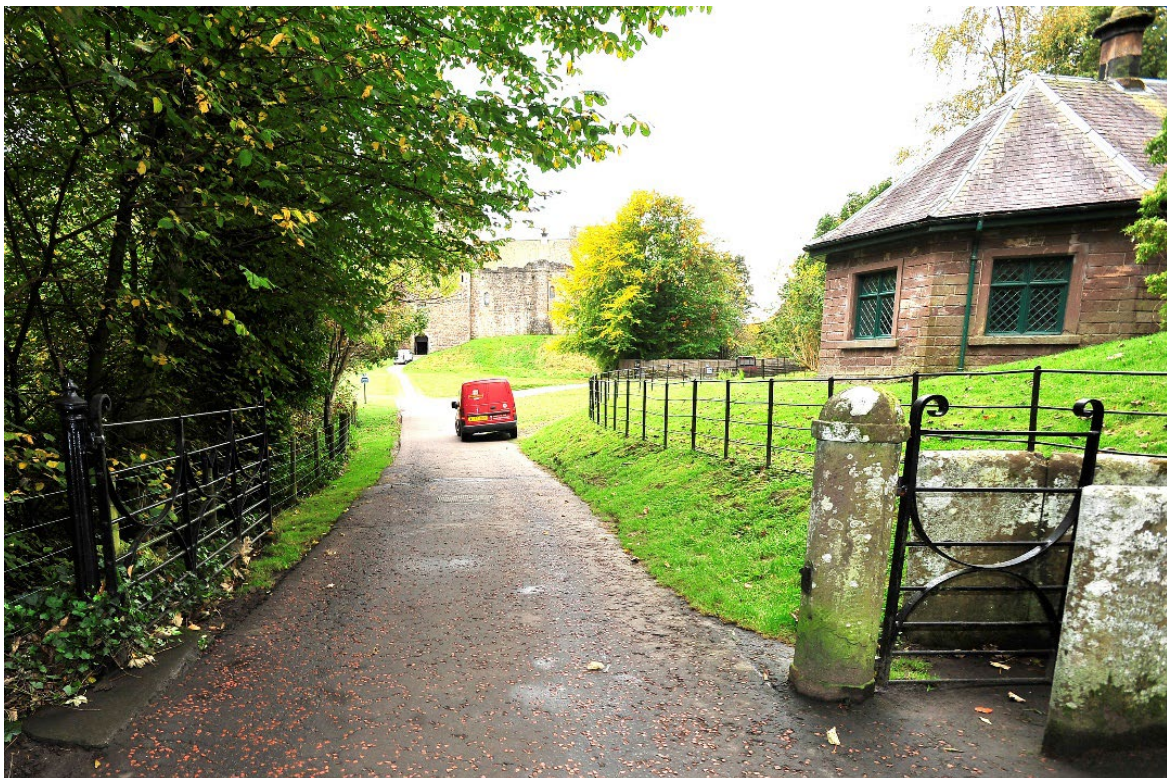
Figure 17: View of approach to Doune Castle including example of high-quality 'kissing gate', with cottage behind. © Crown Copyright HES.
