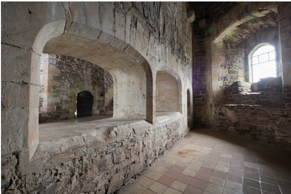
Figure 5: View through the servery into the kitchen. © Historic Environment Scotland.
