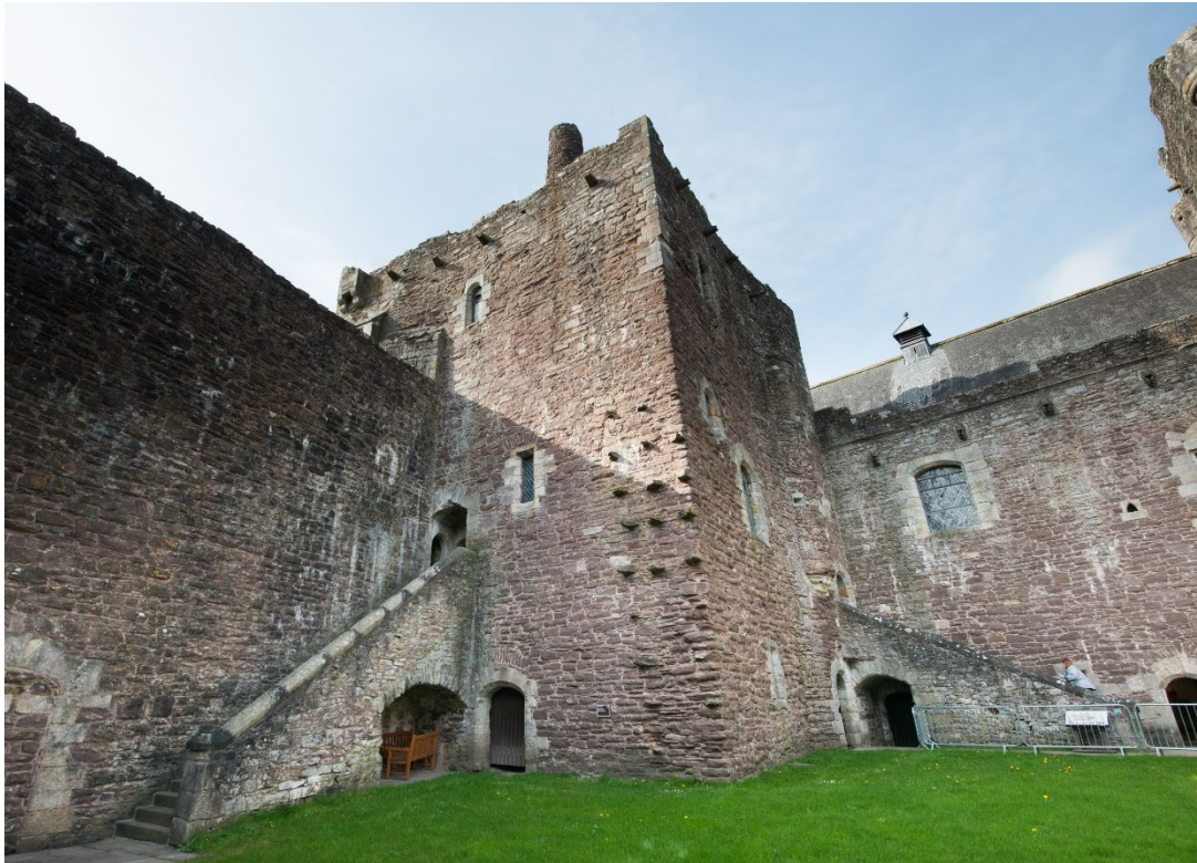
Figure 4: Kitchen tower with 'tusking' visible in centre of image as a series of projecting stones. © Historic Environment Scotland.
