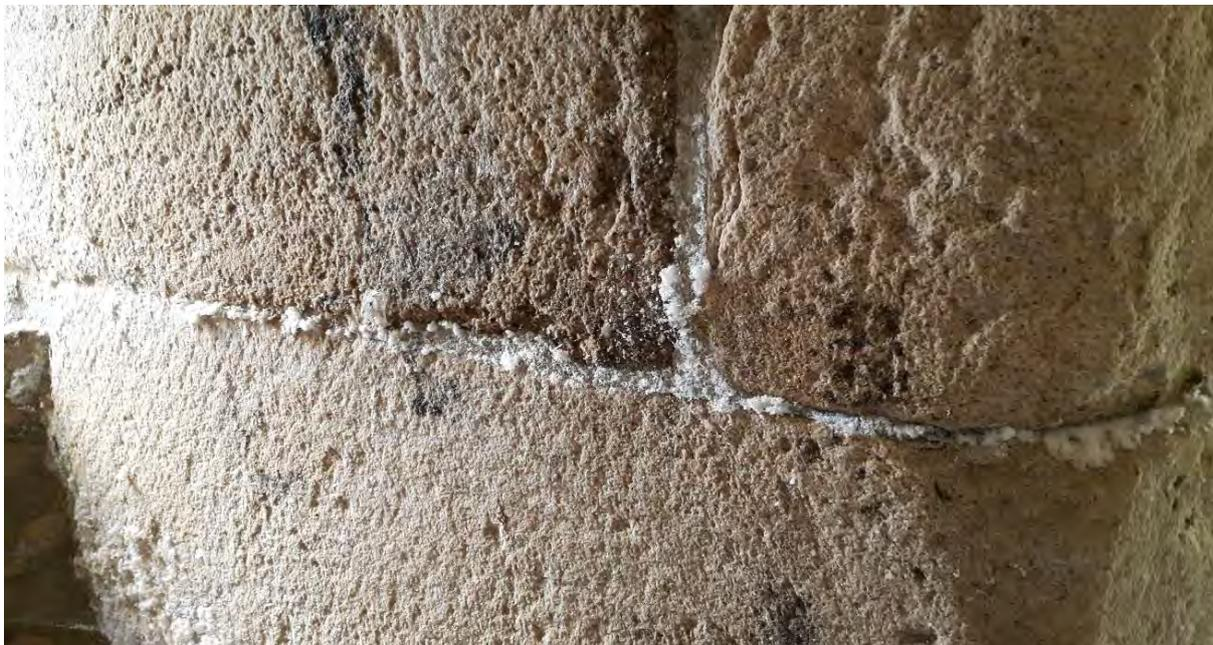
Figure 3: Sacrificial protection in practice - precipitation of soluble salts in mortar joints at Aydon Castle, Northumberland (18<sup>th</sup> century agricultural buildings).
