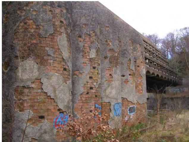
Delaminating/missing render from brick silo shaped chapels
