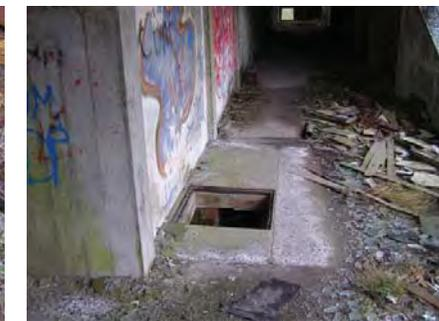
**Plates T4:** Blocked entrances to a basement and an open access into an under-floor or basement area. These areas would need to be investigated and would probably, at least initially, be classified as confined spaces.
