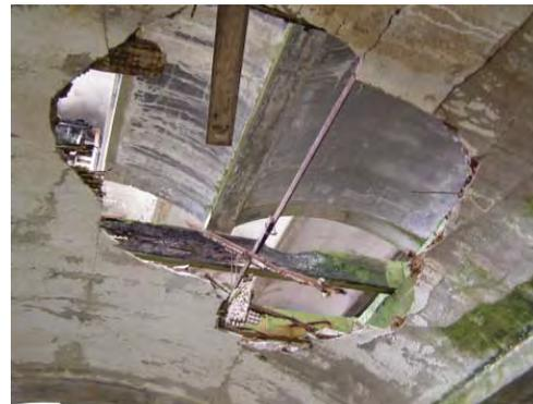
Damaged plastered vault
