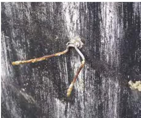
Corroding cast in metal wall ties
