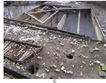
**Plates T2:** Unsafe, rotten and partially collapsed roofs.
