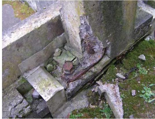
Corroded bolt fixings at base of concrete posts
