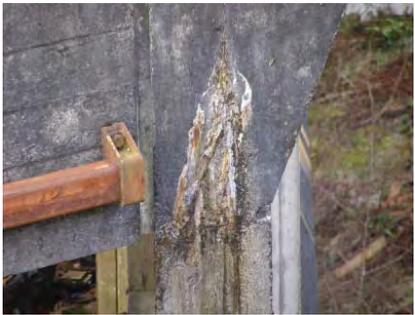
Exposed corroded reinforcement
