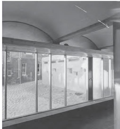
View of vaulted ceilings, formed with metal hy-rib section, and showing also the timber cradle screen header
