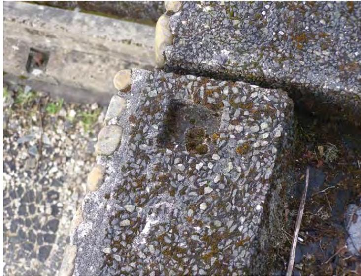
Displacement of corner handrail post
