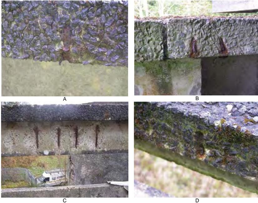
**Plates T14:** Exposed reinforcement and surface spalling associated with corroded reinforcement on the hidden and less obvious surfaces of the pre-cast panels.
