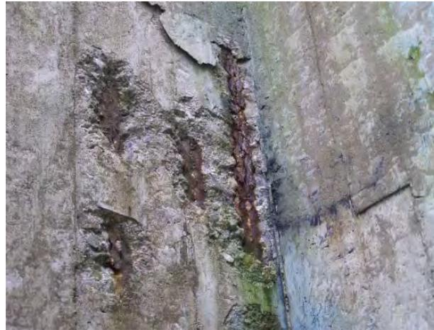
Exposed corroded reinforcement
