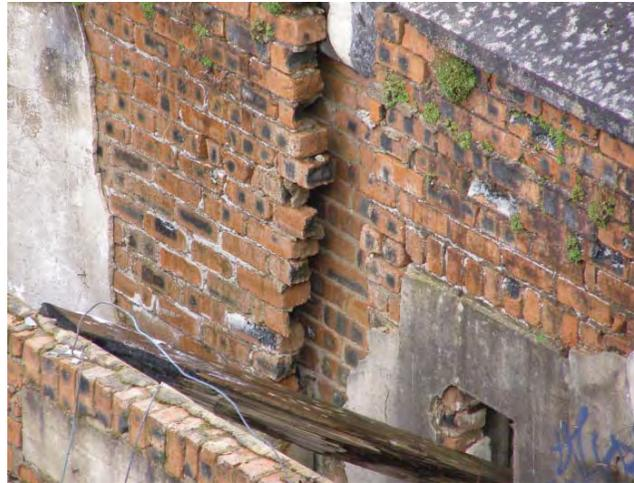
Corrosion of wall ties
