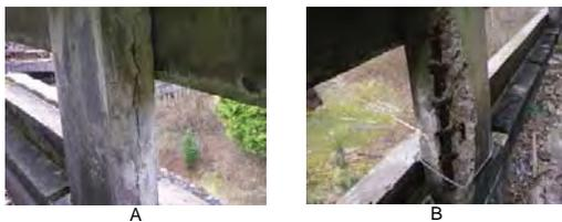
**Plates T11:** Typical cracking and spalling to a stub columns.
