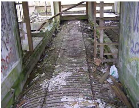
Floor missing vault viewed from above showing metal Hi-Rib lath support structure
