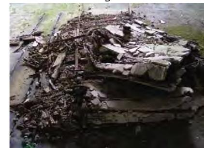
**Plates T3:** Collapsed roofing materials, debris and unprotected edges.
