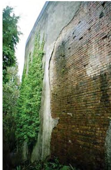
Delaminating/missing render leading to saturated brickwork
