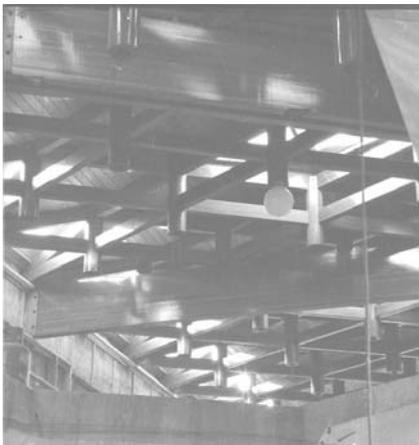
Timber lattice beam roof structure of teaching block
