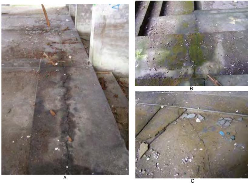
**Plates T10:** Cracking through the suspended floor to the main building, possibly reflecting hidden structural details and / or relative movement/s of the structure.
