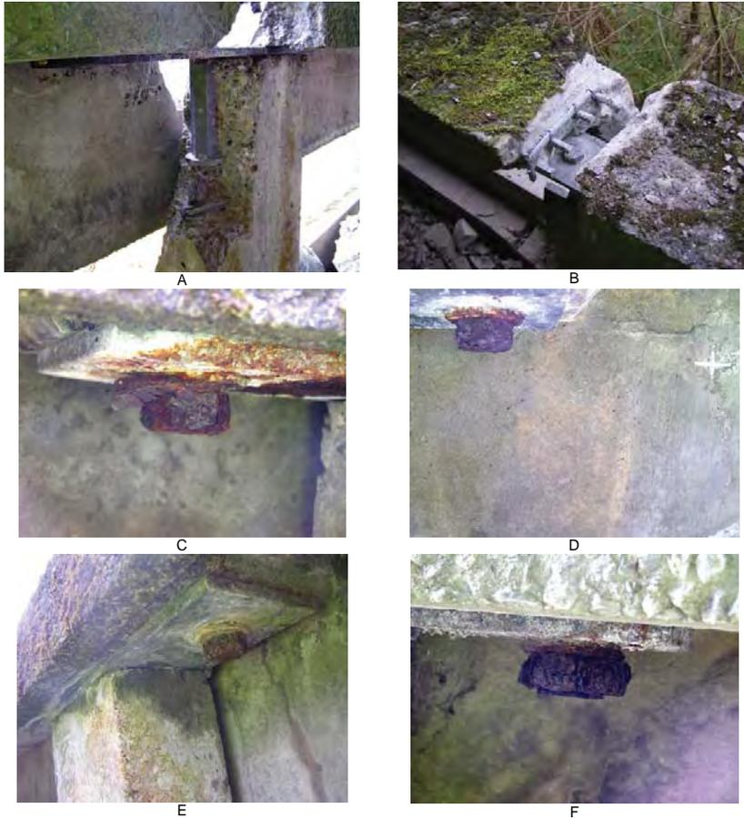
**Plates T18:** The stub columns and pre-cast handrail units had been cast with threaded steel sockets at fixing positions. Steel plates had been bolted onto the tops of the stub columns, with further bolts through the steel plates and up into the backs of the handrail units. The steel elements had been galvanised, but in some locations the galvanising had deteriorated and corrosion was apparent.
