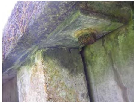
Corroded bolt fixing to underside of handrail panels
