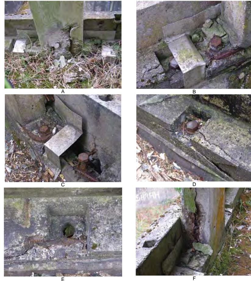
**Plates T17:** Deterioration and distress associated with the lower panel and stub column fixings.
