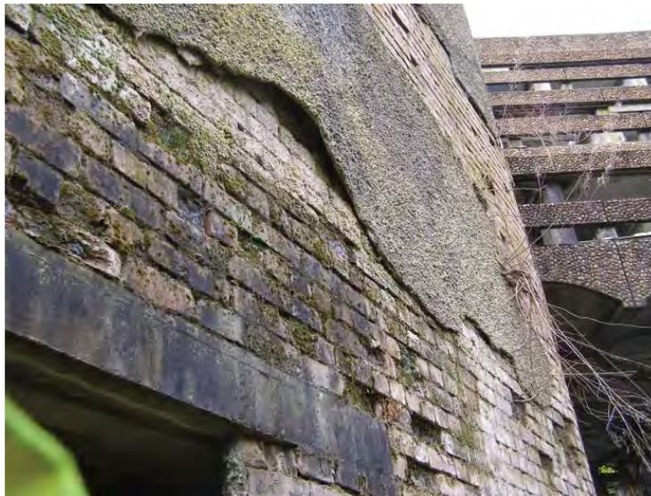
Lost and delaminating render with consequential brick damage
