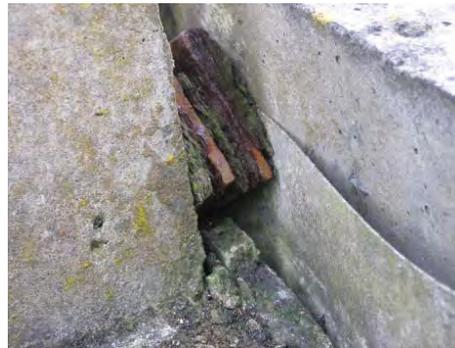
Corroded shims between handrail post and facade forcing panels out of alignment
