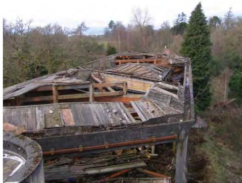
Damaged timber roof of teaching block all original copper roof covering missing
