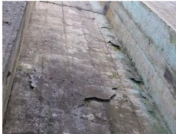
Delamination of concrete surface
