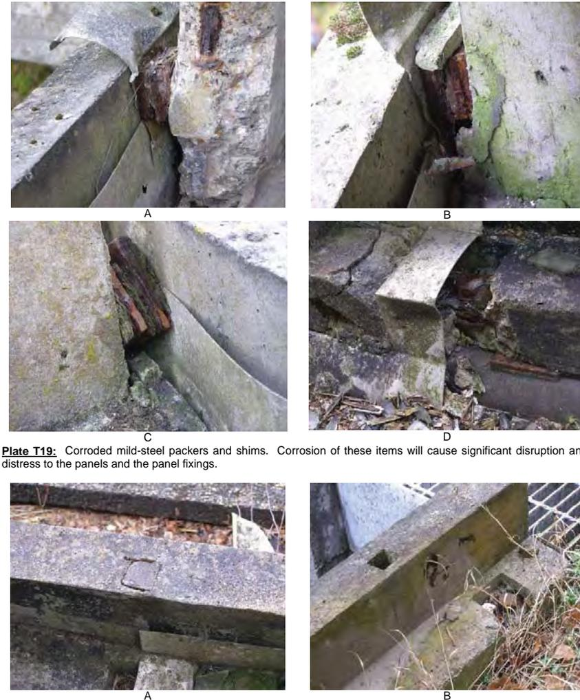
**Plate T19:** Corroded mild-steel packers and shims. Corrosion of these items will cause significant disruption and distress to the panels and the panel fixings.
