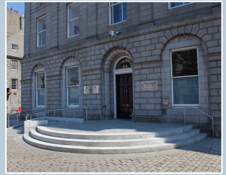
New steps and ramp at the Castle Street Annexe of the Sheriff Court in Aberdeen. High-quality contemporary design and materials provide improved access for all users of the building.
