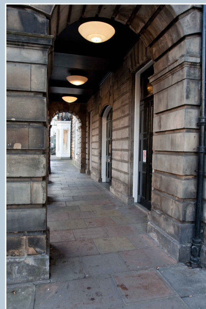
The Assembly Rooms, George Street, Edinburgh, where the pavement level has been raised at the main entrance to eliminate a threshold.
