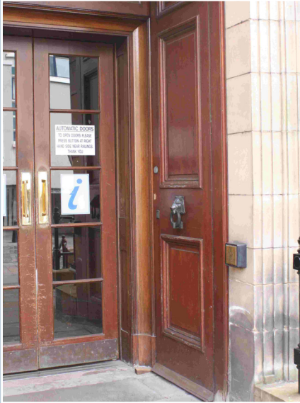
The door into Linlithgow's County Buildings opens automatically, and also has a manually operated push pad. © West Lothian Council.
