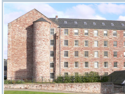
A new lift tower in complementary style was added to the East Mill at Stanley Mills, Perth and Kinross, as part of its conversion to residential accommodation.
