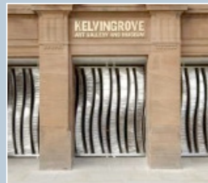
New wide openings were created at the rear of Kelvingrove Art Gallery in Glasgow to provide level access to the building.
