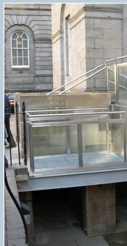
This platform lift provides alternative access from the pavement to the side entrance of General Register House in Edinburgh.
