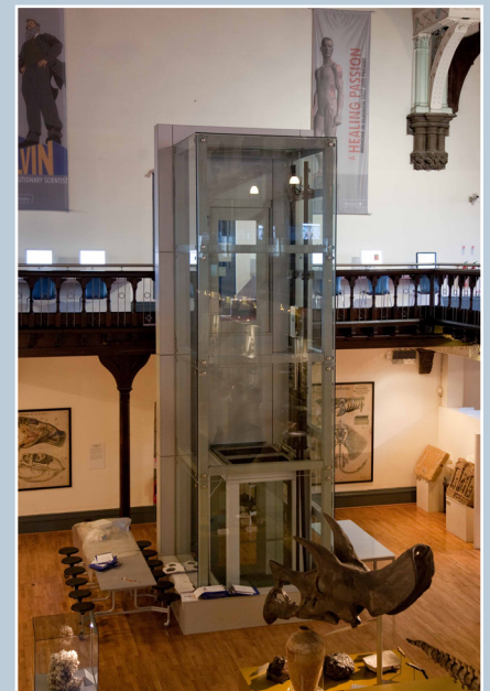
The Hunterian Museum, Glasgow University, completed circa 1870 to designs by Sir George Gilbert Scott. A contemporary glazed lift has been inserted to enable access to the upper gallery of the main exhibition space.
