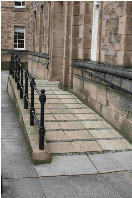
Linlithgow County Buildings, West Lothian. Attention is drawn to this ramp by the use of a variety of textures, carefully designed to complement the character of the building. © West Lothian Council.
