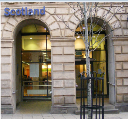
Kirkcaldy, Fife. Ramped and stepped access was achieved in this busy pedestrian street by removing the original door and a window to create an internal lobby. Equality of access was achieved and the principal feature of the building's ground floor, the arcade of round-headed arches, was maintained.
