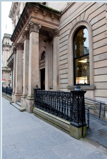
Buchanan Street, Glasgow, where a ramp constructed in a discreet location over the basement area enables easy access for all to this shop.
