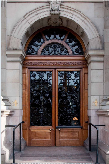
An accessible entrance to the City Chambers, Glasgow, part of a well-considered access arrangement that takes in both physical and management aspects of approaches, entrances, and moving around the building. The pavement has been adjusted to lessen the gradient of the ramp. Different colours are used to demarcate the ramp, and the texture creates a non-slip surface. Railings are provided for support. The doors operate from a large push control, and there is a speakerphone for assistance if necessary. Signage indicates the accessible entrance and continues throughout the interior of the building. An access guide is available online, or at the building, for blind or visually impaired visitors. Loan wheelchairs are also available.
