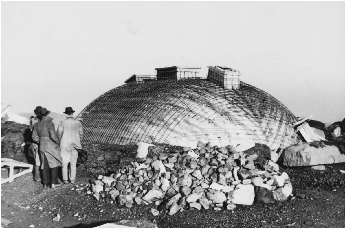
Figure 12: Concrete dome under construction © Crown Copyright: HES
