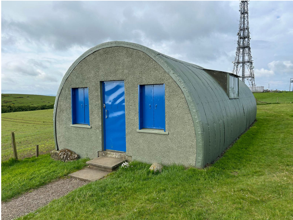
Figure 10: Nissen Hut, now used as a visitor centre. © Historic Environment Scotland
