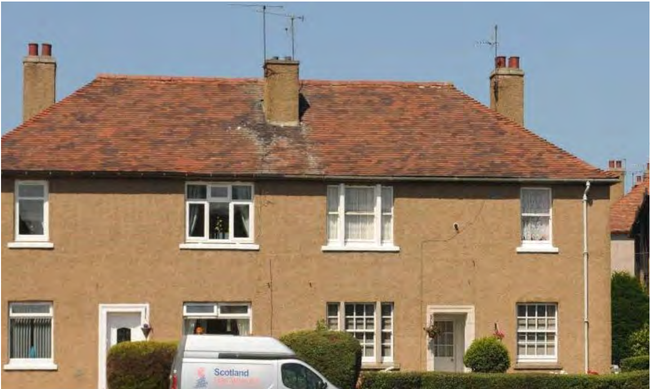
Figure 9 - A 'four in a block' type house designed for social housing in Scotland in the inter war period.
