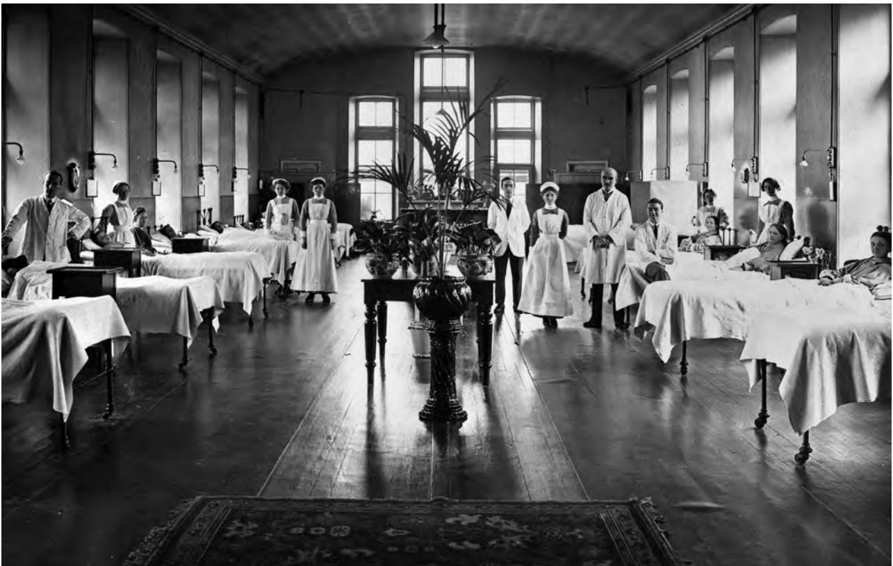
Figure 1 - Ward 15 in the Royal Infirmary of Edinburgh in 1917. Note the high ceilings and windows on both sides for cross ventilation. © Survey of Private Collection. Dr G L Malcolm-Smith album. Courtesy of HES.
