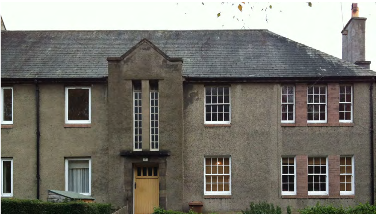
Figure 8 - Social Housing units in Edinburgh designed by the City Architect Ebenezer MacRae in 1936; a traditional style with modern elements.
