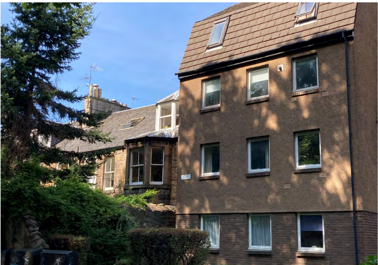
Figure 7 - Modern type housing from the 1980s seen next to a 19th century colony flat in Stockbridge, Edinburgh. Note the low ceiling height and relatively smaller windows in the newer building.
