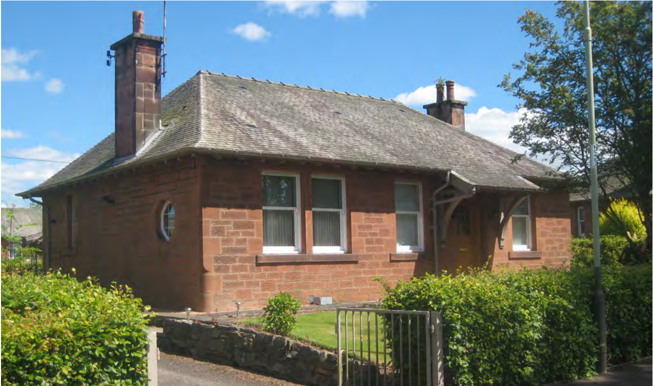
Figure 10 - One of the cottages built by Alexander Bell on the edge of Perth. Image © The Gannochy Trust
