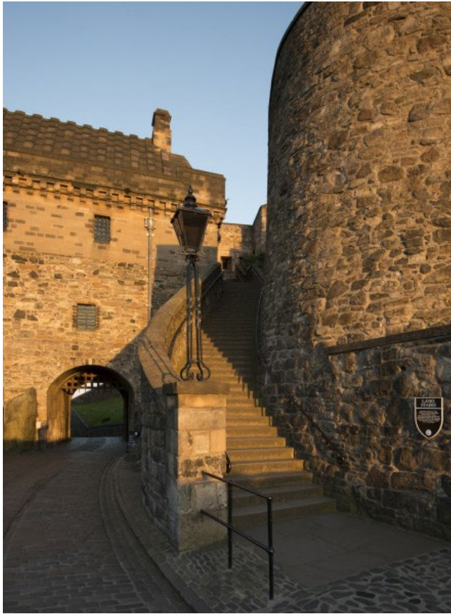
Lang Stairs, Portcullis Gate and Argyle Tower, looking south-east
