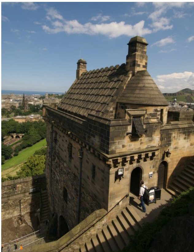
Lang Stairs, Portcullis Gate and Argyle Tower, looking north-east
