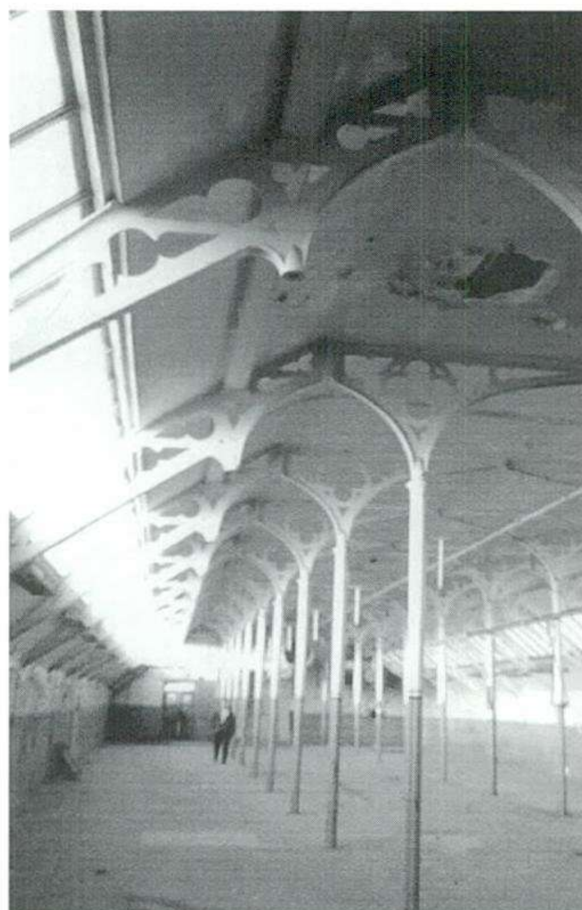
Figure 1: Cast-iron gothic roof trusses in South Mills, Dundee. Circa 1855
