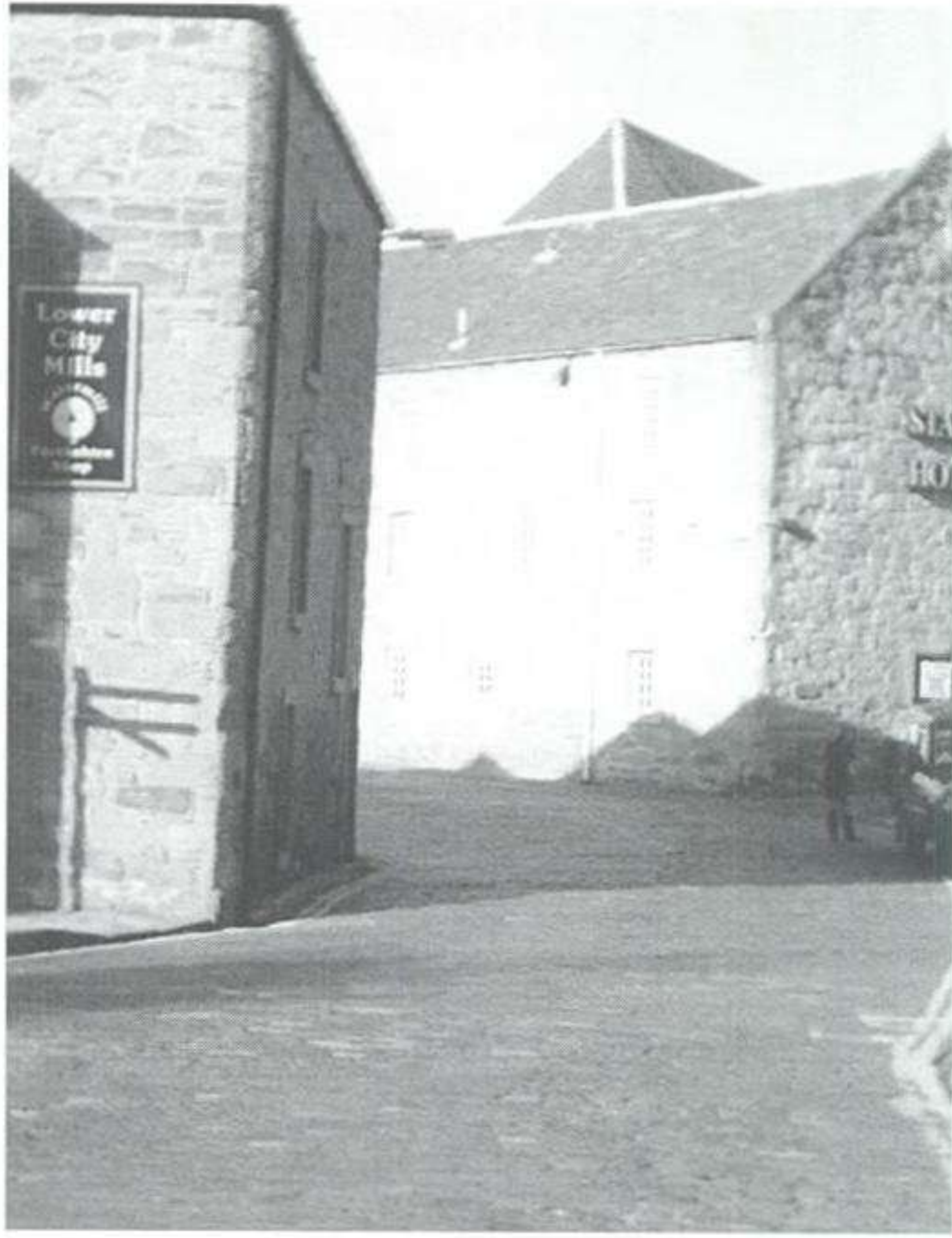
Figure 8: The City Mills, Perth. A wonderful combination of slate, sandstone and granite setts
