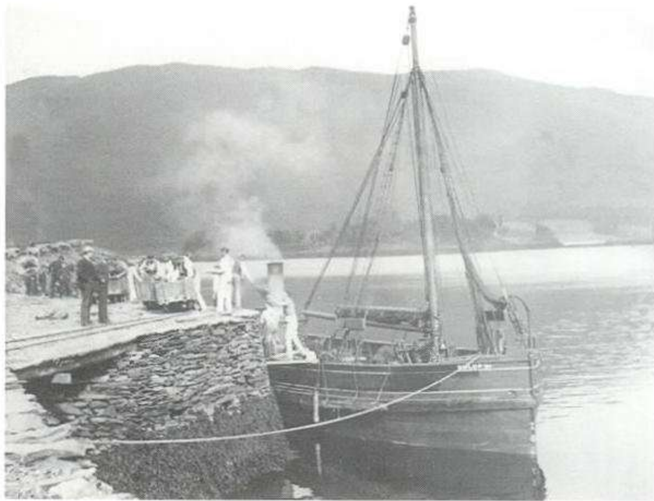
Loading slates on to a small steamship at Ballachulish in around 1900. The railway wagons came direct from the quarry, via an inclined plane, to the quay. Note the dressing tables in the left background
