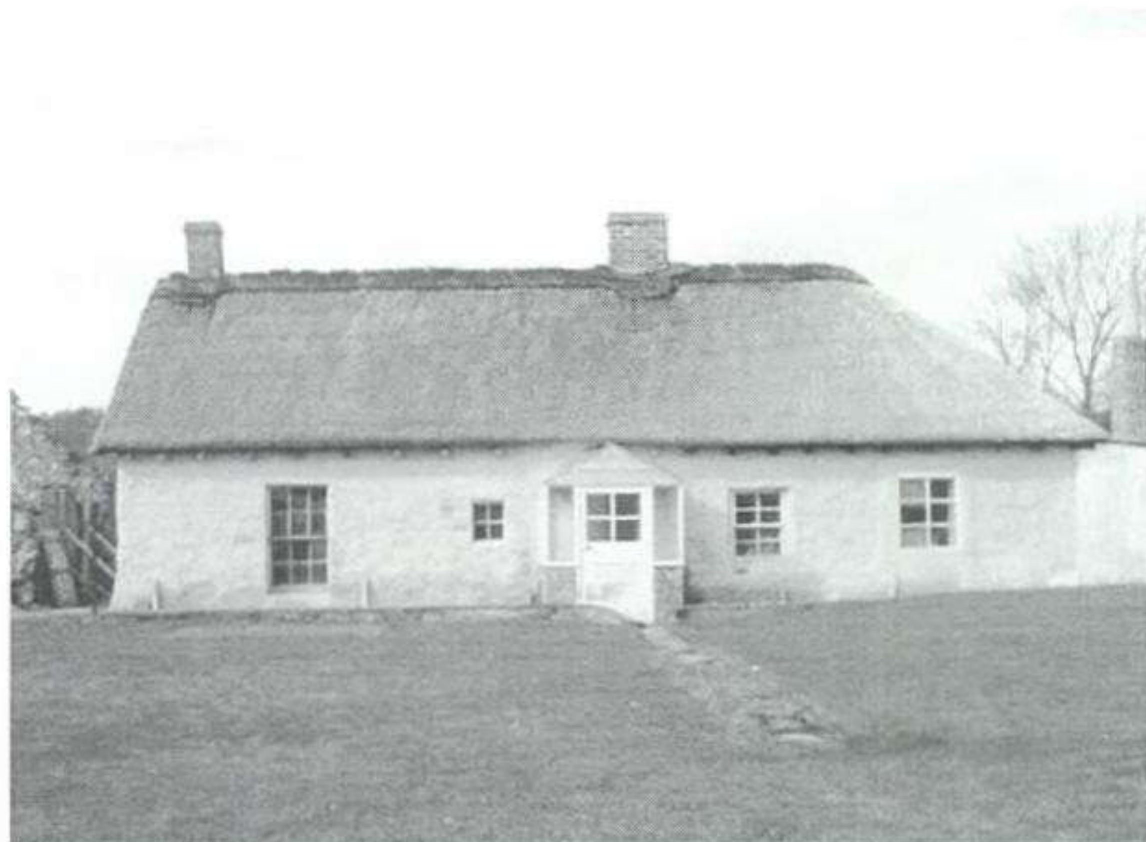
Figure 2: The Old Schoolhouse, Cottown, Carse of Gowrie, newly restored clay wall and reed thatch
