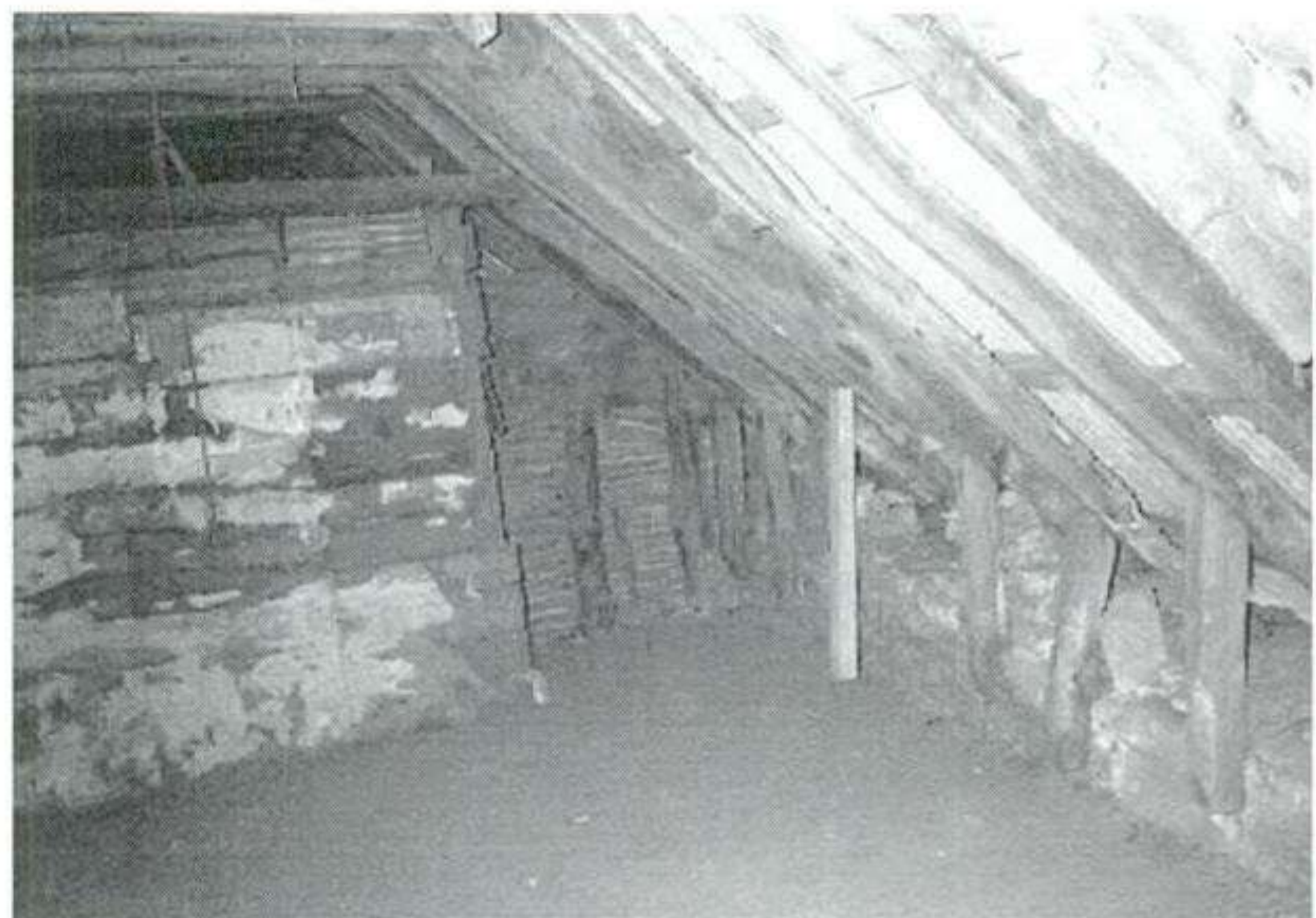
Figure 5: Ashlar post roof at High Street, Brechin
