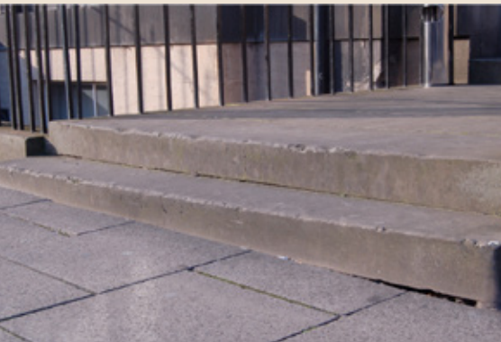
Fig. 1 Simple block step and platt, constructed from large slabs of stone.
