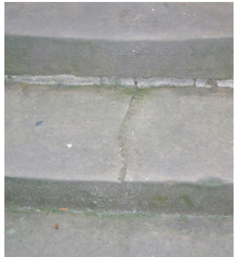
Fig. 5 Evidence of past settlement can be historical and need not be a cause for concern.
