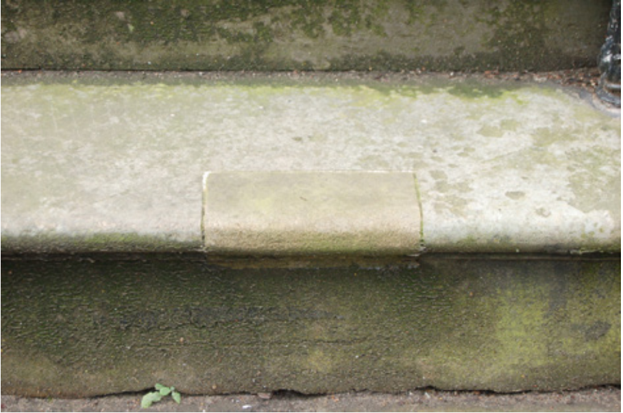
Fig. 9 Stone for indent repairs should be carefully matched to the original.
