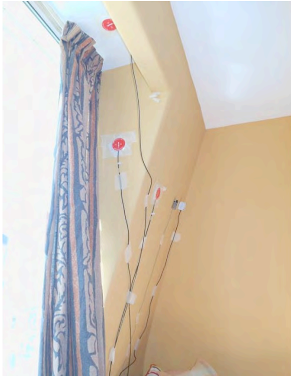
Fig. 23 Heat-flow mats in position on the coomb and dormer
