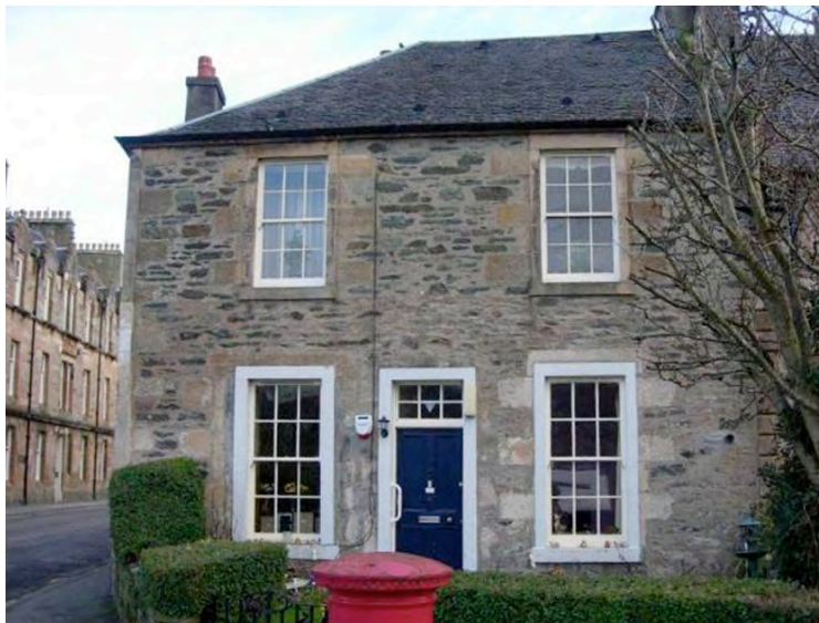
Fig. 27 External view of the door at Colbeck Place
