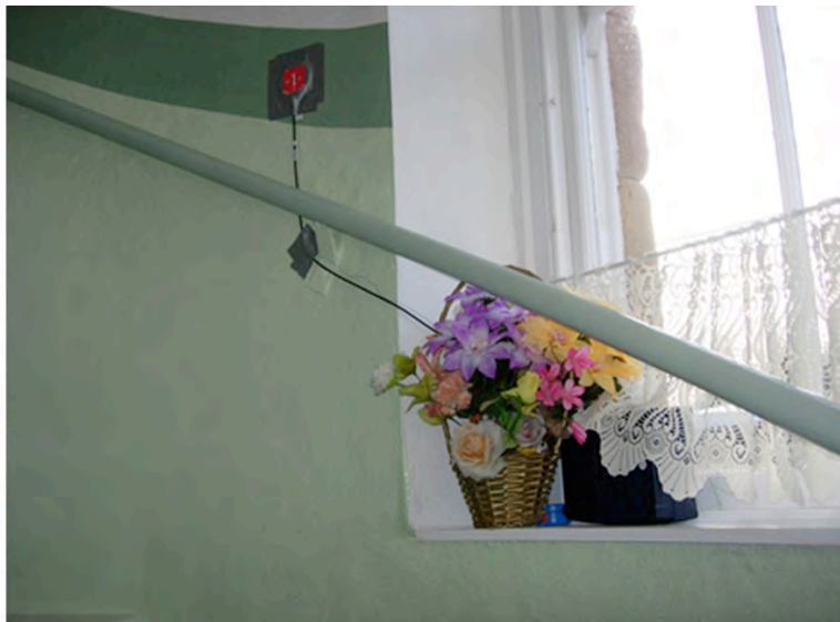
Fig. 26 Heat-flow mat placement in the stairwell post-intervention
