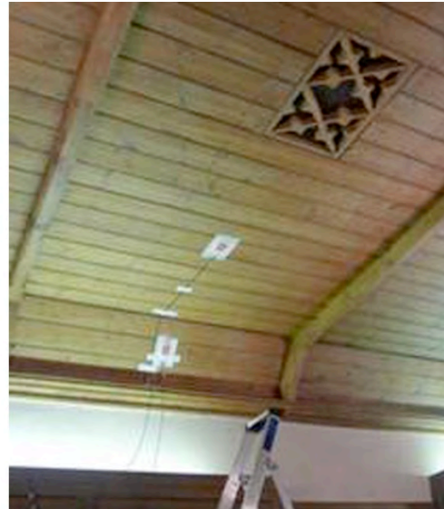
Fig. 34 Heat-flow mats on the ceiling and coomb
