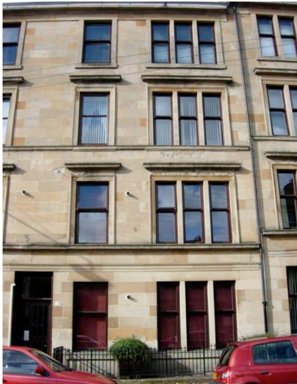
Fig. 31 External view of the property at Whitevale Street, Glasgow
