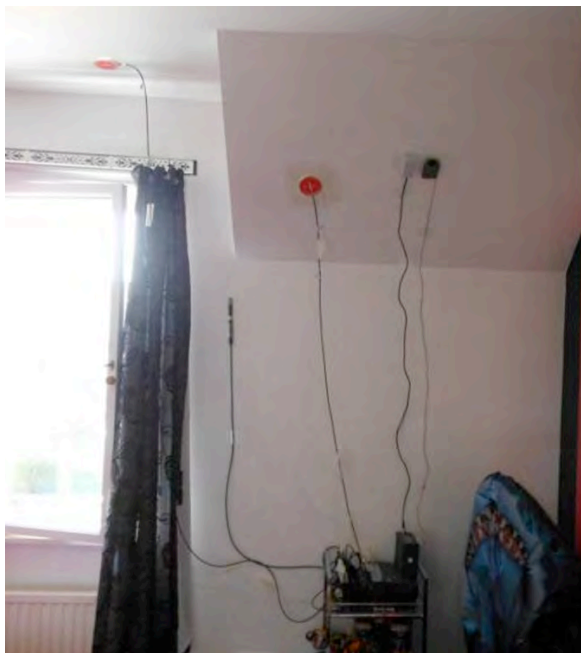
Fig. 21 Heat-flow mats on the coomb and ceiling
