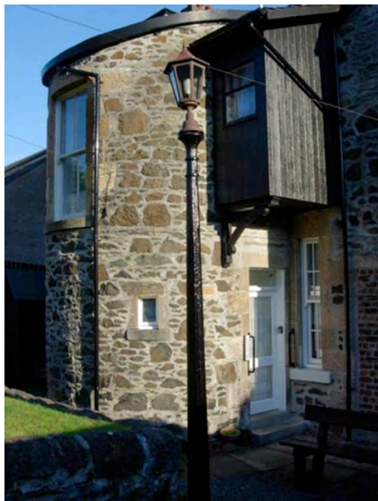
Fig. 25 Exterior view of common staircase
