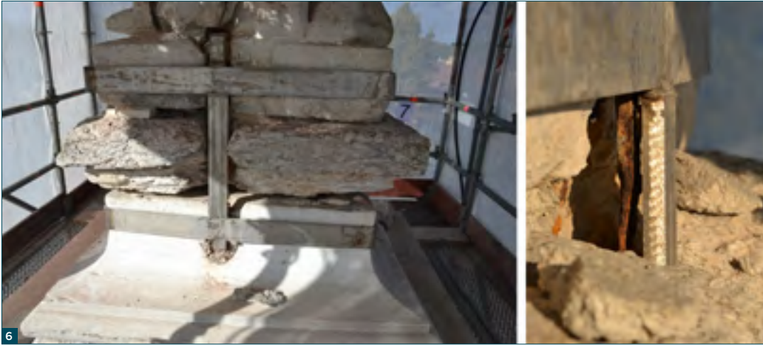
Figure 6: Podium of the statue. The external metal support ring in stainless steel has been welded to the damaged parts, accelerating oxidation.
