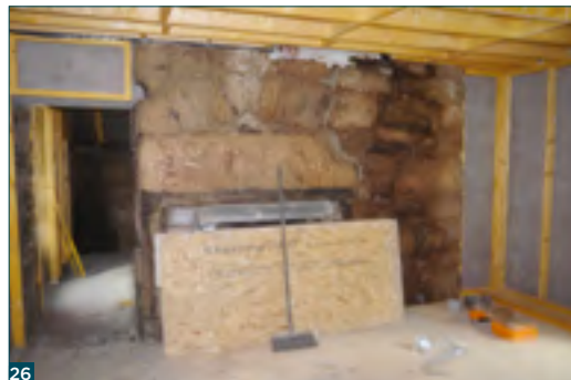
Figure 26: Wall linings stop short of the fireplace to display the graffiti.
