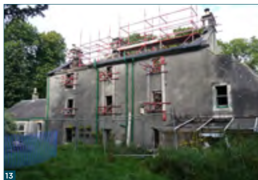
Figure 12: Temporary works in progress.
