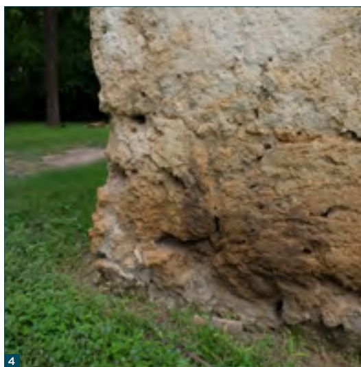
Figure 4: North-west corner of the church of Concepción.
