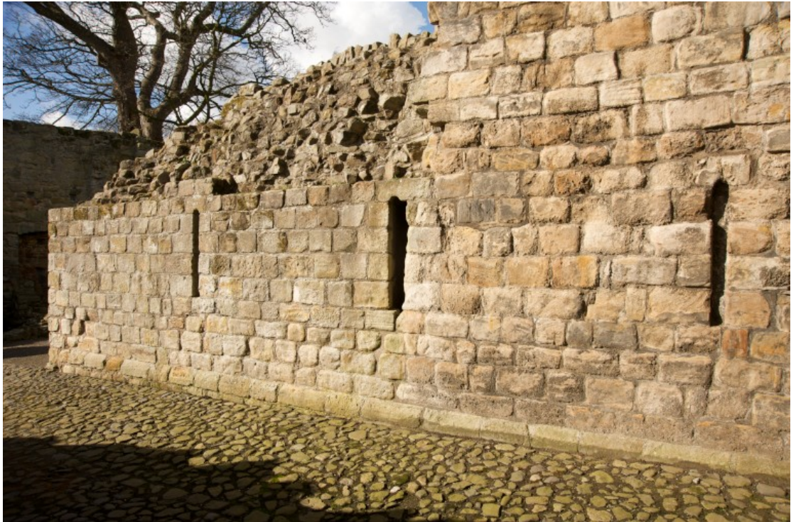
Base of the old tower, South elevation
