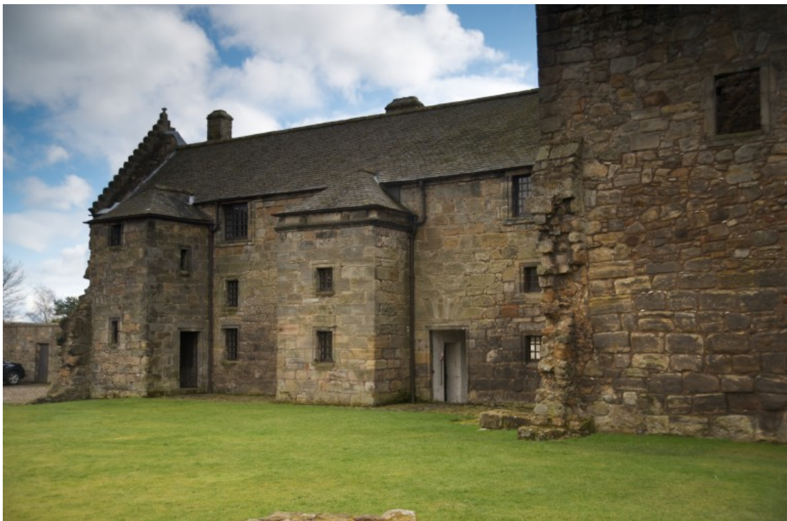
East range, North elevation
