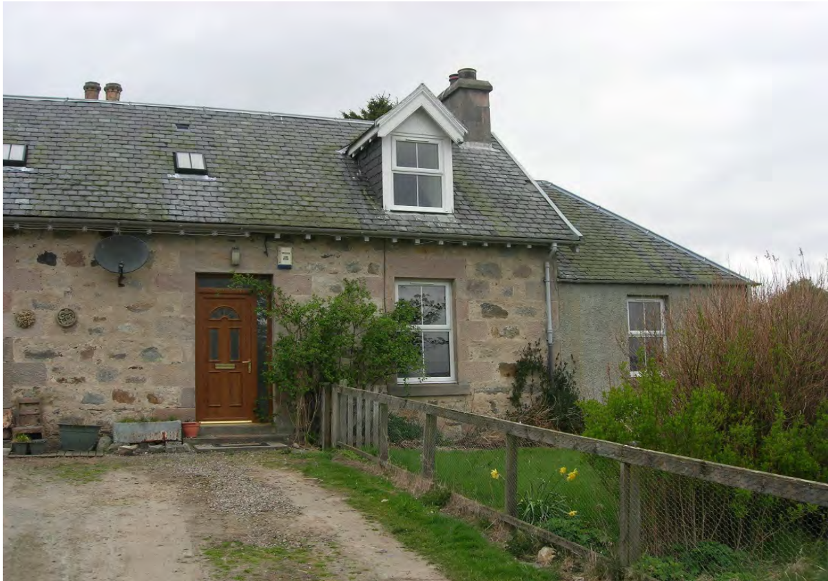
Figure 1. Holm Farm Cottage, showing the original building and the modern bathroom extension on the right.
