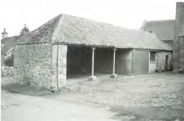
208 Implement shed open to the outer courtyard at Standingstone, East Lothian.
