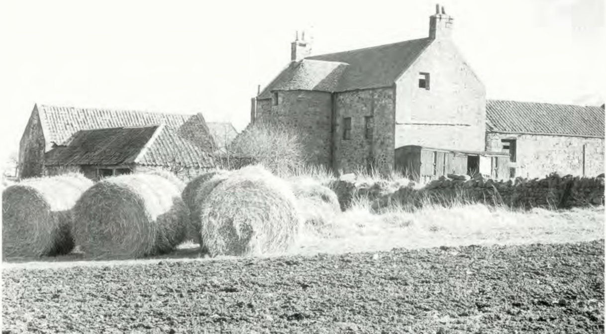
31 A two and a half storey farmhouse with semi-circular rear stairtower at Hilly, West Lothian. The farm buildings are close to the house.
