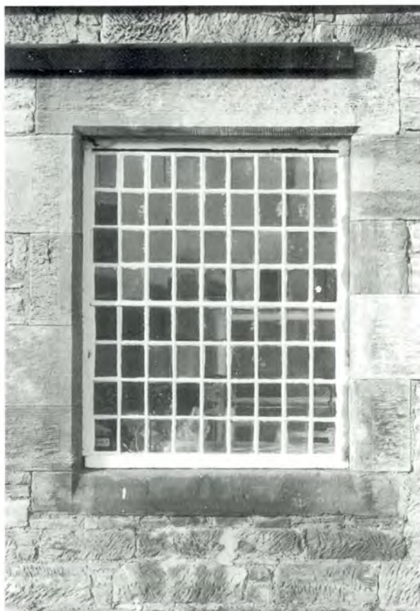
435 Unaltered original cast-iron fixed-light workshop window.
