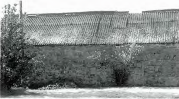
149 A corrugated-iron roof at Buteland Farm, Edinburgh.
