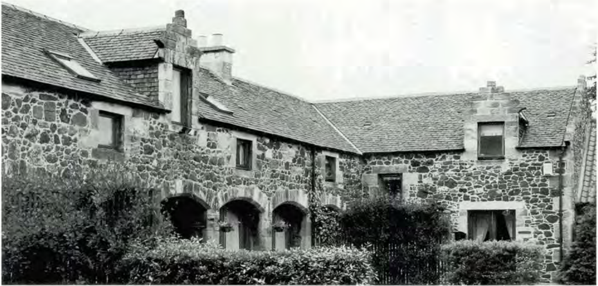
190 New windows in existing dormer openings at Waughton, East Lothian. Single-pane pivot windows have been used, to provide a simple, unfussy replacement for the boarded shutters.
