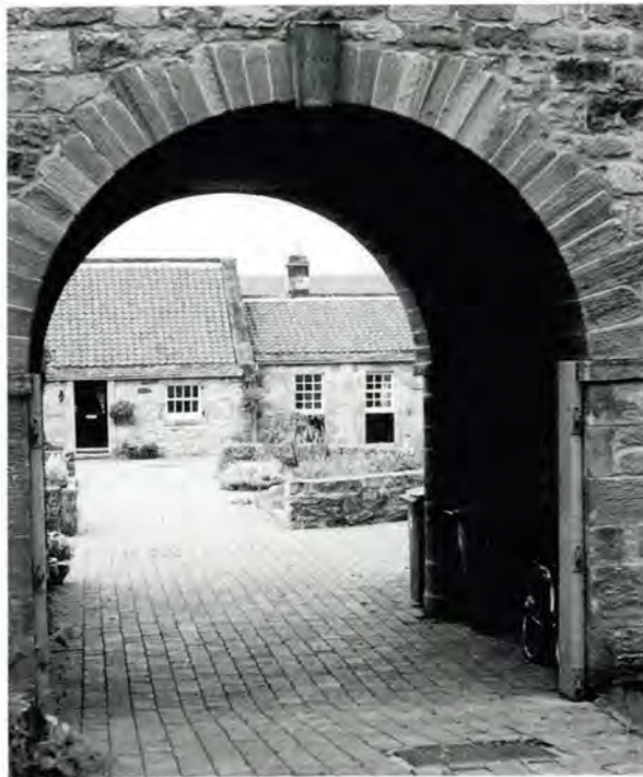
262 The same view after conversion, showing doors altered to form windows. The number of panes in the window on the left has been increased in replacing the window. Sash and case windows have been used in the door openings, with a rather domestic result, but fitting neatly into the openings. Avoiding the strong contrast between the window and the panel below by using a single colour (preferably dark) is usually more successful, as at 253.
