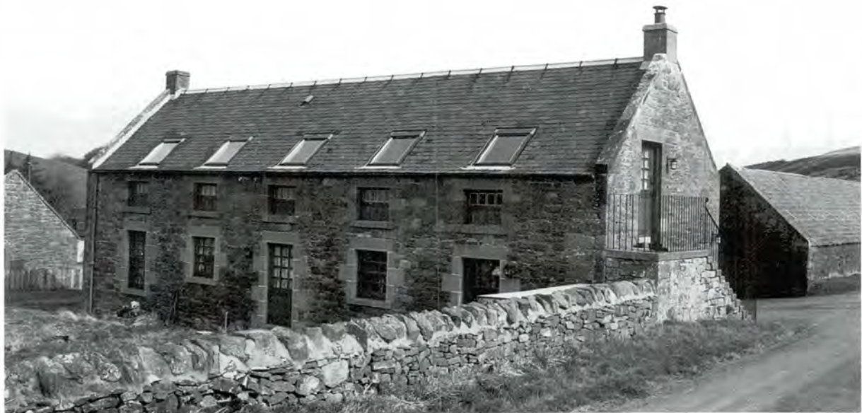
204 The replacement rooflights after conversion at Newmains, East Lothian. They have been carefully arranged to line up with existing openings, but would have looked more like the original ones if smaller and slightly higher up the roof. The ground floor openings are all new and alter the appearance of the building considerably, but the granary windows have been renewed to match the originals.
