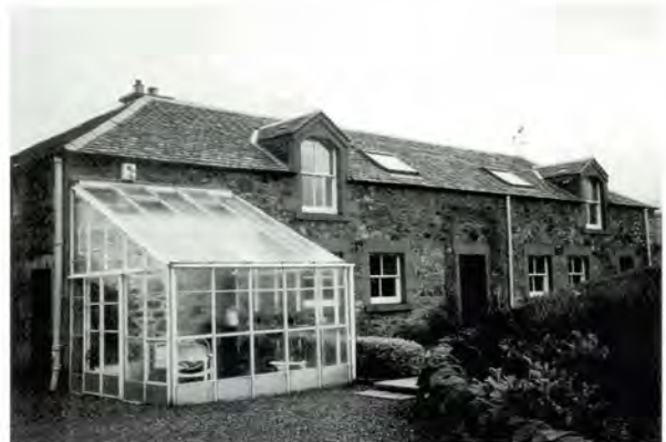
336 An added conservatory (Huntly, Midlothian) unbalances a symmetrical facade.
