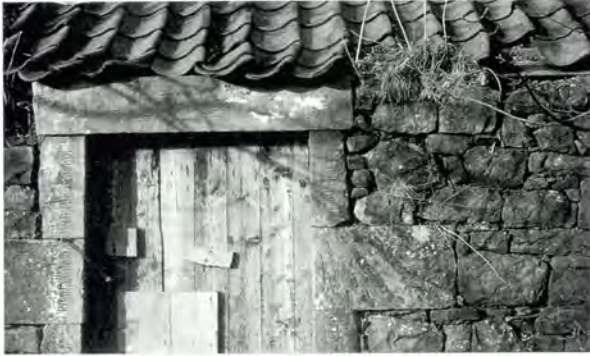
244 Boarded door of very crude construction, employing rather basic methods for securing and repair (West Lothian).
