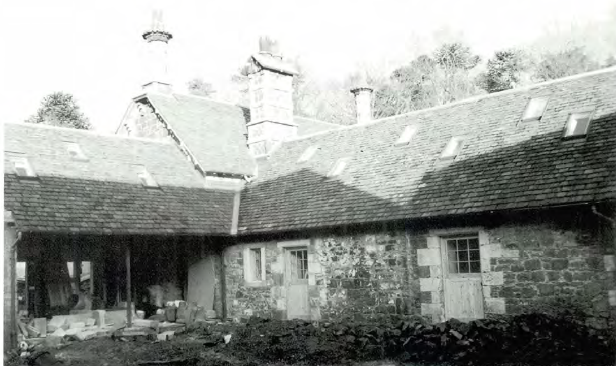
254 Doors renewed to match originals (Gowanbank, West Lothian). Note the pattern of rooflights, which conforms to the original, and uses reasonably small low-profile rooflights, even though of a modern type. This project has tried hard to follow acceptable conservation principles and is generally successful.
