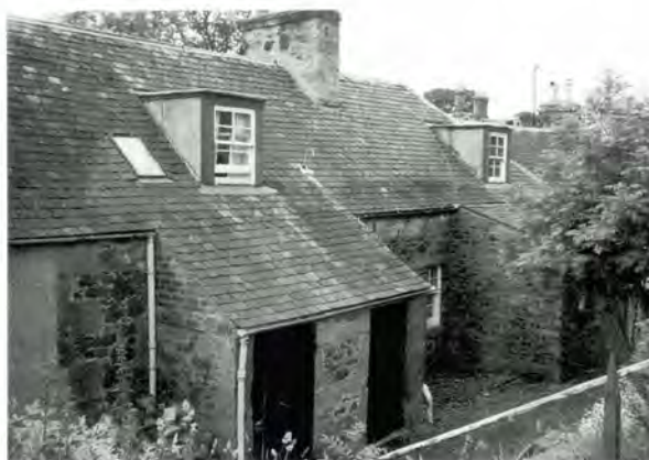
332 Rear view of Sheriffhall Cottages, East Lothian, showing brick and stone outhouses.
