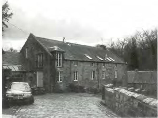
394 View of the watermill at Redhall from the north-east after conversion to two houses. In the roof there are four large new rooflights, a flue and a chimney. There are new glazed windows in the existing openings, even where these would have been boarded. New stone walls divide the road from the other ground.
