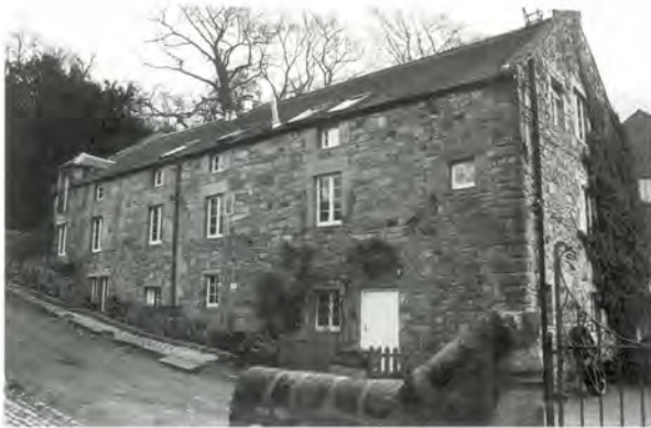
395 View of the north elevation of the watermill at Redhall after conversion. Only one or two of the openings at the lower level have been altered, and the ground level lowered in front of the mill.
