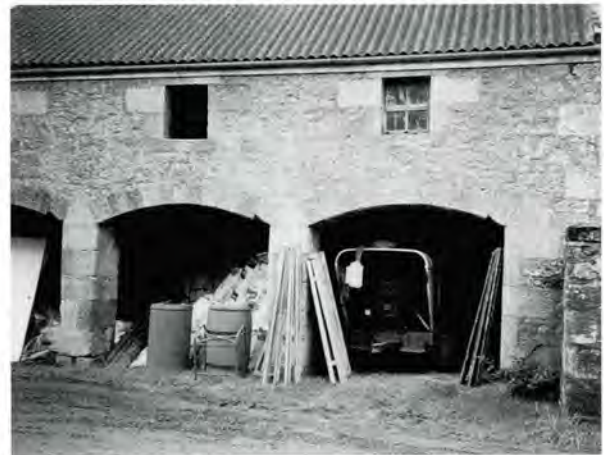
263 Cart arches with windows to granary above (Outerston, Midlothian). Solid rubble masonry, with dressed stones at openings.
