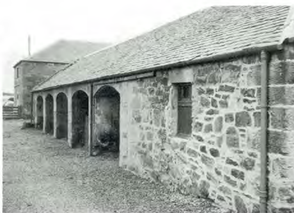
53 Single-storey cartshed at Fountainside, Midlothian.
