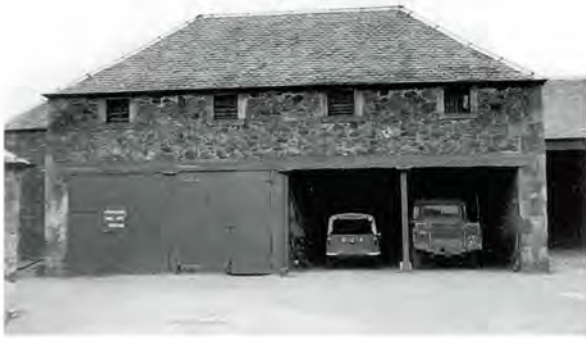
267 Flat-lintelled cartshed openings (Chapel, East Lothian). The lintel is wooden.
