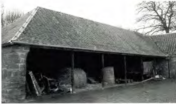
55 Implement shed at Spittal Farm, East Lothian.
