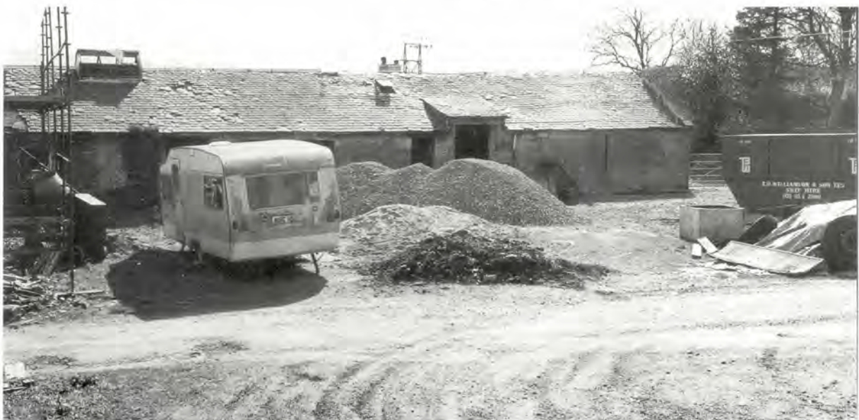
420 The south side of the courtyard during conversion.
