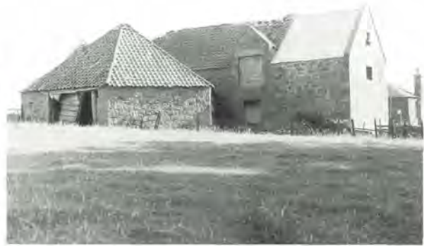
384 The horse mill and barn before conversion. The openings were boarded up and the roof in very poor condition, partly recovered in corrugated iron.
