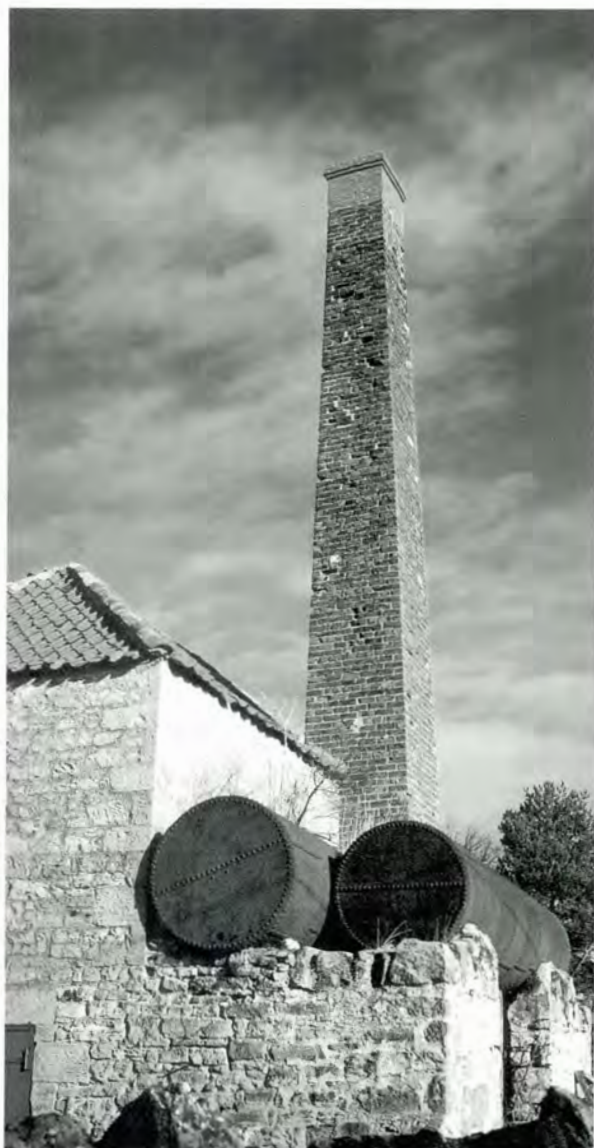
107 Brick chimney stalk at Samuelston, East Lothian. The top has been recently rebuilt.
