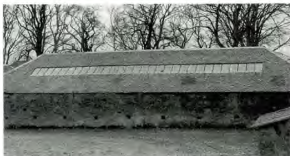
198 A long skylight in a farm roof at Braidwood, Midlothian. This is a traditional method of arranging skylights, especially in industrial buildings.
