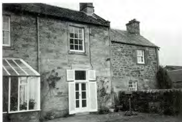
236 A window converted to a door at Yorkston, Midlothian. The proportions, scale and framing are different, heavier and simpler, changing the appearance. But the shutters are the most jarring alteration, being quite out of character.
