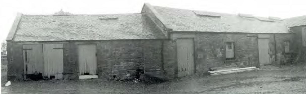
424 The north side of the courtyard (in different ownership) is unconverted.
