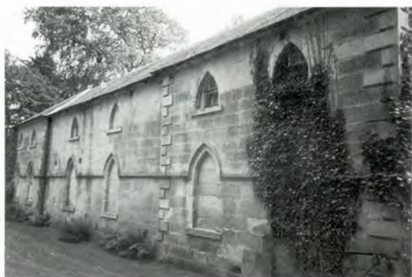
103 A restrained gothic style at Melville Castle's coach house and stable in Midlothian, employing projecting quoins, hoodmoulds running into string courses and tooled ashlar masonry. The windows are regularly spaced, but some are blind.
