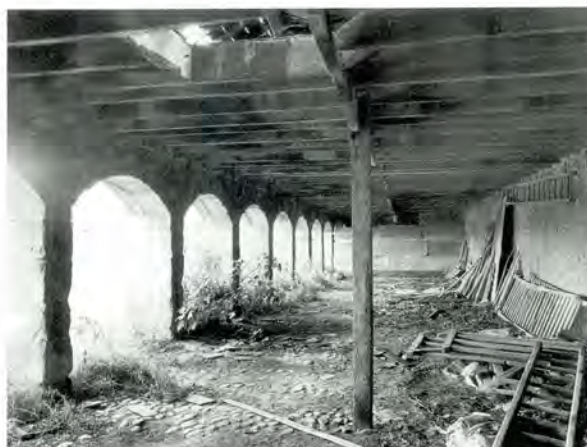
309 Interior of a cartshed (East Barns, East Lothian) showing cobbled ground surface and exposed joists at ceiling. A hatch from the granary above allowed grain to be loaded directly into the carts.
