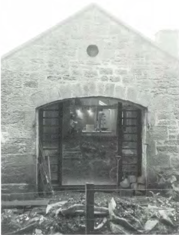
428 The gable arch has deeply recessed window with a dark frame. Original hinges remain, and double doors (vertically-boarded and outward-opening) may be reinstated.
