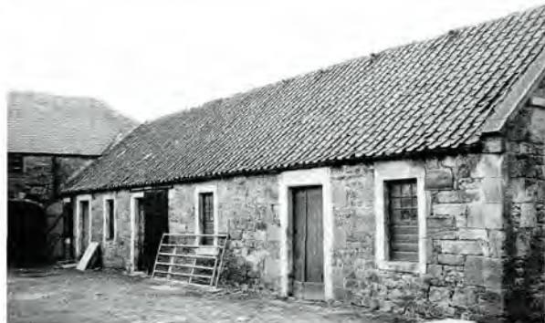
164 Vents in a pantiled roof at Millrig Farm, West Lothian.
