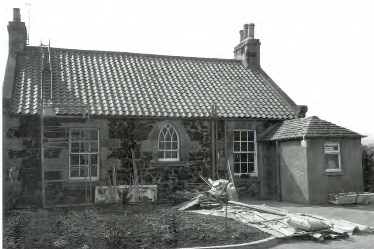
401 Rear elevation of Bield Cottage, showing previous (rendered and slated) extension.
