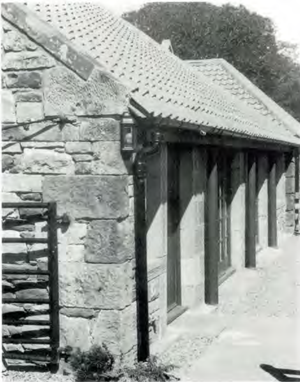
291 Converted implement shed at Garvald Grange, East Lothian. The cast iron columns have been retained and expressed with a screen wall (incorporating windows and doors) built behind them. This at least indicates the original function, and preserves part of the earlier form. The wall is solidly built and well-detailed, but another option is shown in the next illustration.
