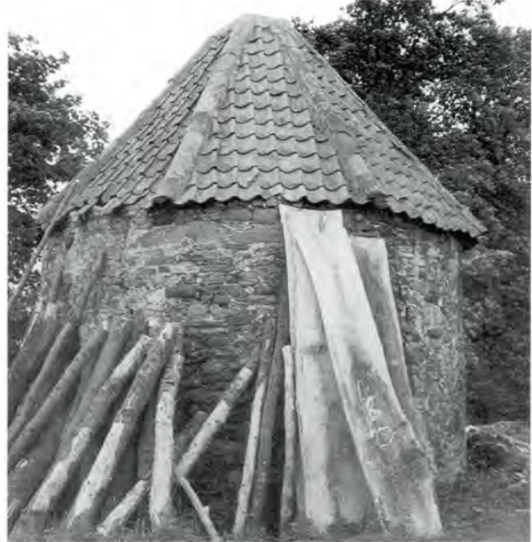
88 Corn drying kiln at Luffness Mill, East Lothian.
