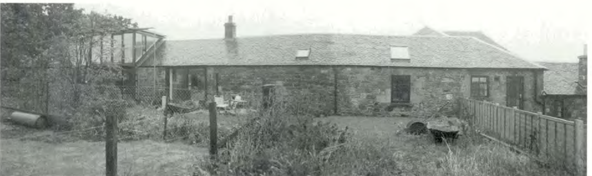
427 Rear elevation showing openings (to left) where masonry has been replaced by windows and roof by the new glazed dormer and balcony. A major change to the character; but limited to one area. See also the open wire fence (to left) in contrast to the neighbour's solid timber fence (to right). As the window head in the bedroom (centre) is low, a rooflight was required for ventilation, but could have been smaller.
