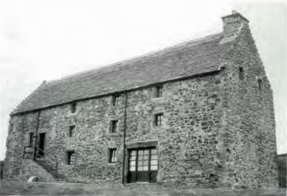
146 The completed roof at Whitekirk. A fine original detail was lost when diminishing courses were not incorporated into the roof detailing.
