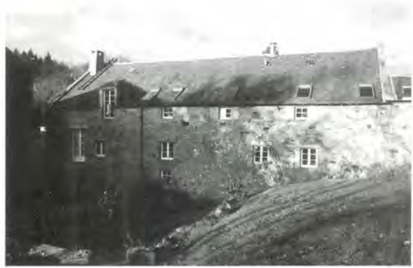
396 The south elevation of the watermill at Redhall, showing the new dormer window, new rooflights, chimney and flue.
