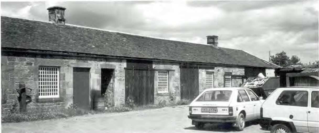
433 Late-nineteenth or early-twentieth century sliding doors to wider openings seen here before renewal.
