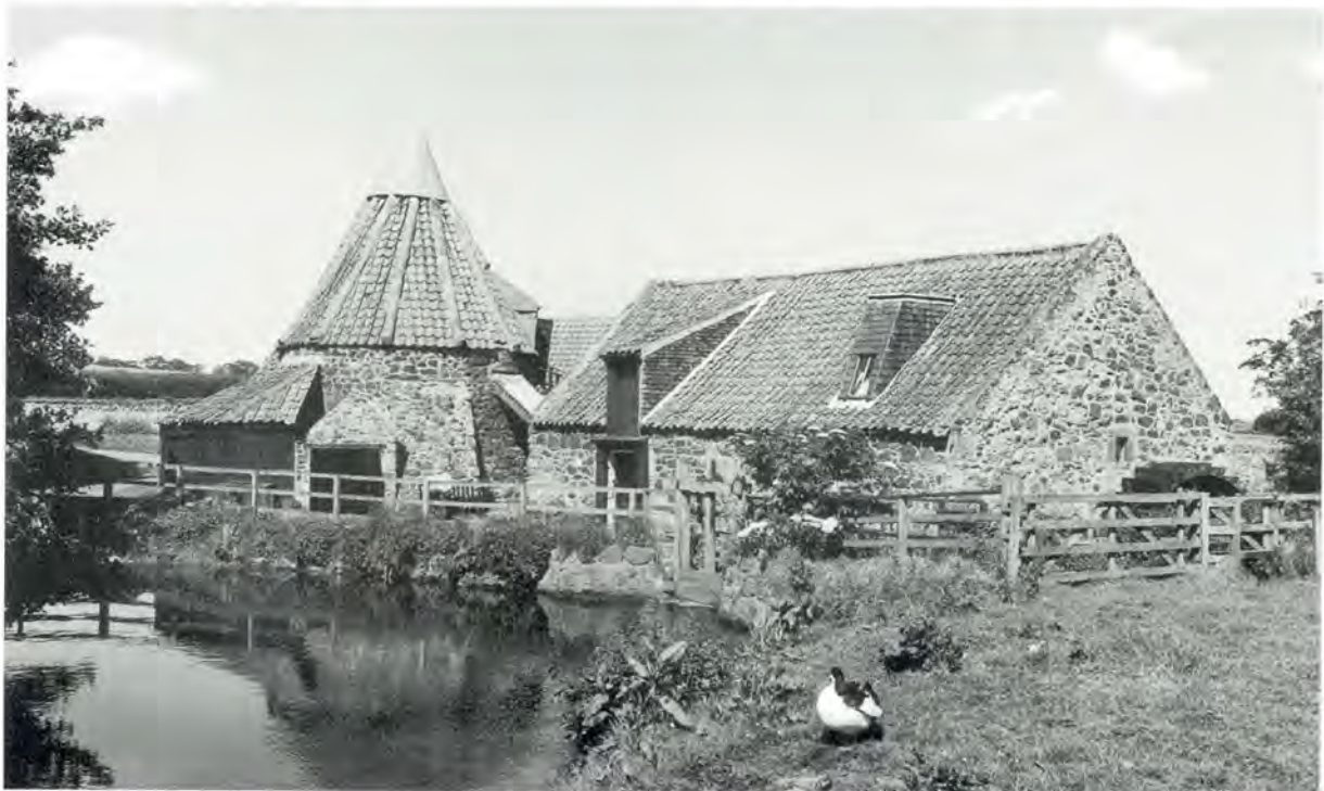
26 Preston meal mill, East Lothian. This seventeenth/eighteenth century watermill is now in the care of the National Trust for Scotland.
