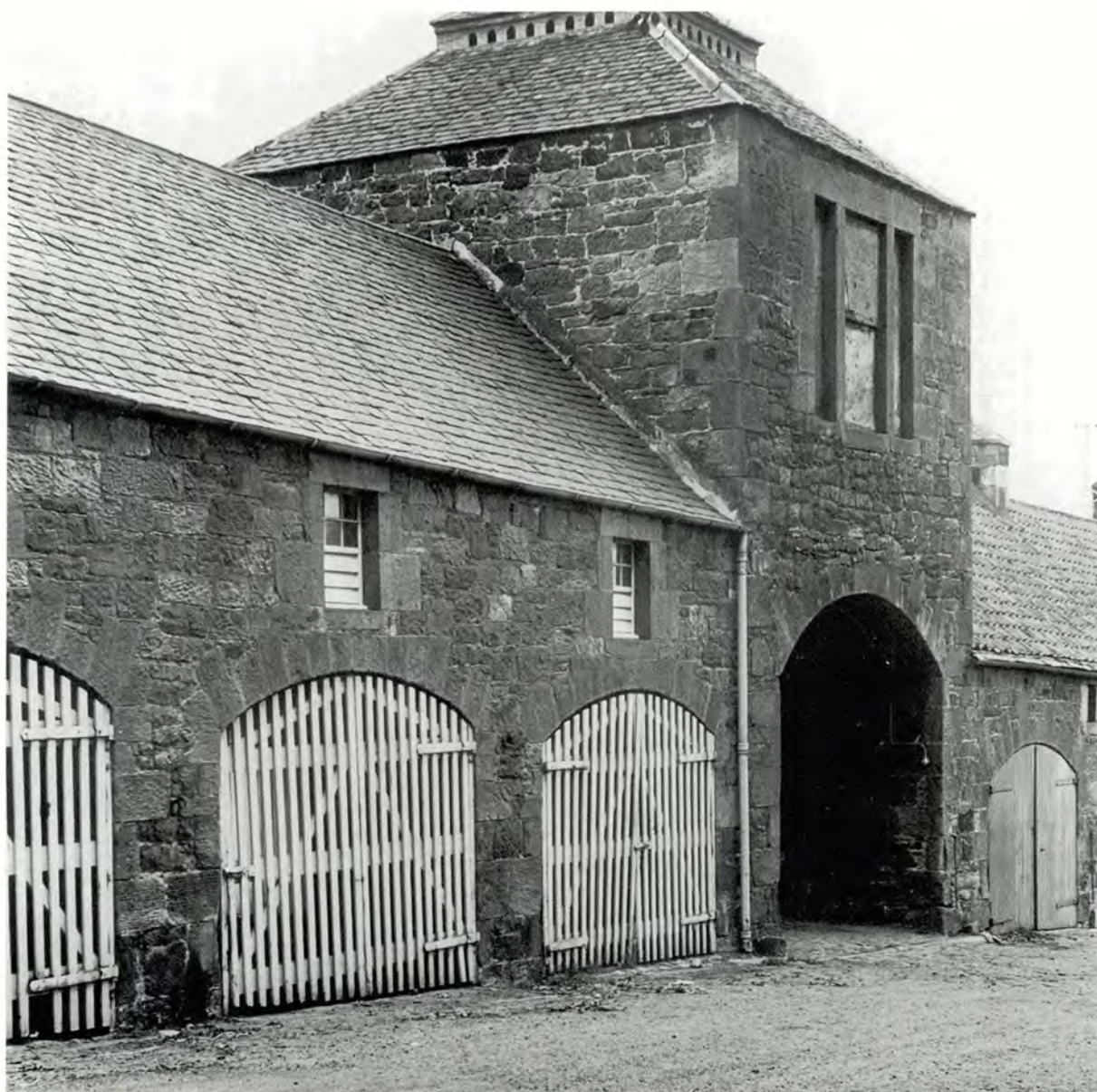
271 Open-boarded doors to cart arches (Harelaw, East Lothian).
