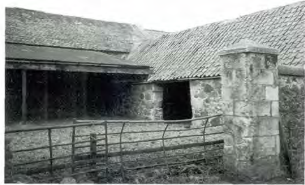
416 Redside steading before conversion; cattle court and shelter shed.
