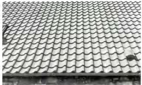
166 Concrete 'pantiles' used in a conversion at Hallhill, East Lothian.
