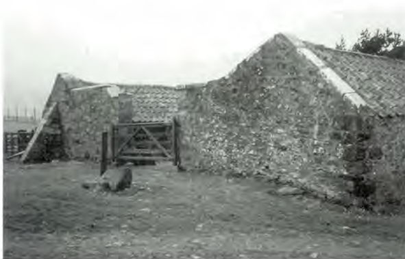
70 Exterior view of sheep house at Glede Knowe, Midlothian.
