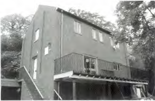
397 The grinding mill at Redhall after conversion, with a new balcony (using the two cast iron columns from the original interior), new access stair, cement-based render over the brickwork, and modern doors and windows.
