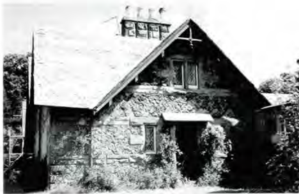
168 Polychromatic slating at Kingscavel Cottages, West Lothian, incorporating a mixture of slate types.
