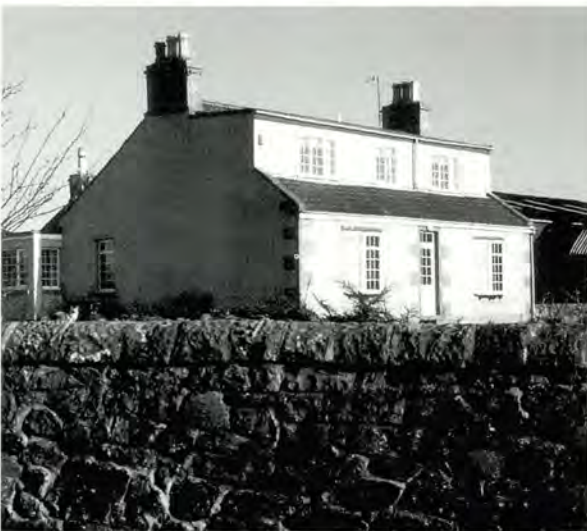
192 Box dormers are not traditional, and drastically alter the profile of a pitched roof (West Binny, West Lothian).
