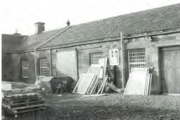
432 This illustration also includes the same part of Thornybank Steading after window alterations and renewal of the door.
