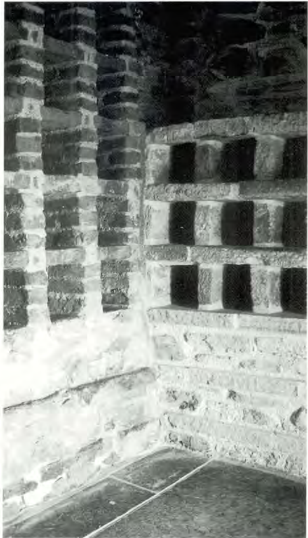
446 Existing brick and stone nesting boxes have been retained.
