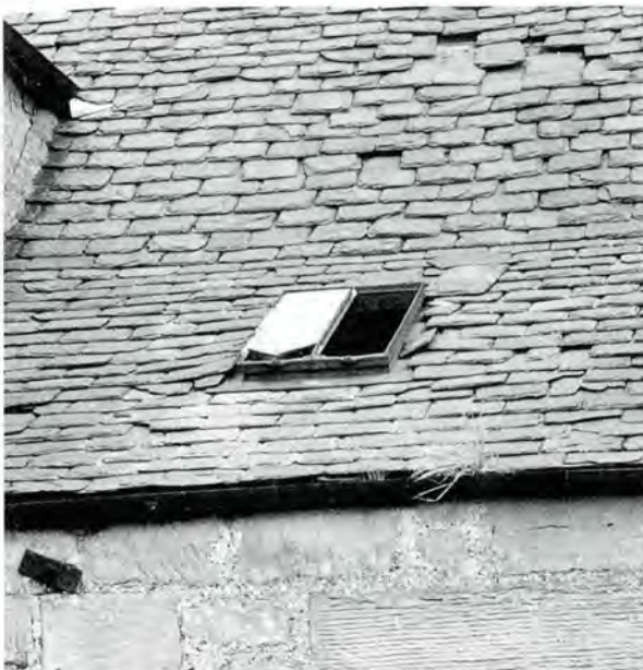
195 Traditional cast-iron rooflight, with central astragal at Waterstone, West Lothian.
