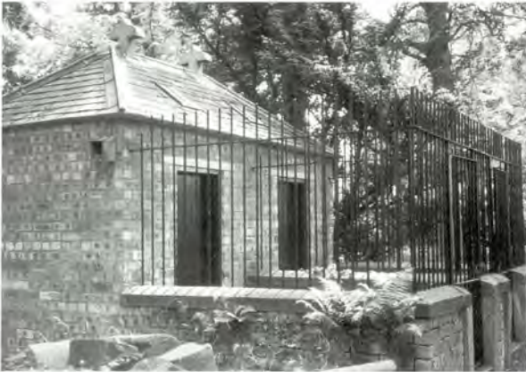
41 Kennels at Stobshiel, East Lothian. Note the brick construction and Welsh slate roof.
