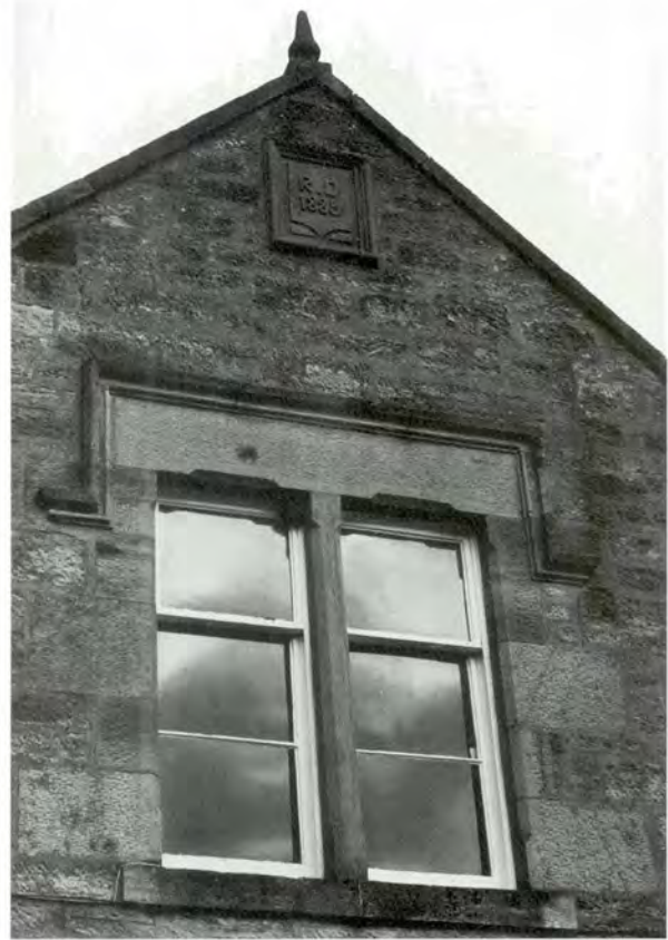
214 Victorian three-pane, vertically-sliding, timber sash and case windows, arranged in a pair (Temple farmhouse, Midlothian).
