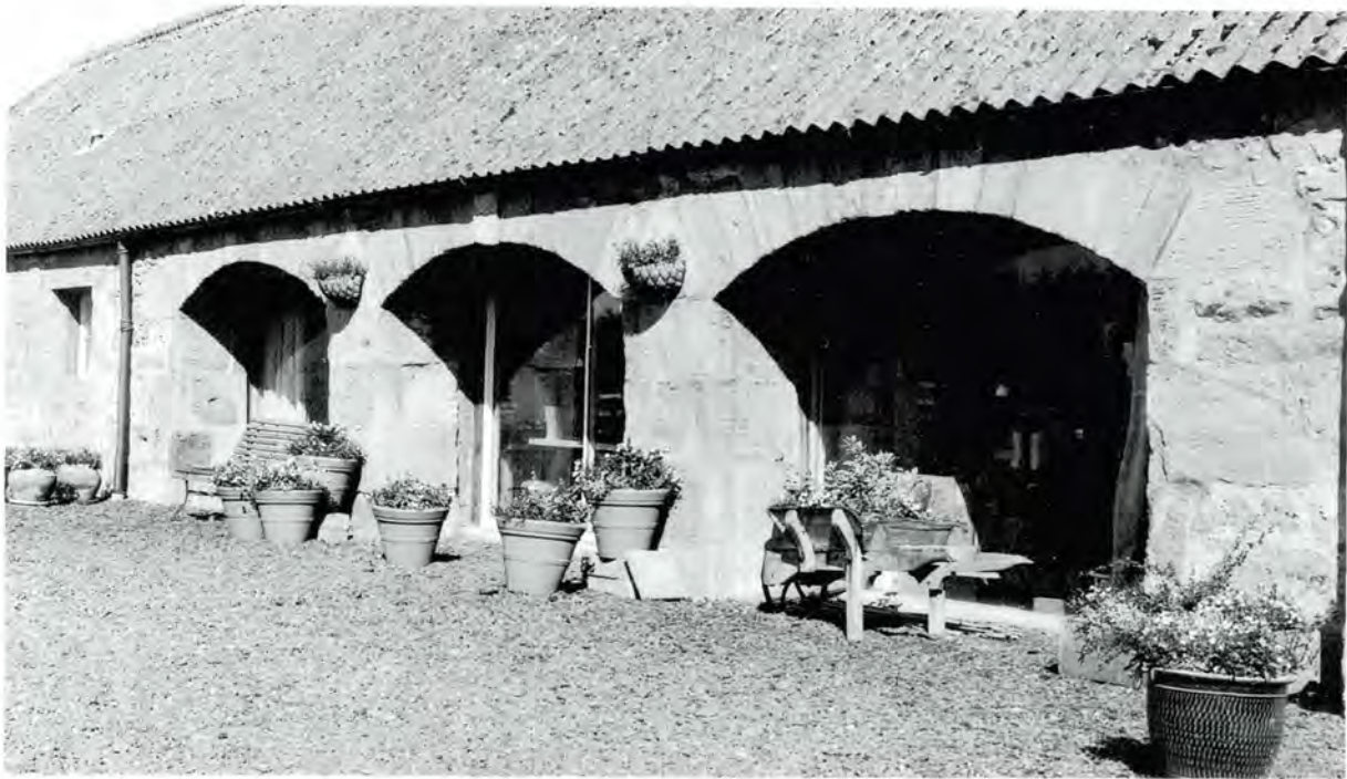
281 Another successful glazed infill to cart arches at Myreside, East Lothian, where the cartshed has been converted to workshop and office use. The glass is deeply recessed so that the openings still read as arches, and framing (very slender) is only visible in the central arch. If this had been of a darker colour, rather than white, it would hardly have been visible.
