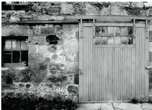
272 A sliding door (boarded and partially glazed) conceals the opening behind (Almondhill, Edinburgh).
