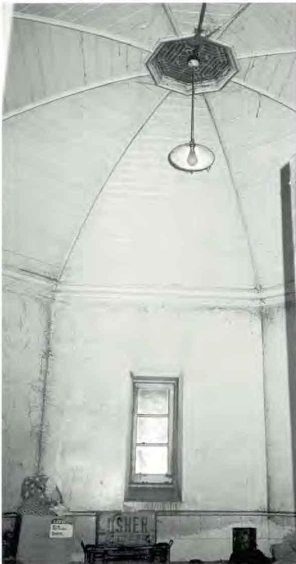
318 Dairy interior at Hedderwick Hill Stables, East Lothian. There are tiles below the dado and the upper walls are plastered. The window is small, and the ceiling high and vented, to keep the space cool.
