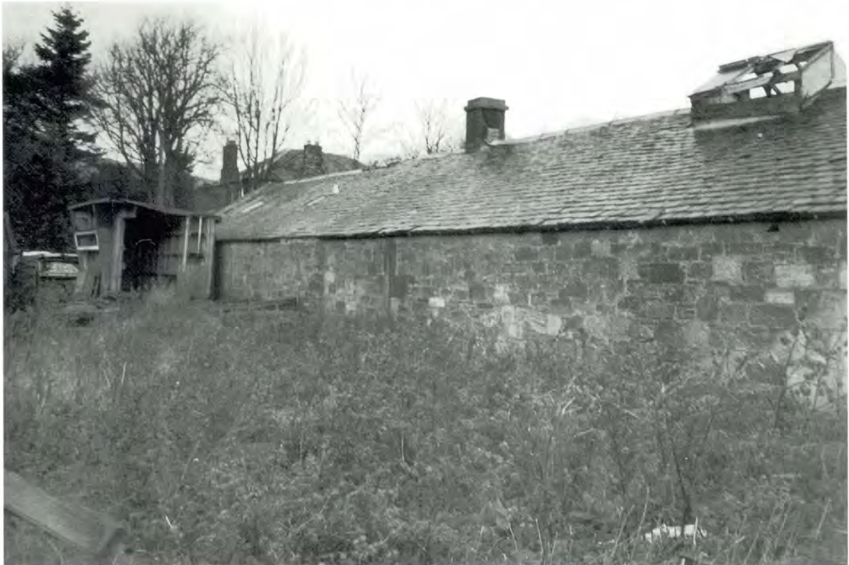
421 The same range seen from the rear before conversion.
