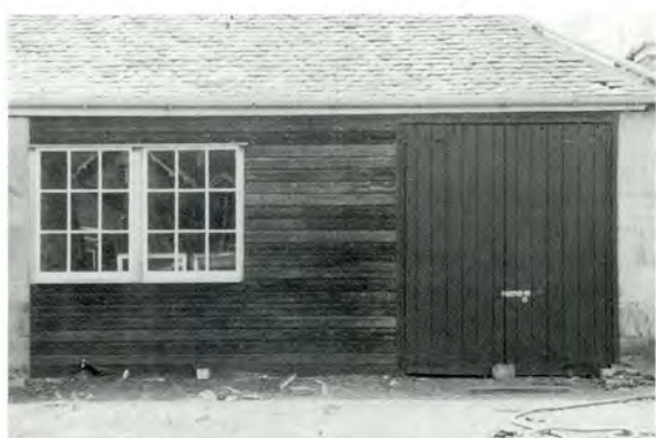
438 Store after erection of screen wall with doors and windows.
