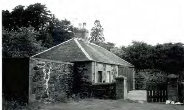
328 A separate stable and stableyard at Balgone, East Lothian.
