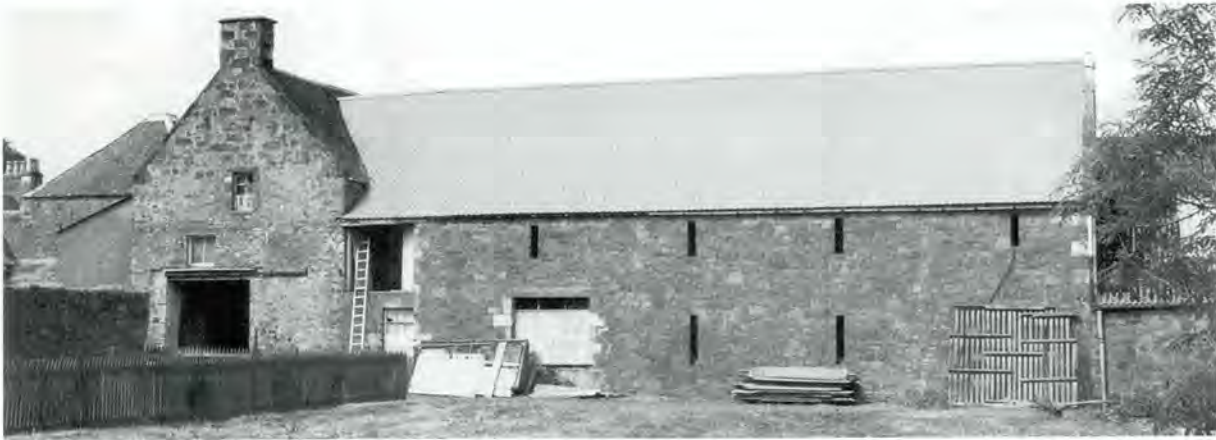
230 Ventilation slits in a barn at Drem, East Lothian.
