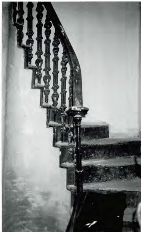
302 Modest stone stair with cast iron balustrade and polished timber handrail.
