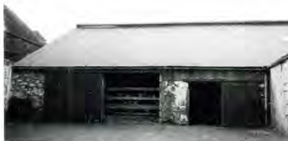
182 New sheet-metal roof at Rosebery Home Farm, Midlothian.
