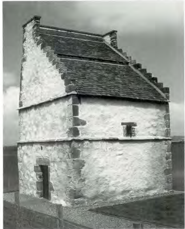
441 Athelstaneford doocot from south after repair and reharling, showing the new gravel path and simple wire fencing.
