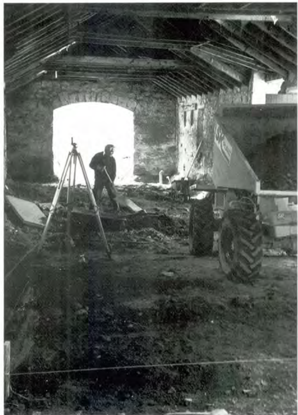
422 Interior during conversion.
