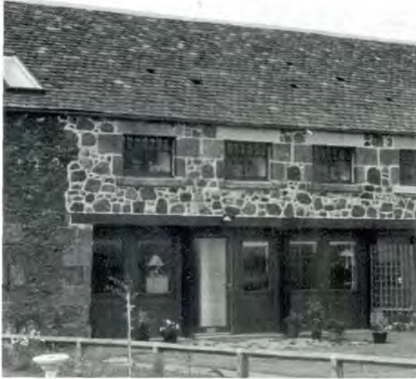
413 Detail of granary windows after conversion
