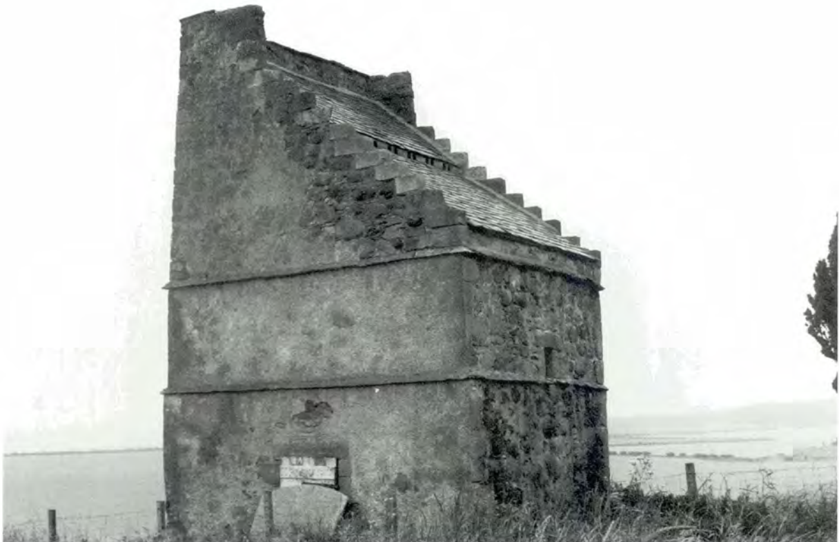
440 Athelstaneford doocot from south-west before works.
