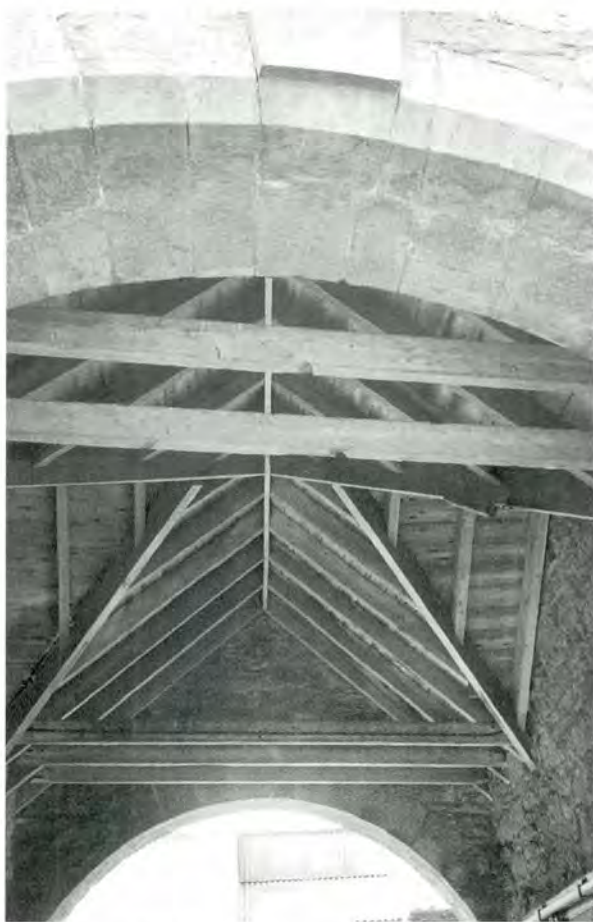
186 Internal roof structure to pend at Wamphray, East Lothian.
