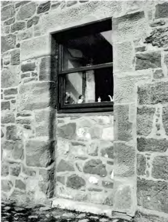
257 A modern example of doorway infill (Newmains, East Lothian). Both the window and the stone blocking are recessed, to leave the original shape showing, but the visual division into two distinct parts detracts from the form.
