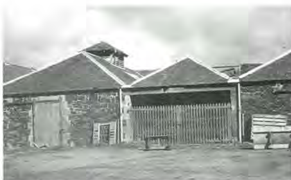
176 Slated roof at Bangour, West Lothian, with zinc ridge flashings and valleys, cast-iron rainwater goods, small pipe ridge vents to the left and a larger box vent.
