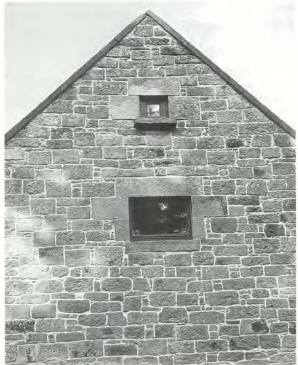
386 The south gable after partial reconstruction. Stones were numbered and reused, so that the rebuilt area is not visibly different from the original. Inward-opening casement windows have been provided in the existing openings.
