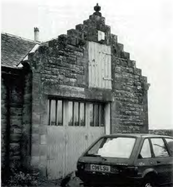
293 Enlarged gable opening (Gladhouse Villa, Midlothian). The widening has been to one side only with an asymmetrical result.
