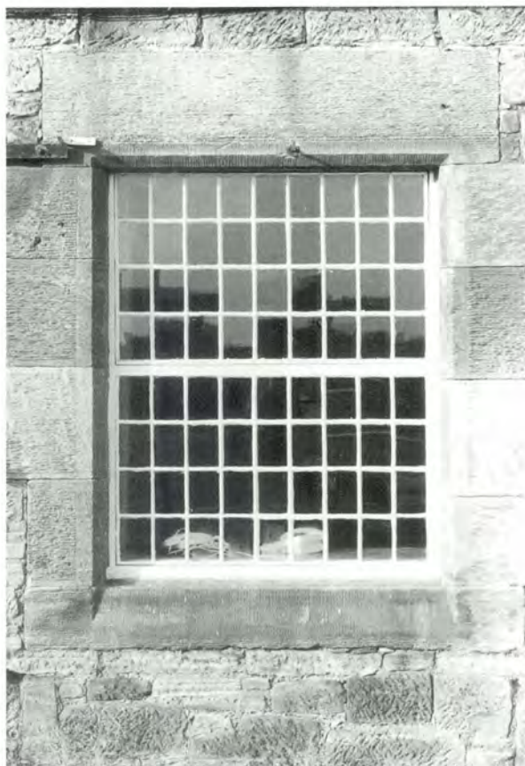
436 Workshop window after alteration to include opening hopper.
