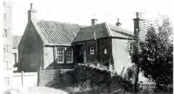
382 The cottage at Cauldhame before repairs and refurbishment.
