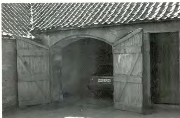
270 An arched opening with double doors. They are ledged, braced and boarded, side-hung and outward-opening (Bridgend, West Lothian). This gig house is eminently suitable for use as a garage.
