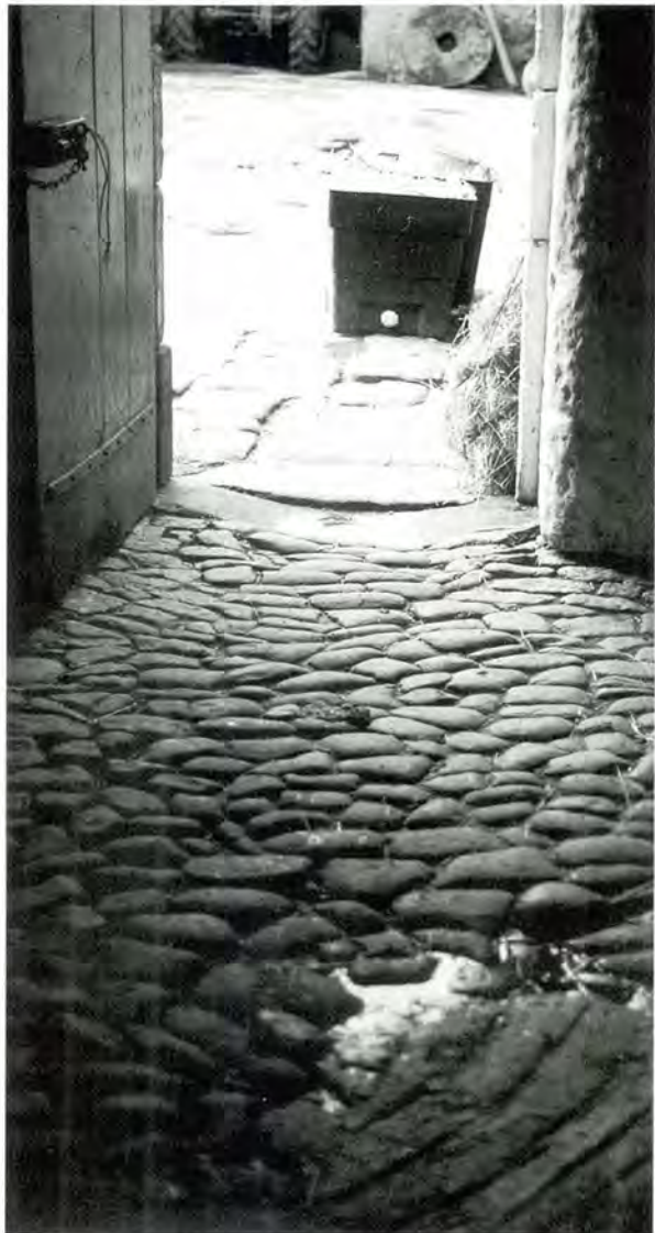
305 Cobbled stable floor (Wester Gormyre, West Lothian).
