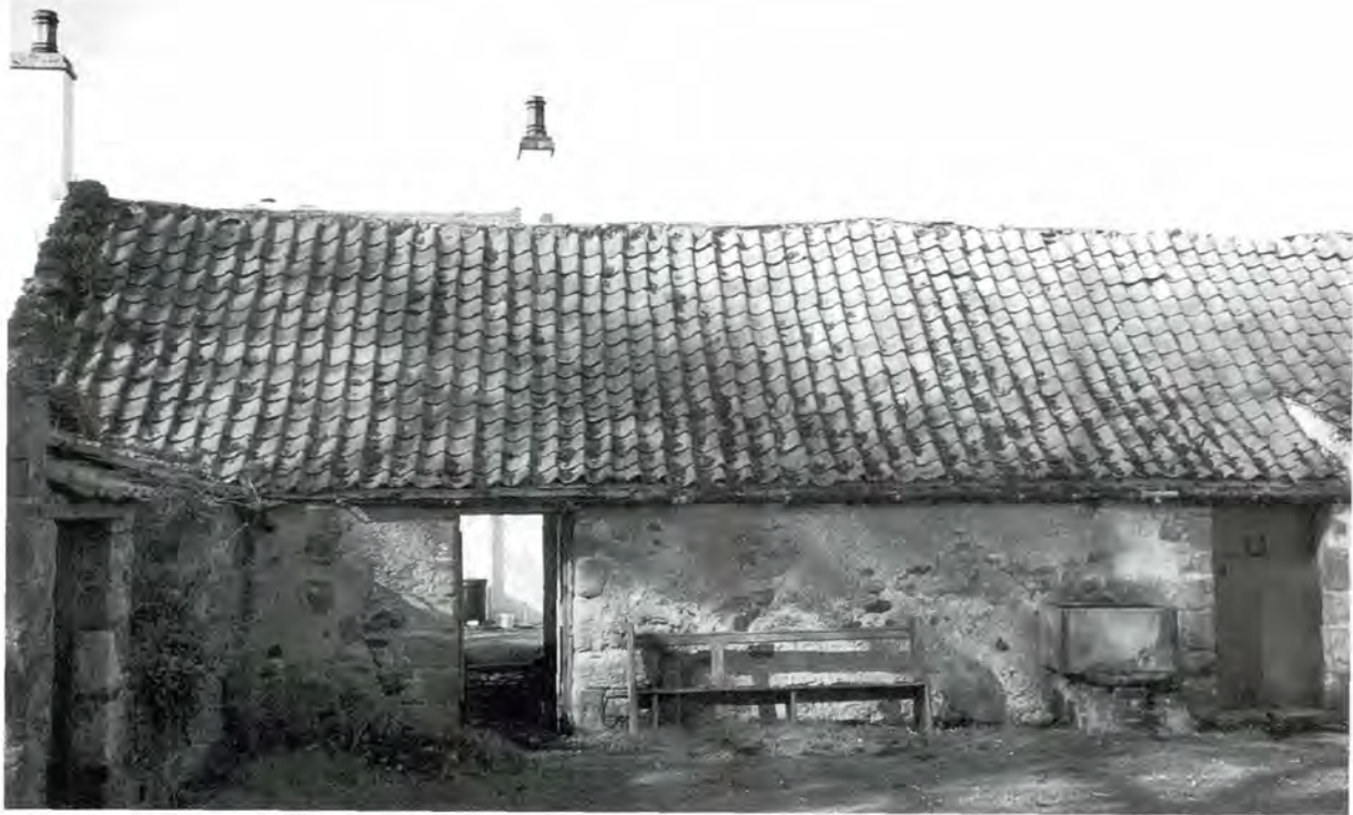
130 Lime harl to walls at Luffness Mill House, East Lothian.
