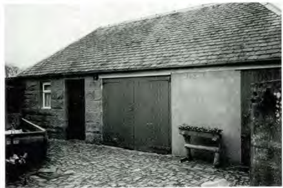
115 This alteration to the openings at Millbank Cottage, Midlothian, has employed a cheaper material than stone, and masked its use by rendering the affected area of wall, and lining it out to match the scale of the masonry. The render is an inferior and less distinctive material than the original stone.
