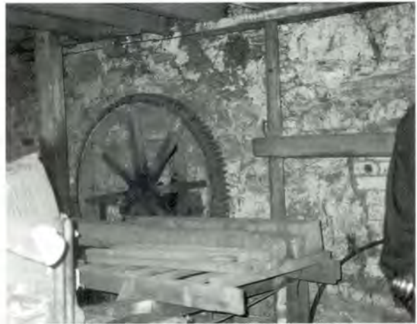
319 Interior at Mavishall Sawmill, East Lothian, including machinery.
