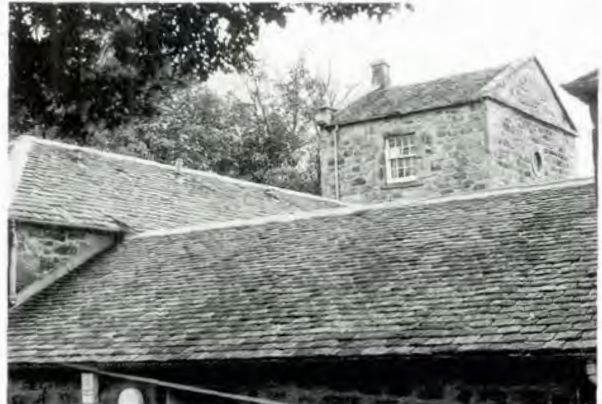
148 West Highland slates on roofs at Calder House Steading, West Lothian.
