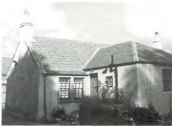
383 The cottage after repair: the later chimney has been removed from the extension and the render stripped and replaced by a lime harl. The windows have been repainted in a dark stain.
