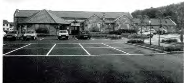
358 Vast parking areas dominating the converted steading at Lauriston Farm, Edinburgh.
