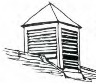
Wooden louvered box ridge vent at the Brunt, East Lothian. The cap is metal, the flashings to the slates are lead or zinc.
