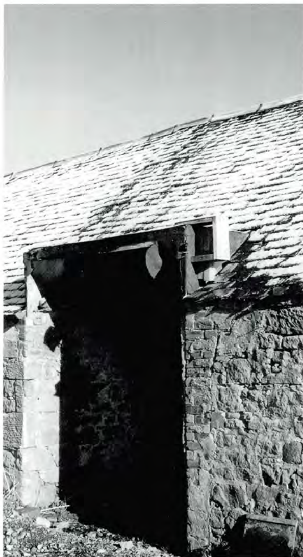
273 An existing opening heightened and widened (note brick to one side) to accommodate larger farm vehicles (Buteland, Edinburgh).
