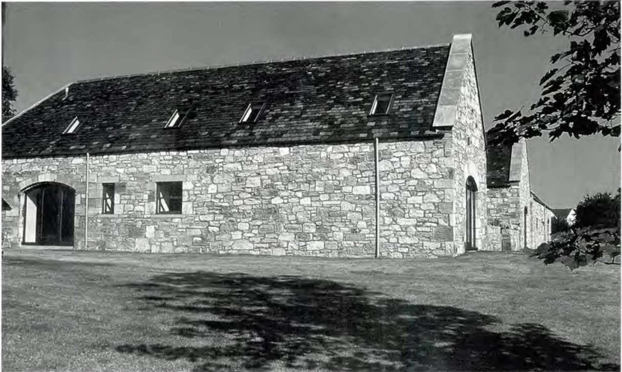
125 A reconstructed farm building at Boghall, West Lothian, with raised wallhead. As in the previous examples, the rubble masonry is not levelled off every few courses as authentic traditional rubble usually was and the courses tend to curve gently. However, the use of smaller stones as pinnings, and the variation in the size and shape of stones is slightly better in this case.
