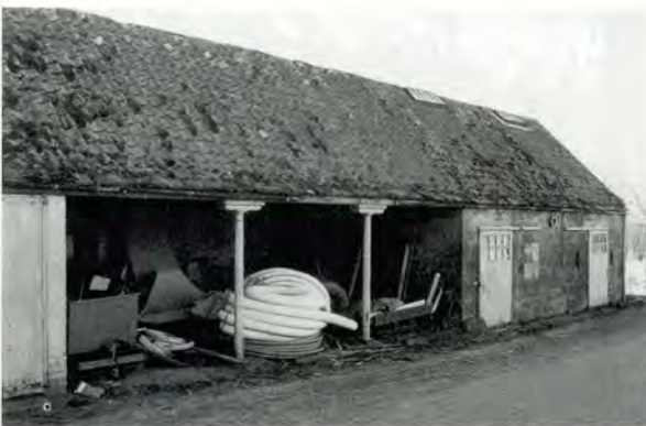
277 Implement shed, with typical flat lintels and cast iron columns (Lennoxlove, East Lothian).
