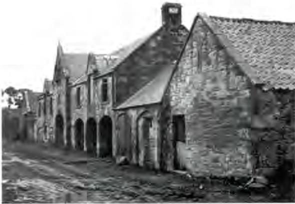
211 Gables and cart arches arranged symmetrically to either side of a central pend on this elevation at Ballencrieff, East Lothian.
