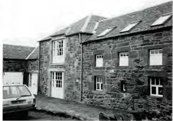
233 New windows which in some of the openings maintain or to some extent reflect the previous window forms. But the windows at the left have changed completely from the originals, whatever these were. They would all be better painted a darker colour. The wallhead may have been heightened. (Newmains, East Lothian).
