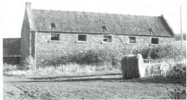
203 Rooflights in a granary at Newmains, East Lothian, before conversion to residential use.
