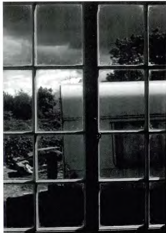
218 Original (circa 1860) double side-hung casement window at Gowanbank, West Lothian.
