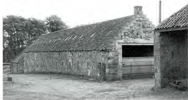
197 Glass paniles spaced regularly along a roof at Millrig, West Lothian.
