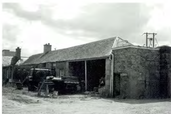
437 Open-fronted store at Thornybank standing before enclosure.
