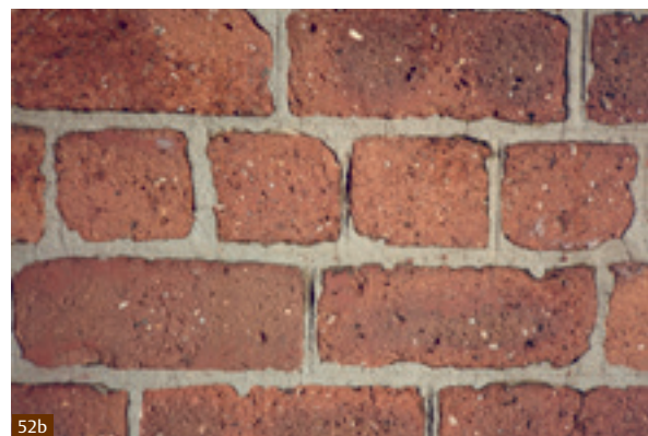
Fig. 52 Damage to brickwork from cleaning. The vitrified surface (known as the fire skin) which can be seen on the un-cleaned brick (a) has been removed from the cleaned brickwork (b) leaving the brick more vulnerable to moisture penetration and decay.
