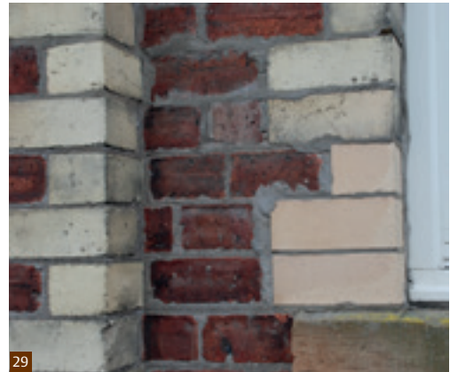
Fig. 28 Inappropriate patching-in of bricks of the wrong colour set in hard cementitious mortar giving a poor quality repair.
