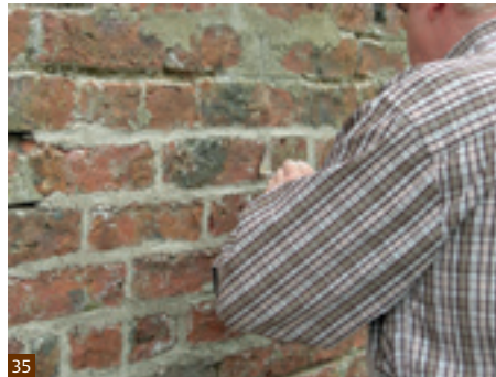
Fig. 34 New mortar is pushed back firmly into the pre-dampened joint using an appropriately sized tool.
