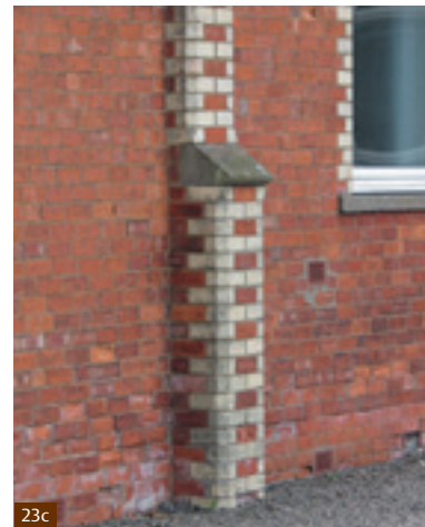
Fig. 23 Special shaped bricks in use for a variety of applications: a. Bullnose bricks used for window cill; b. Arch voussoirs bricks; c. Splayed bricks for corner details.
