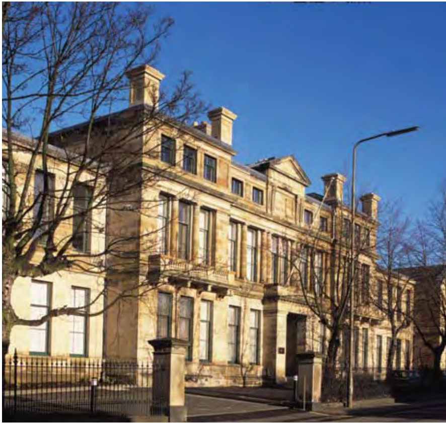
Fig 7.7 Former Edinburgh Hospital for Incurables, Longmore House, Edinburgh, converted 1993-4.
