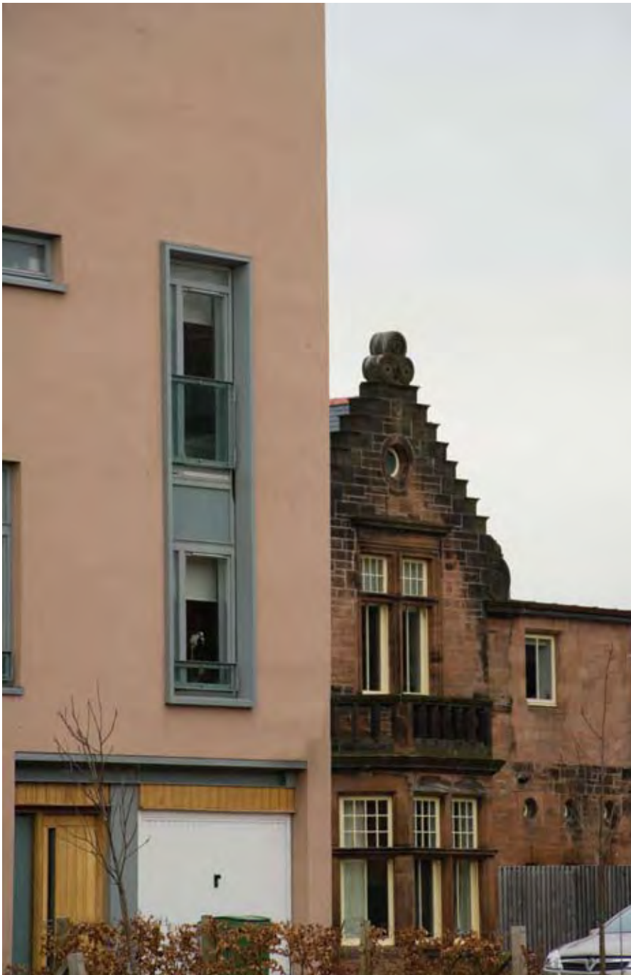
Fig 7.4 Former City of Glasgow District Asylum, Gartloch, converted from 2003.
