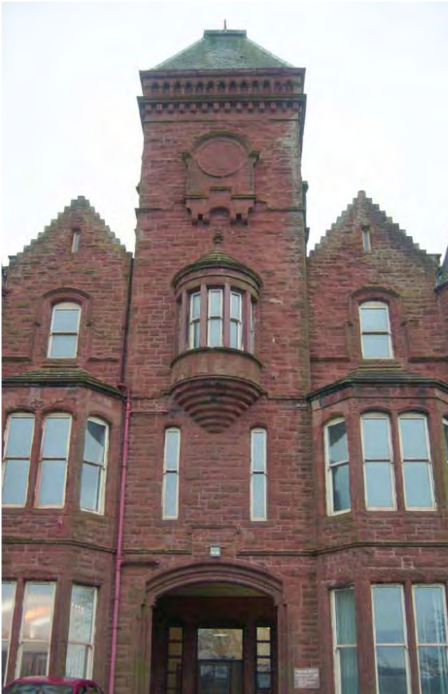
Fig 4.8 Detail of Ravenscraig Hospital, Greenock, John Starforth, 1876-9.
