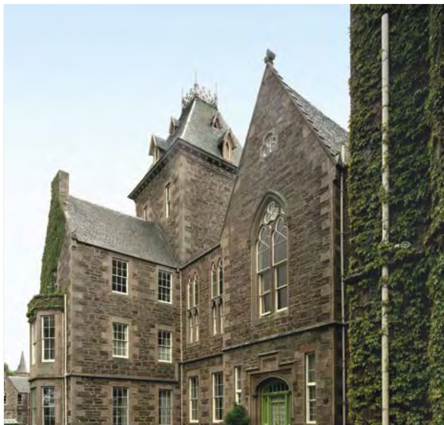
Fig 3.4 South front of Craig Dunain Hospital, Inverness, James Matthews, 1864.
