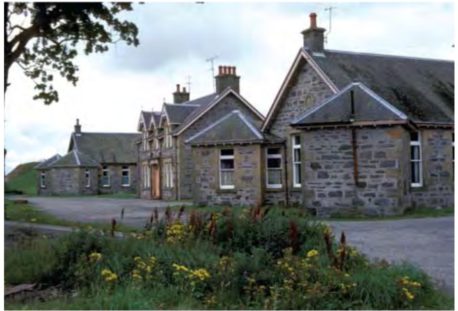
Fig 5.3 Former Meadowside Hospital Kincaig, Alexander Cattanach, 1906.
