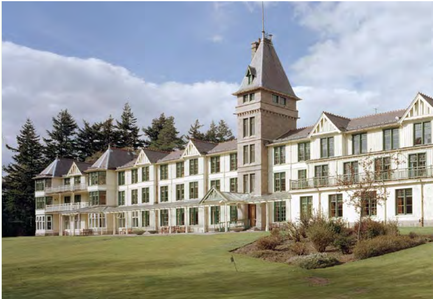
Fig 5.8 Nordrach-on-Dee Hospital, Deeside, George Coufts, 1900. © Crown Copyright: RCAHMS. Licensor www.rcahms.gov.uk
