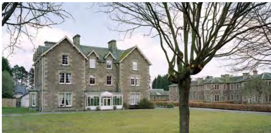
Fig 3.7 Pinel Lodge, Murthly Hospital, Perth, built in grounds of hospital, 1894.
