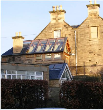
An extension to a house in a conservation area, set back from the front elevation, of glass and timber that echoes conservatories in the area.
