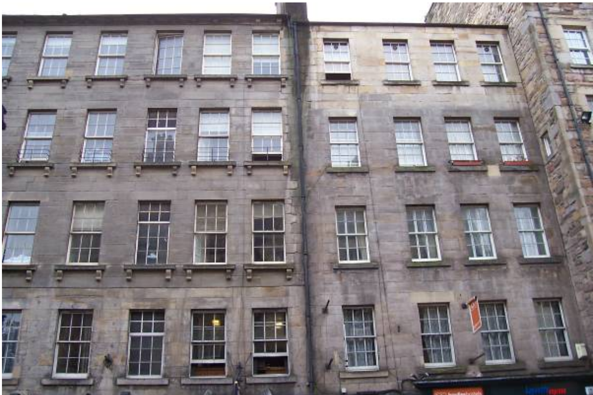
Figure 4. Glazing forms a large proportion of many tenement walls
