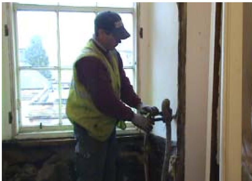
Fig. 3. Insulation being blown behind the existing linings
