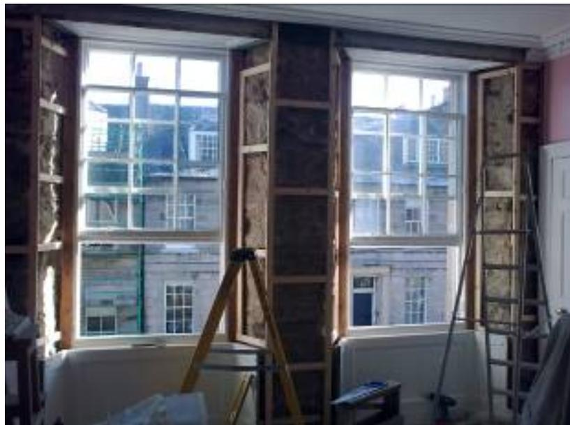
Fig. 30. Reframing and wall upgrade work
