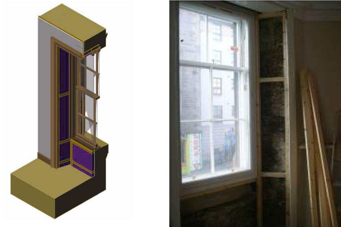
Fig. 17. Diagram and photograph showing reframing around window opening
