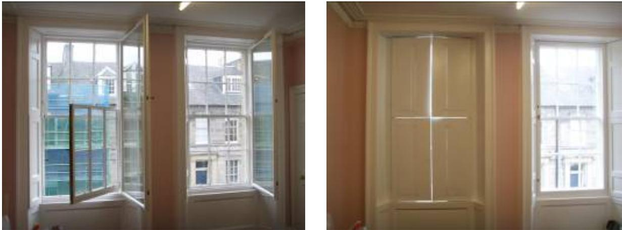
Fig. 33. Completed works showing function of secondary glazing, simplex hinges and shutters
