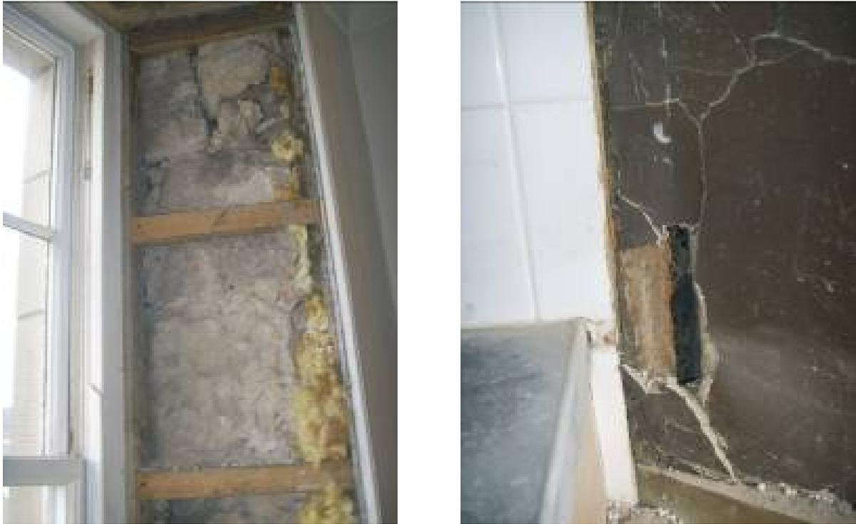
Fig. 25. Sealing of wall edges prior to insulation being blown in
