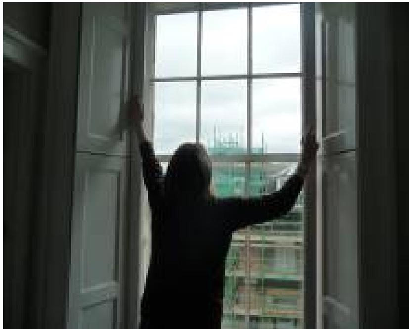
Fig. 36. Tenants pointed out that “you have to stretch both your arms wide and push hard to close the window from the tilt position. Not easy unless you are tall and strong”.
