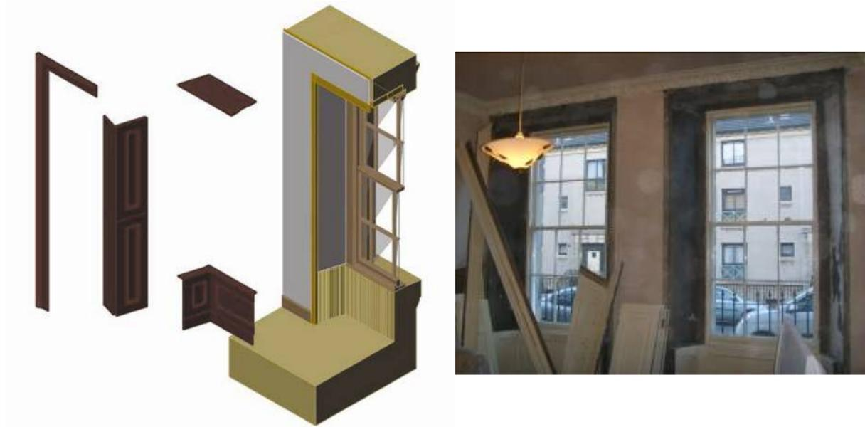
Fig. 2. Diagram and photograph showing dismantling of the window sets
