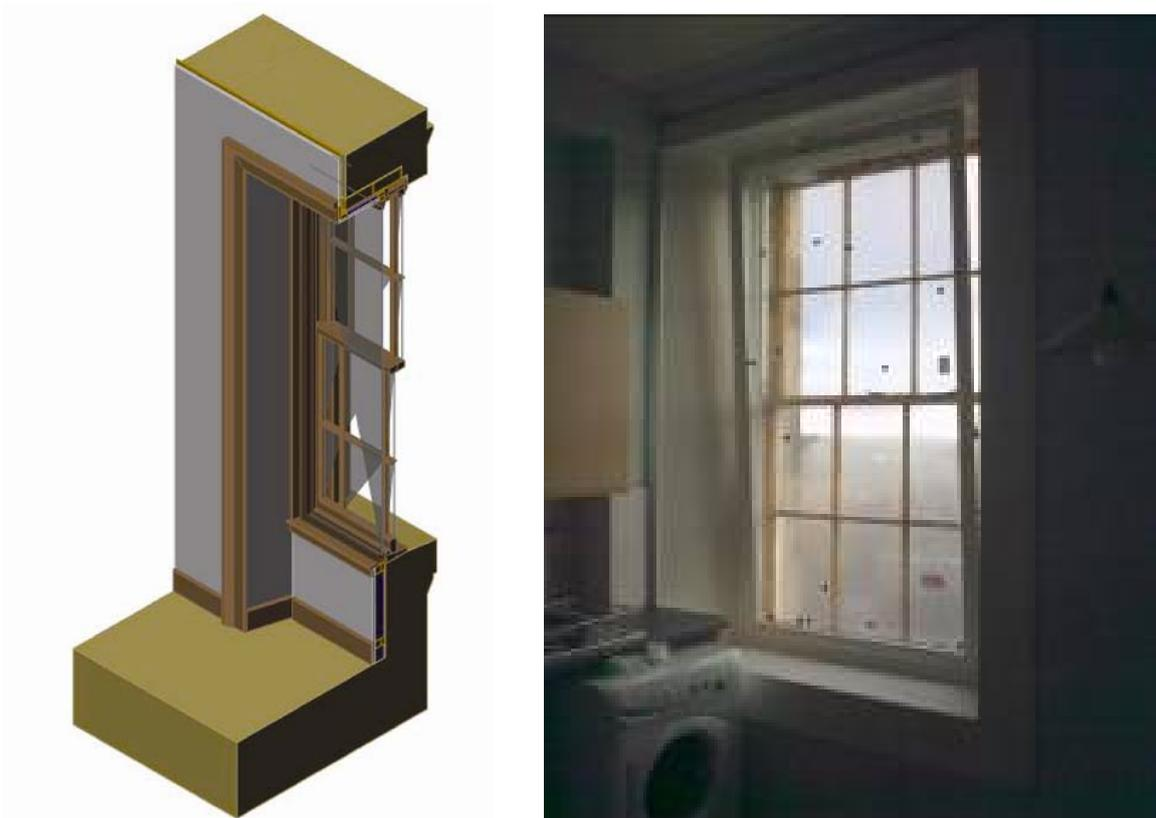
Fig. 27. Completed works to window opening showing tilting secondary glazing
