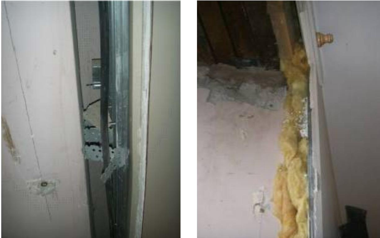
Fig. 14. Open gaps (left) and gaps filled with mineral wool (right) prior to blown insulation
