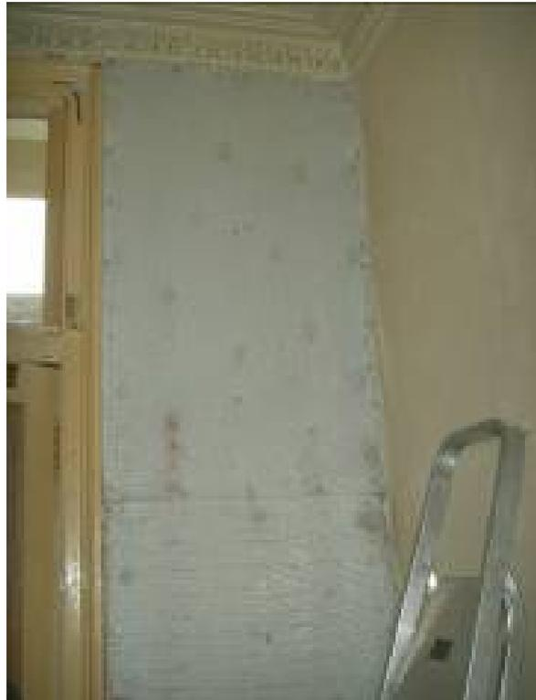
Fig. 9. Thin internal wall insulation
