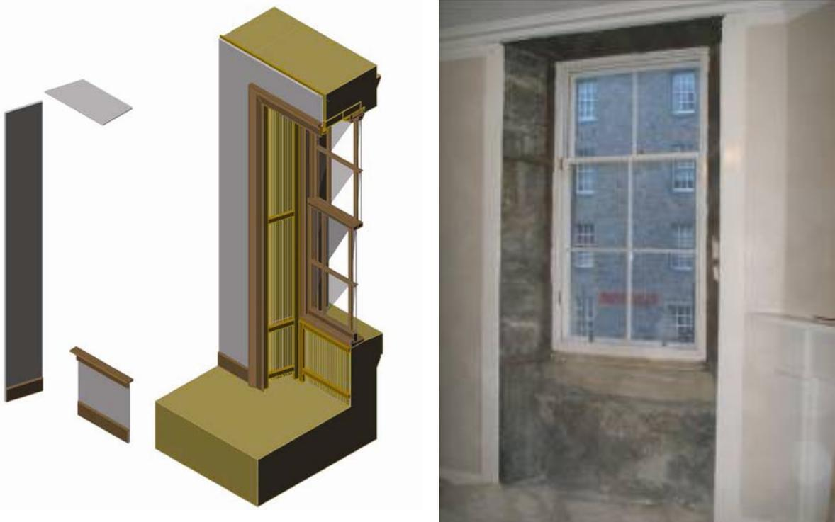
Fig. 16. Diagram and photograph showing downtakings
