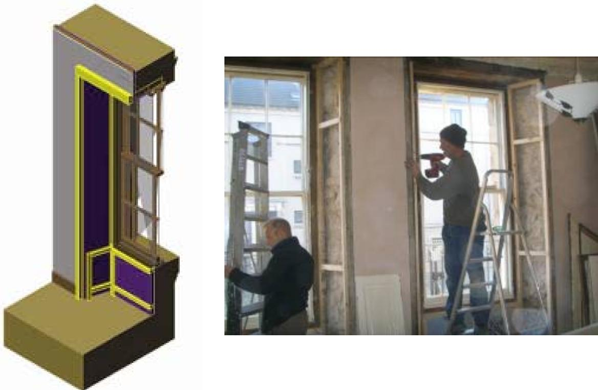
Fig. 4. Diagram and photographs showing reinstatement of window framing
