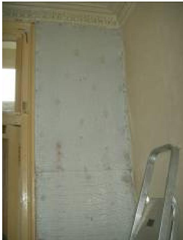
Fig. 9. Thin internal wall insulation
