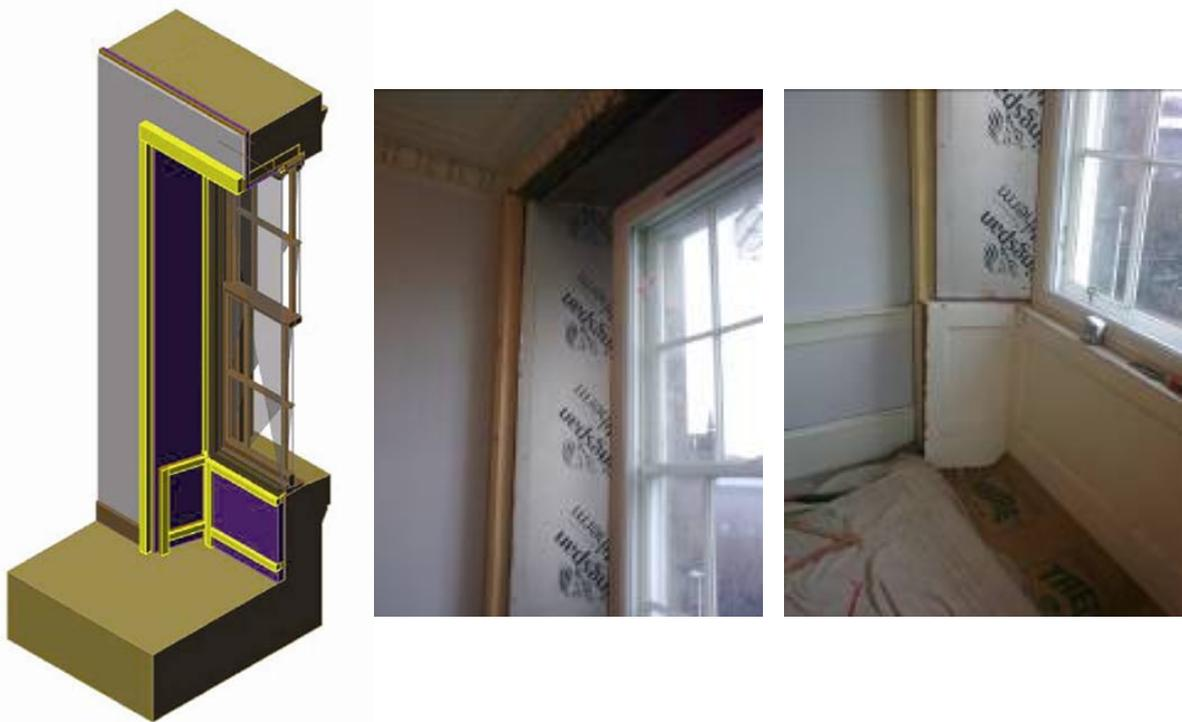
Fig. 22. Diagram and photographs showing insulation to shutter pockets
