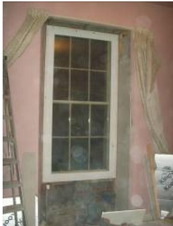
Fig. 6. Drawing and photograph showing new secondary glazing in position
