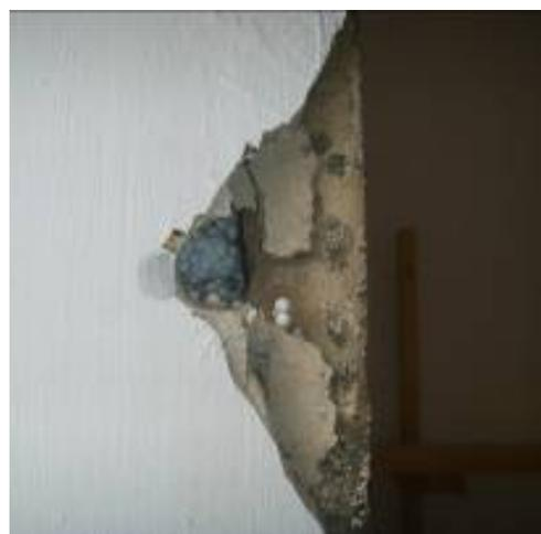
Fig. 21. Bonded bead being blown in behind plaster
