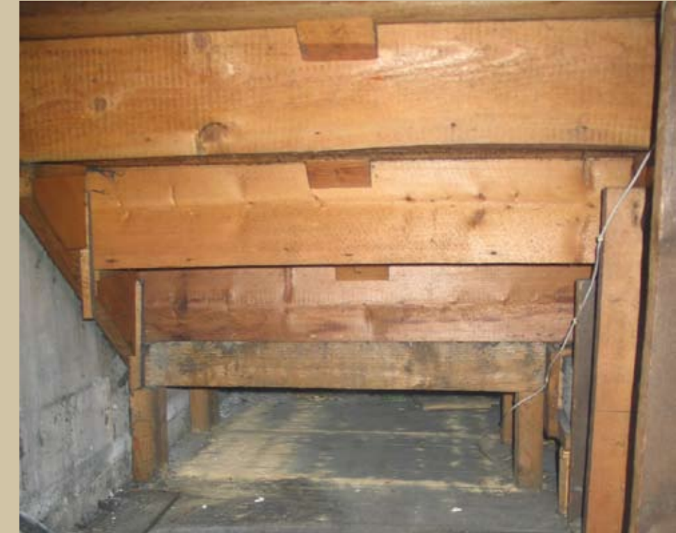
Re-fixed blocks holding tread and risers securely in place
