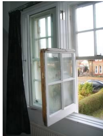
Fig. 3. Access to original windows for cleaning was maintained
