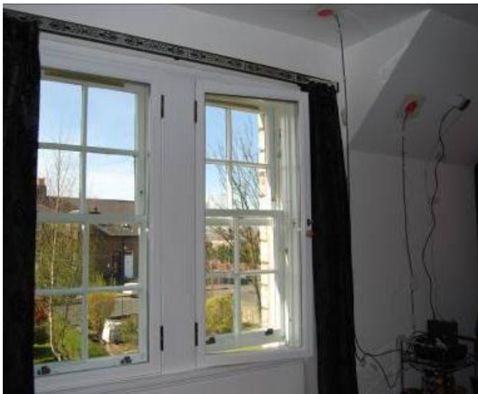
Fig. 2. The timber double-glazed secondary glazing. Testing equipment from Napier University also seen on right.
