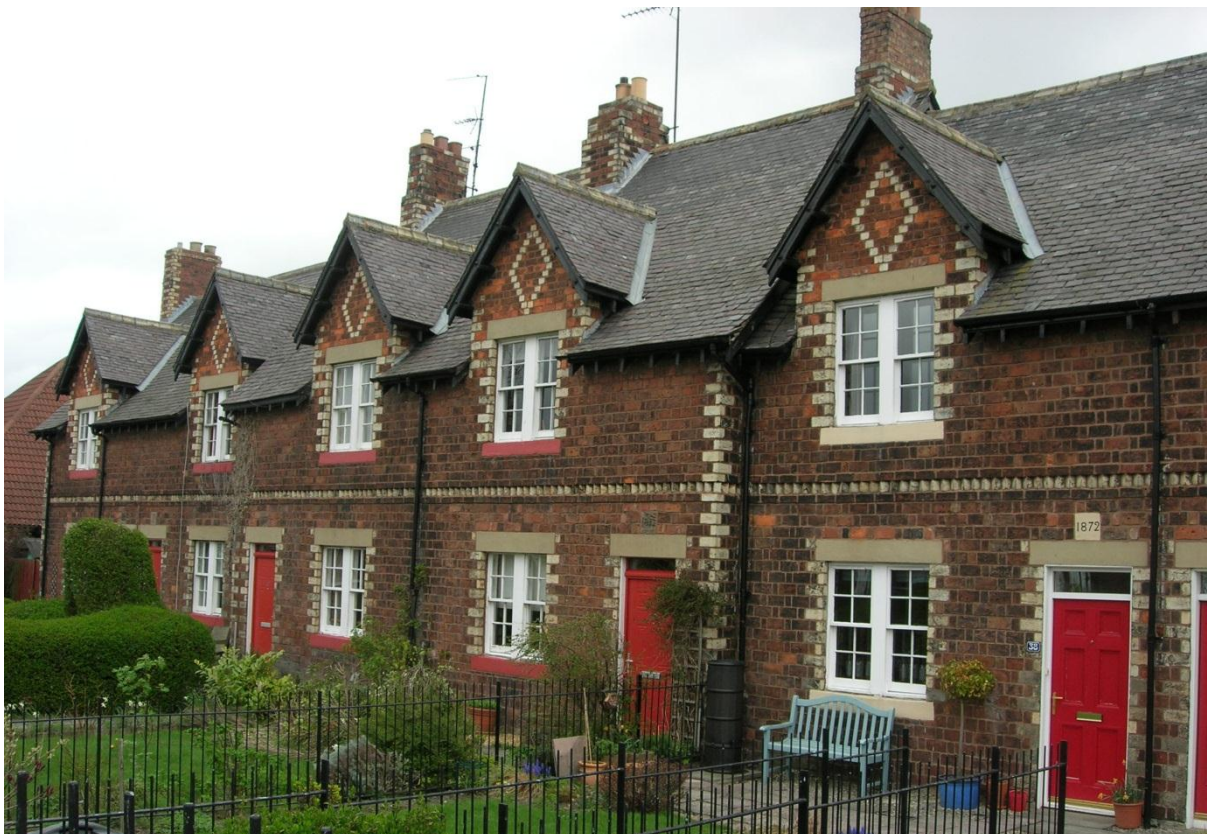
Fig. 1. Front elevation of Newtongrange Cottage
