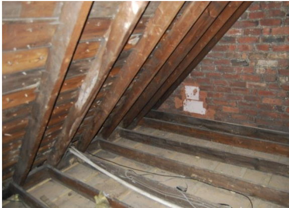
Fig. 5. Ceiling space prior to insertion of insulation
