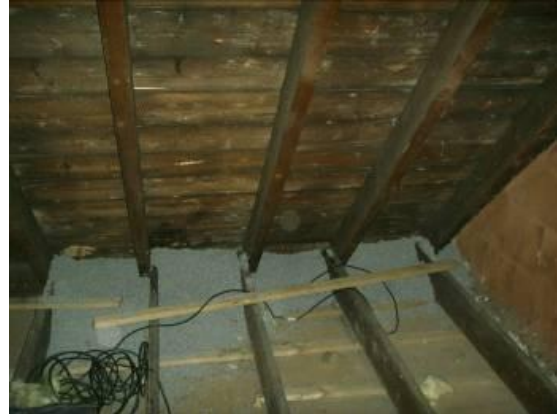
Fig. 6. The bonded bead insulation installed in the cooms
