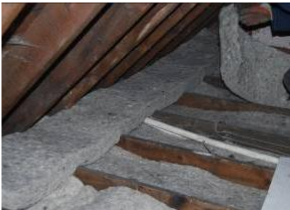
Fig. 7. Insulation between and over joists
