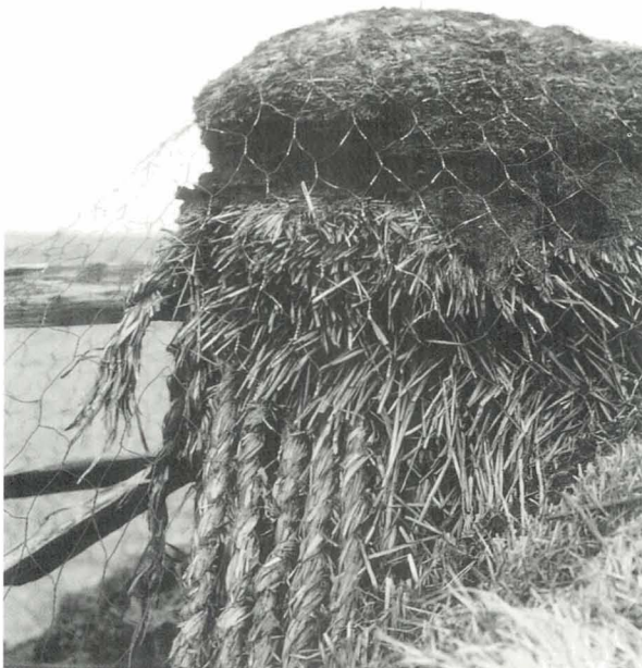
Straw over simmens held in place with chicken wire.
