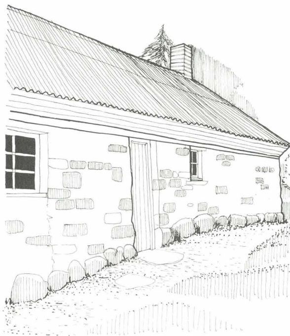
Thatch boxed-in under corrugated iron. Red Roofs, Liff, Angus (B.W.)
