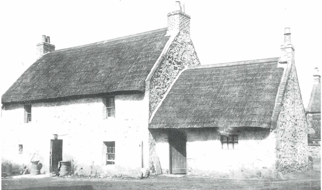
Corstorphine, Midlothian c1900. A cereal or reed thatch on a well-built two storey building. The horizontal lines across the roof are formed by raip and scob fixing. (National Museums of Scotland)
