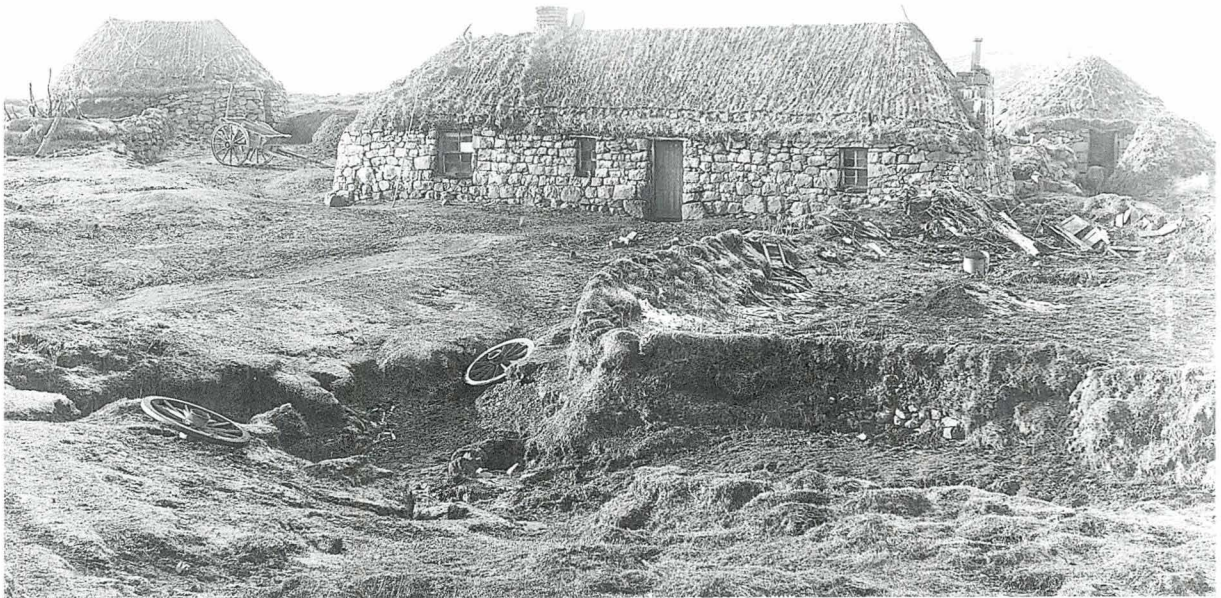
A Skye crofters' home. A thatch of cereal straw, bent or rush, roped and weighted with stones. (G.W.W. Aberdeen University Library C7409)
