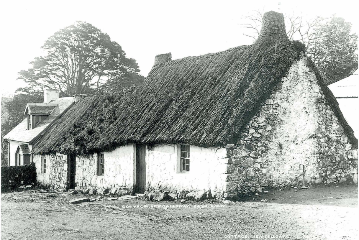
A cottage, New Galloway, Dumfries and Galloway. The dark colour and coarse texture suggest this might be a broom thatch. Note the rolled skewes, roped chimney heads and scob and wand fixings at the ridge. (G.W.W. Aberdeen University Library E1509)
