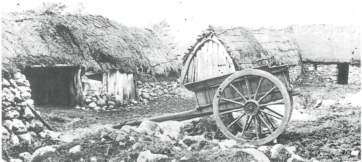
A Highland Steading, Kinlochewe, Wester Ross. A range of thatch types are shown. On the right the main farm house uses a method of secret fixing, the range to its left is secured using timber wands. The cart shed to the left of the photograph may have a deteriorating cereal or rush thatch although there are indications that turves or clay may be exposed at the surface. (G.W.W. Aberdeen University Library 0748)
