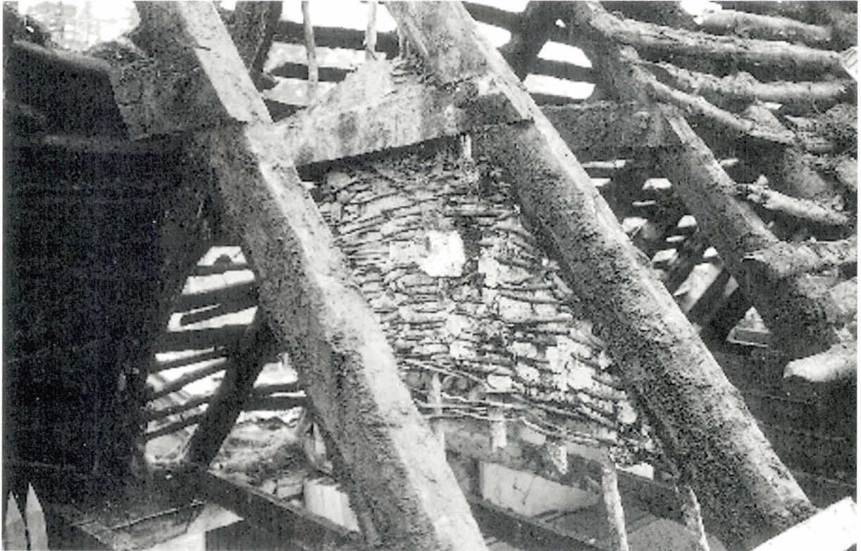
Johan Cottage, roof timbers and wattle panelling. (S.Whyment)
