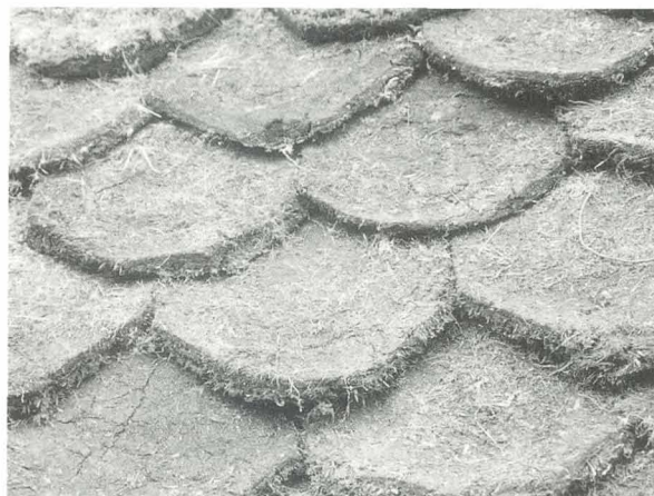
Overlapping basal turves, Luib, Skye. (B.W.)
