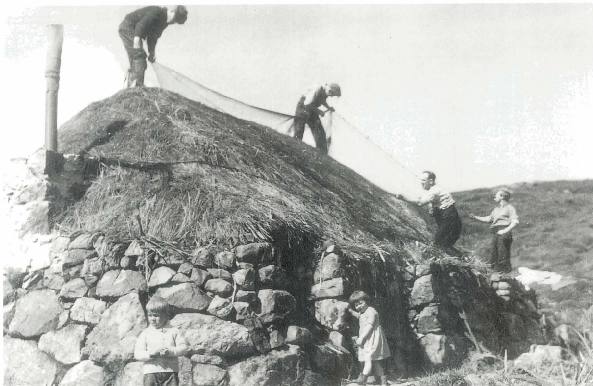
Netting and roping a thatch of cereal or bent on the Uists. (National Museums of Scotland C7684)
