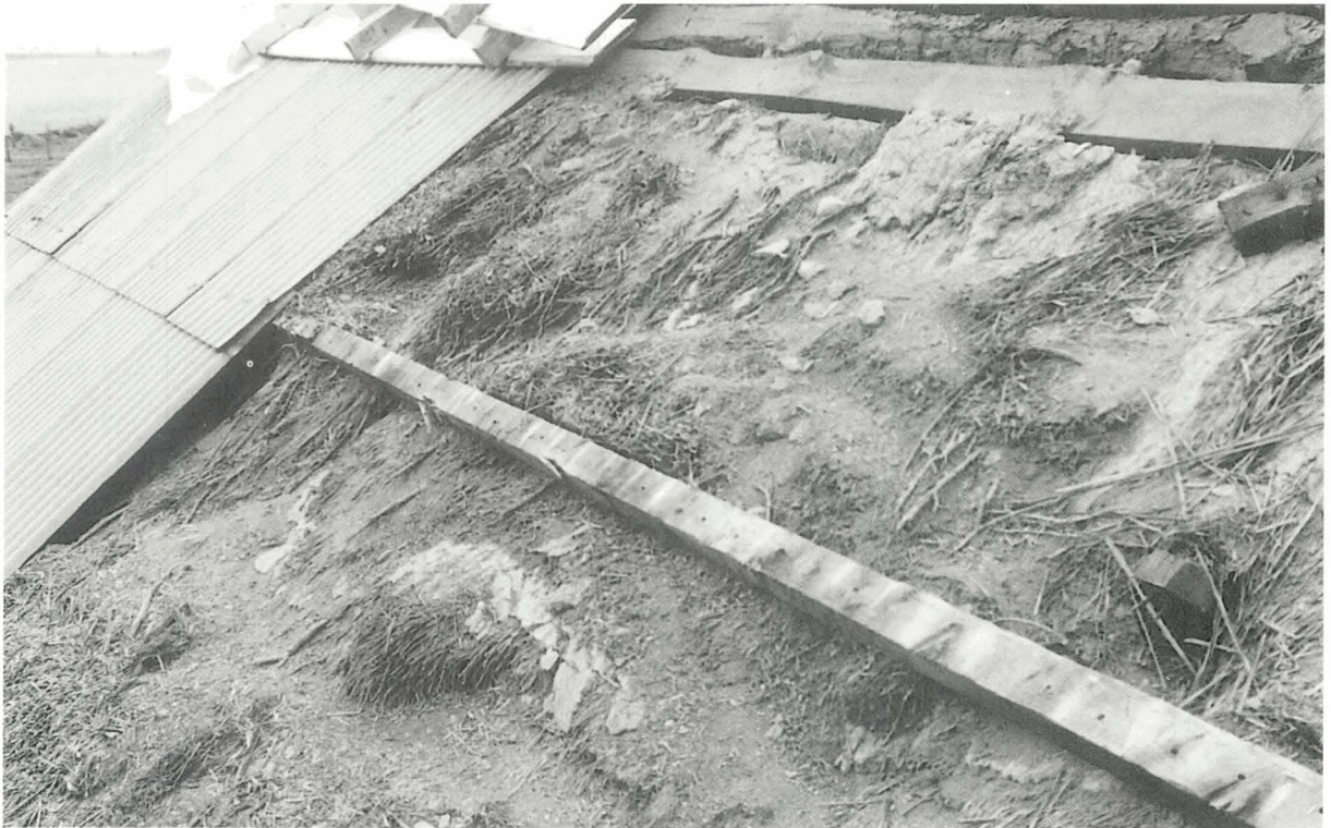
The eroded surface of clay, straw and broom. (T.H.)
