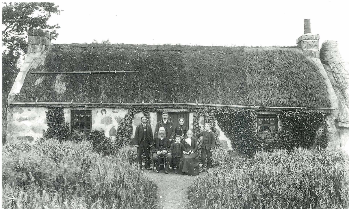
Ardoyne, Aberdeenshire. Possibly a broom thatch held down by chicken wire with a turf ridge. Note the rolled skew and roped chimney and fixings on the older house to the right. (National Museums of Scotland C5041)
