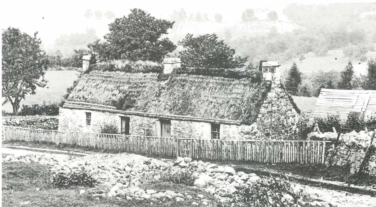
Pitlochry, Perthshire. Possible bracken thatch with turf ridge and skews. The eaves are secured with crook and caber fixings. Note also the false chimney heads with timber lums against them. (G.W.W. Aberdeen University Library)
