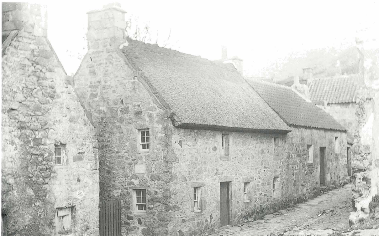
Michael Bruce's Cottage, Kinnesswood, Loch Leven. Probably one of the earliest reed thatches in the area. The reed would have been stitched to the roof and the gable capped with turf. This commonly used roofing style superseded earlier cereal thatches in many east coast towns. Most have now been replaced with pantiles (G.W.W. Aberdeen University Library F5351)
