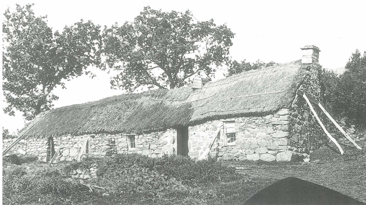
Mrs Ferguson's Inn, Bridge of Turk, Perthshire. These buildings show cereal or rush thatches in different states of repair. Scobed timber wands have been used to fix parts of the roof and stitched timber wands as fixings at the apex. (G.W.W. Aberdeen University Library F2883)
