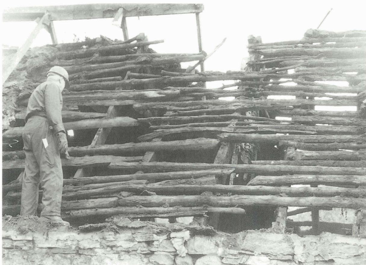
Johan Cottage, roof timbers following the removal of the thatch. (S.Whyman)
