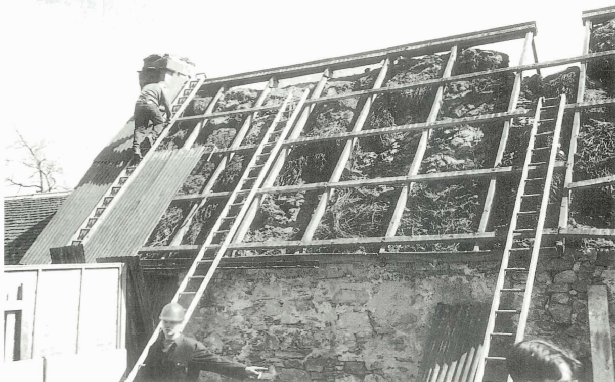
Johan Cottage, view of the north face of the roof. (S.Whyman)
