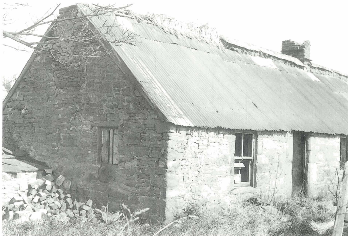
Thatch is often preserved under corrugated iron or other sheet materials. In this case the thatch was of reed. Murroes, Angus. (B.W.)
