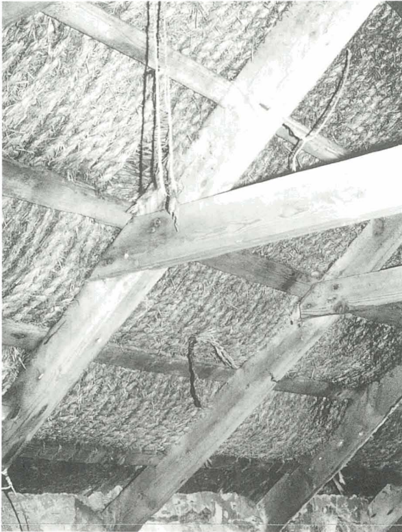
Gears, Orkney 1996. A needle thatched roof from the inside.
