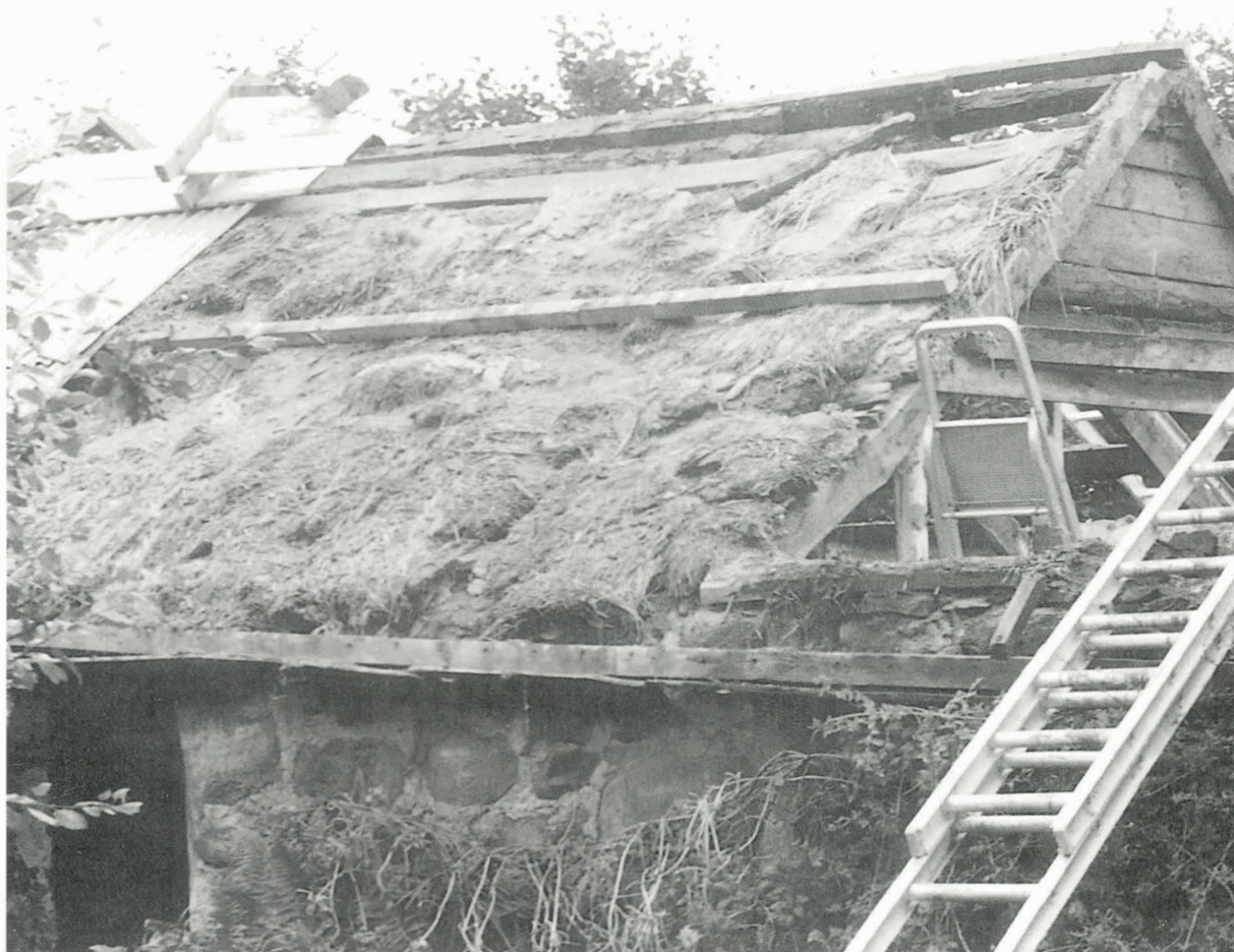
Corse Croft, Huntly, Aberdeenshire after removal of the sheet metal. (T.H.)
