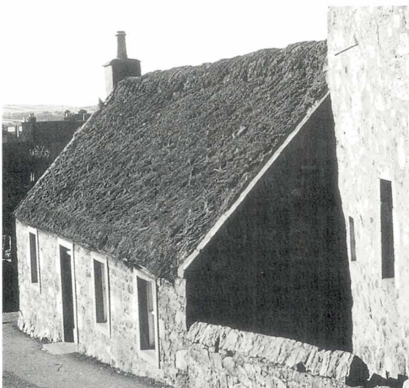
Auchtermuchty, Fife. This roof consisted of a basal turf layer originally with an oat straw thatch. At a later stage short layers of reed were driven through the oat straw. The ridge was capped with a mudwall mix and turf. Before (1974) and after (1980) renovation (B.W.)
