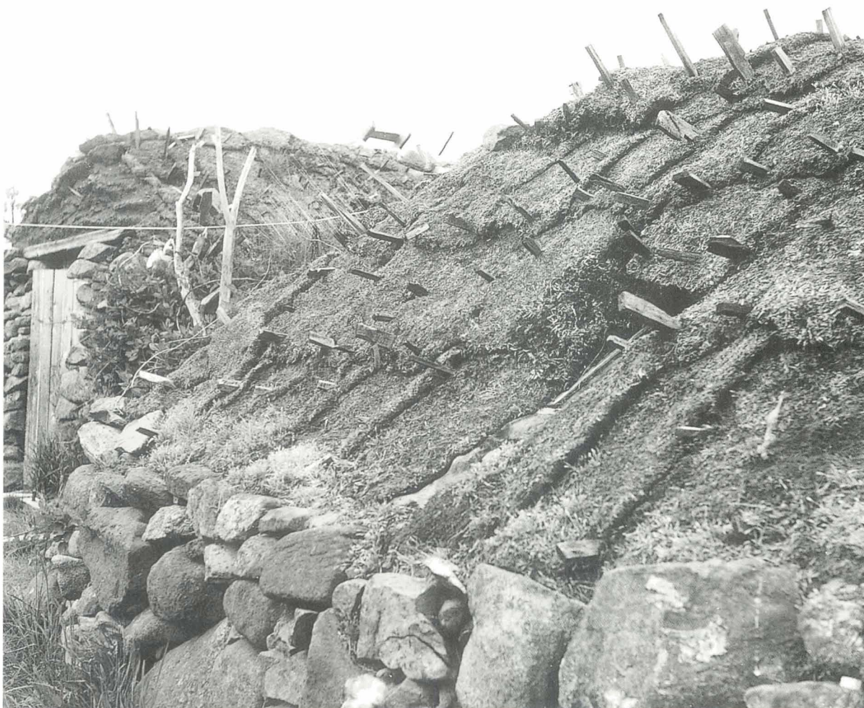
The bull's house on a Muckle Row croft, Orkney. Roof turves retained with wooden pins –1962. (Orkney Library)
