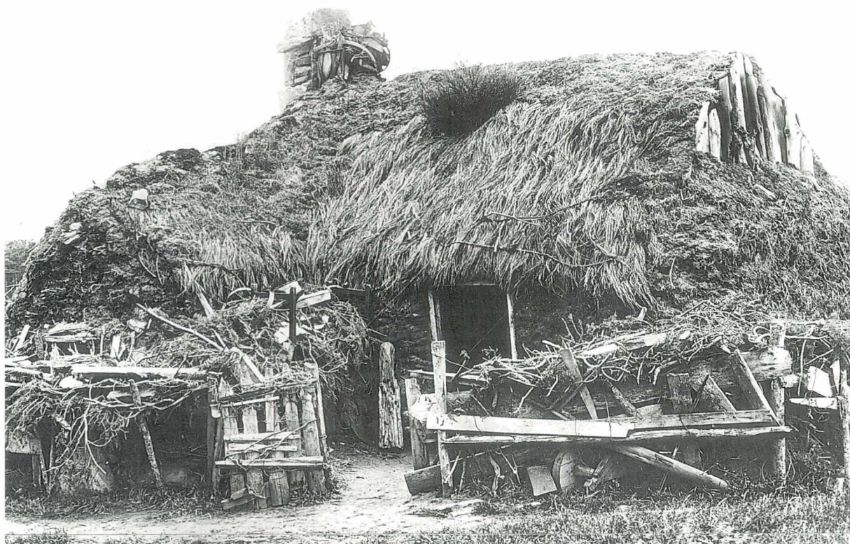
Annie Shaw's Castle, Nairn. This building has been repaired many times. Broom would appear to have been used to fix the roof. (G.W.W. Aberdeen University Library C1184)
