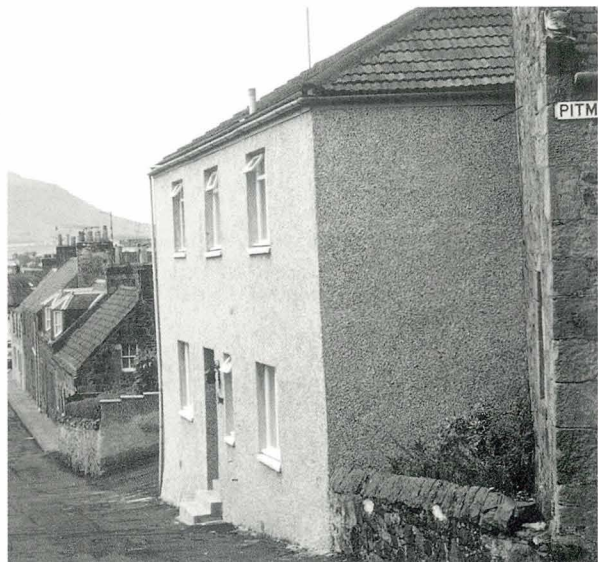
Auchtermuchty, Fife. This roof consisted of a basal turf layer originally with an oat straw thatch. At a later stage short layers of reed were driven through the oat straw. The ridge was capped with a mudwall mix and turf. Before (1974) and after (1980) renovation (B.W.)
