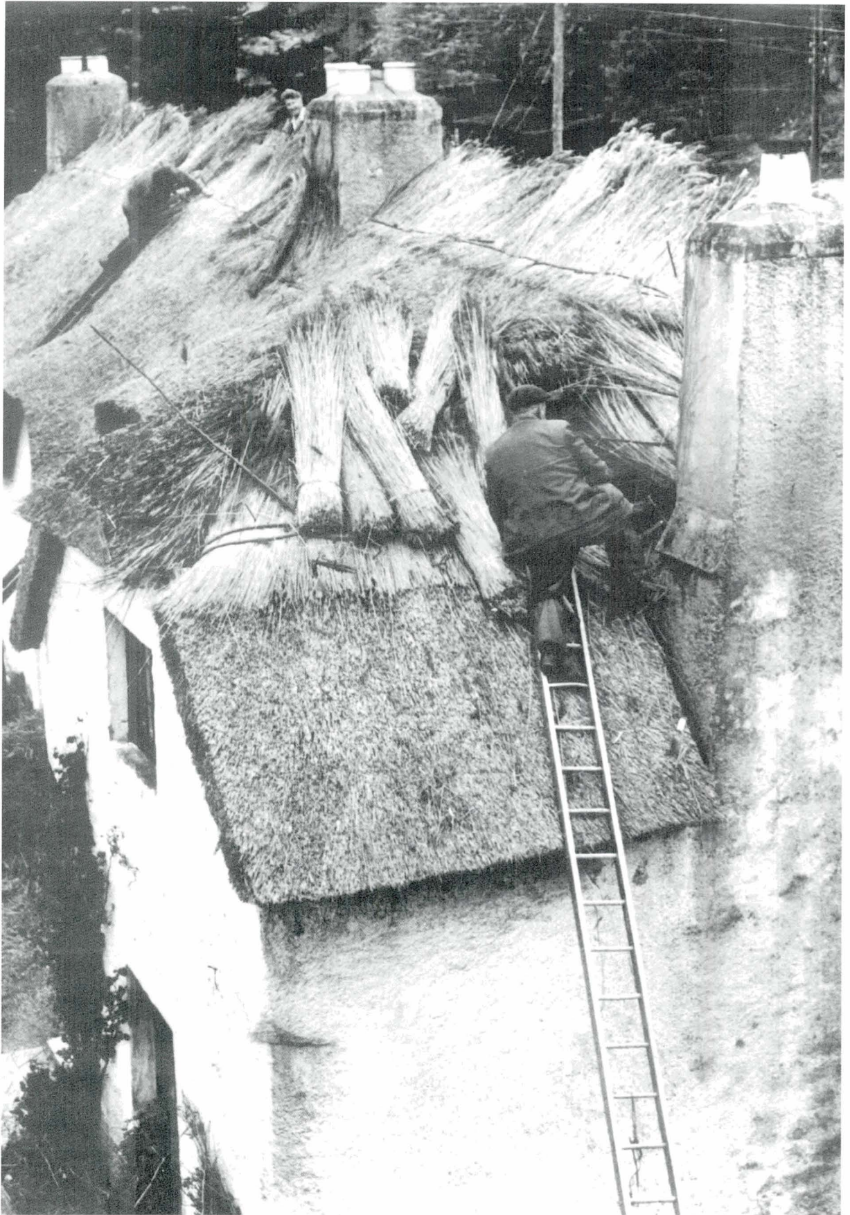
Balnald Cottages, Fortingall, Perthshire. Re-thatching with reeds. (Dundee Courier)
