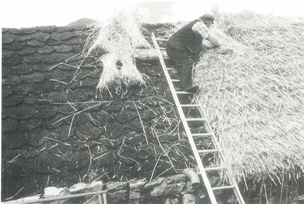
Cereal thatch over turf – Duncan Matherson, Luib, Skye. (B.W.)
