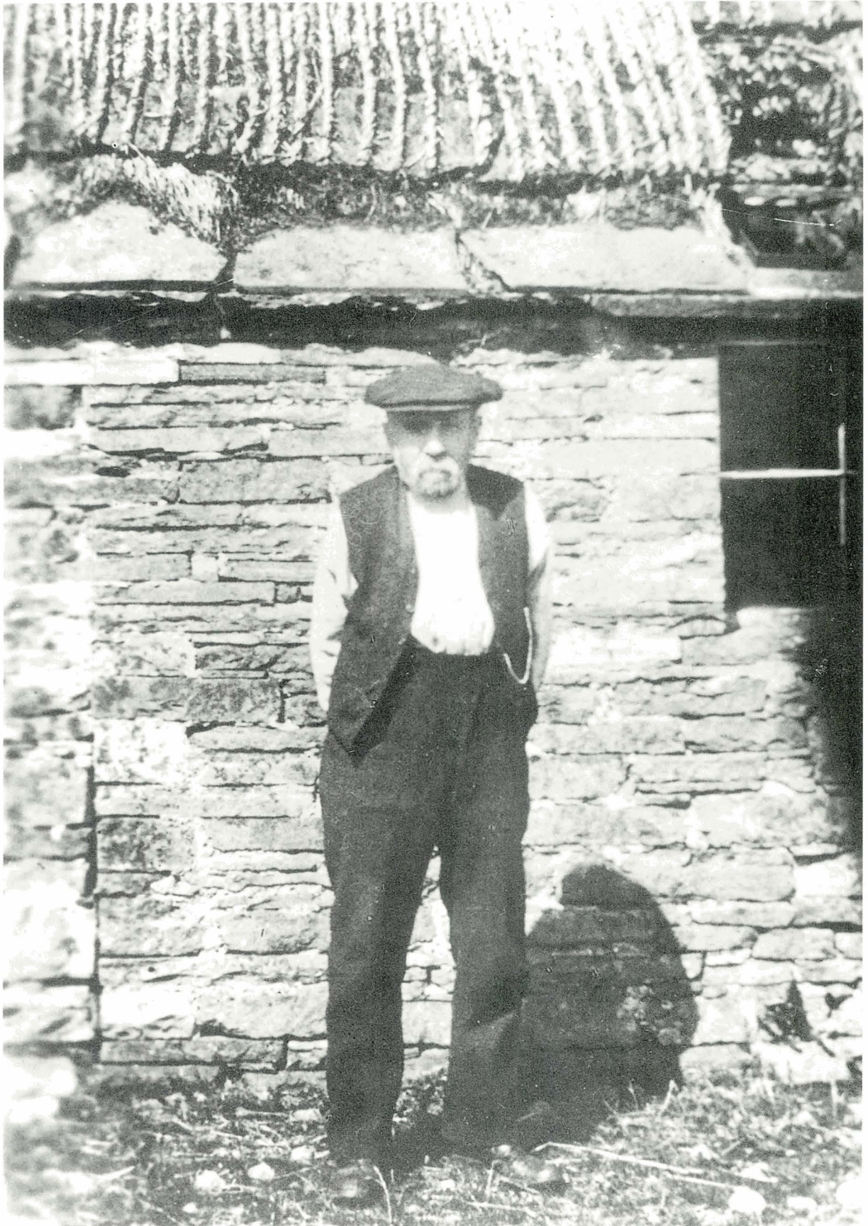
A needle thatch from Faray, Orkney. Note the Orkney flagstone at the eaves and the rooflight over the window. (National Museums of Scotland C8332).
