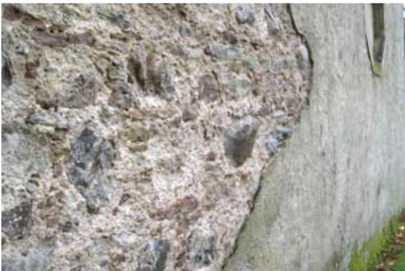
*Illus 3.13 Typical failure of hard cement render on a soft mortar rubble wall. (Photo: D Urquhart).*
