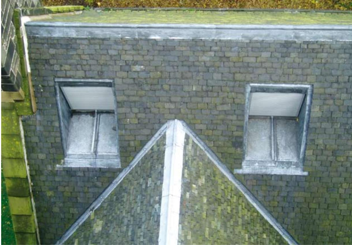
*Illus 3.14.5 Inset dormer vents on a traditional pitched slated roof. Inset dormer vents eliminate the need for large, intrusive ventilation grills.*
