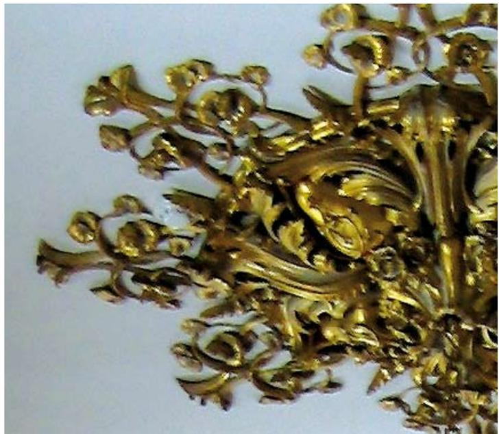
*Illus 2.11.2 Very discreet smoke detector set into historic ceiling. The detector head is located to the left of the ceiling rose (Photo: I Gough).*
