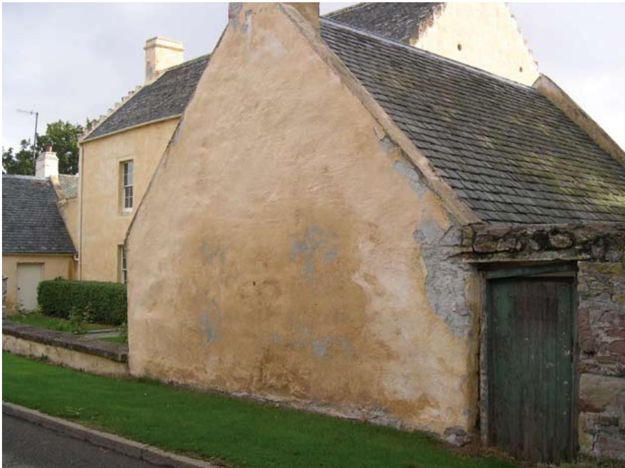
*Illus 3.12(a) Recent lime coating showing exceptionally high moisture loading in the wall due to water penetration at roof level and to moisture from the ground. (Photo: D Urquhart).*
