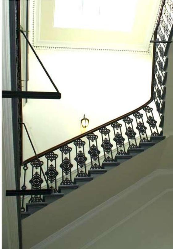
*Illus 1.1.11 Fine example of cantilevered stone staircase in this former hospital converted to offices. Note the slenderness of the self-supporting stone steps and the original iron balustrade. (Photo: Historic Scotland).*
