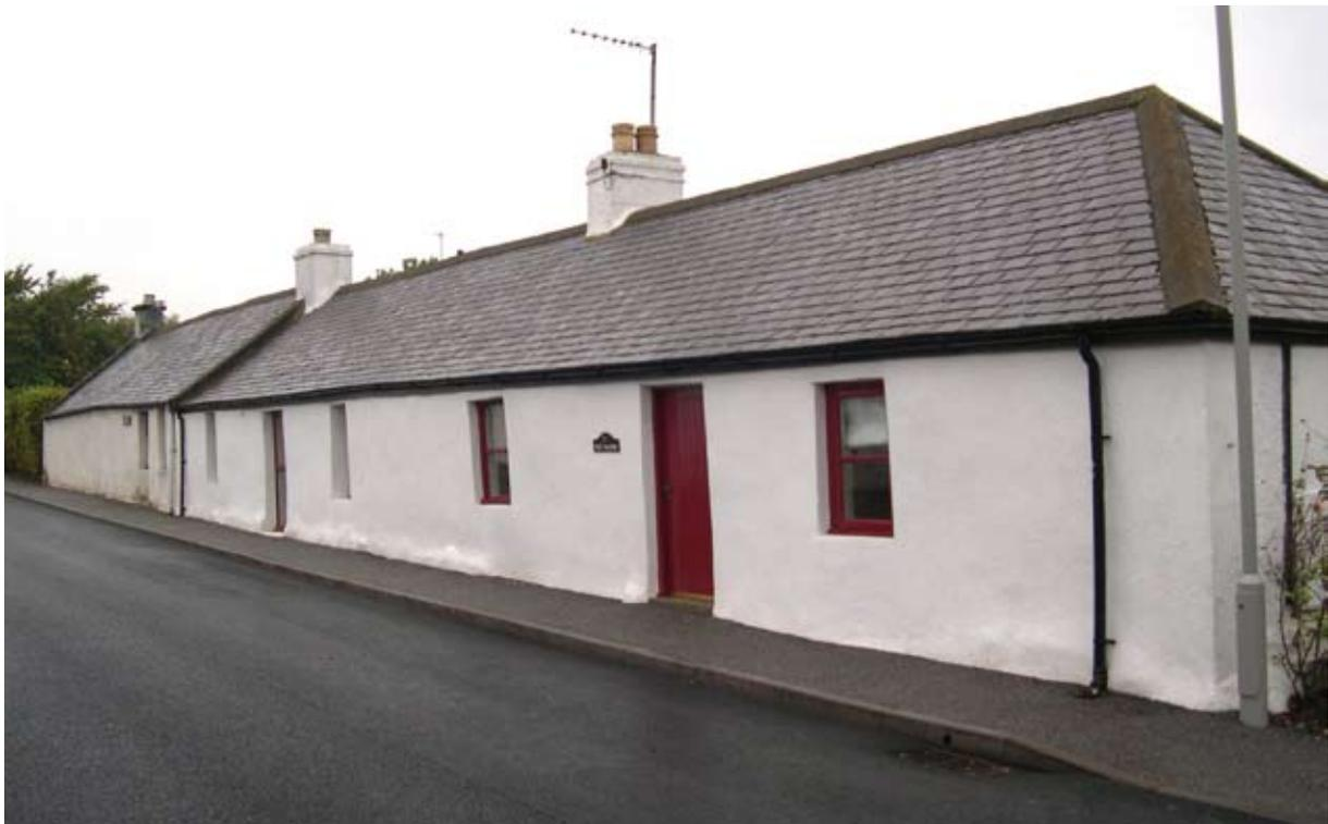
*Illus 3.3 Clay and bool cottages (C(S) Listed), Morayshire. Unfortunately, now rendered with a hard cement mortar Note: boulder base course and modern slated roof, which replaces the original traditional 'clay thatch'. (Photo: D Urquhart).*
