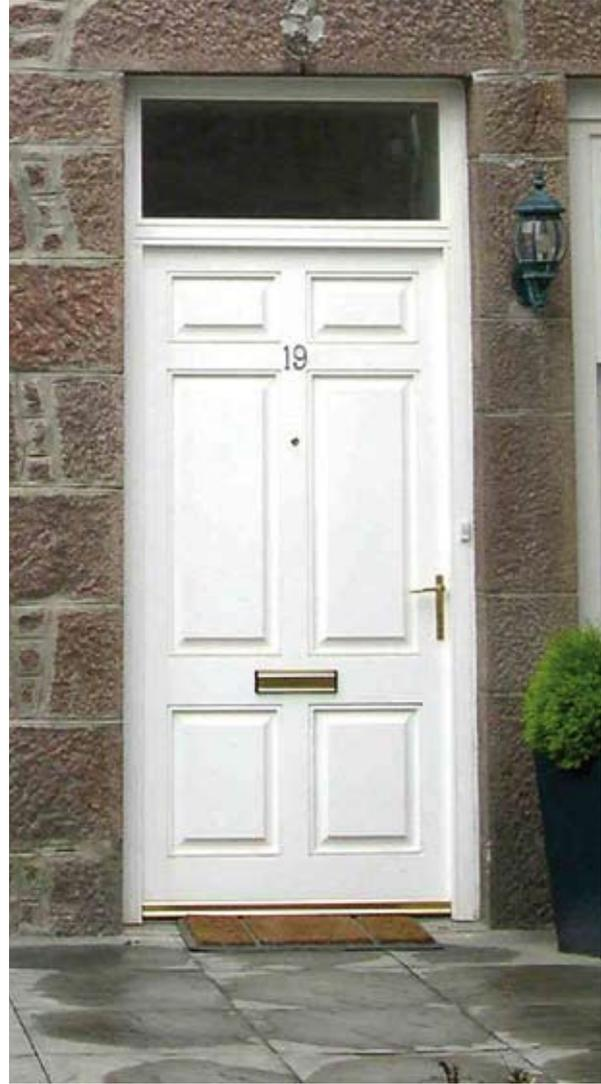
*Illus 3.16(b) The door on the right is an acceptable modern timber door in a building (circa 1904) converted to apartments and replaces a door that was not original to the building (Photo: D Urquhart).*
