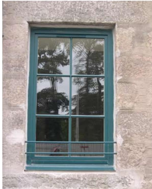
*Illus 3.16.1 New window frame fixed into resized opening in this former mill converted to apartments. Note the rather poorly executed mortar pointing around the repositioned stone sill.*
