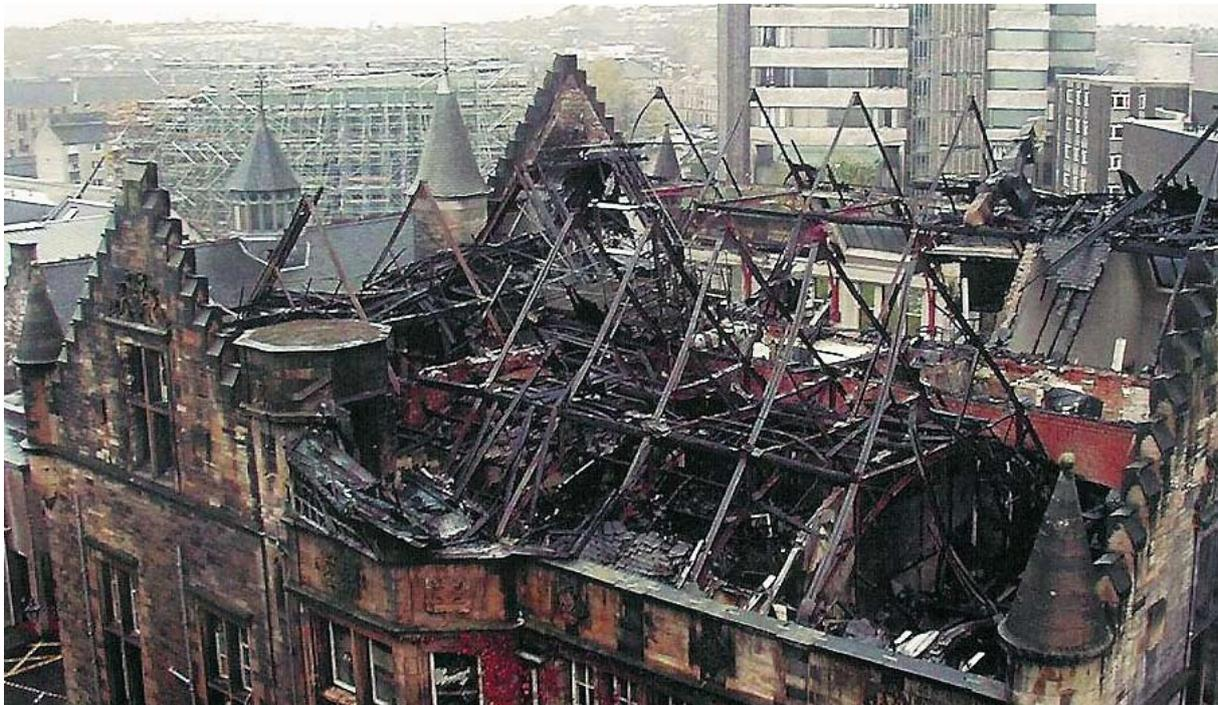
*Illus 2.4.1 The presence of large, unpartitioned roof voids has resulted in severe fire damage to the roof and interior of this Category A listed university building. (Picture by Leigh Johnston, Historic Scotland and reproduced here from TAN 28).*
