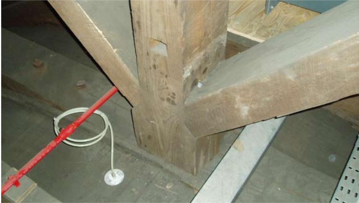
*Illus 2.11.1 Installation of an aspirating smoke detector system in a ceiling void. Shown is the main plastic air pipe with an 8mm diameter tube from it to go through an 8mm hole in the roof boarding (Photo: S Brown).*
