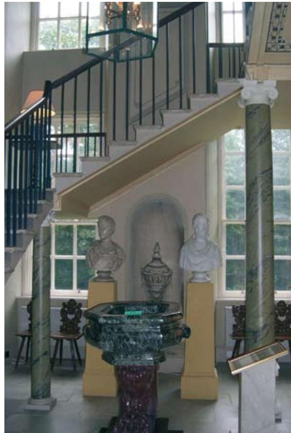
*Illus 5.1 Structural support for this stair in Duff House would be difficult to determine using current design criteria (Photo: D Urquhart).*
