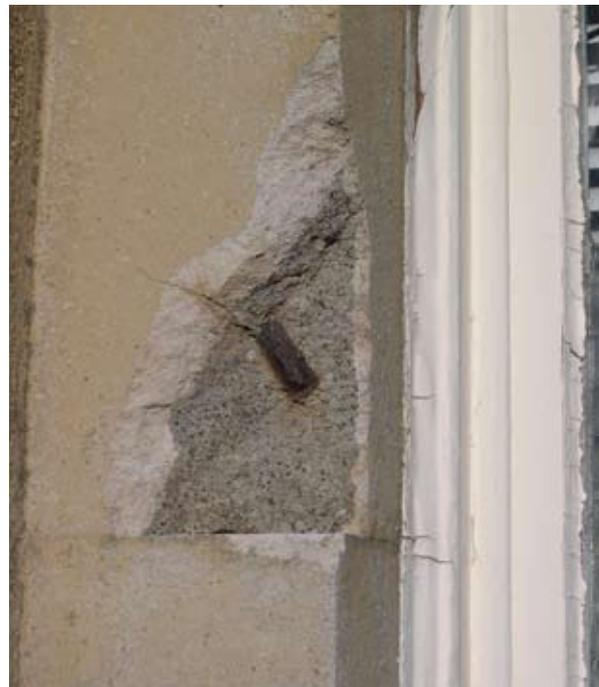
*Illus 2.2 Sandstone façade repaired with precast concrete synthetic stone instead of matching stone indents. Corrosion of steel reinforcement has caused spalling of the block. (Photo: D Urquhart).*
