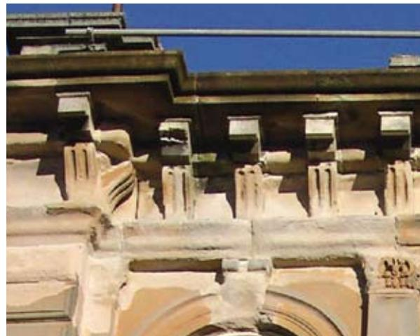
*Illus 2.3. An example of inappropriate replacement elements is illustrated on this B listed building. Stone brackets supporting the stone cornice have been replaced with reinforced precast concrete brackets. The reinforcement is corroding creating a risk of falling masonry. An original stone balustrade supported on the cornice has been removed. (Photo: D Urquhart).*
