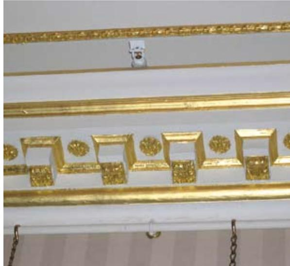
*Figure 2.15.2 Sidewall sprinkler head above a cornice in Duff House. (Photo: D Urquhart).*
