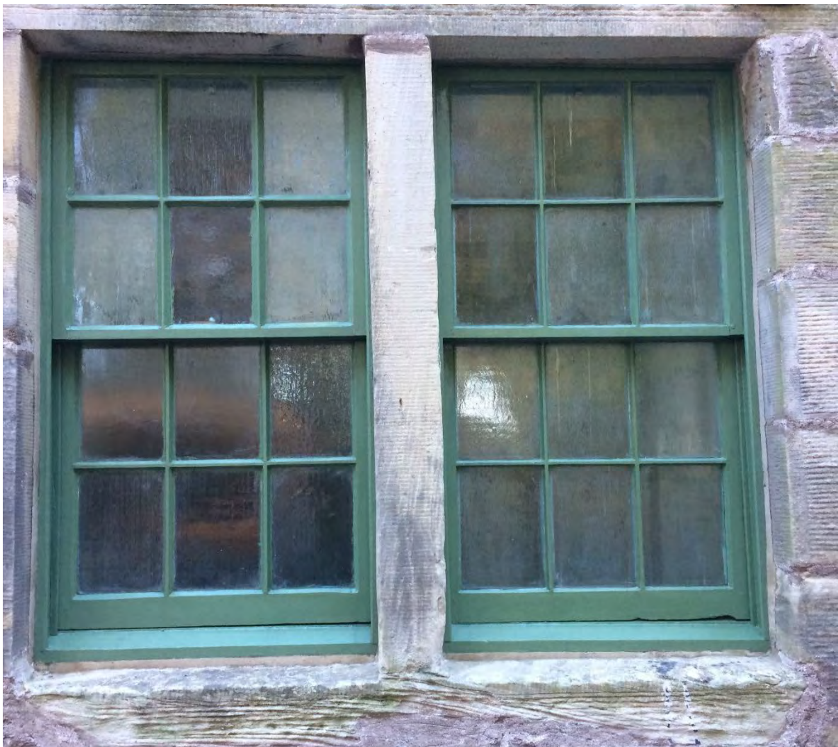
Figure 9. The lower windows of the stable block windows painted with linseed oil paint.
