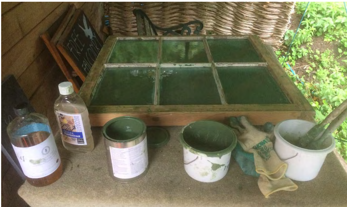
Figure 8. The sash removed ready for painting with the linseed oil paint. All previous layers of paint had been removed down to bare wood.
