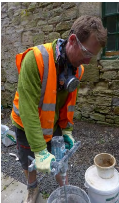
Figure 4. Trial mixes being prepared using a hand-held mixer.
