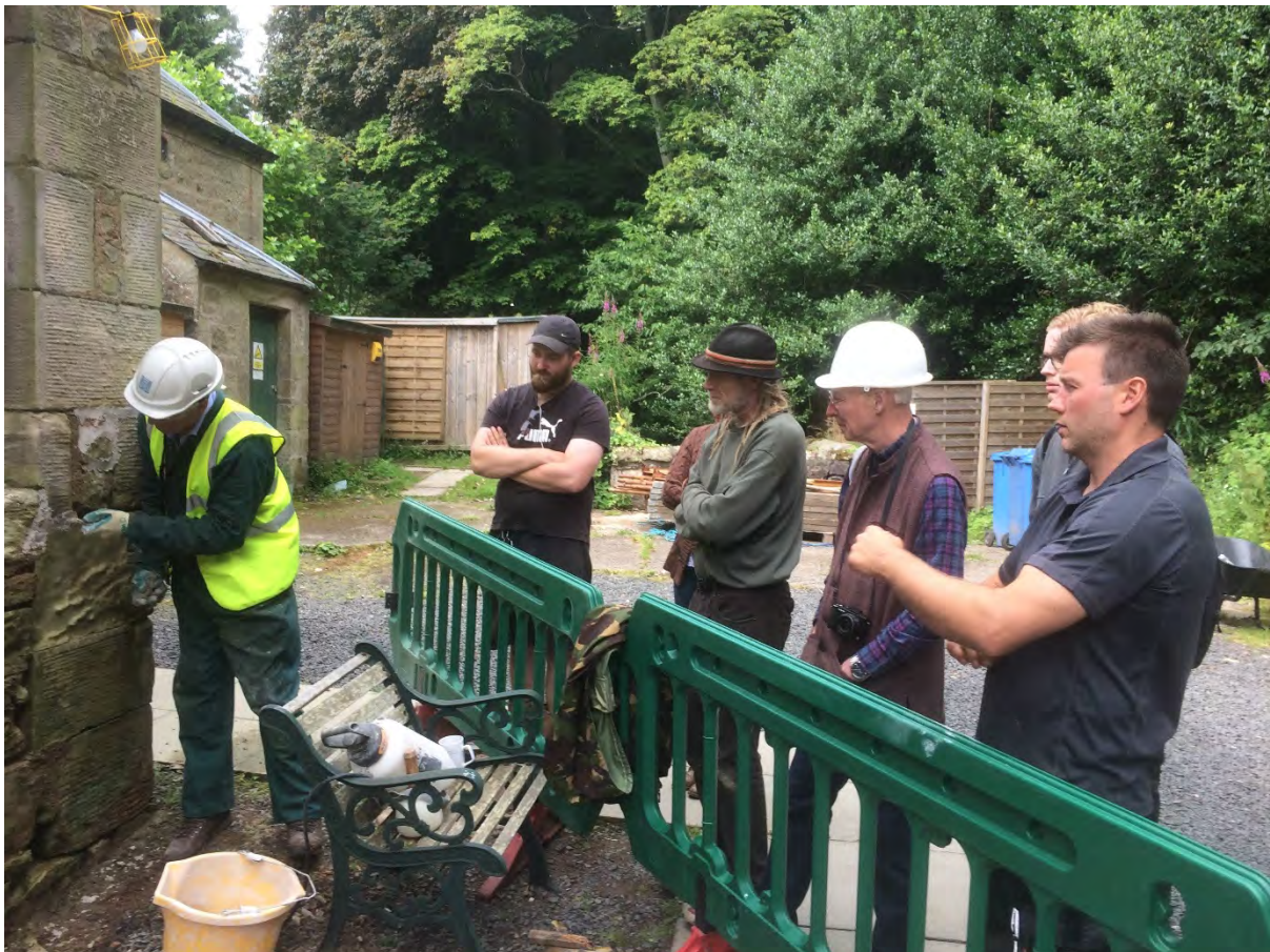
Figure 10. Pointing demonstration during the half-day training session at the start of the project.
