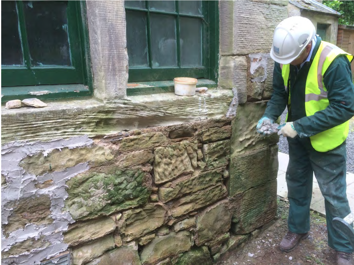
Figure 6. Re-pointing the wall with hot-mixed lime mortar.
