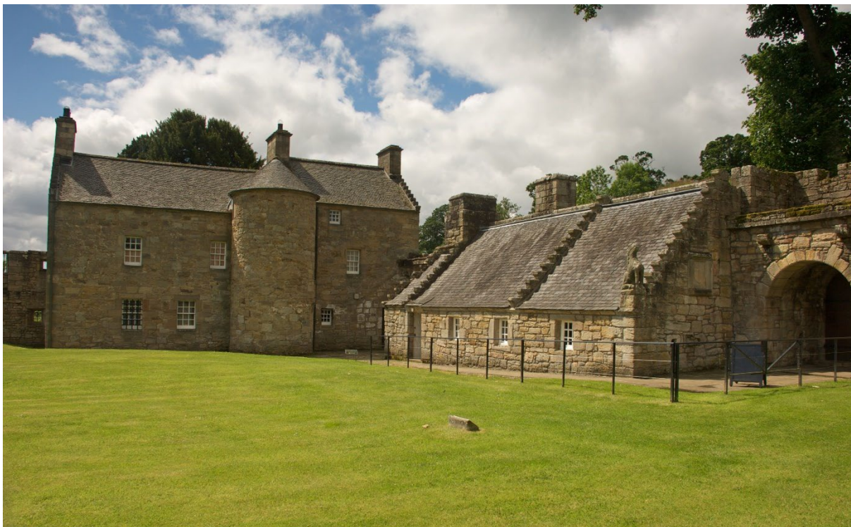
Figure 4: View of 'Andrew Hay's House', offices and gateway, in the south-west corner of the outer court. © Crown Copyright HES.
