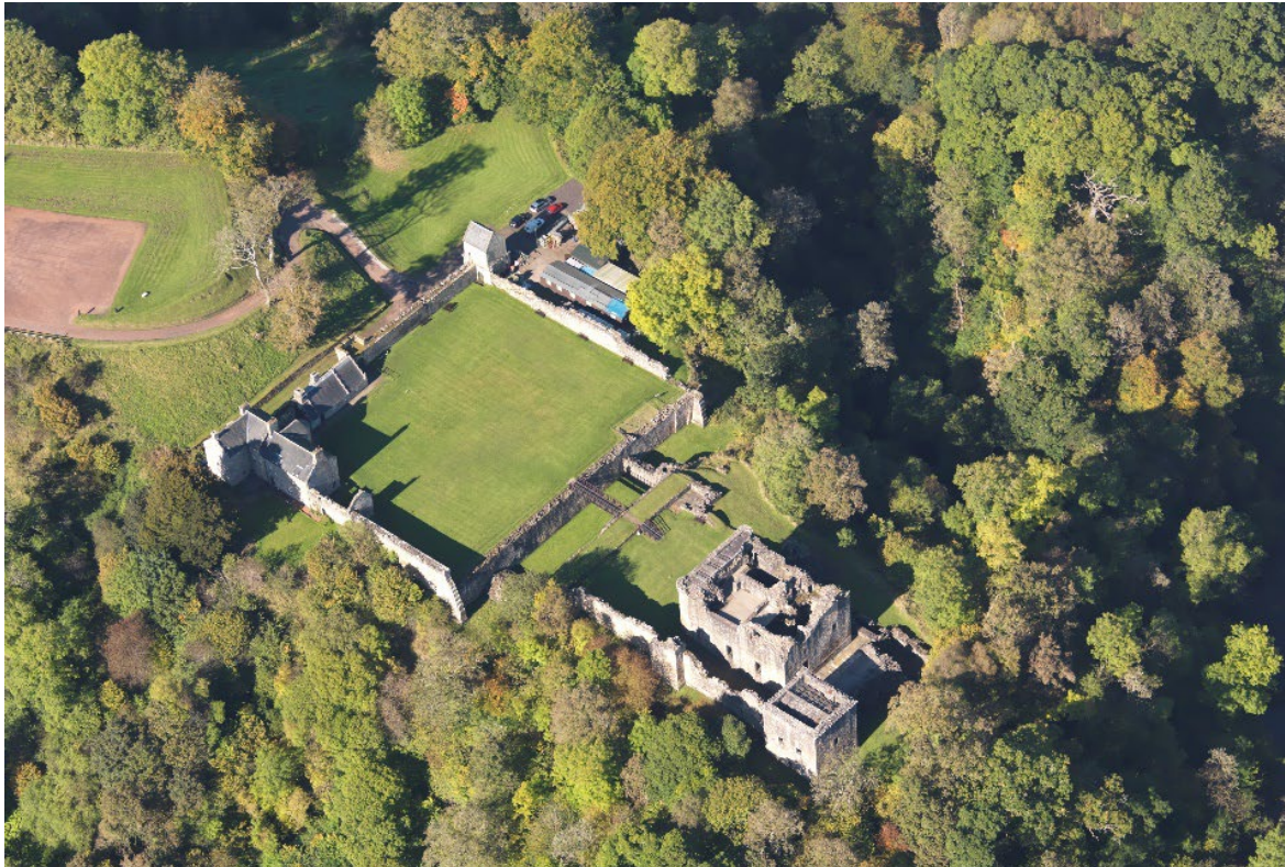
Figure 2: Oblique aerial view of Cragneithan Castle, taken from the south-east. Note steep path leading down from visitor car park. © Crown Copyright: HES.
