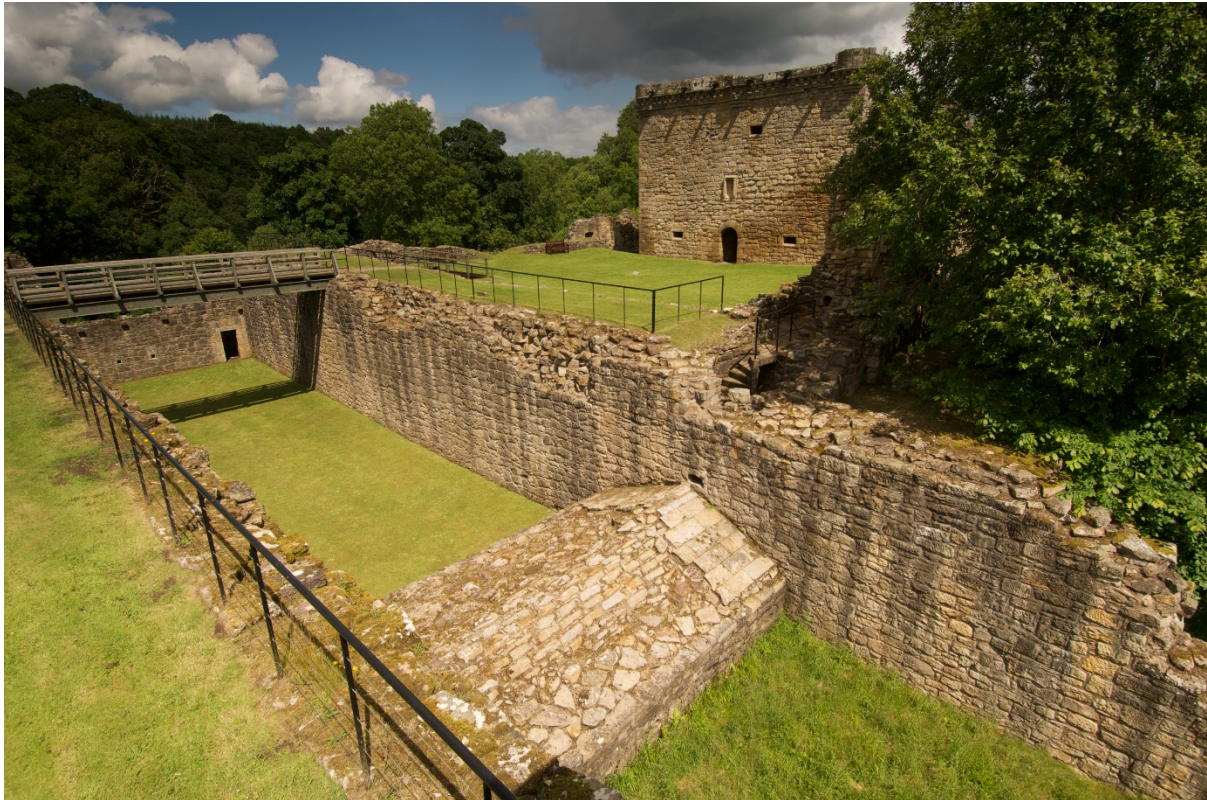
Figure 3: View of the caponier within the stone-faced ditch. © Crown Copyright HES.
