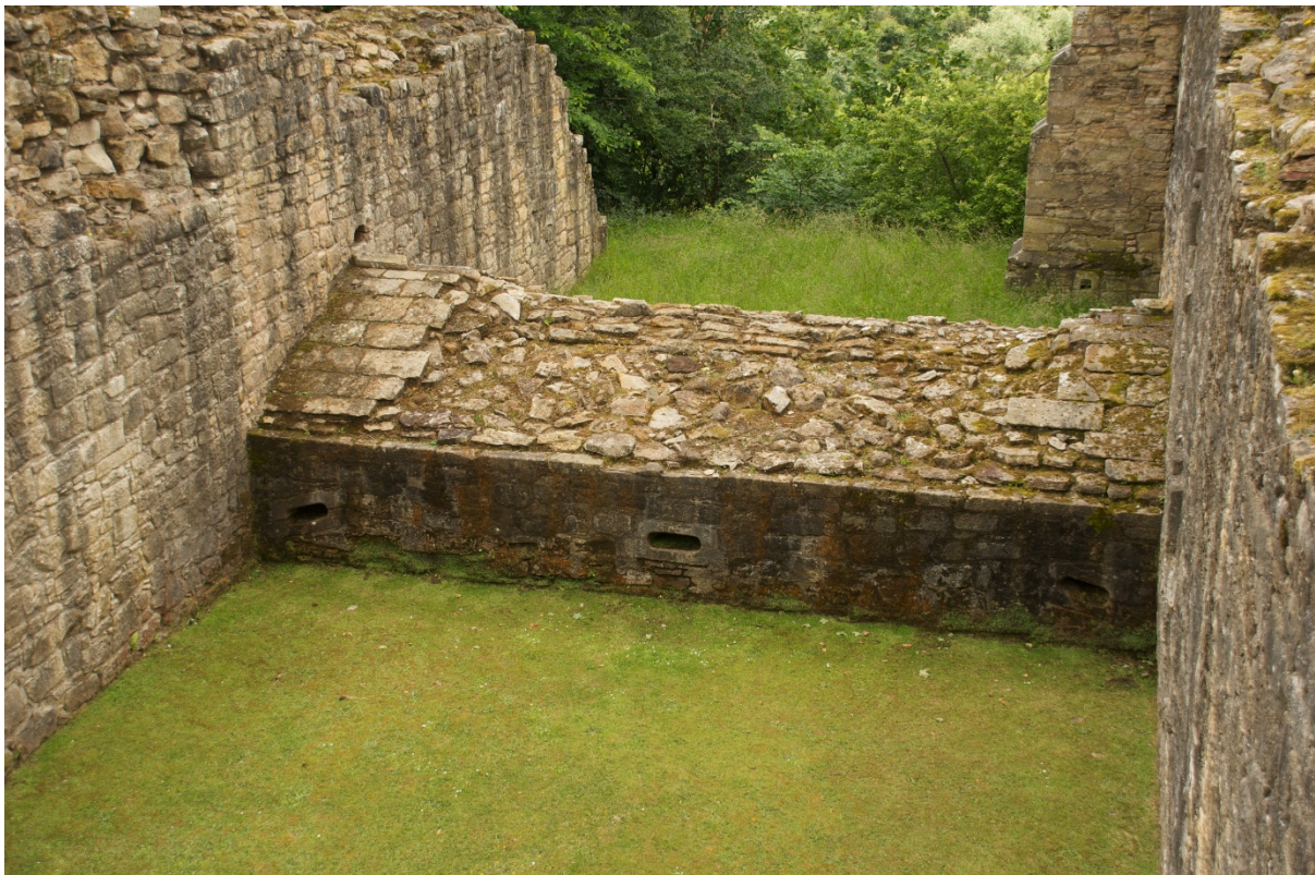
Figure 6: View of the well-preserved caponier. © Crown Copyright HES.
