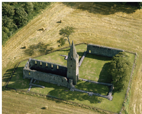
This was once a priory, but most of it has been reduced to foundations, apart from the church with its fine tower. © RCAHMS (John Dewar Collection) Licensor www.rcahms.gov.uk
