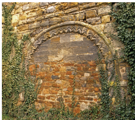
The fine chancel arch in the ruined Gullane Parish Church. The church was built in the 12th century and some Norman features still survive today. This arch would have been blocked up during later alterations. © Crown Copyright: Historic Scotland, www.historicscotlandimages.gov.uk
