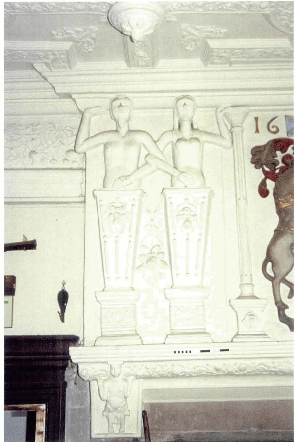
Illus 48. Muchalls Castle, Aberdeenshire; hand modelled figures used on either side of the coat of arms on this overmantel. © Crown copyright Historic Scotland
