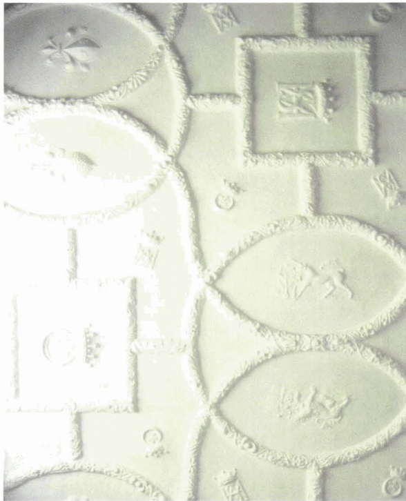
Illus 3. Pinkie House, East Lothian; possibly as early as 1613, the graceful design of this ceiling in the Green room is based on circles and curves, with delicate ribs entirely formed from cast floral enrichment without any underlying run mouldings. © Crown copyright Historic Scotland
