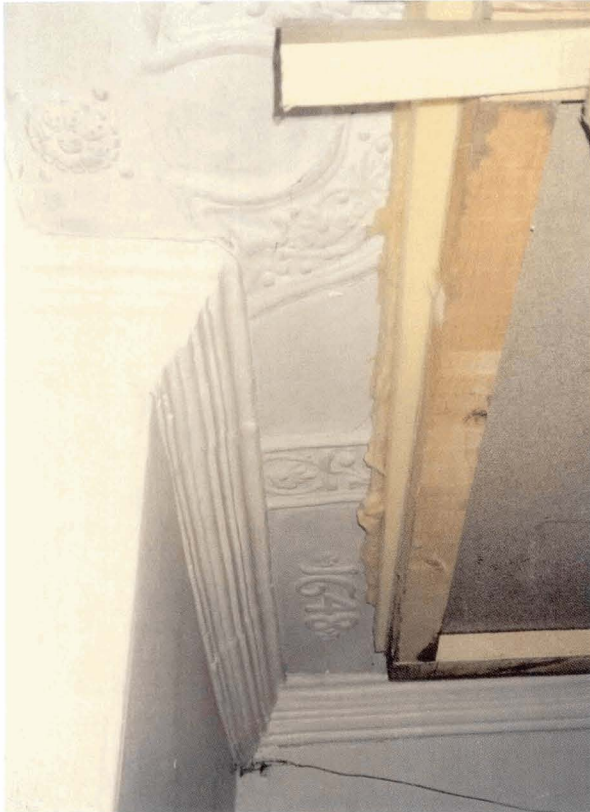
Illus 27. Supporting ceiling from below while repairs take place. © William McVey
