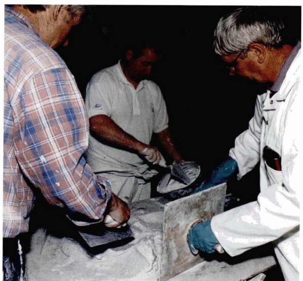
Illust 25. Mixing lime plaster for application. © Crown copyright Historic Scotland
