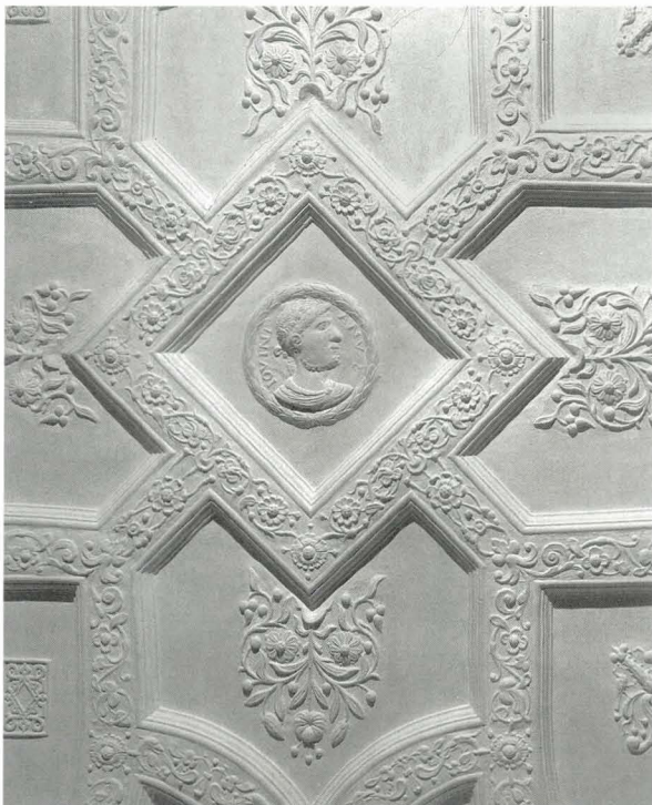
Illus 5. Craigievar Castle, Aberdeenshire; the Blue room ceiling dated 1626 again employs squares, some set diagonally and some set inside quatrefoils, with linking semi-circles. © Crown copyright RCAHMS
