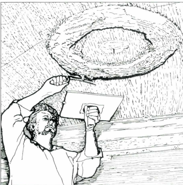
Illus 32. Building up coarse plaster as a base for a circular rib moulding run in-situ; note the central nail acting as a guide. © Crown copyright Historic Scotland/EA Whitfeld
