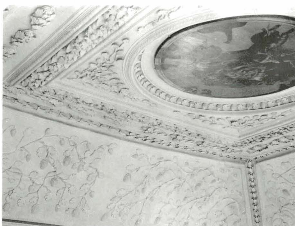
Illus 64. Kellie Castle, Fife (1676); the vine room illustrates changing ideas in plasterwork with its painted central panel and the free-flowing vine motif. © Crown copyright RCAHMS
