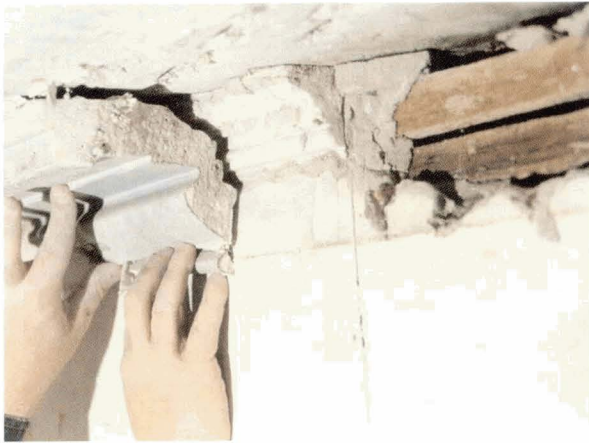
Illus 11. Sandgate, Ayr; there may be vital information hidden behind the plasterwork, as here, where there is an earlier (late C17 or early C18?) cornice behind the visible later one. © William McVey
