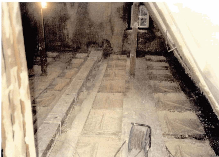
Illus 27. Supporting ceiling from below while repairs take place. © William McVey
