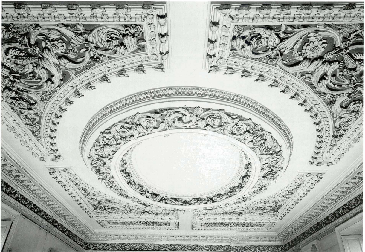
Illus 67. Bannockburn House, Stirlingshire (1680); a baroque style had established itself by this date, replacing the simpler plasterwork of the earlier C17. © Crown copyright RCAHMS
