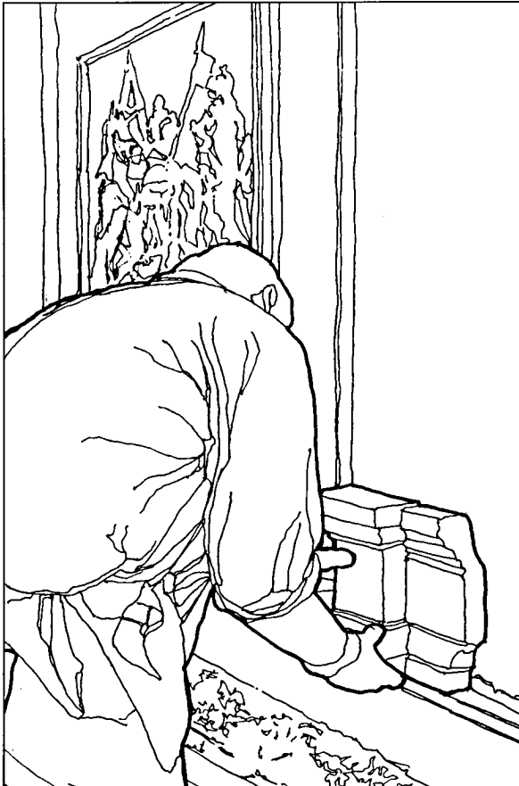
Illus 42. A decorative cast moulding being put into position (from scaffolding) on an overmantel. © Crown copyright Historic Scotland/EA Whitfeld
