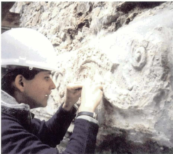
Illus 47. Huntly Castle, Aberdeenshire; this frieze is probably the earliest moulded plasterwork extant in Scotland, said to date from 1602-08. A Historic Scotland specialist consolidates this plaster which is now exposed to the weather. © Crown copyright Historic Scotland
