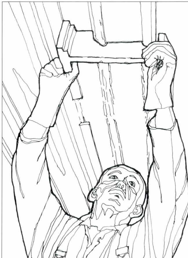
Illus 34. Running base coat for straight in-situ rib with muffled template mounted on a horse, using battens as edge guides. © Crown copyright Historic Scotland/EA Whitfeld
