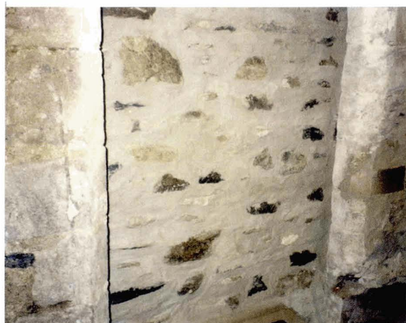
Illus 19. Dubbing out on a rubble stone background to provide a base for application of plaster. © Scottish Lime Centre
