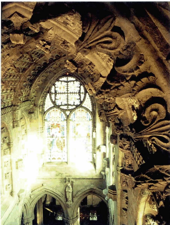
Illus 54. Roslin Chapel, Midlothian; stone bosses and pendants which almost certainly influenced the development of bosses and pendants in plasterwork. © Crown copyright Historic Scotland
