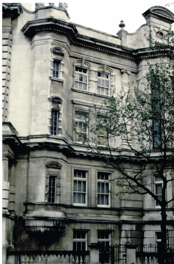
Illus 4. Typical soiling pattern on a limestone building façade. Soiling is heaviest in sheltered areas, unwashed by rainwater or run-off.
