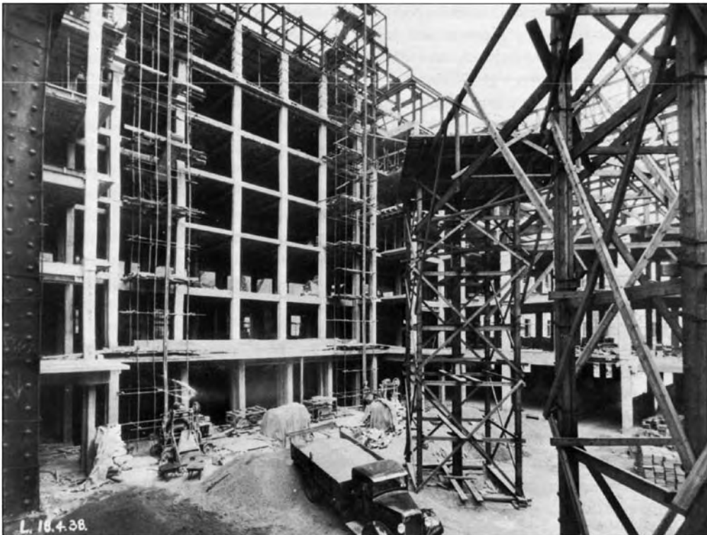
The south front of the main block from the court showing the steel frame being encased in concrete, April 1938.
