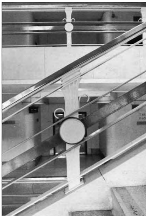
Detail of stair, with ironwork by Thomas Hadden.
