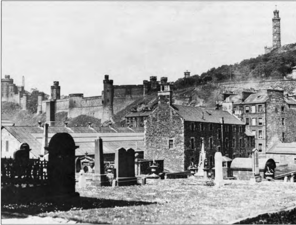
The Calton site from the SE in 1930: with the demolition of the prison blocks the curtain wall took on new qualities of the Picturesque.
