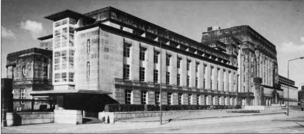
Regent Road frontage from the east, 1989.
