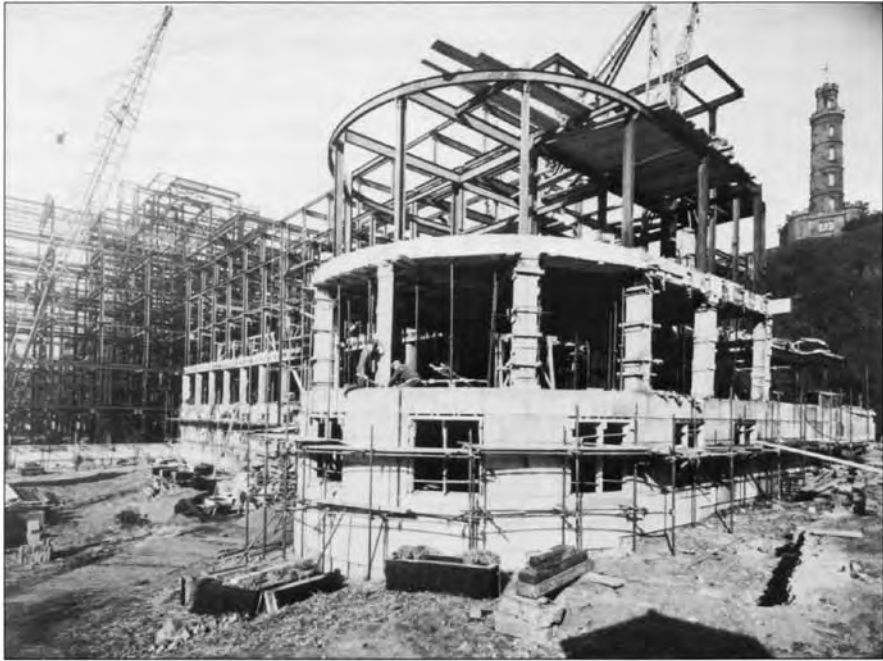
The east pavilion under construction, October 1937.
