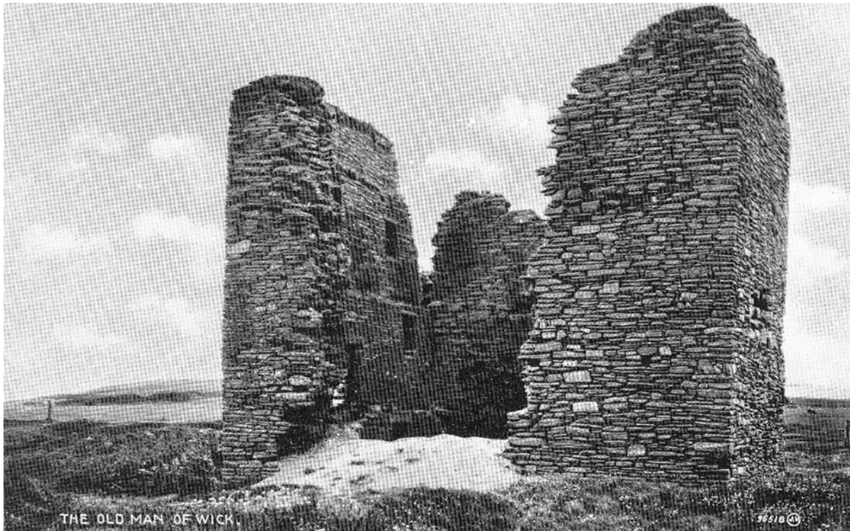
Figure 4: Postcard of Castle of Old Wick (c.1925), looking south-west towards the interior of the masonry tower, from the north-east. Note the presence of two small joist holes on the exterior face of the nearest wall (c.1/3 of the way up the wall), which do not all survive today. The degree of scarring on the tower's north-west face (on the far right here) is also more apparent than is evident today. © Courtesy of HES.
