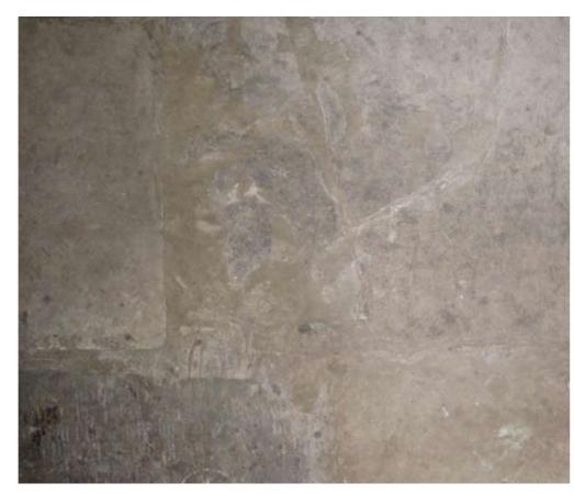
Historic impact damage showing subsequent repair
