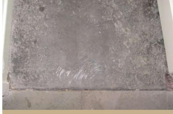
Repaired slab showing grinder marks and cement patching
