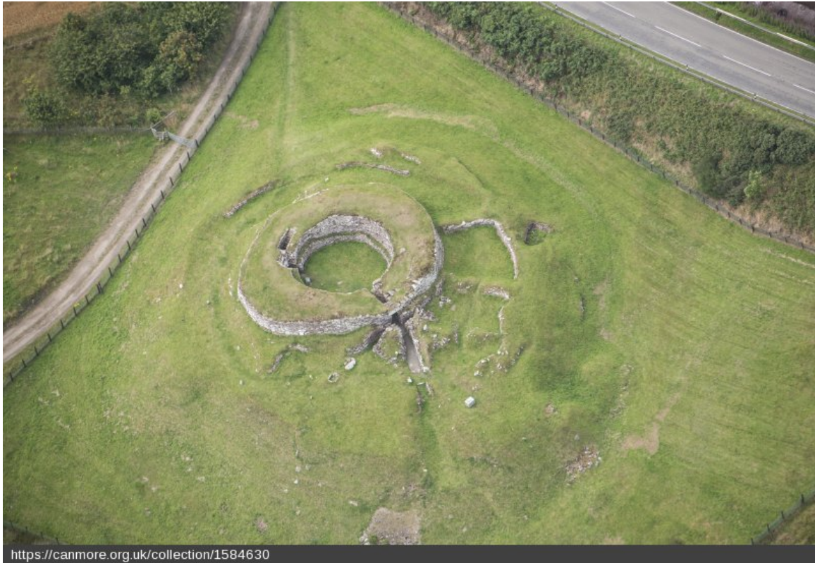
Aerial view, from east-south-east
