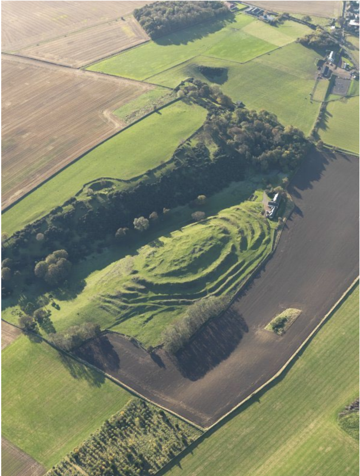
Figure 2: Aerial view from the north-east, showing the higher ground which overlooks the Chesters from the south. © Crown Copyright: HES.
