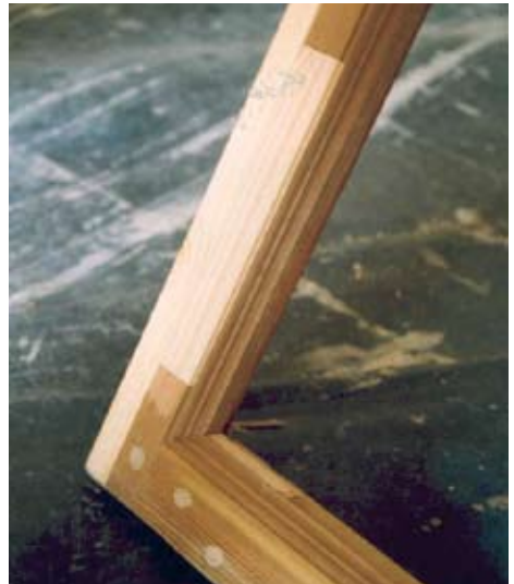
New timber can be used to replace rotten sections
