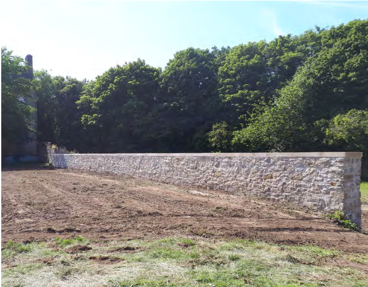
Figure 13. View of the completed wall, with the copes in place, summer 2018.
